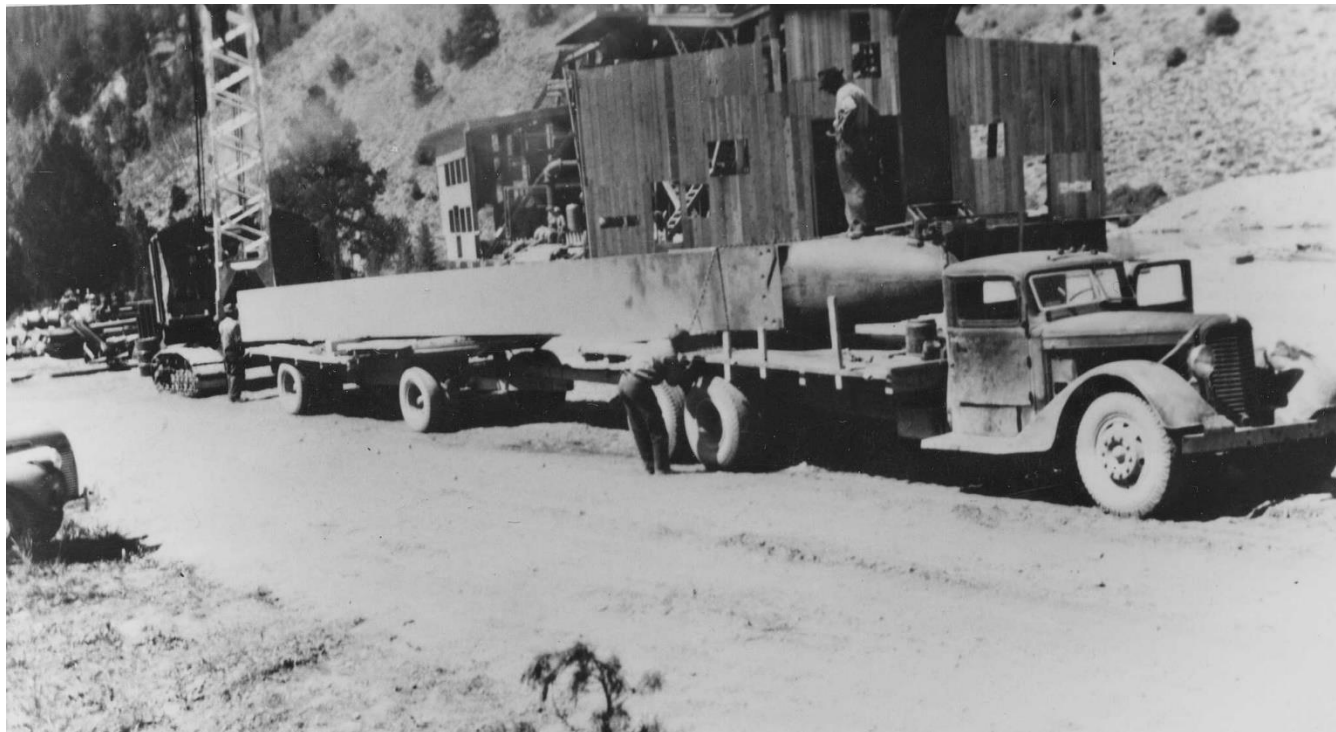
Figure 8: Spud delivery during construction of the Yankee Fork Gold Dredge, port and stern sides, 1940. Photo 2_4_1, courtesy of Yankee Fork Gold Dredge Archives, Land of the Yankee Fork State Park, Challis, Idaho.
