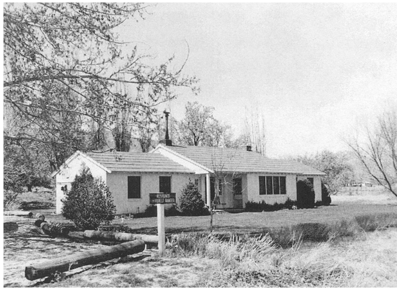
The Carson Ranger Station on the Humboldt-Toiyabe National Forest reflects the shift in design principles from the New Deal era to the post-war period.
