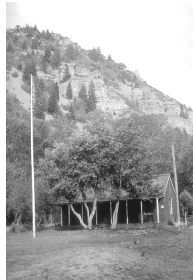
South Fork Ranger Station, Uinta National Forest.
