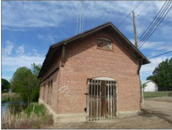
Institute Canal Pump House - located west of where State Street crosses the Galloway Ditch(NRHP Ref# 100000958)
