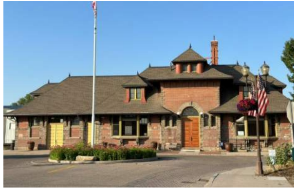
Weiser Train Depot - One State Street (NRHP Ref# 07000006)
