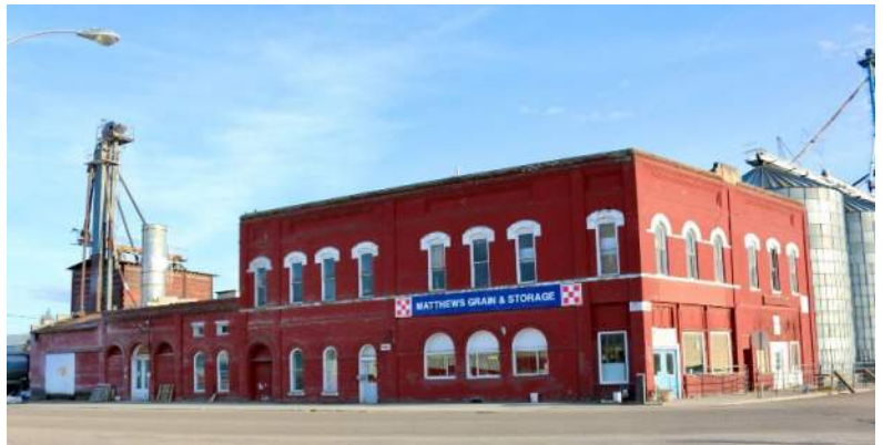
Werneth Building – 135 E Commercial Street
