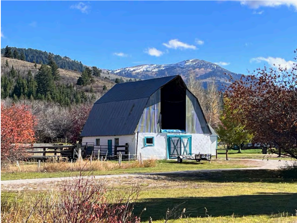
Figure 34. Historic barn in The String Area.
