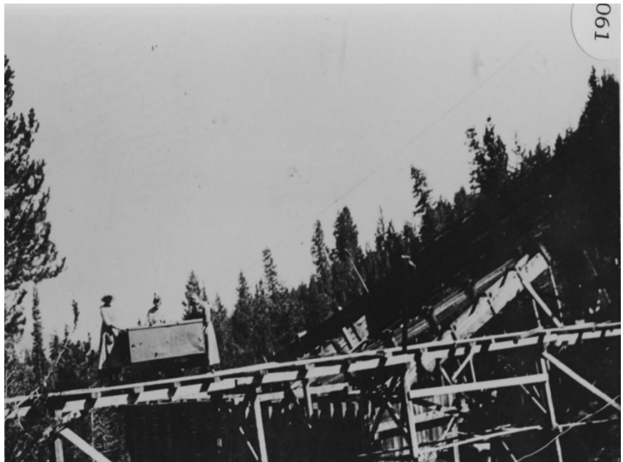
Figure 12. Trestle in Sam, Idaho, used for mining carts ca. 1920. Brigham Young University-Idaho, David O. McKay Library, Archive and Special Collections.
