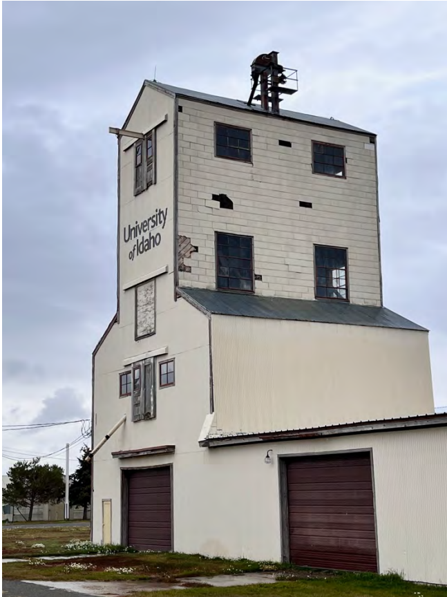
Figure 32. Elevator at Clementsville, now utilized by University of Idaho as the Teton Research and Extension Station.
