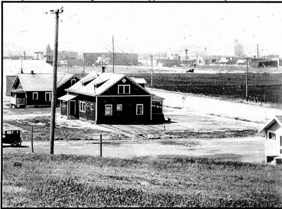
Late 1925 Photograph showing Sparks rear addition in place on extreme right of photo. View to the north overlooking the town square (Bureau of Reclamation Photograph).
