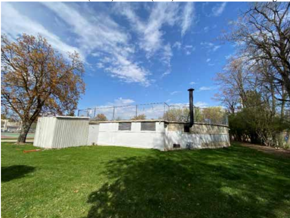
Photo 6: View of side (south) and rear (west) elevations. Camera facing northeast.
