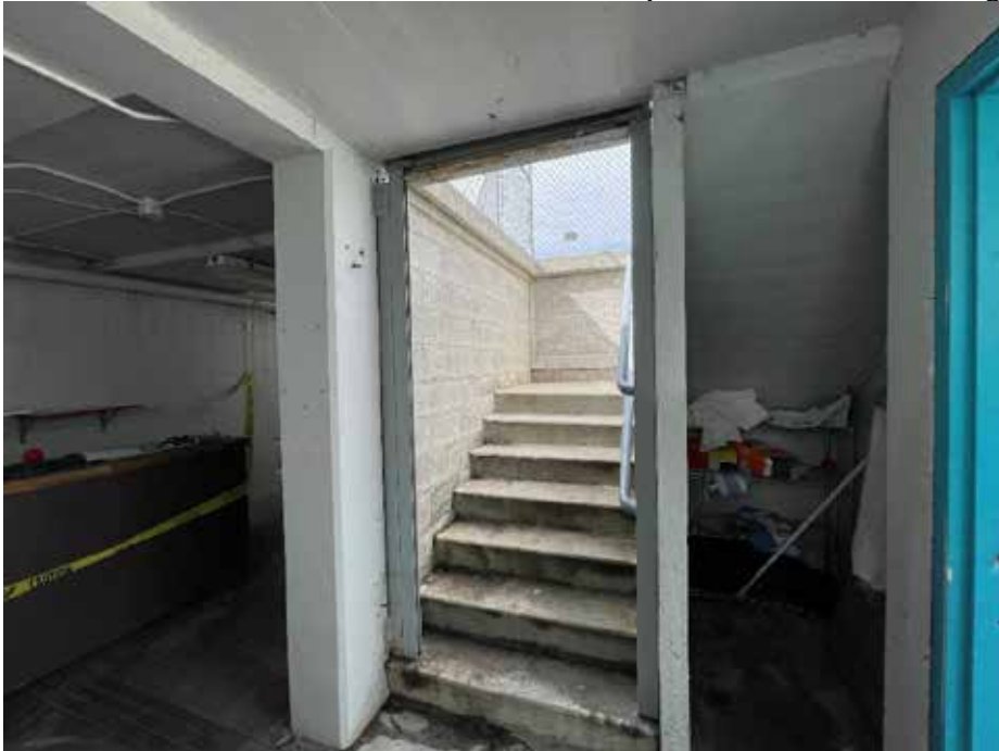
Photo 12: View of entrance vestibule stairs to pool deck. Camera facing north.
