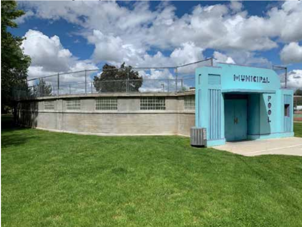
Photo 5: View of primary (east) and side (south) elevations. Camera facing northwest.
