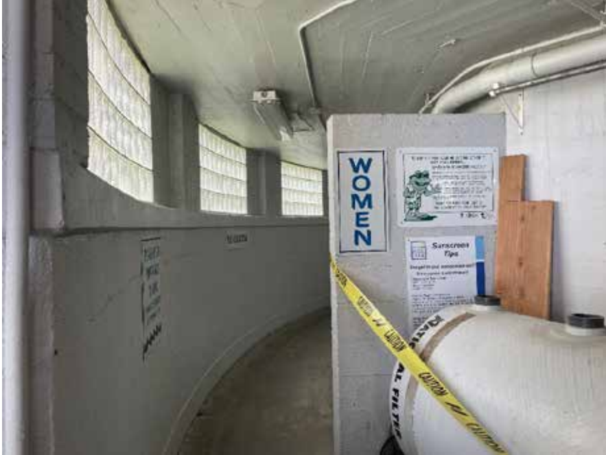
Photo 13: View from check-in lobby towards women's locker room. Camera facing south.
