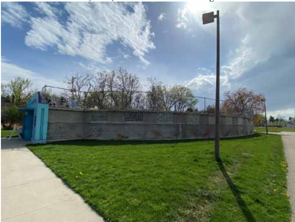
Photo 8: View of side (north) elevation. Camera facing southwest.
