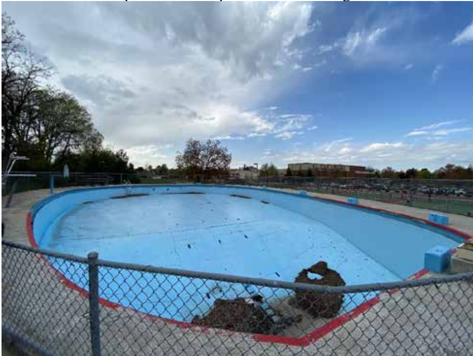
Photo 10: View of pool deck and pool. Camera facing northwest.
