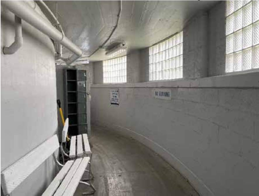
Photo 15: View of men's locker room. Camera facing west.
