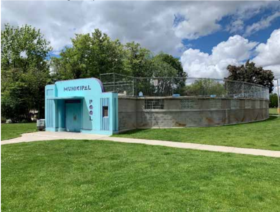
Photo 1: View of primary (east) and side (north) elevations. Camera facing southwest.
