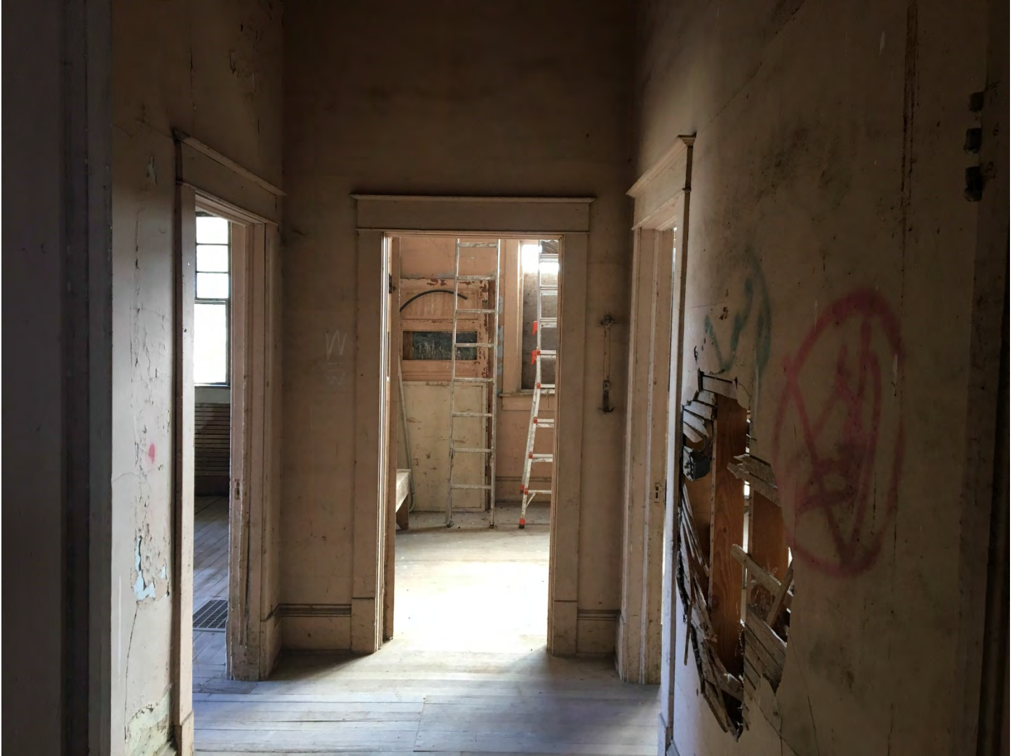
Photo 10 of 18: ID_TwinFallsCounty_RogersonSchool_0010 Interior, hallway, looking east
