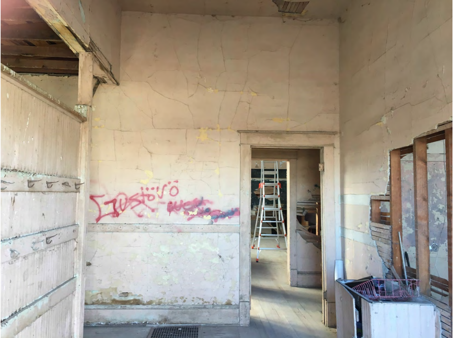
Photo 8 of 18: ID_TwinFallsCounty_RogersonSchool_0008 Interior, entrance foyer, looking south
