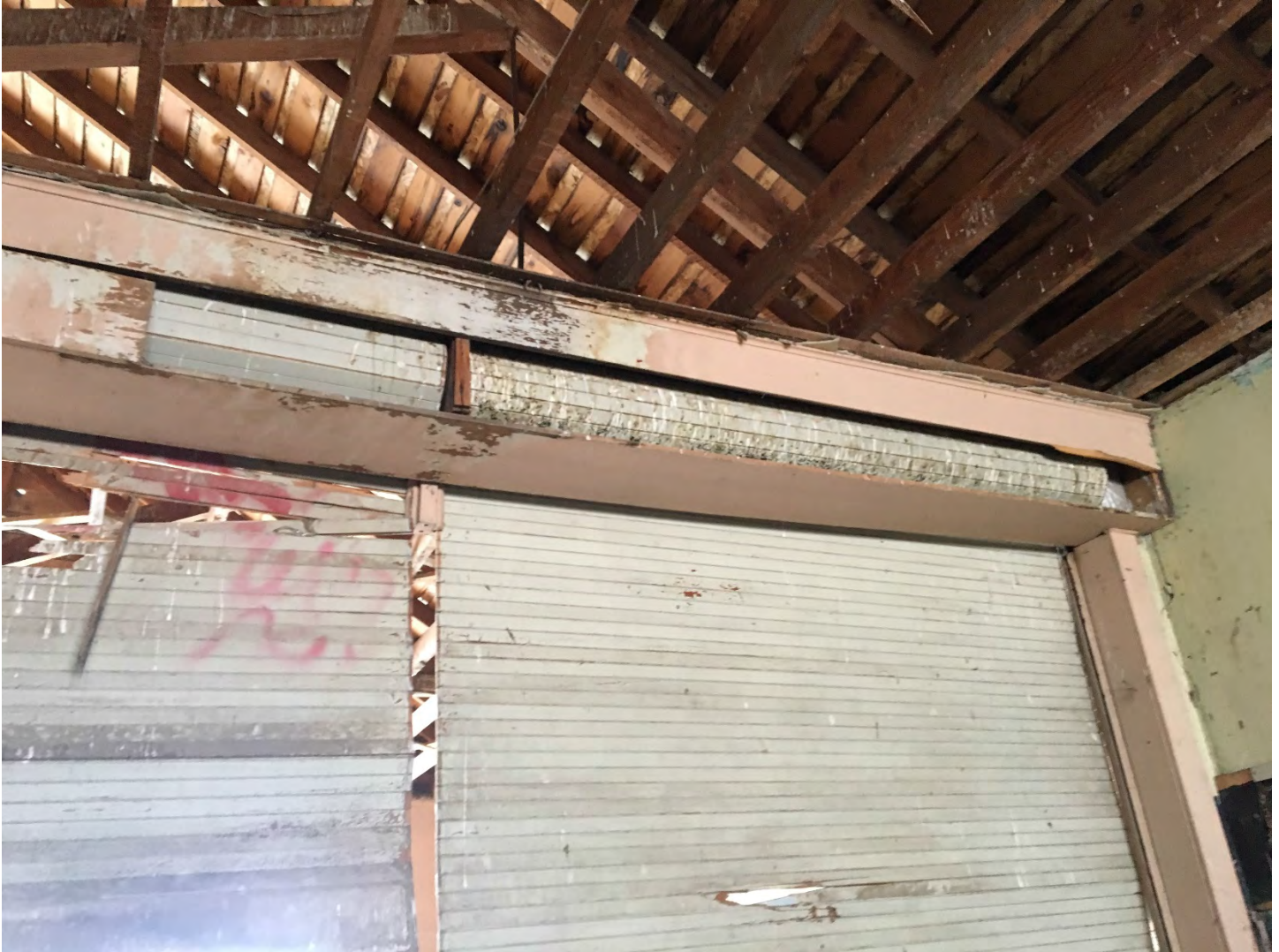
Photo 16 of 18: ID_TwinFallsCounty_RogersonSchool_0016 Interior, detail of classroom partition, looking east
