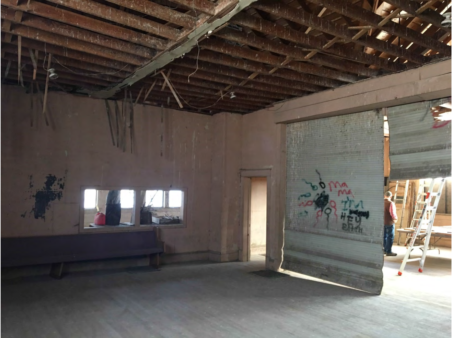
Photo 13 of 18: ID_TwinFallsCounty_RogersonSchool_0013 Interior, west classroom space, looking northeast
