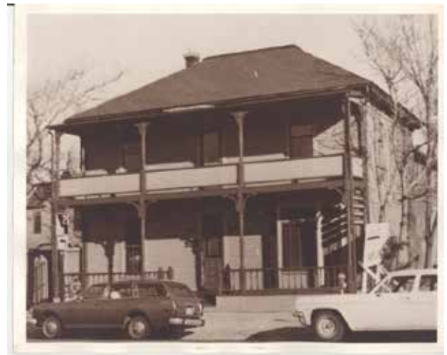
Star Rooming House, 1970s. See figure 12. Source: Basque Museum and Cultural Center Collection.
