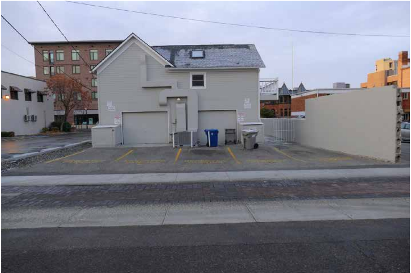
Photo 5. ID_AdaCounty_RobbinsHouse_0005.tif Rear (north) elevation, looking southwest
