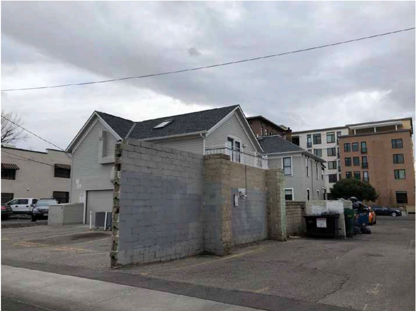
Photo 6. ID_AdaCounty_RobbinsHouse_0006.tif View from alleyway showing remains of fronton, looking south
