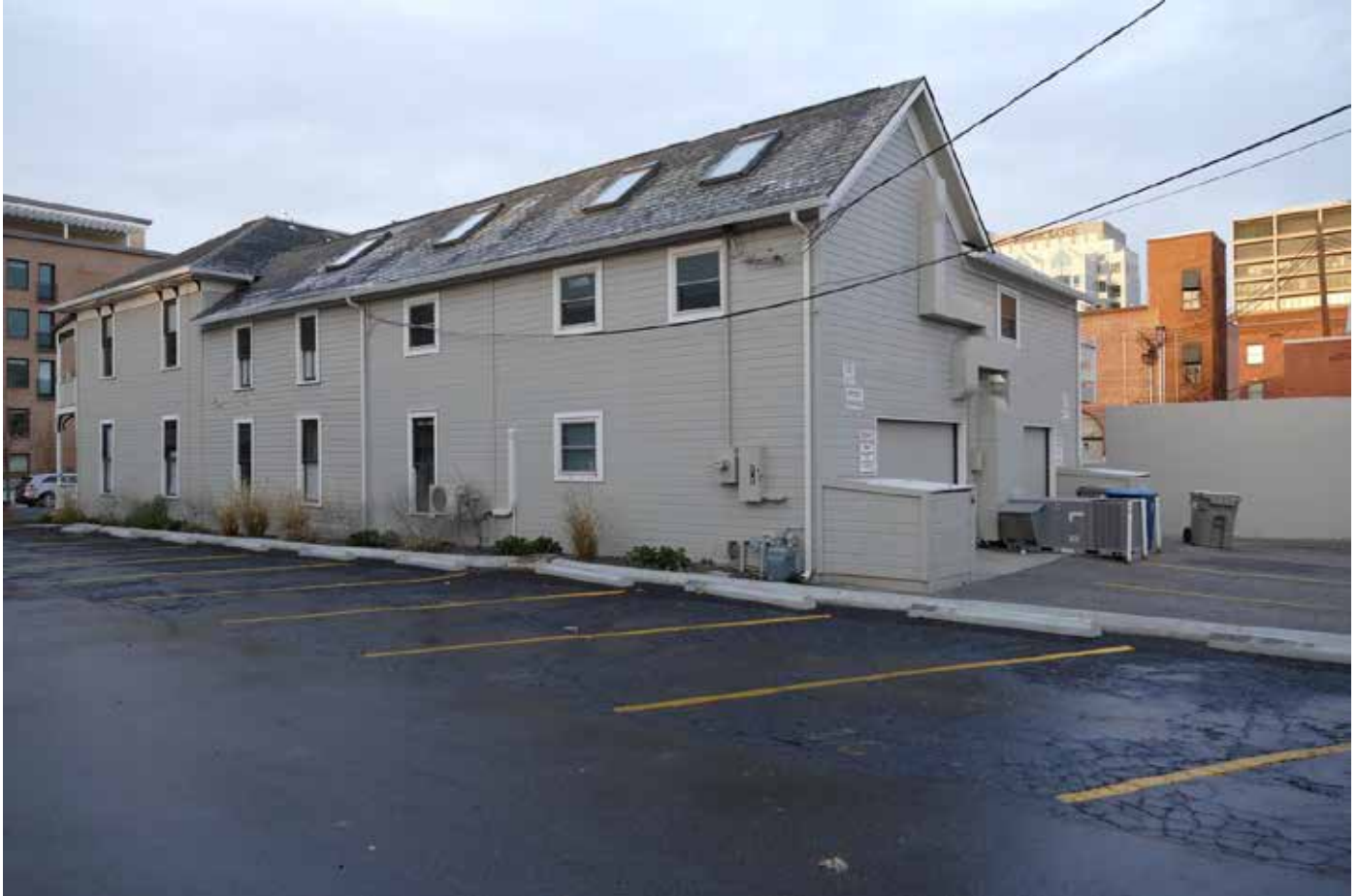
Photo 4. ID_AdaCounty_RobbinsHouse_0004.tif Rear (north) and east elevations, looking west
