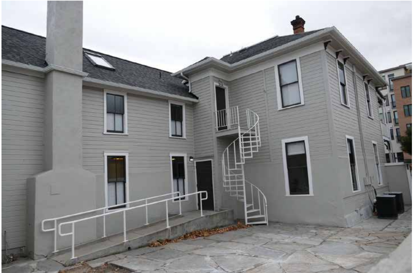
Photo 8. ID_AdaCounty_RobbinsHouse_0008.tif Partial view of west elevation, with spiral staircase at the center, looking south
