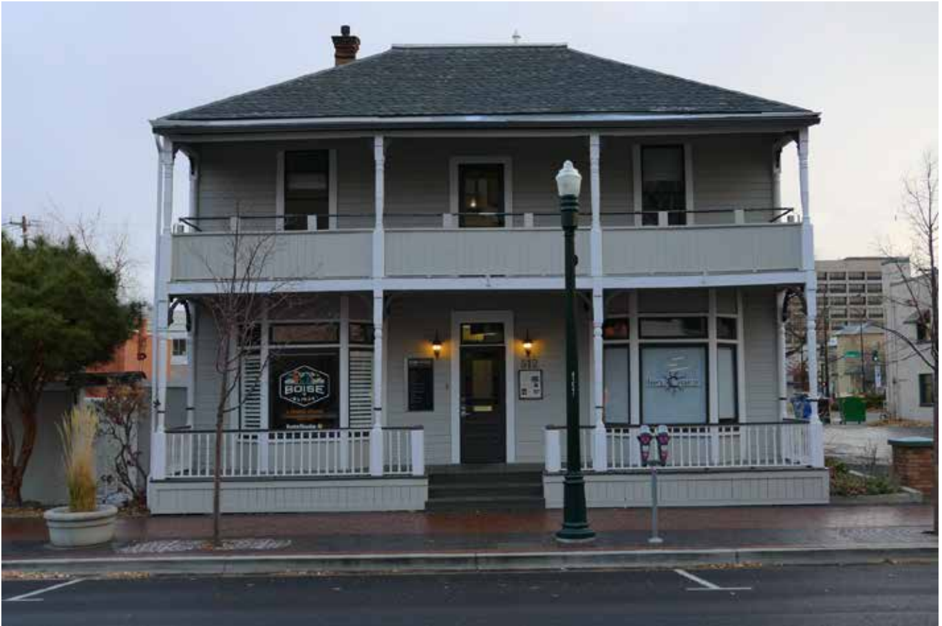
Photo 2. ID_AdaCounty_RobbinsHouse_0002.tif Primary (south) elevation, looking northeast
