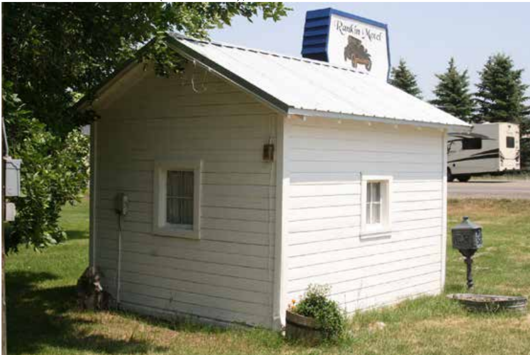
Photo 32: Office Cabin (resource 12), view of west and south elevations. Camera facing northeast.
