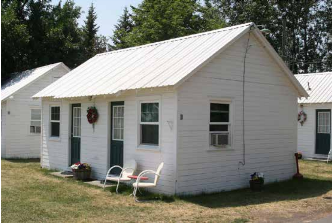
Photo 12: Cottage 3 (resource 3), view of east and north elevations. Camera facing southwest.
