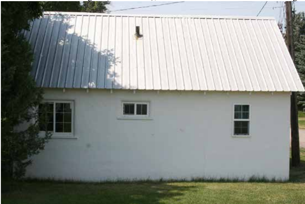
Photo 34: Stucco Cottage 1 (resource 13), view of east elevation. Camera facing west.
