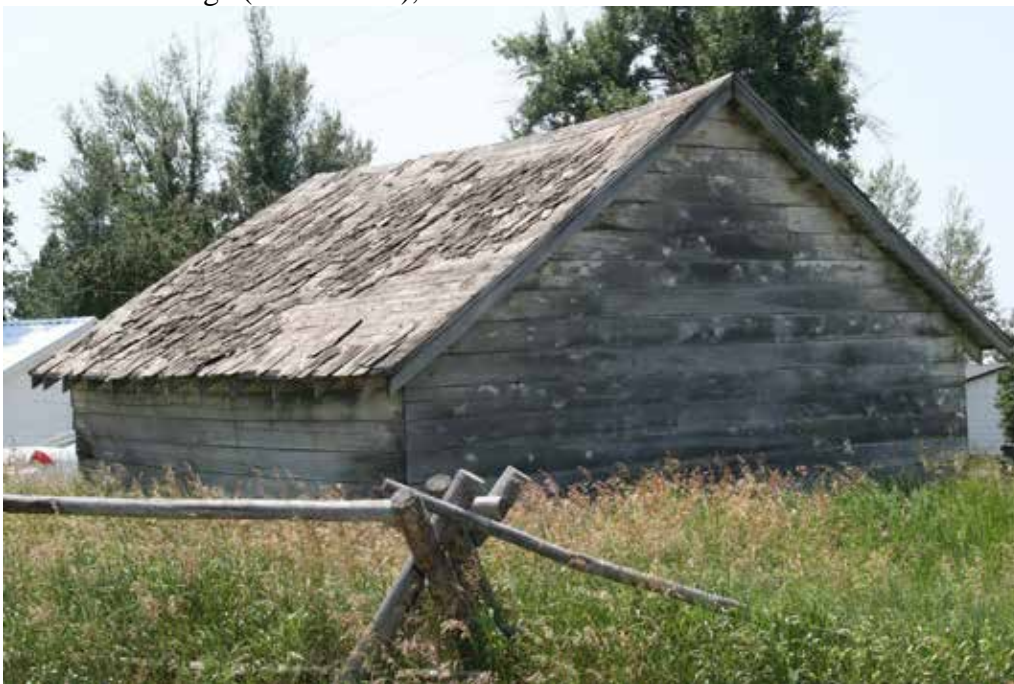
Photo 29: Garage (resource 10), view of east and north elevations. Camera facing southwest.
