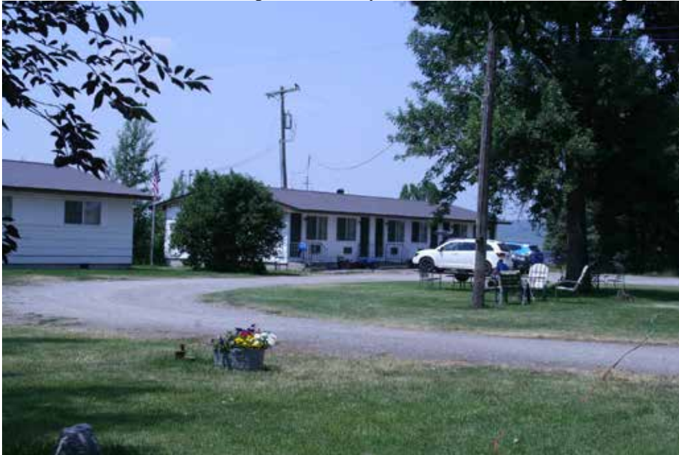
Photo 3: View across U-Shaped Driveway (resource 1), Camera facing northwest.
