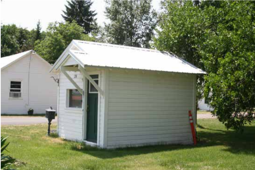
Photo 31: Office Cabin (resource 12), view of east and north elevations. Camera facing southwest.
