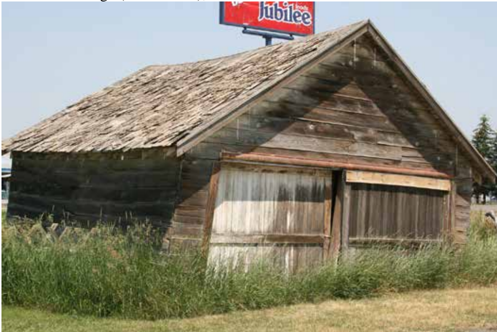
Photo 28: Garage (resource 10), view of west and south elevations. Camera facing northeast.
