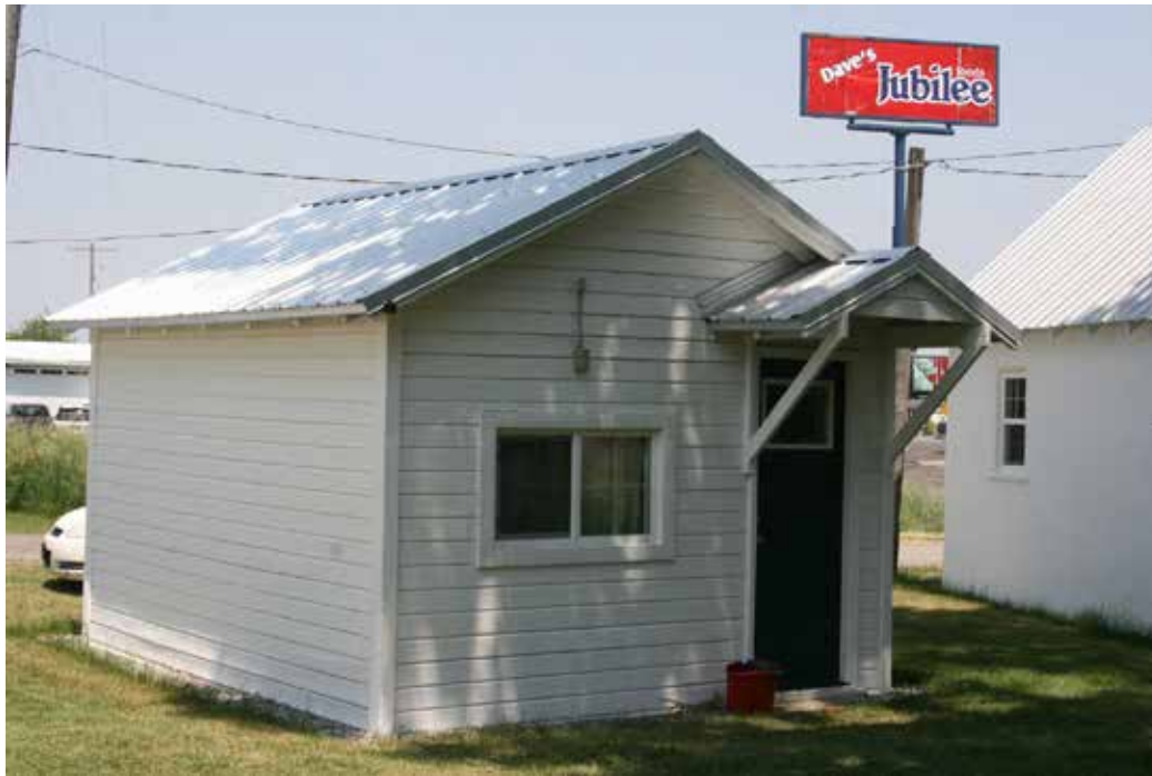
Photo 38: Laundry Room Cabin (resource 15), view of west and south elevations. Camera facing northeast.
