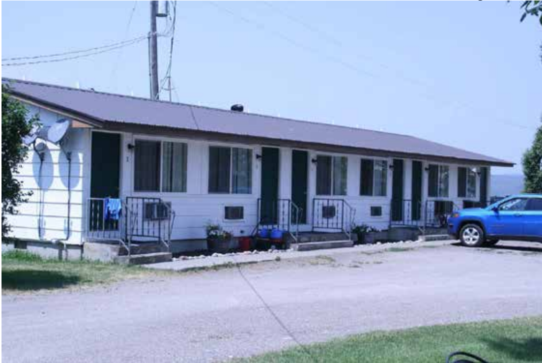
Photo 24: Motor Court (resource 9), view of east elevation. Camera facing northwest.
