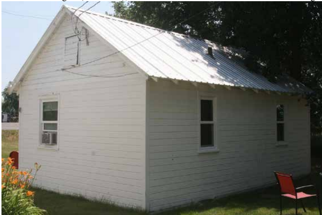
Photo 11: Cottage 4 (resource 2), view of north and west elevations. Camera facing southeast.
