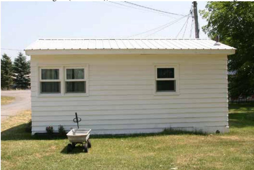
Photo 17: Cottage 6 (resource 5), view of west elevation. Camera looking east.
