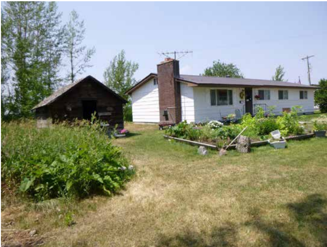
Photo 20: Ranch House/Motel Office (resource 8), view of south and east elevations. Camera facing northwest.
