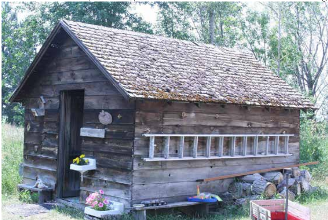
Photo 19: Woodshed (resource 7), view of east and north elevations. Camera facing southwest.
