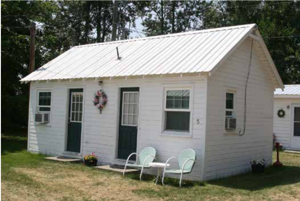
Photo 14: Cottage 5 (resource 4), view of east and north elevations. Camera facing southwest.
