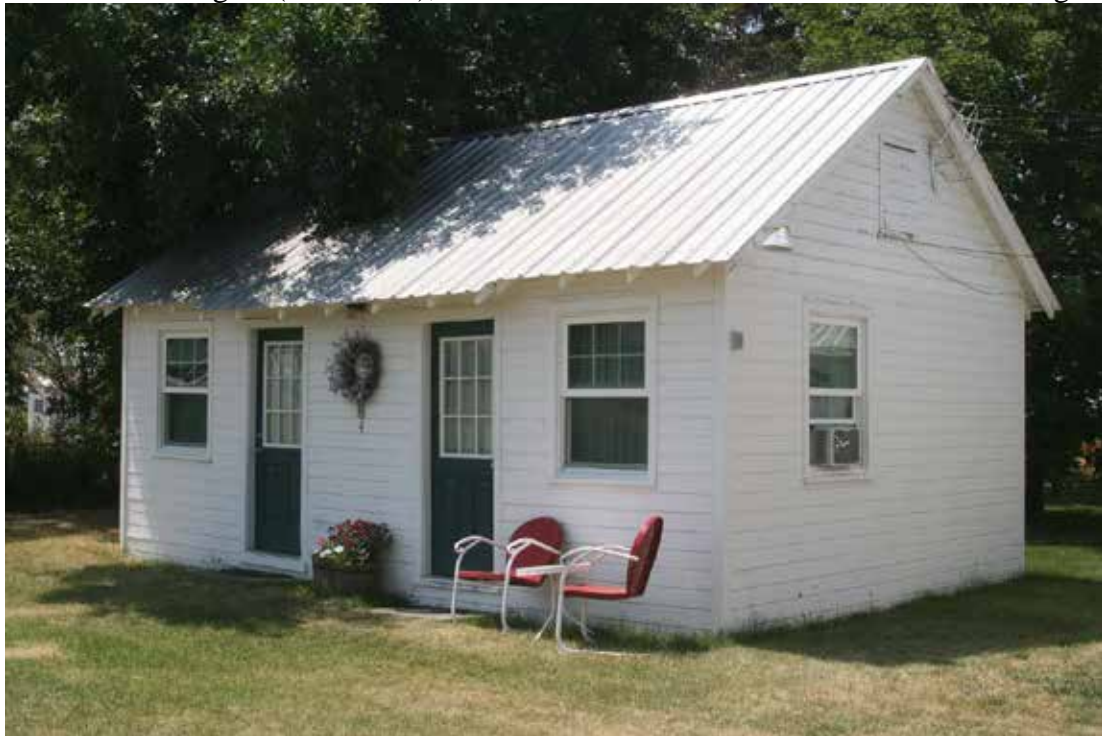
Photo 10: Cottage 4 (resource 2), view of east and north elevations. Camera facing southwest.
