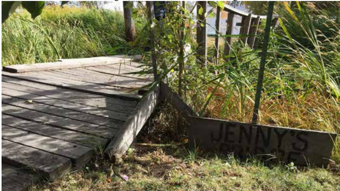
Photo 18: View of Footbridge (resource 6). Camera facing southeast.
