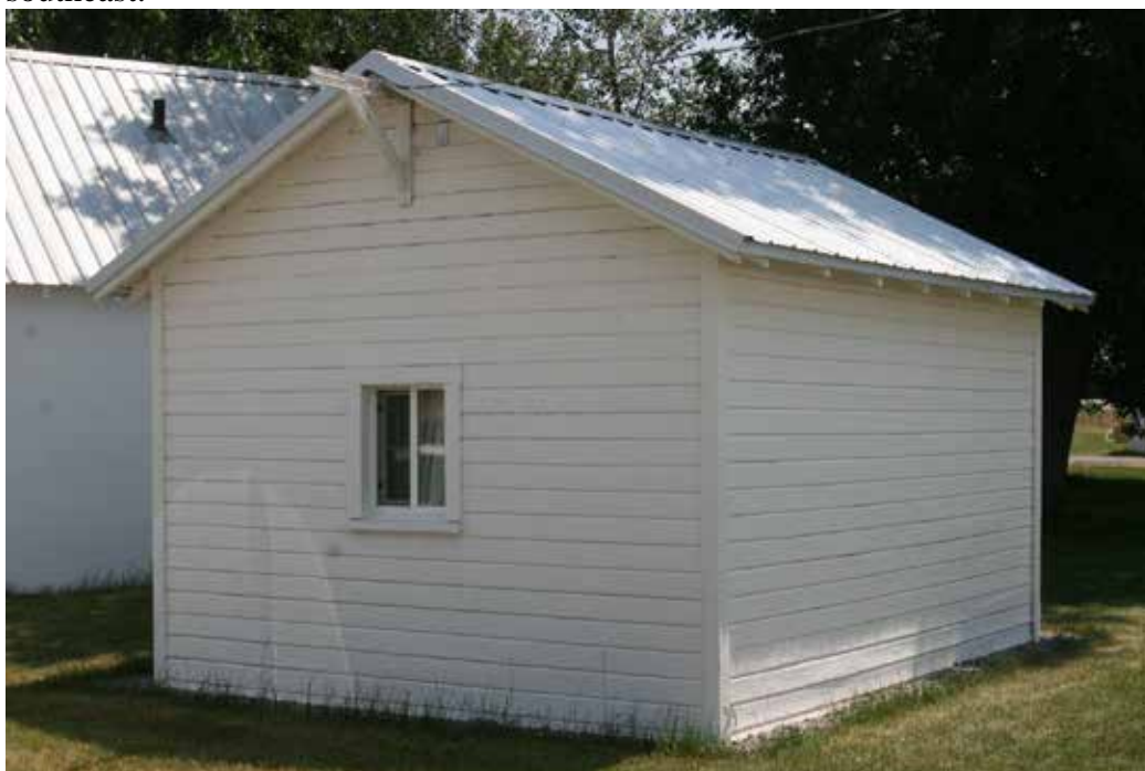
Photo 39: Laundry Room Cabin (resource 15), view of north and west elevations. Camera facing southeast.
