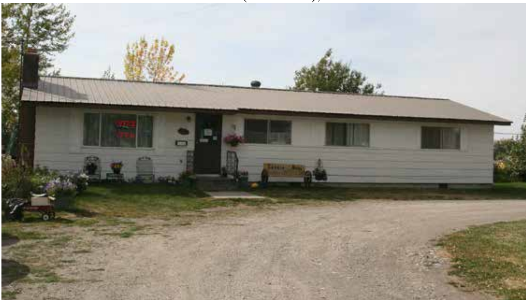
Photo 21: Ranch House/Motel Office (resource 8), view of east elevation. Camera facing west.
