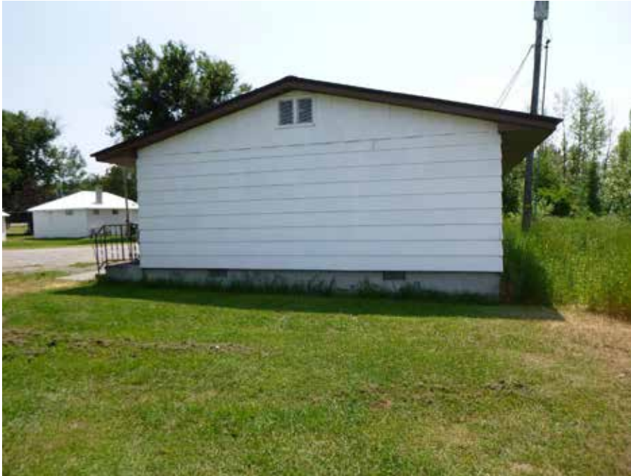
Photo 26: Motor Court (resource 9), view of north elevation. Camera facing south.
