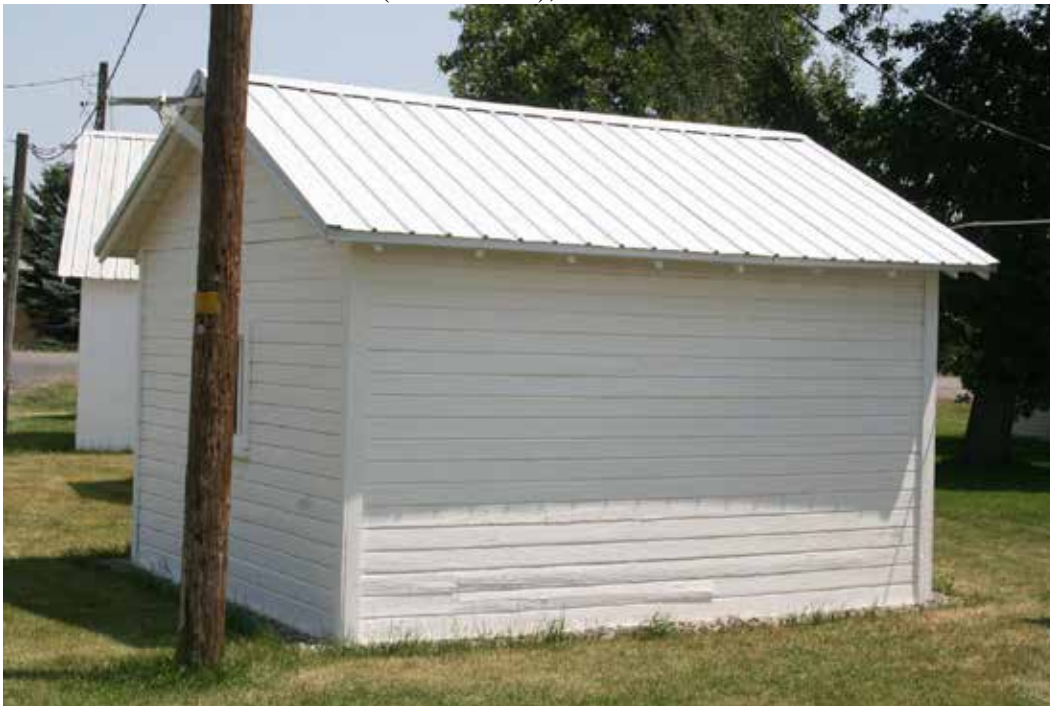
Photo 41: Pool Room Cabin (resource 16), view of north and west elevations. Camera facing southeast.
