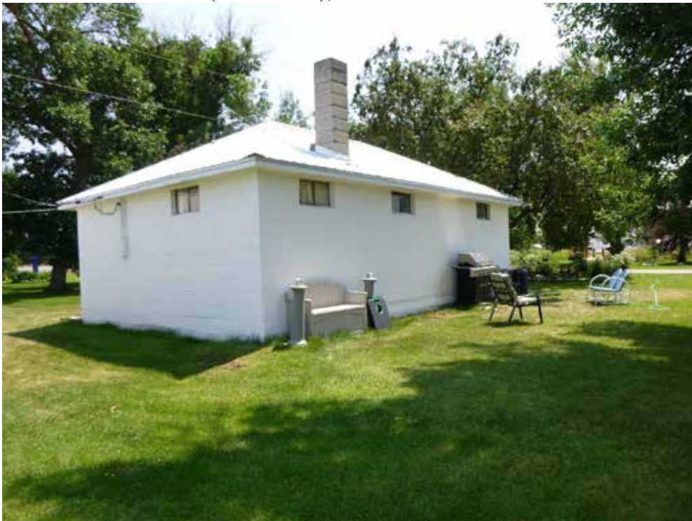
Photo 43: Washhouse (resource 17), view of north and west elevations. Camera facing southeast.
