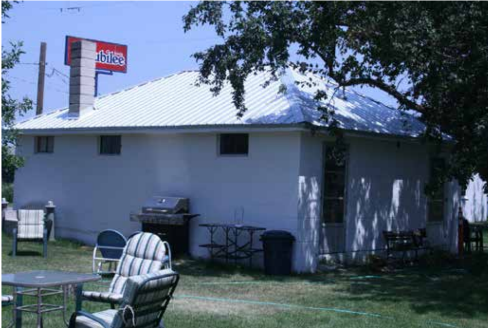
Photo 42: Washhouse (resource 17), view of west and south elevations. Camera facing northeast.
