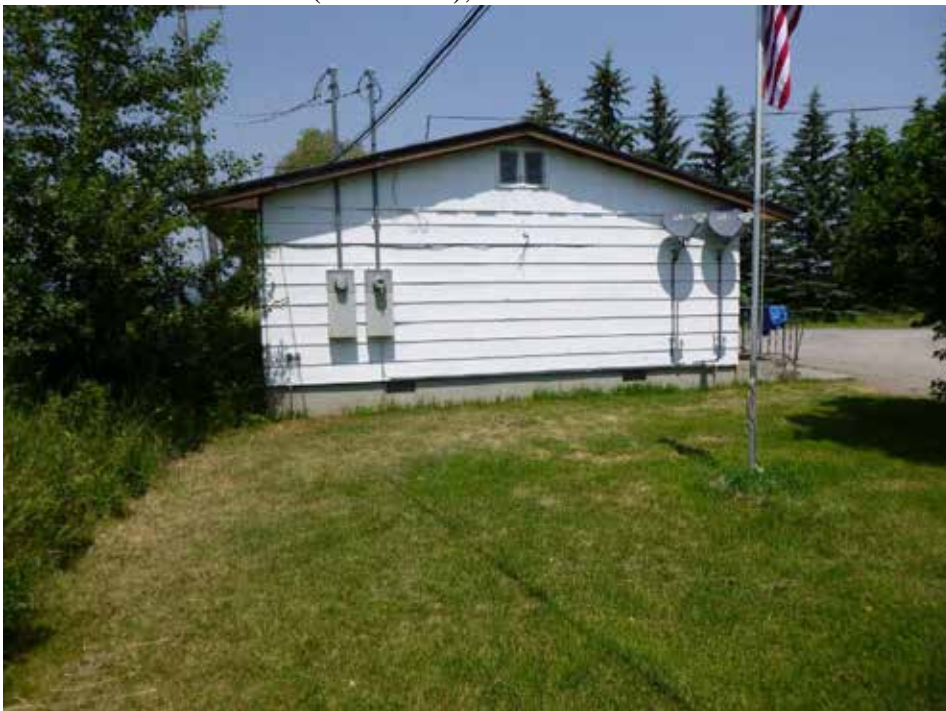
Photo 25: Motor Court (resource 9), view of south elevation. Camera facing north.
