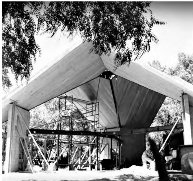
Figure 4 Photograph taken during construction in 1958, showing construction of roof structure containing the truss deck system. 14 Also depicted are corner walls which feature the building's three entrances. These structures remain in place today unaltered from original construction.
