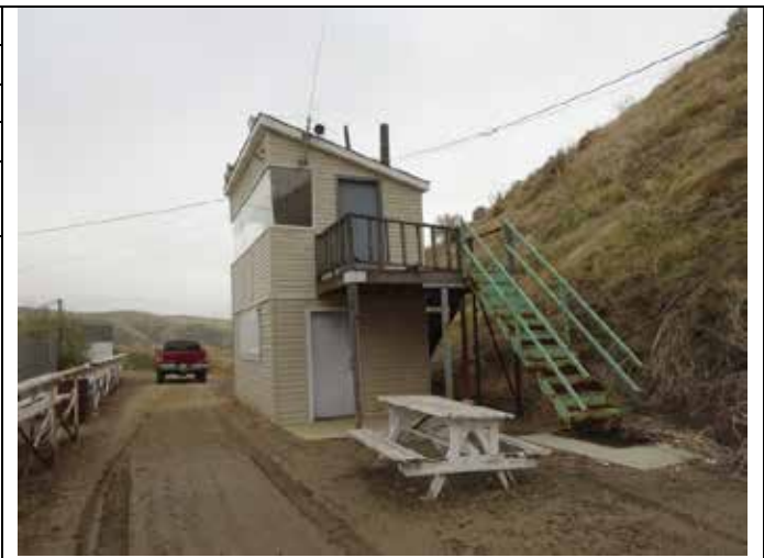
Photo: This image shows the north side of the press box (camera facing south).
