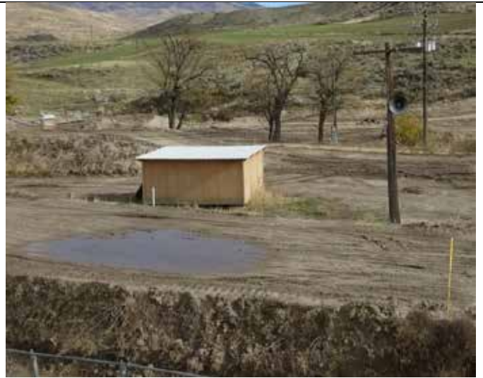
Photo: The photograph shows the north side of the pumphouse (camera facing southeast).
