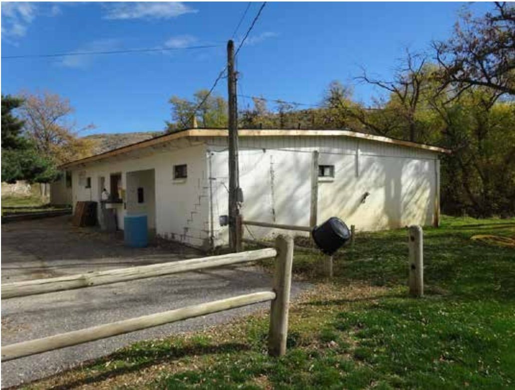
Photo 13. Northwest corner of clubhouse, facing SE
