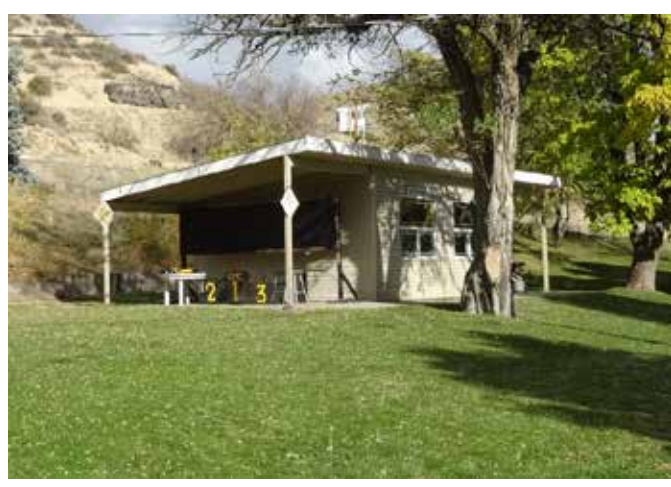
Photos: The top photo shows the primary south elevation of the concessions building (camera facing north). The bottom photo shows southwest corner of the concessions building (camera facing northeast).
