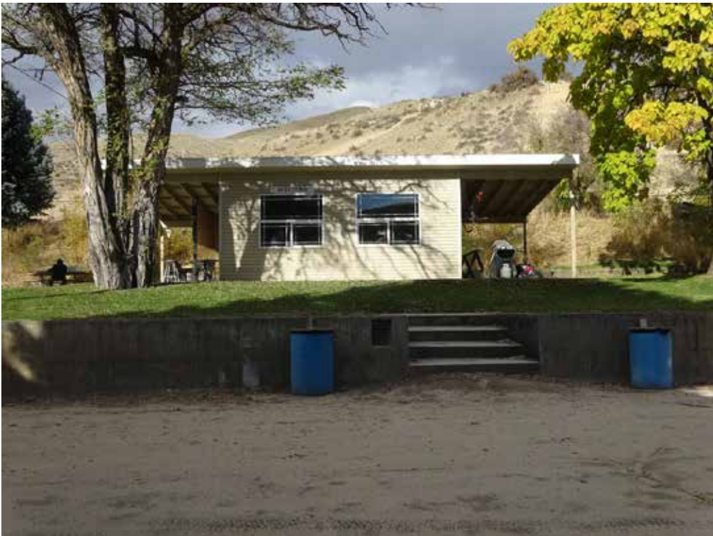
Photo 16. Concessions building, facing N
