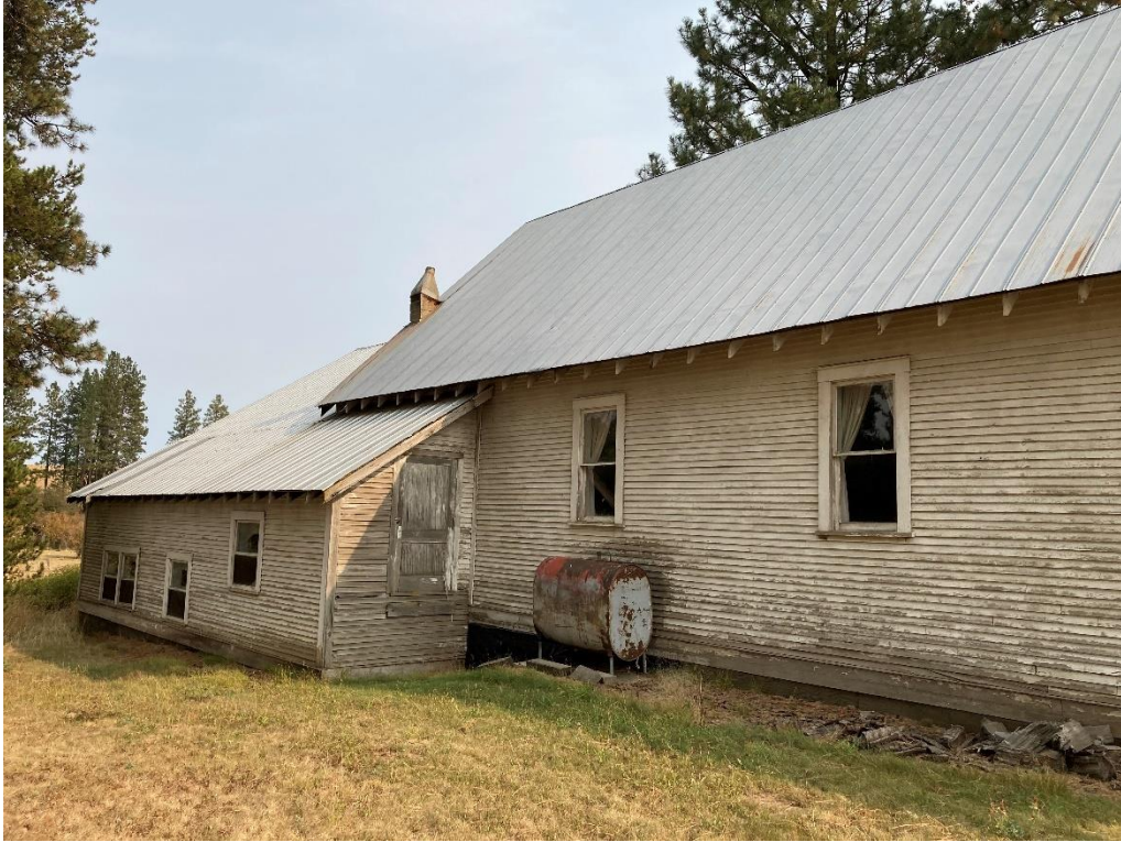
Photo 7. Side (northwest) elevation, facing east.
