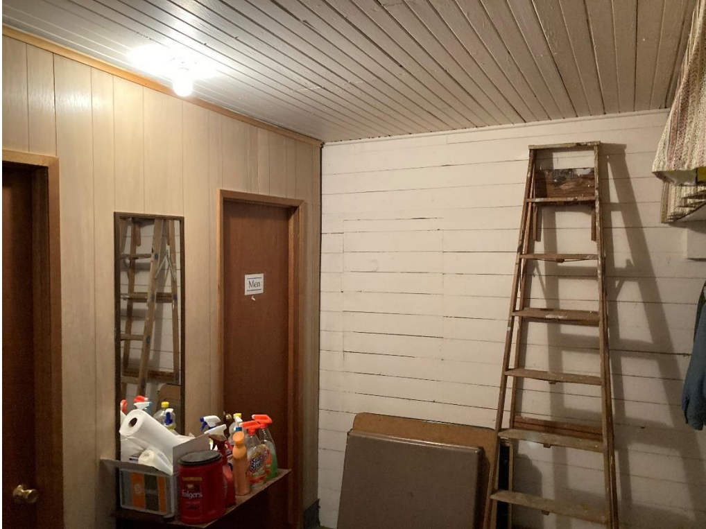
Photo 17. Front anteroom addition, coatroom, facing south.
