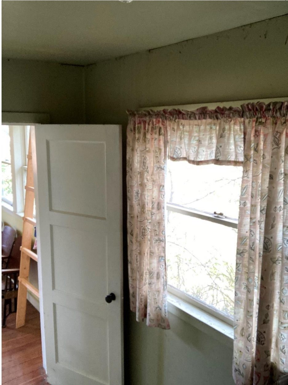
Photo 46. Rear addition juvenile grange coatroom, facing east.
