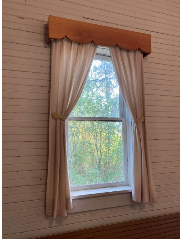
Photo 30. Main hall, wood double-hung window and valance, facing southeast.
