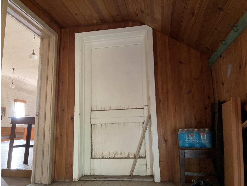
Photo 50. Rear addition basement stairwell, facing southwest.
