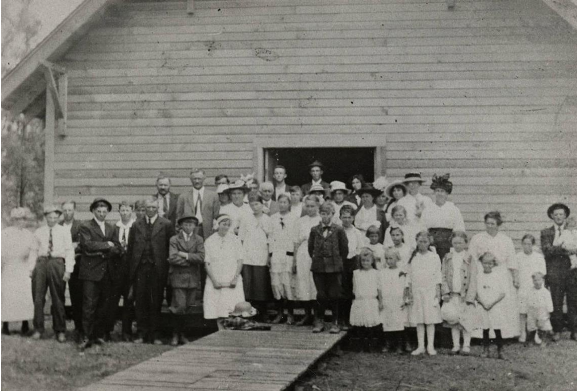
Figure 1. View of front elevation, 1935, facing northeast.
