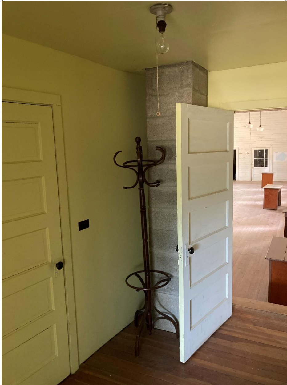
Photo 36. Rear addition, juvenile grange hall anteroom, facing southwest.
