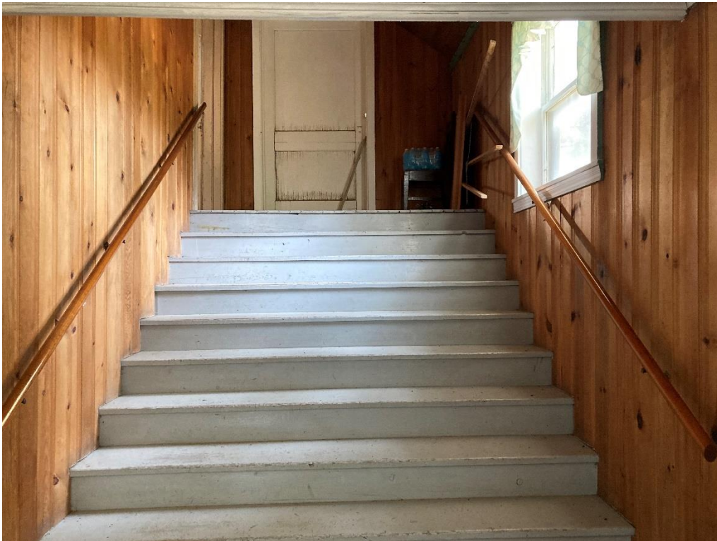
Photo 51. Rear addition basement stairwell, facing southwest.
