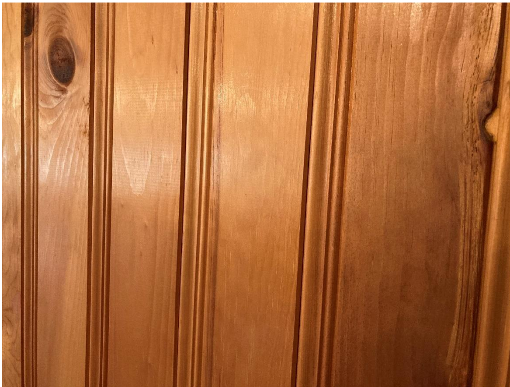
Photo 33. Main hall, knotty pine siding on inset stage, facing north.
