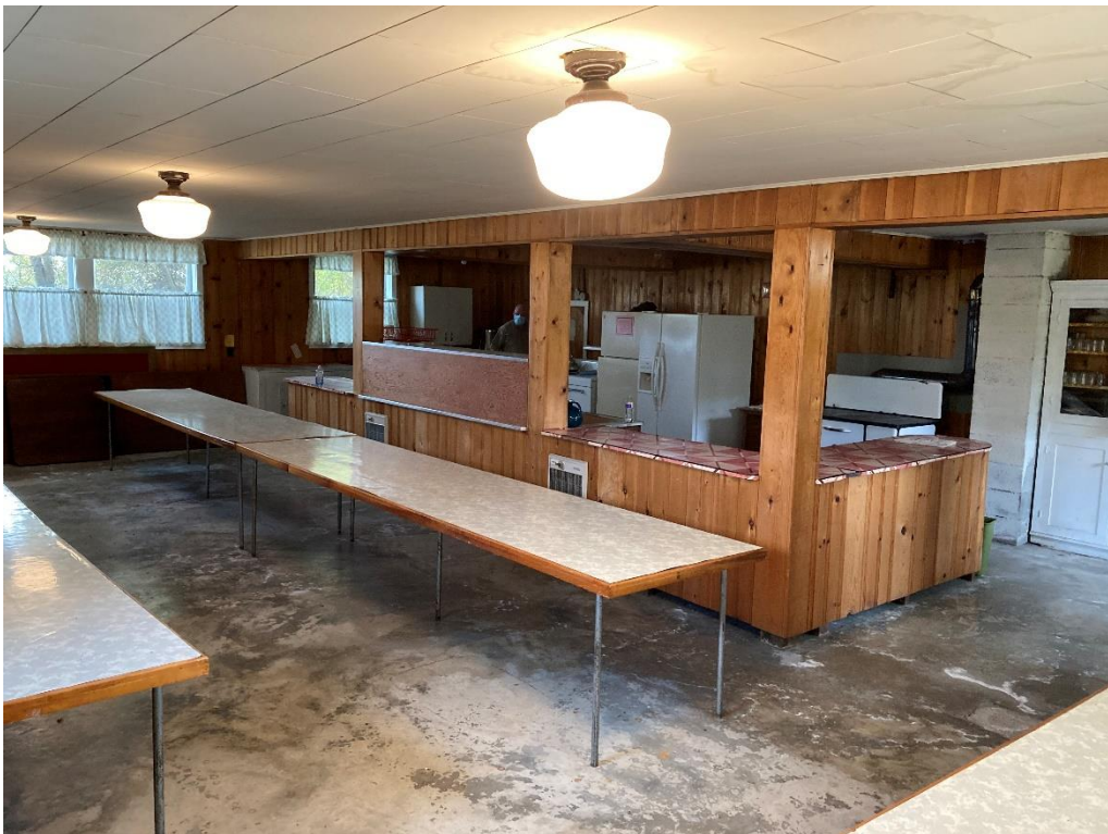
Photo 57. Rear addition basement kitchen/dining room, facing southeast.
