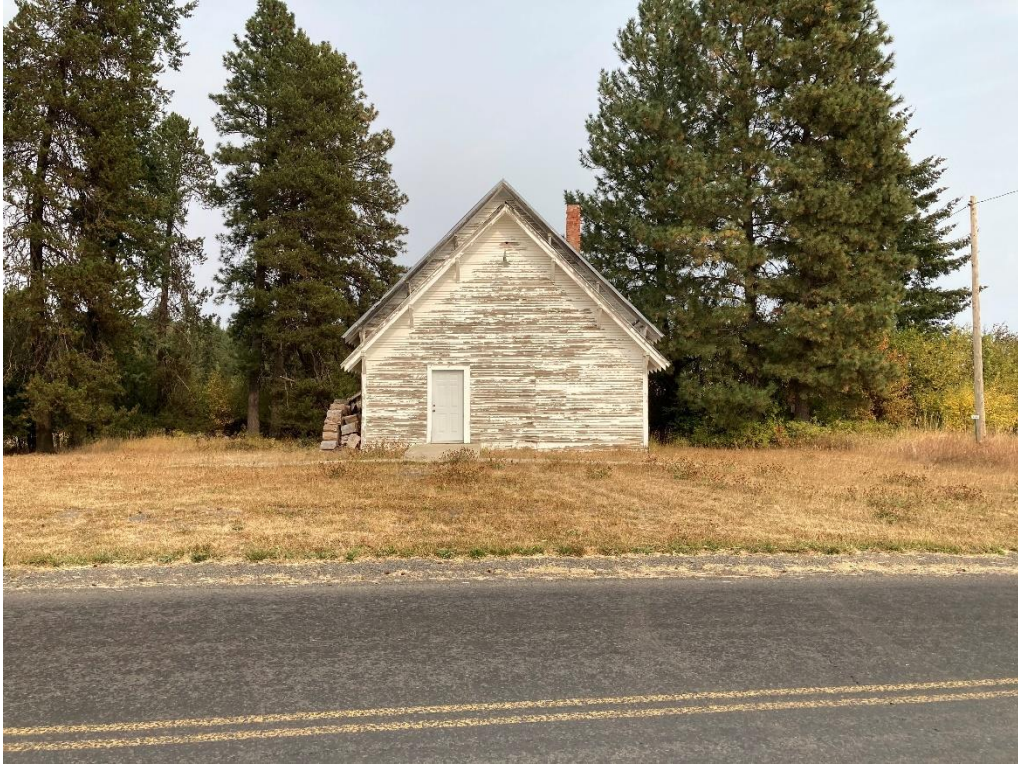
Photo 3. Front elevation and setting, facing northeast.
