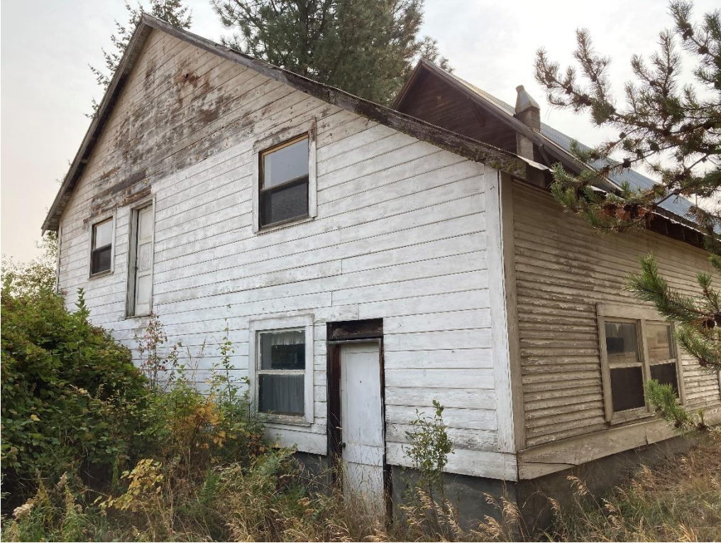
Photo 9. Rear and side (northwest) elevations, facing south.
