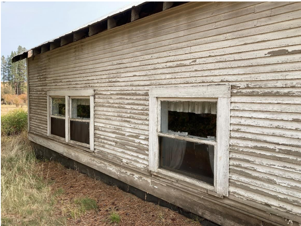
Photo 8. Rear addition, side (northwest) elevation, facing east.
