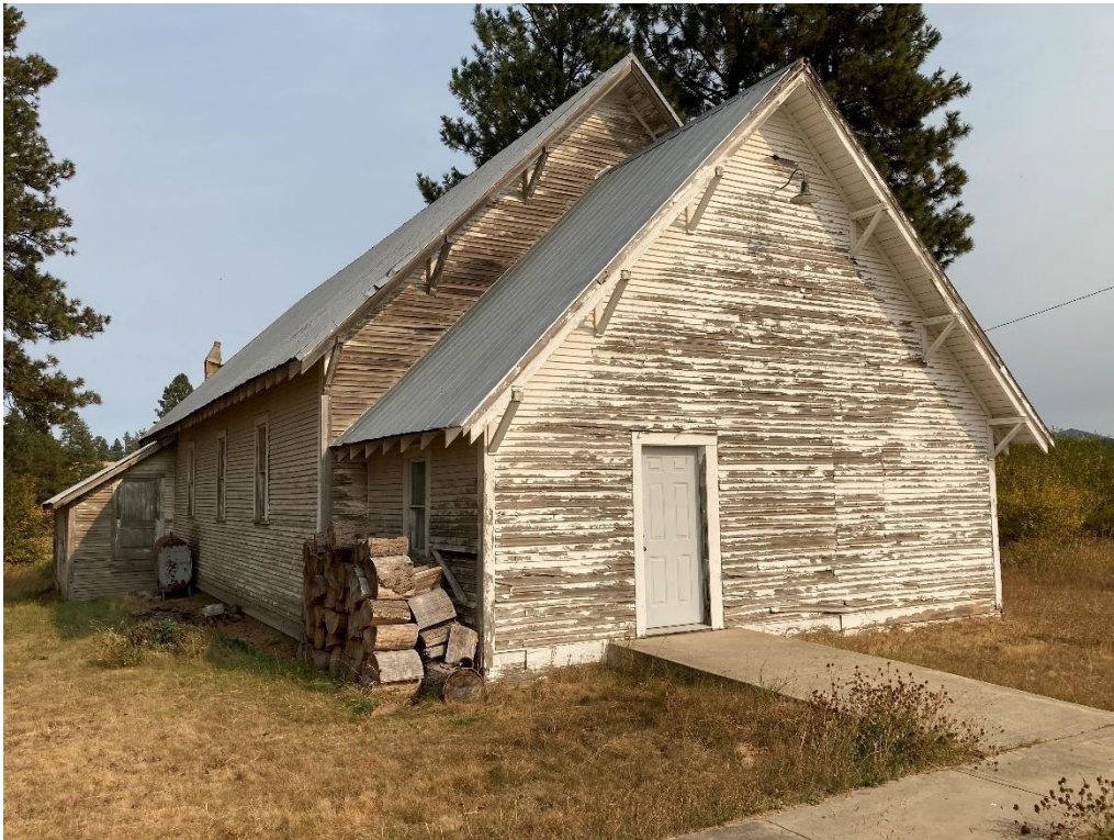
Photo 2. Front elevation with setting, facing northeast.
