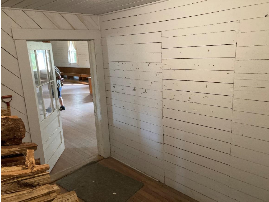
Photo 13. Front anteroom addition, foyer, facing east.
