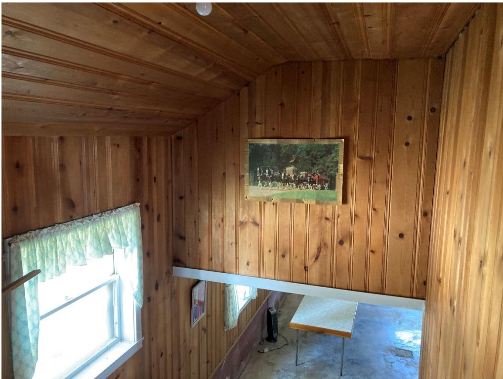
Photo 49. Rear addition basement stairwell, facing northeast.
