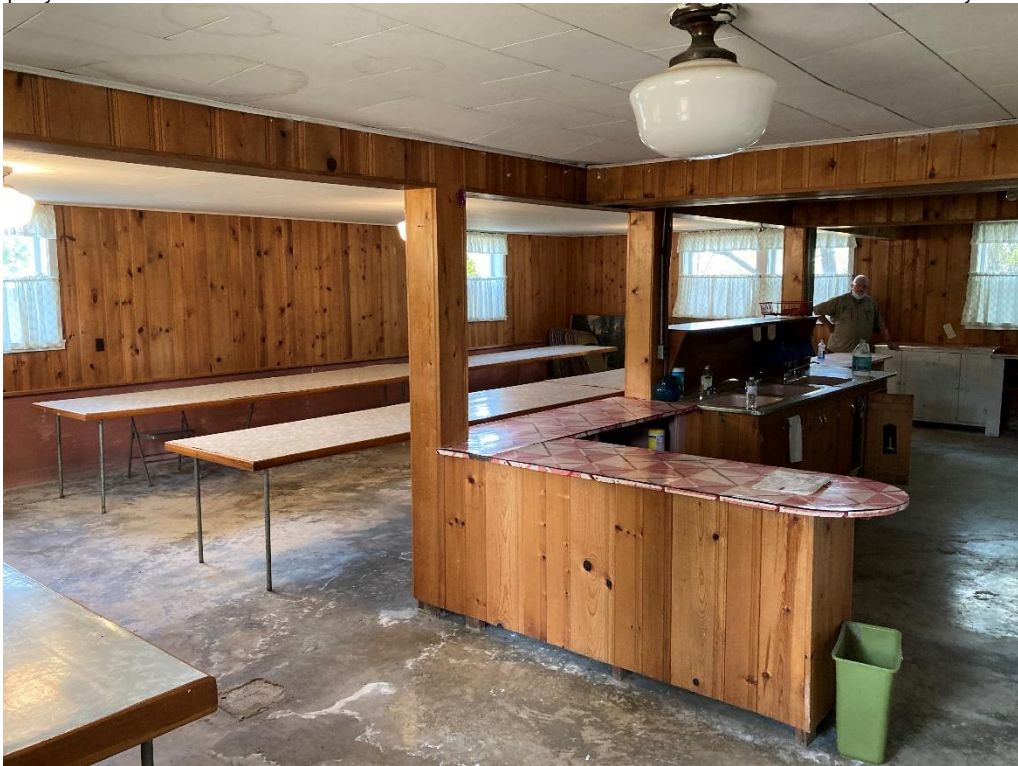
Photo 52. Rear addition basement kitchen/dining room, facing east.
