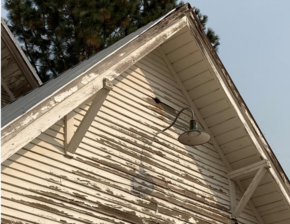
Photo 5. Front anteroom addition, with barn light and attic vent, facing northeast.
