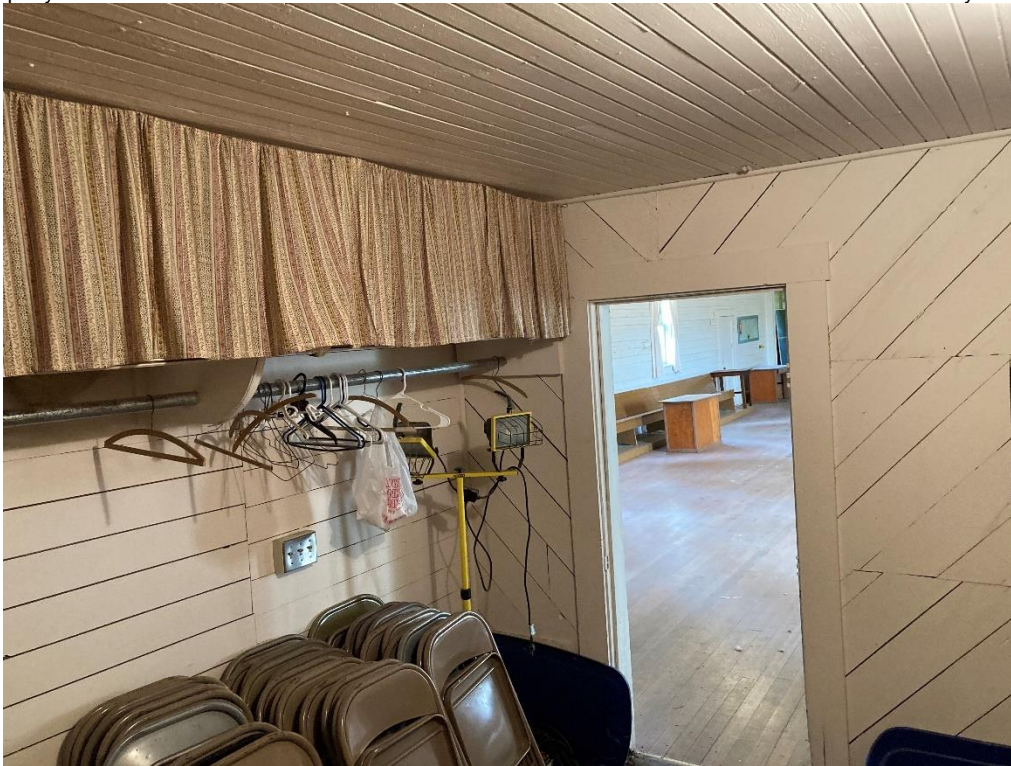
Photo 19. Front anteroom addition, coatroom, facing north.
