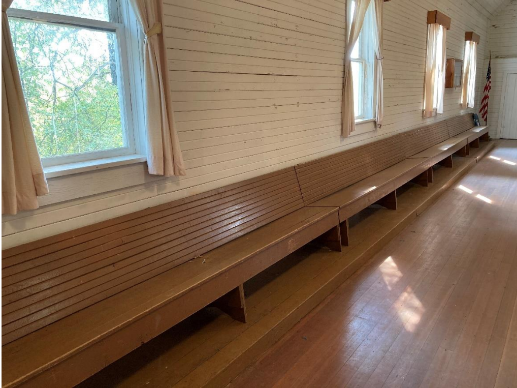
Photo 28. Main hall, wood pews, facing south.
