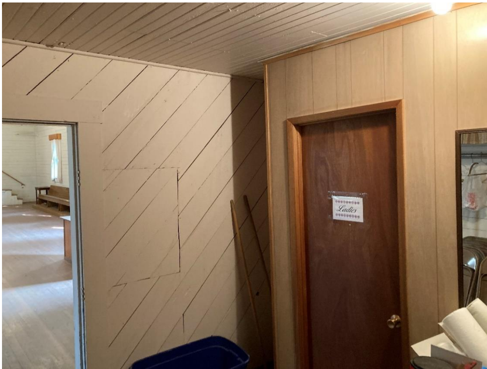
Photo 20. Front anteroom addition, coatroom and restrooms, facing east.
