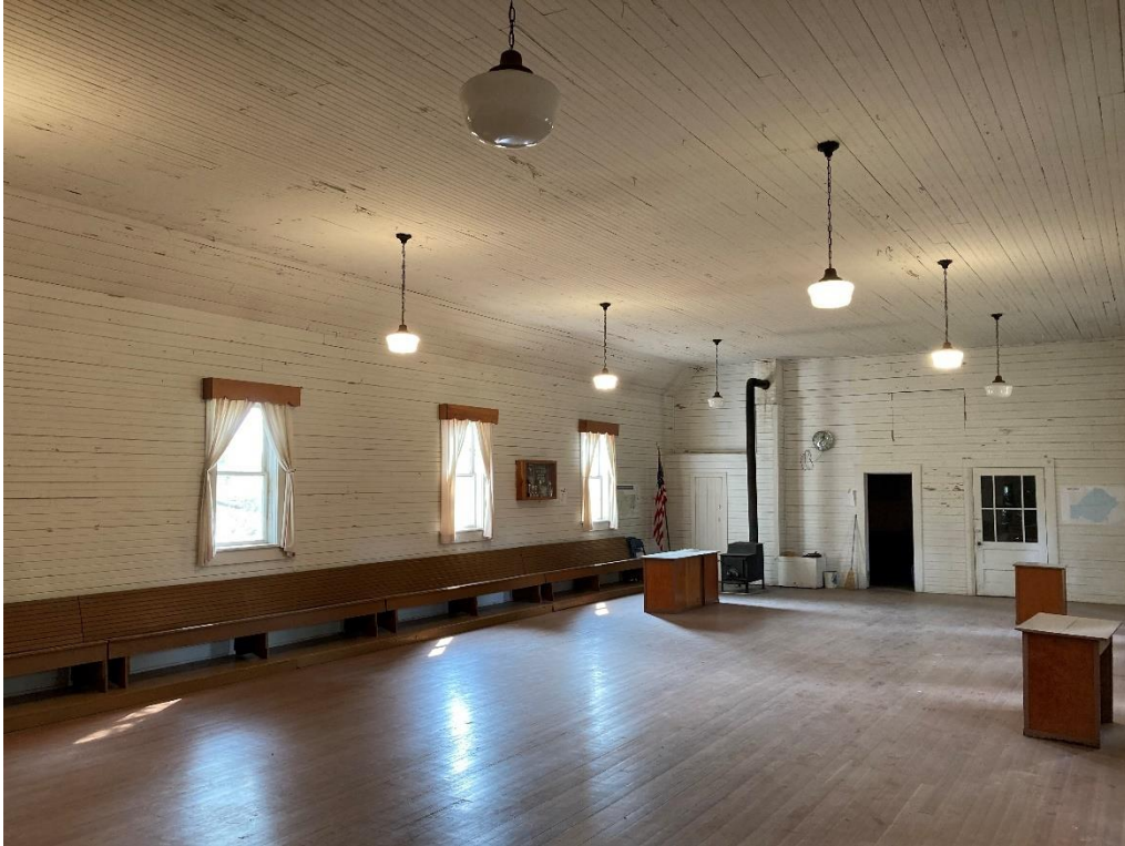
Photo 26. Main hall, facing south.
