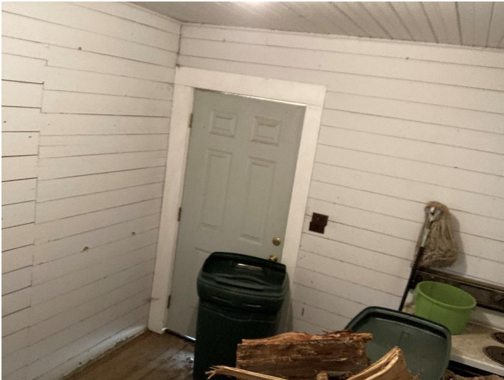
Photo 16. Front anteroom addition, foyer, facing south.
