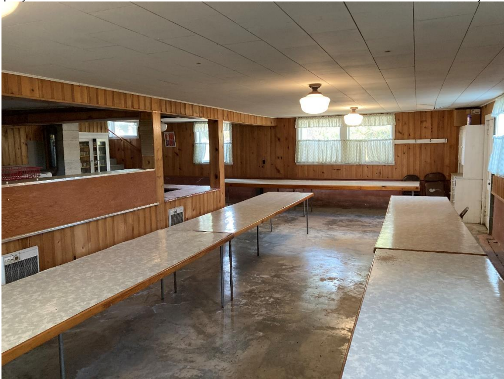
Photo 56. Rear addition basement kitchen/dining room, facing northwest.
