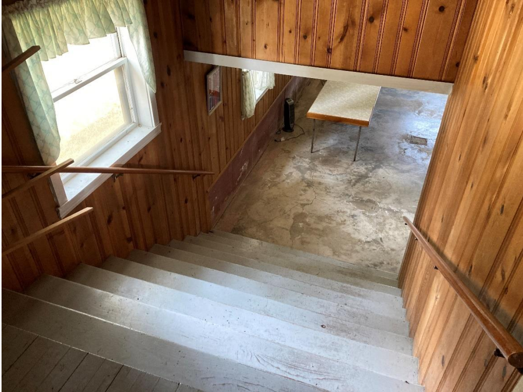
Photo 48. Rear addition basement stairwell, facing northeast.
