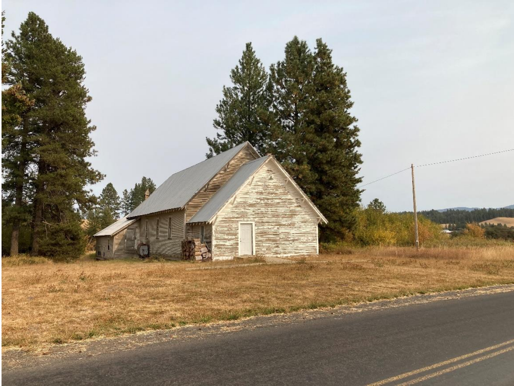
Photo 1. Front elevation with setting, facing northeast.
