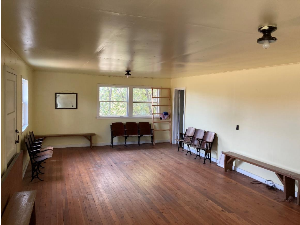
Photo 42. Rear addition, juvenile grange hall, facing southeast.
