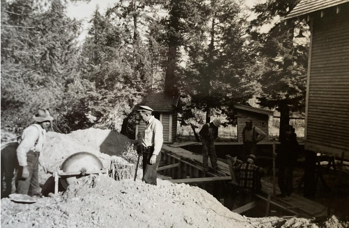
Figure 3. View of men building new rear addition foundation, 1952, facing east.
