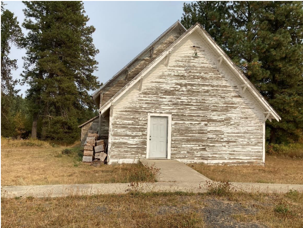
Photo 4. Front elevation, facing northeast.
