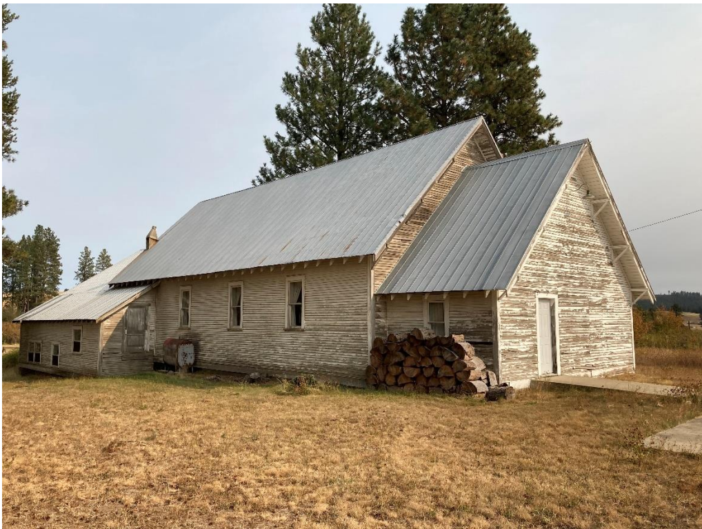
Photo 6. Front and side (northwest) elevations, facing east.
