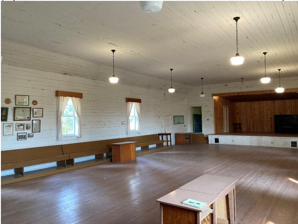
Photo 23. Main hall, facing north.
