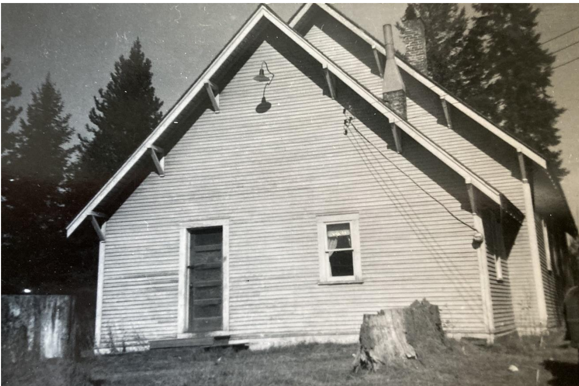
Figure 2. View of front elevation with 1936 anteroom addition, 1952, facing northeast.
