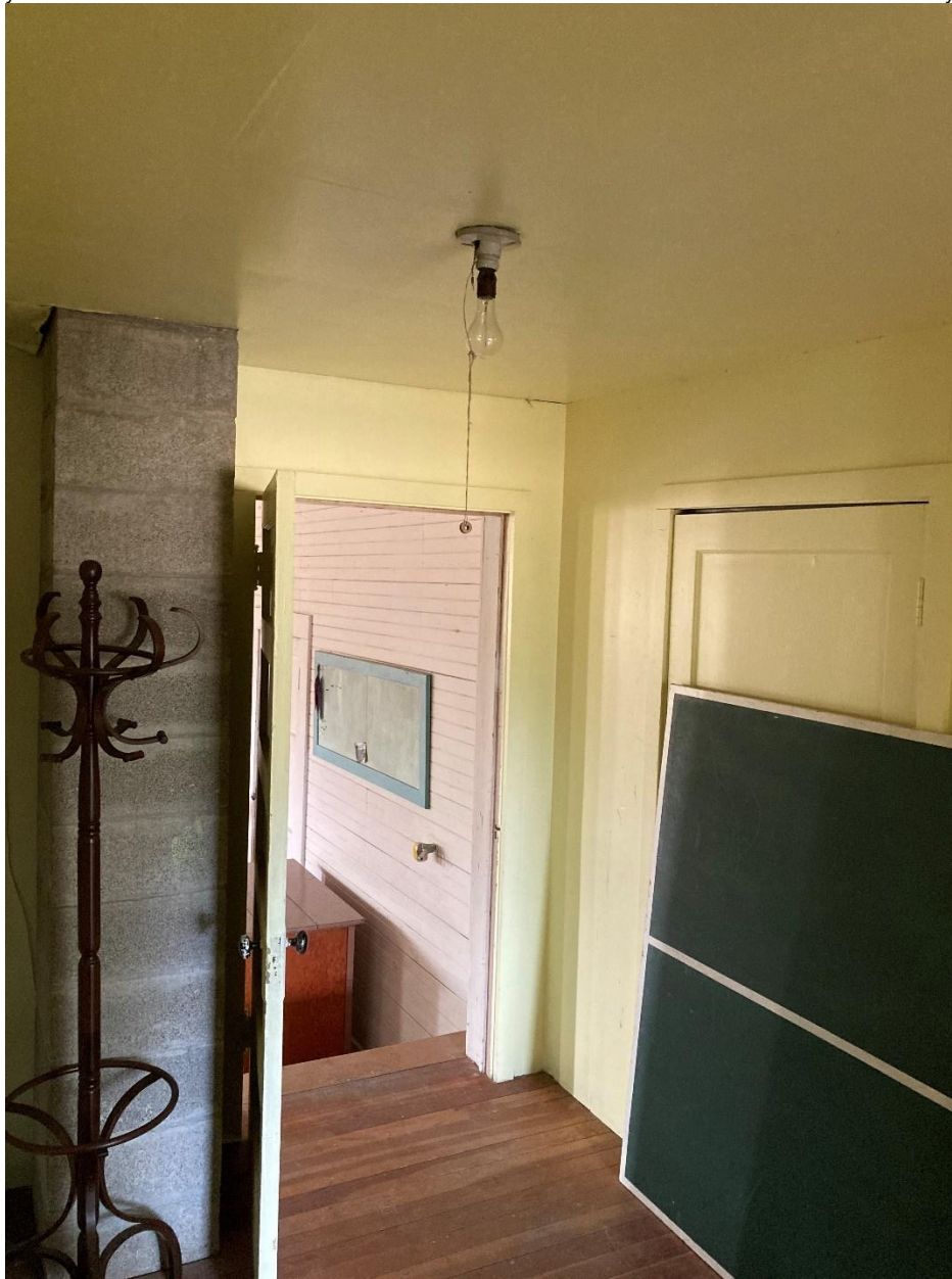
Photo 37. Rear addition, juvenile grange hall anteroom, facing west.
