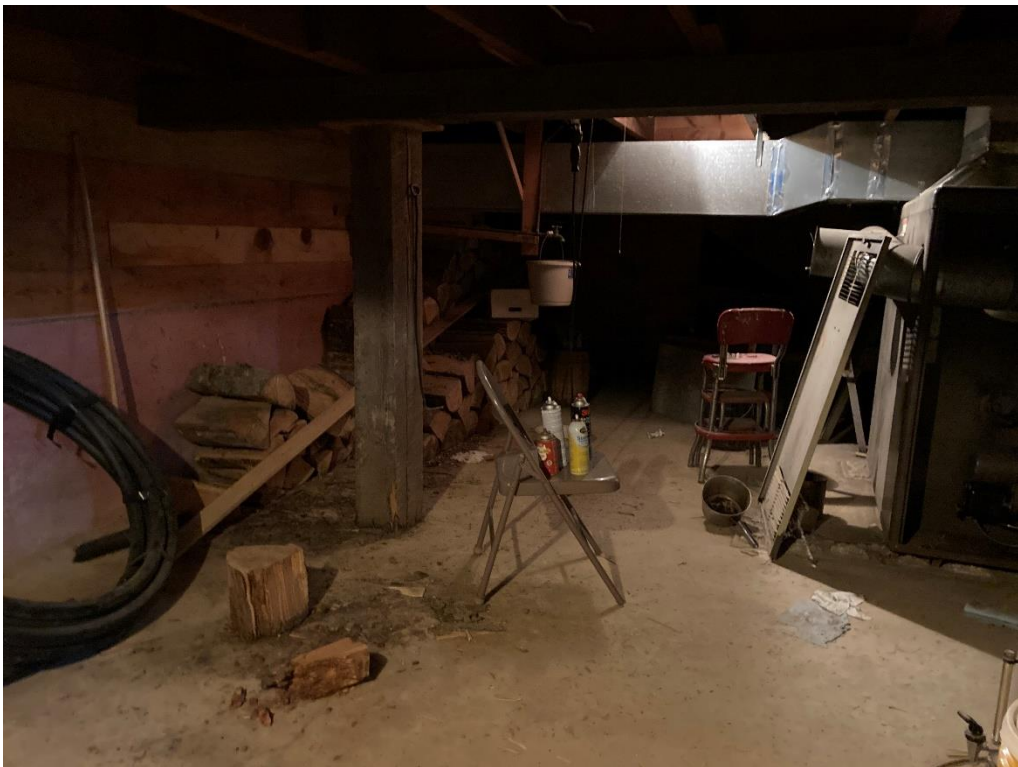
Photo 59. Rear addition basement storage room, facing west.
