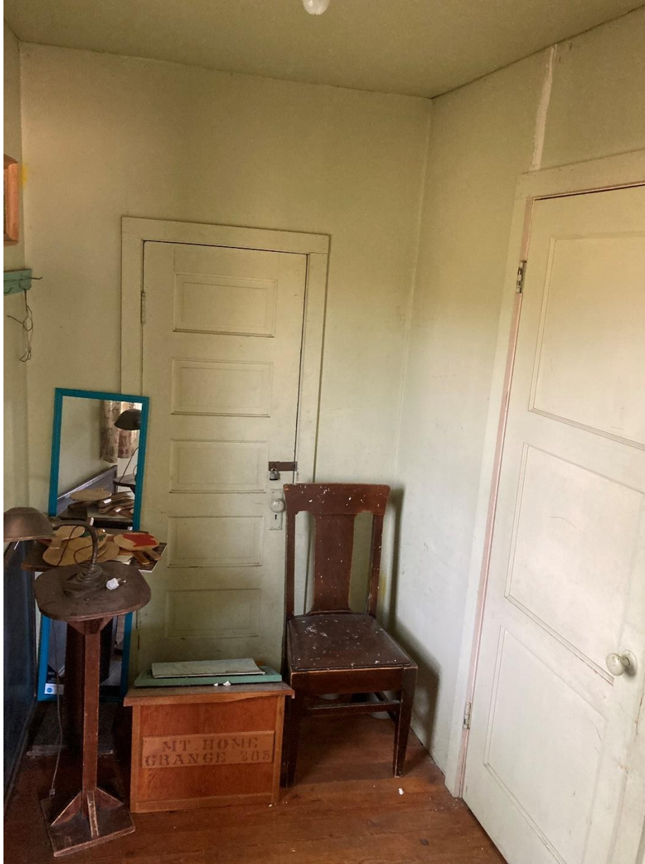
Photo 44. Rear addition juvenile grange coatroom, facing west.
