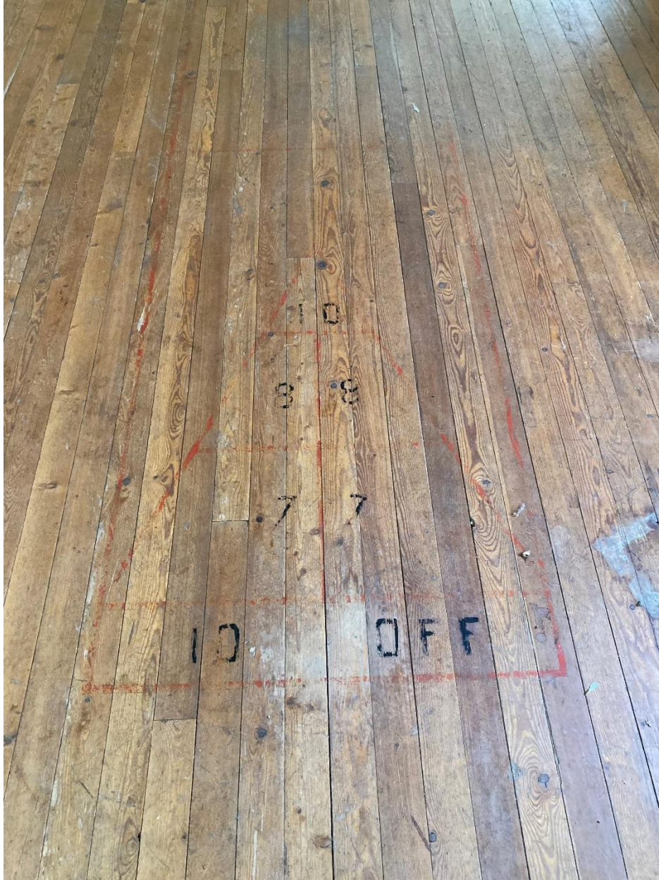
Photo 40. Rear addition, juvenile grange hall, hardwood flooring, facing northeast.
