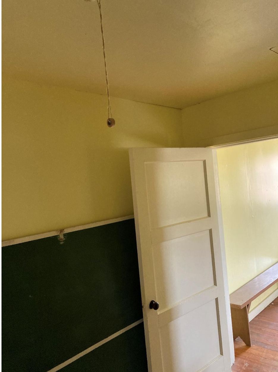
Photo 35. Rear addition, juvenile grange hall anteroom, facing north.
