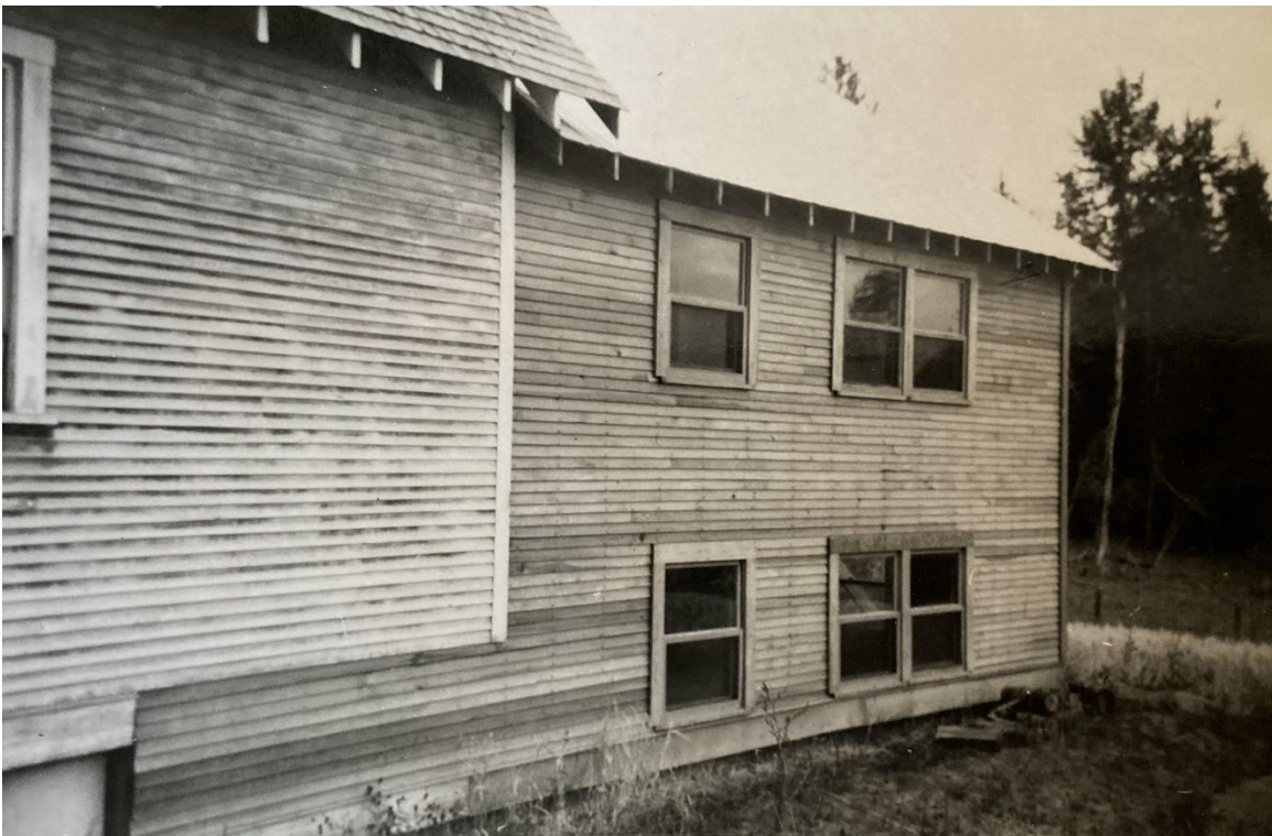
Figure 4. View of new rear addition, 1953, facing north.
