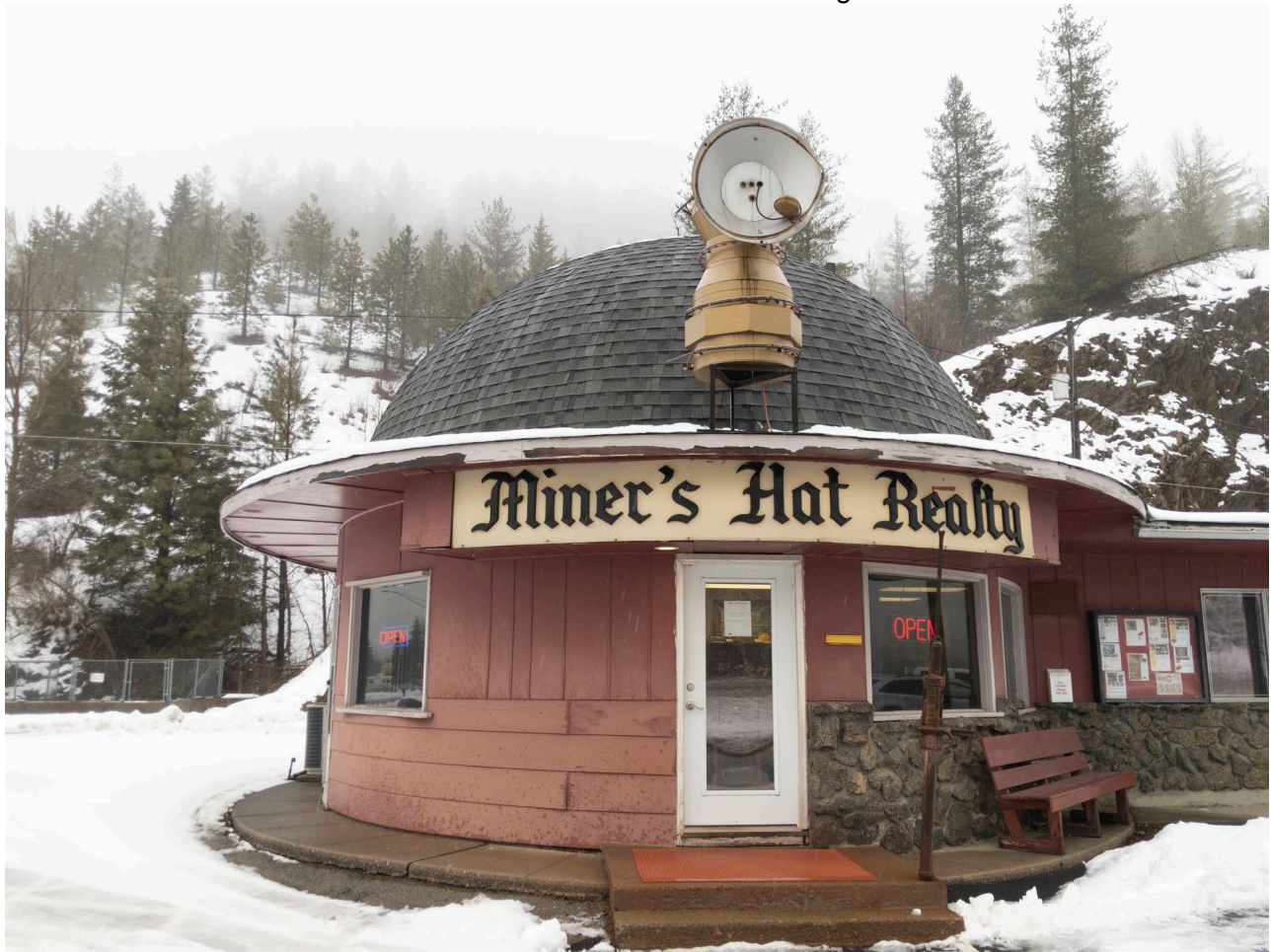
Photo #6: View of main entrance on southwest elevation. Camera facing north-northwest.
