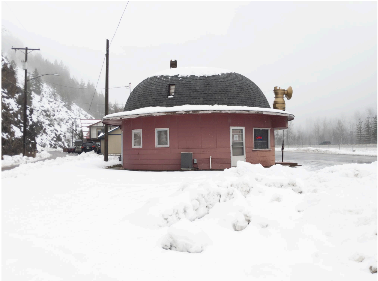
Photo #5: View of west elevation. Camera facing east.
