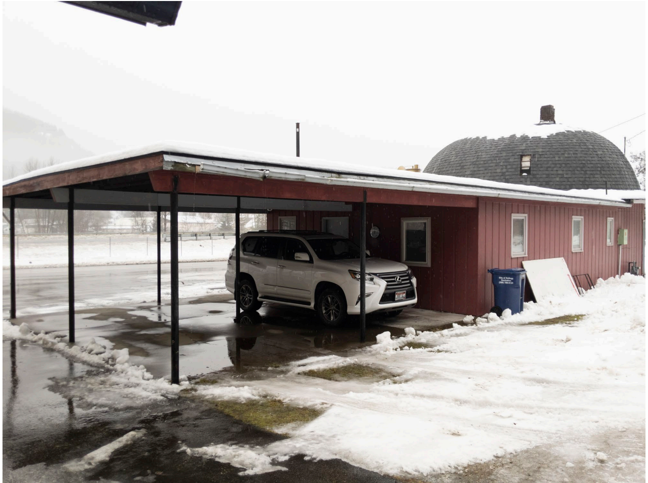
Photo #3: View of southeast (left) and northeast (right) elevations. Camera facing southwest.
