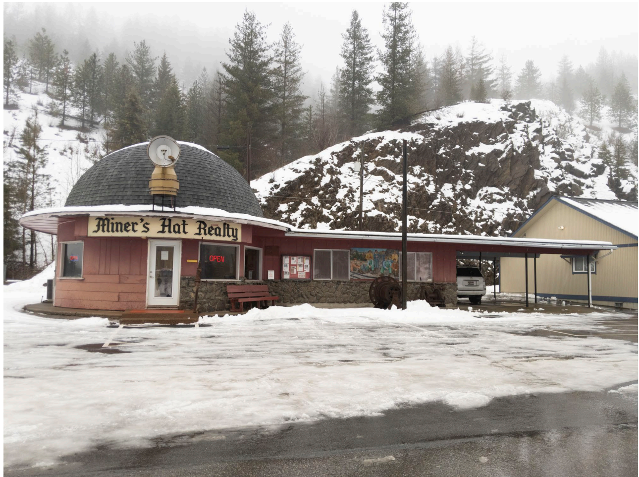
Photo #1: View of façade (southwest elevation). Camera facing northeast.
