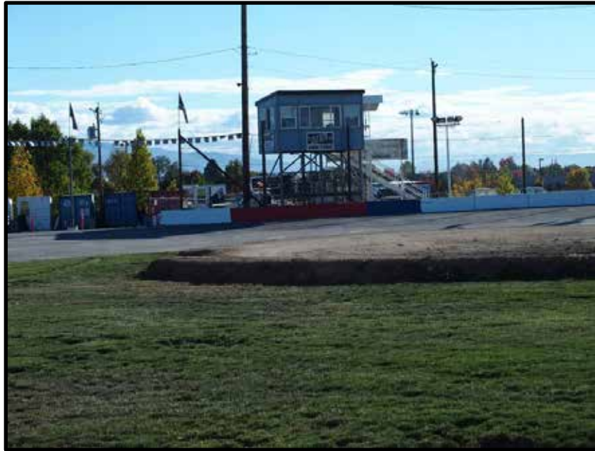
Photo 53 of 63: Resource 24. Camera facing southeast.
