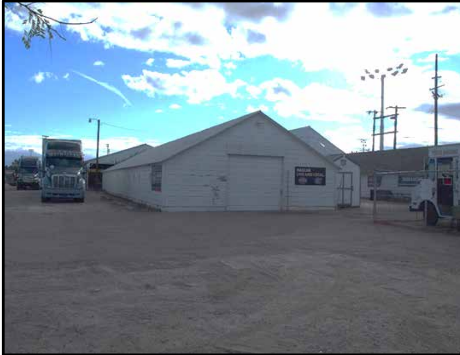
Photo 39 of 63: Resource 18. Camera facing east.
