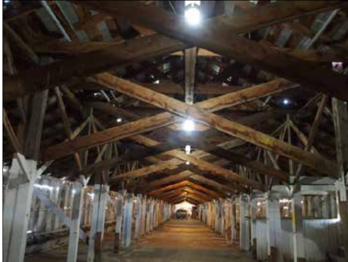
Photo: View looking east of interior trusses and support beams
