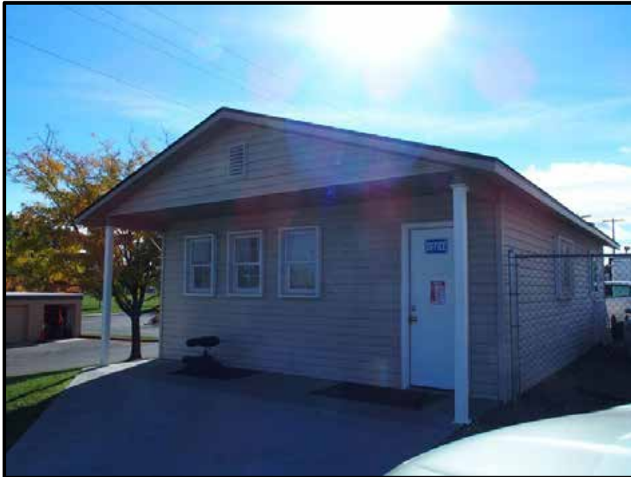
Photo 27 of 63: Resource 15. Camera facing southeast.
