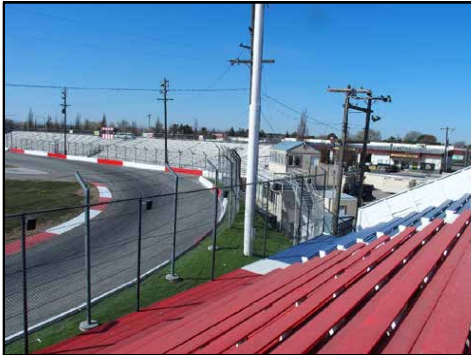
Photo 3 of 63: Overview from Resource 17, Dairy Barn/Grandstand. Camera facing southwest.
