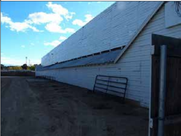
Photo: View looking east
