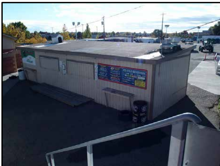
Photo 22 of 63: Resource 12. Camera facing southeast.
