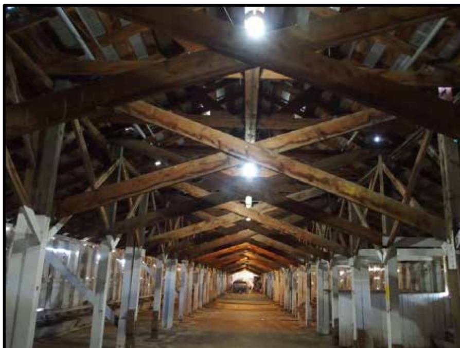
Photo 32 of 63: Interior of Resource 16 showing trusses. Camera facing east.
