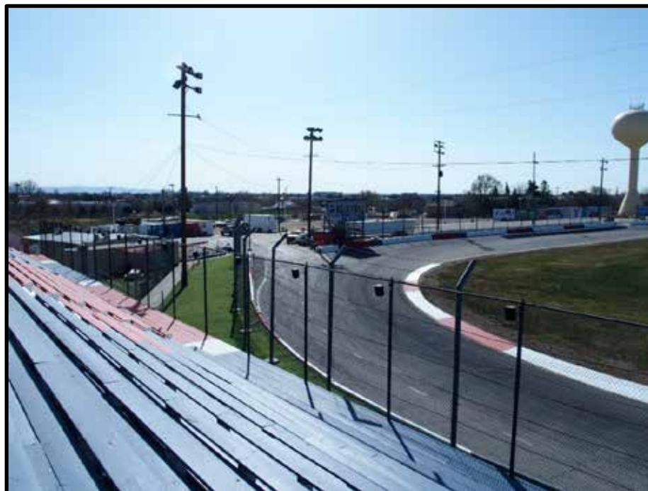
Photo 2 of 63: Overview from Resource 17, Dairy Barn/Grandstand. Camera facing southeast.
