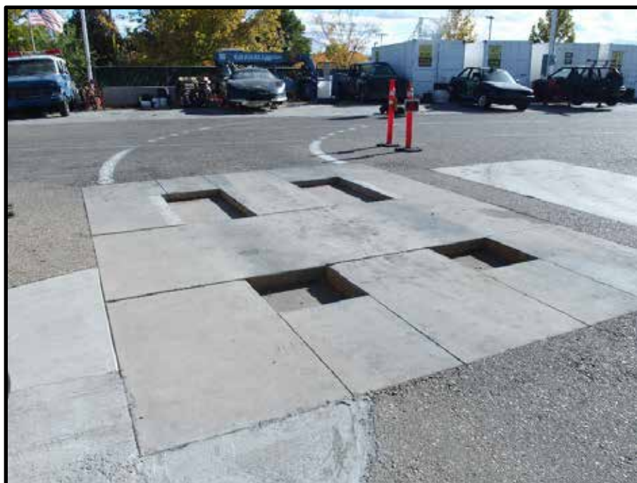
Photo 56 of 63: Resource 25. Camera facing southeast.
