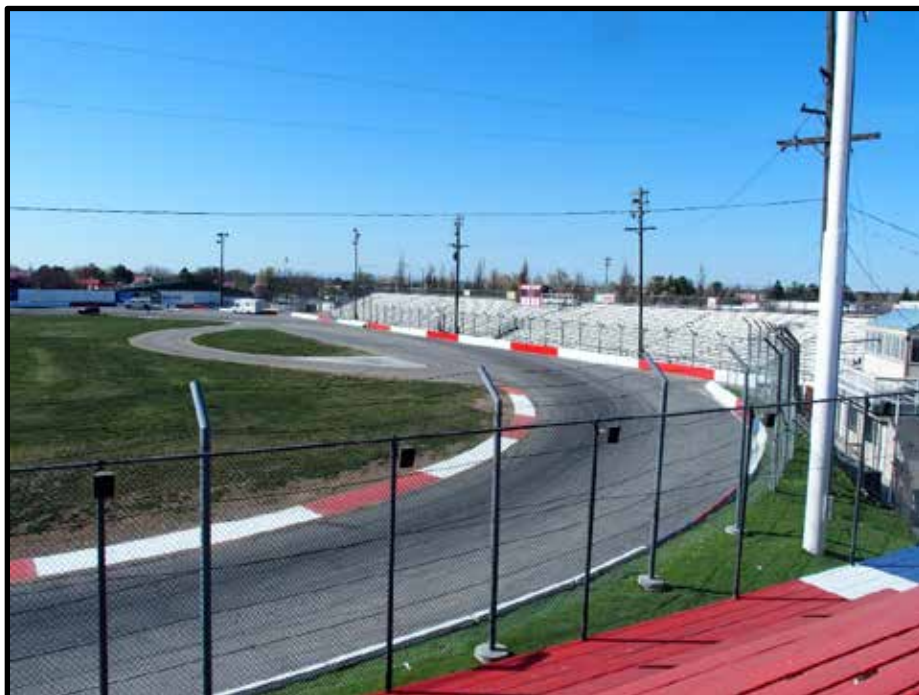
Photo 4 of 63: Overview from Resource 17, Dairy Barn/Grandstand. Camera facing south.
