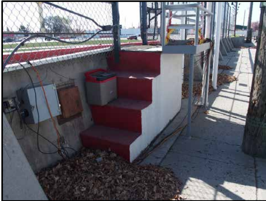
Photo 21 of 63: Resource 11. Camera facing southeast.
