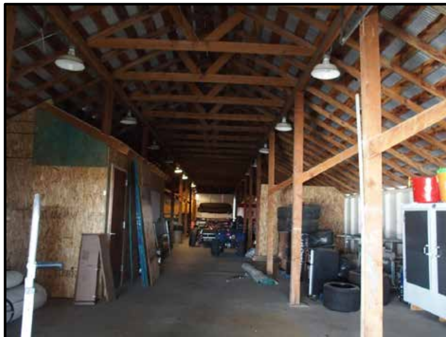
Photo 42 of 63: Interior of Resource 18. Camera facing west.
