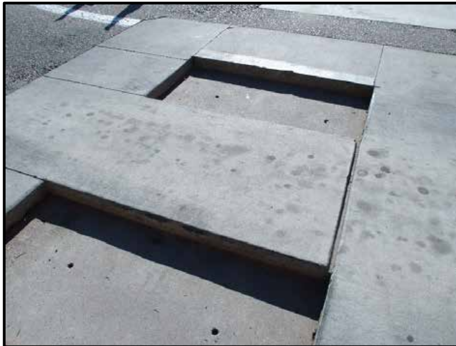
Photo 55 of 63: Resource 25. Camera facing southeast.
