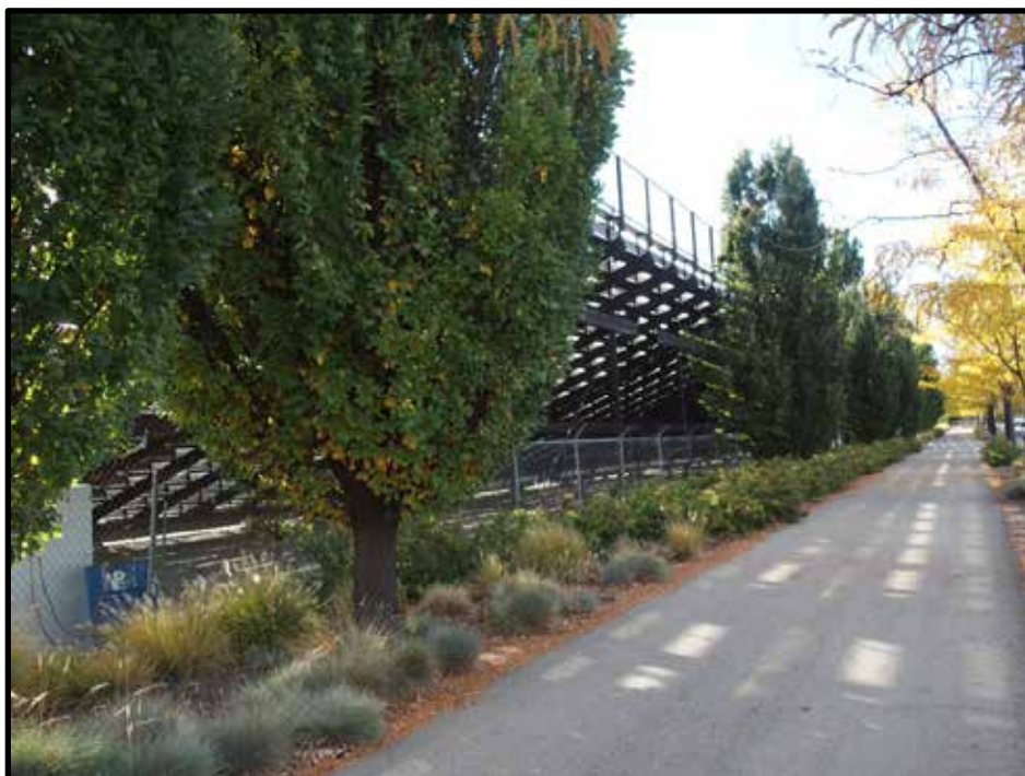
Photo 14 of 63: Resource 4, west elevation. Camera facing south.
