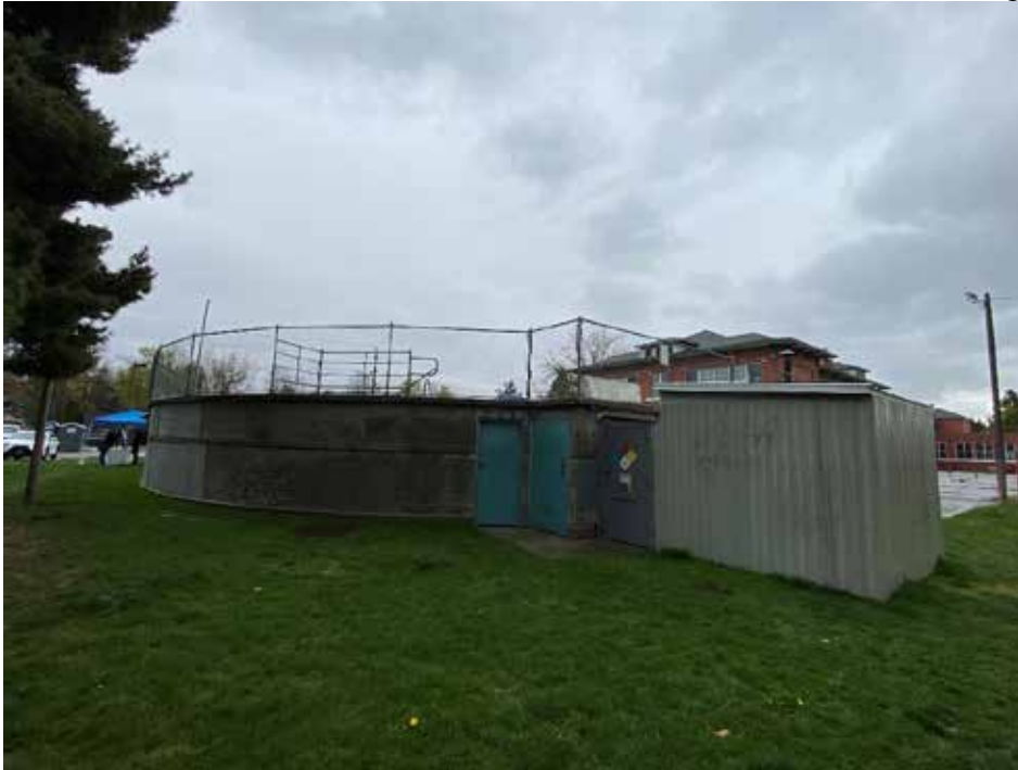
Photo 12: View of rear (west) and side (north) elevations. Camera facing southeast.
