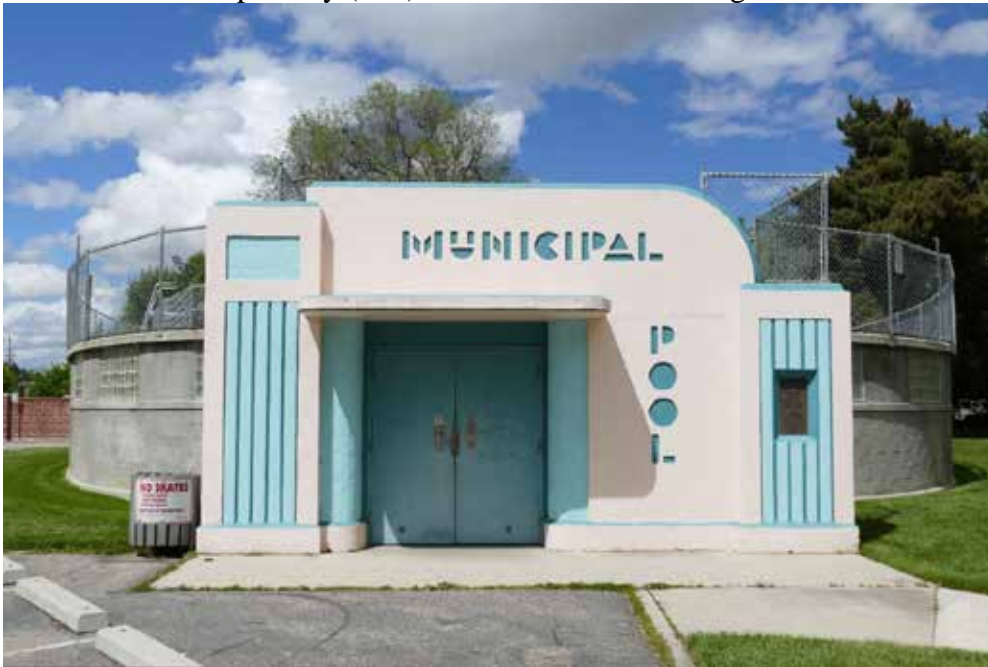
Photo 5: View of primary (east) elevation. Camera facing west.
