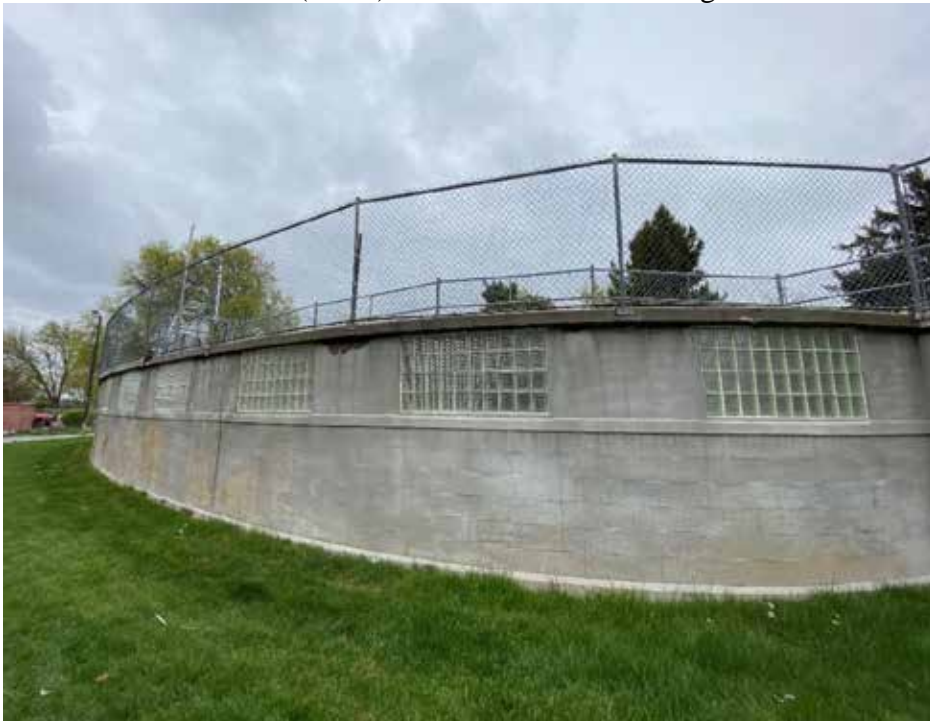
Photo 9: View of side (south) elevation. Camera facing northwest.
