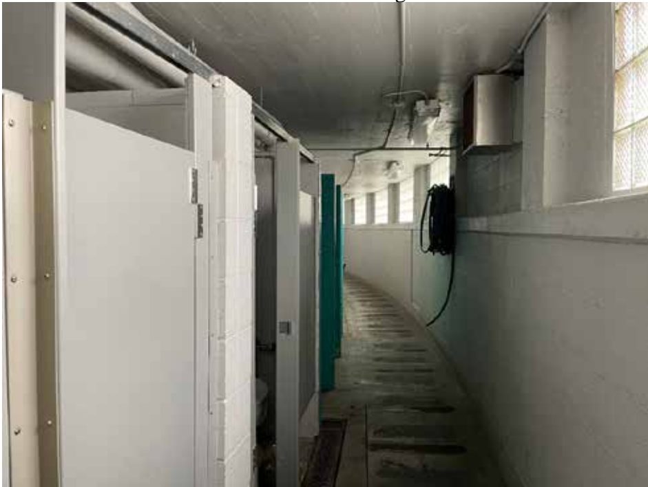
Photo 17: Men’s locker room. Camera facing west.
