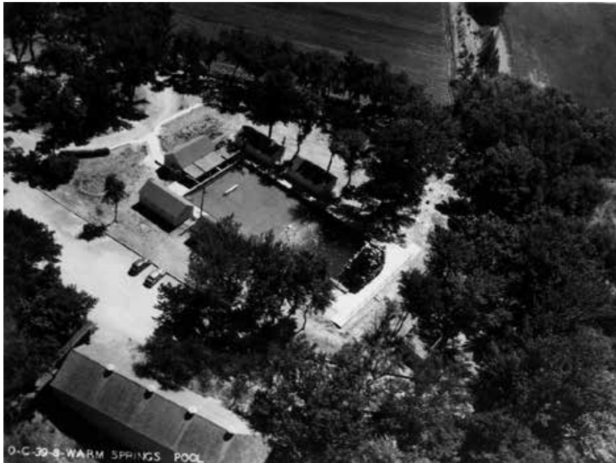
Figure 8: Natatorium, Boise Idaho, Aerial view of open-air pool after 1936, Date Unknown Source: Idaho State Archives
