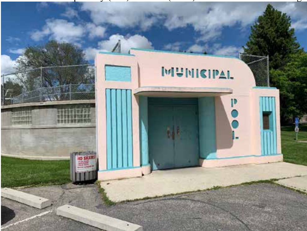
Photo 6: View of primary (east) and side (south) elevations. Camera facing northeast.
