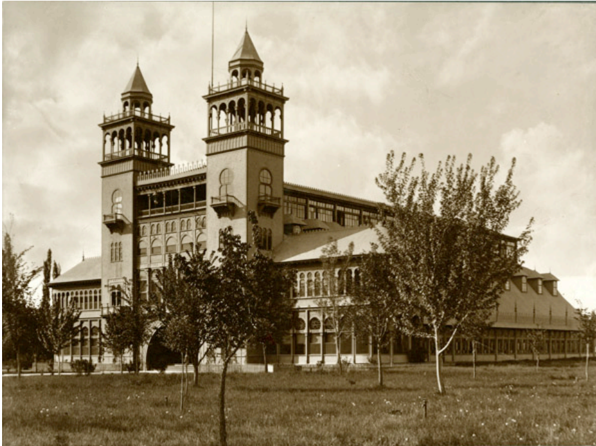
Figure 6: Natatorium, Boise, Idaho, Exterior view, Date Unknown Source: Idaho State Archives.
