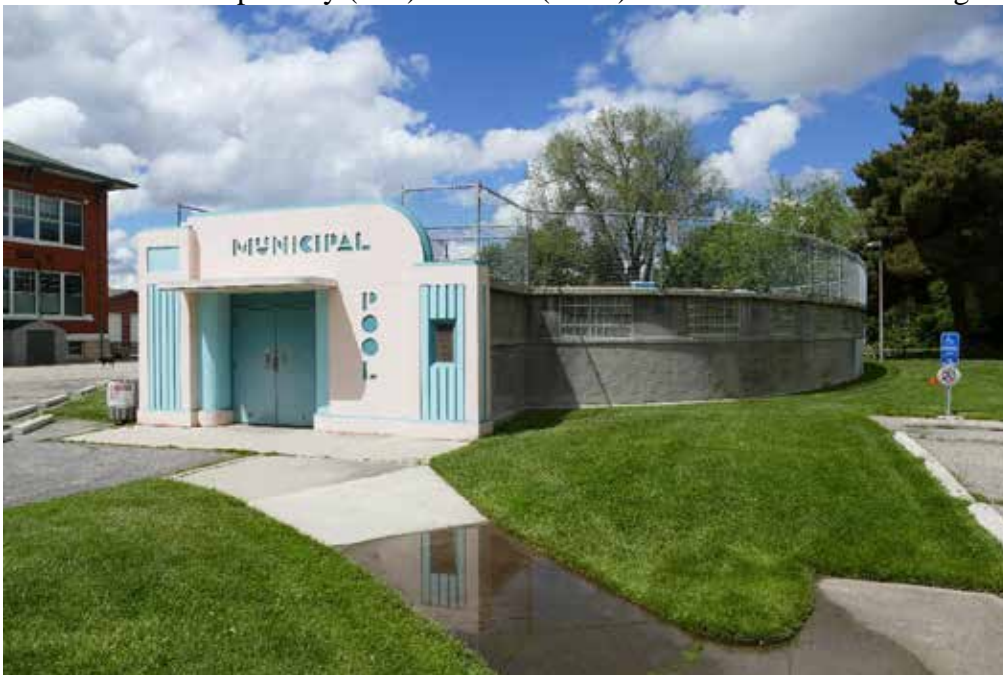
Photo 4: View of primary (east) and side (north) elevations. Camera facing southwest.
