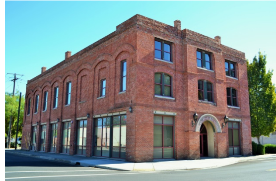
Figure 95. Building at 908 Idaho Street.
