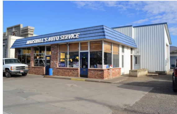
Figure 71. Building at 865 D Street.
