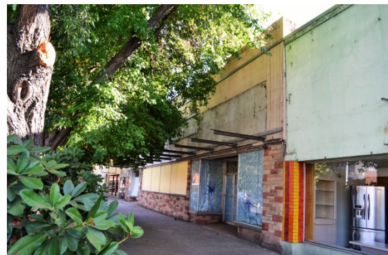
Figure 43. Building at 800 Main Street (west).
