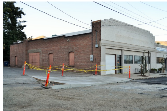
Figure 86. Building at 132 New 6th Street (east).
