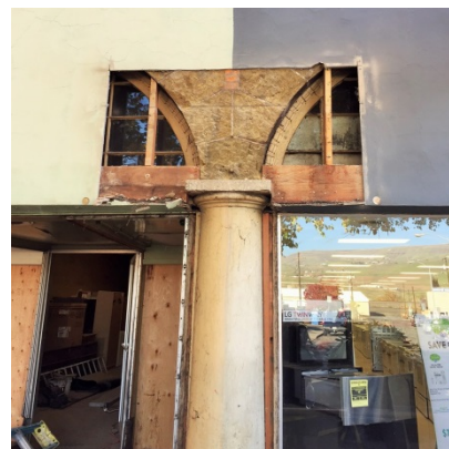
Figure 42. Detail of building at 716 Main Street, November 2016.
