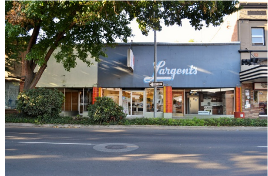
Figure 41. Building at 716 Main Street, September 2016.
