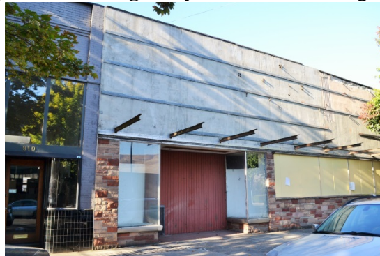
Figure 44. Building at 800 Main Street (east).
