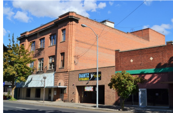
Figure 59. Building at 855 Main Street (the 3- and 4-story building).
