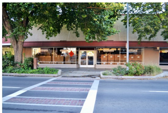
Figure 62. Building at 825 Main Street (west).
