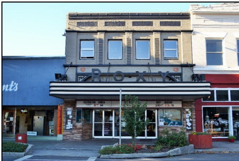
Figure 22. Classical Revival style (upper level): Building at 714 Main Street (Resource Number 10), north (front) elevation.
