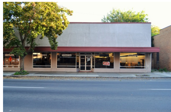
Figure 61. Building at 825 Main Street (east).
