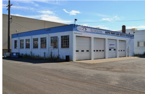
Figure 79. Building at 508 Beachey Street.
