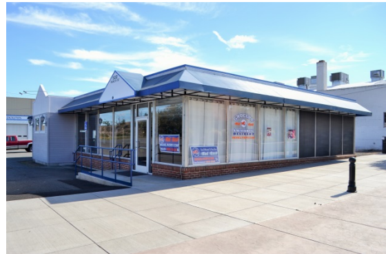
Figure 78. Building at 502 Beachey Street.
