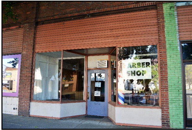
Figure 11. Storefront at 844 Main (Resource Number 20); view to the south. Transom lights have been covered.
