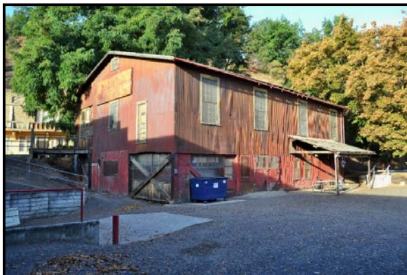
Figure 29. Utilitarian / Industrial building type: Building at 132 New 6 th Street (Resource Number 57), east and south sides.
