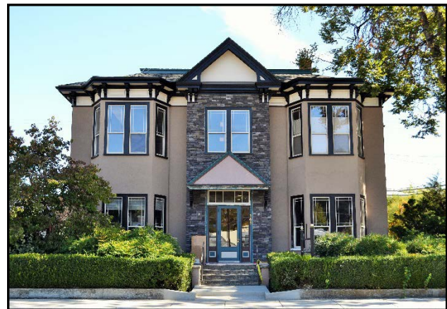
Figure 14. Former residence, former funeral home (Resource Number 66); view to southeast.
