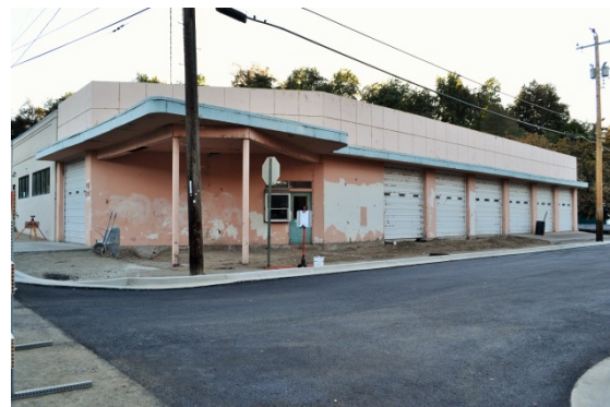
Figure 83. Building at 818 F Street.
