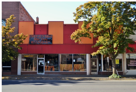
Figure 55. Building at 854 Main Street; building is section of restaurant to left.
