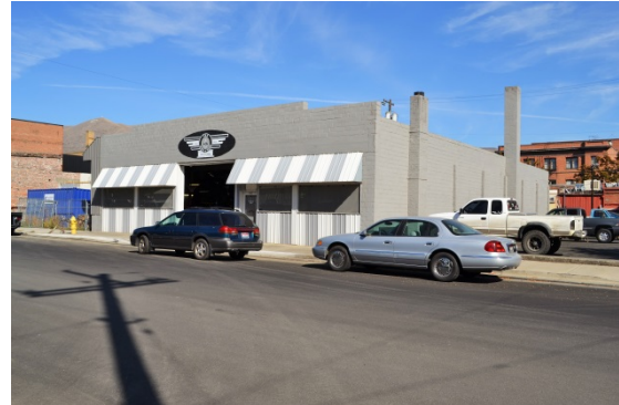
Figure 80. Building at 847 F Street.
