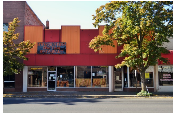
Figure 54. Building at 854 Main Street; building is section of restaurant to right.
