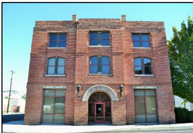
Figure 15. Former bottling plant, former commercial laundry (Resource Number 65); view to southeast.
