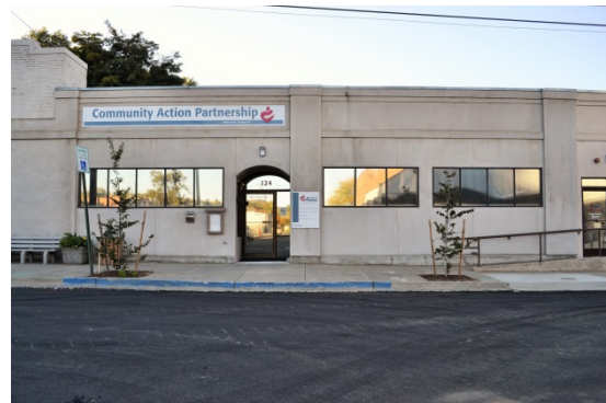
Figure 85. Building at 124 New 6th Street (south).
