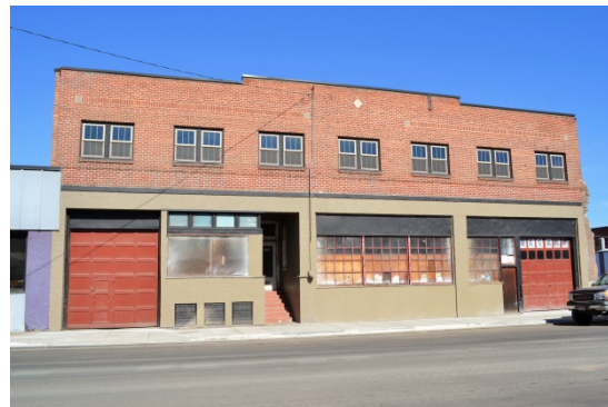
Figure 81. Building at 835 F Street.
