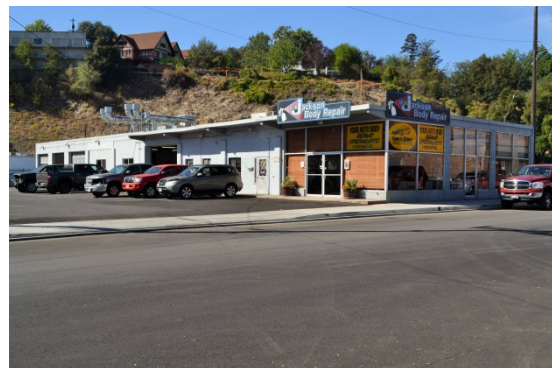
Figure 89. Building at 856 F Street.
