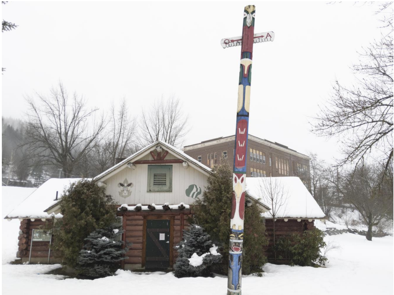
Photo #1: View of façade (east elevation) and totem pole in foreground. Camera facing west-southwest.
