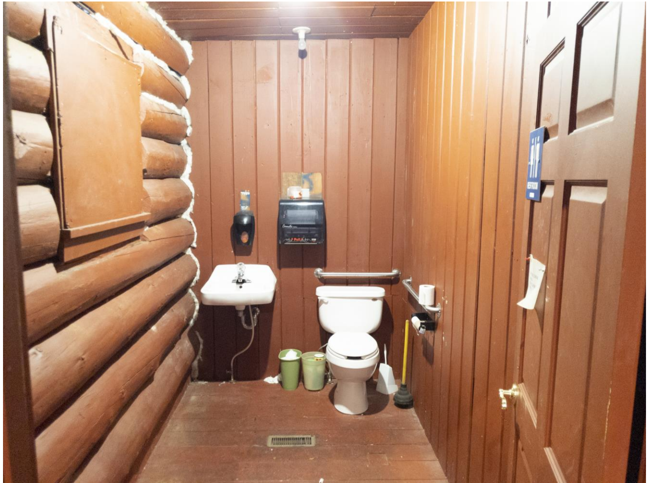
Photo #15: View of two-piece washroom. Camera facing south-southeast.
