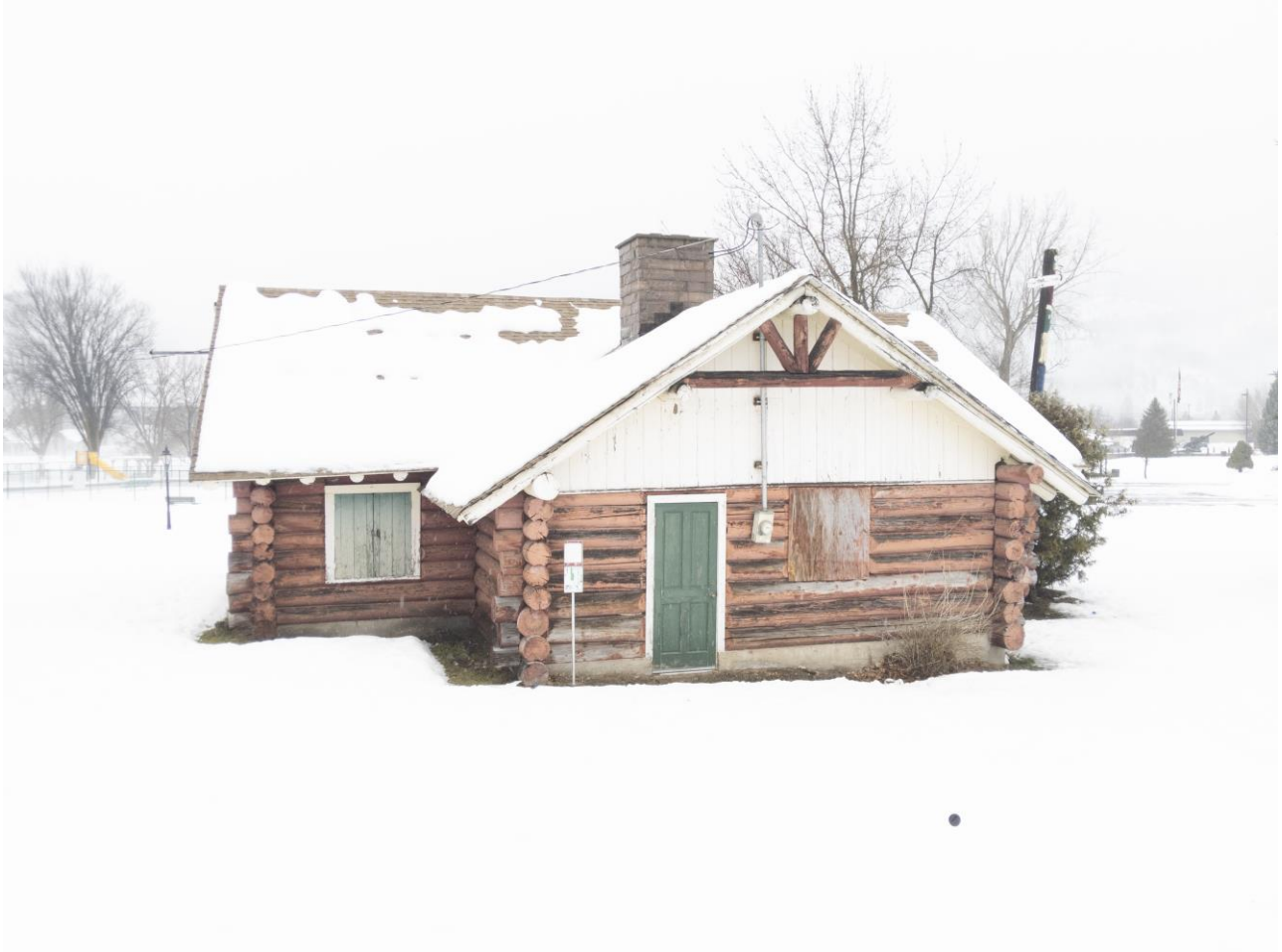
Photo #6: View of south elevation. Camera facing north.
