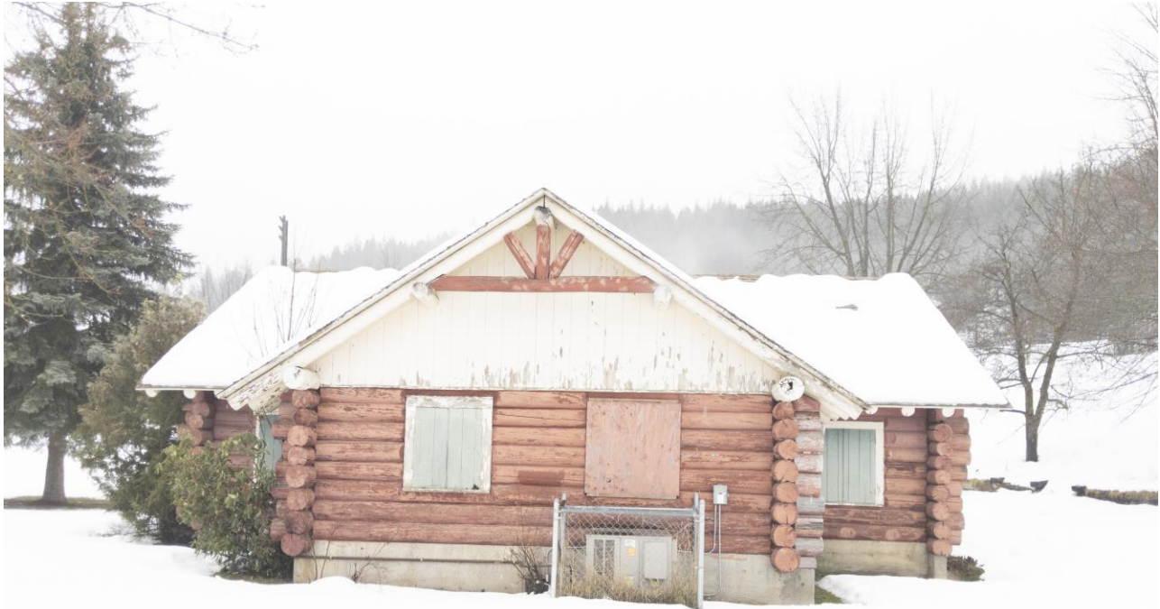
Photo #3: View of north elevation. Camera facing south-southeast.
