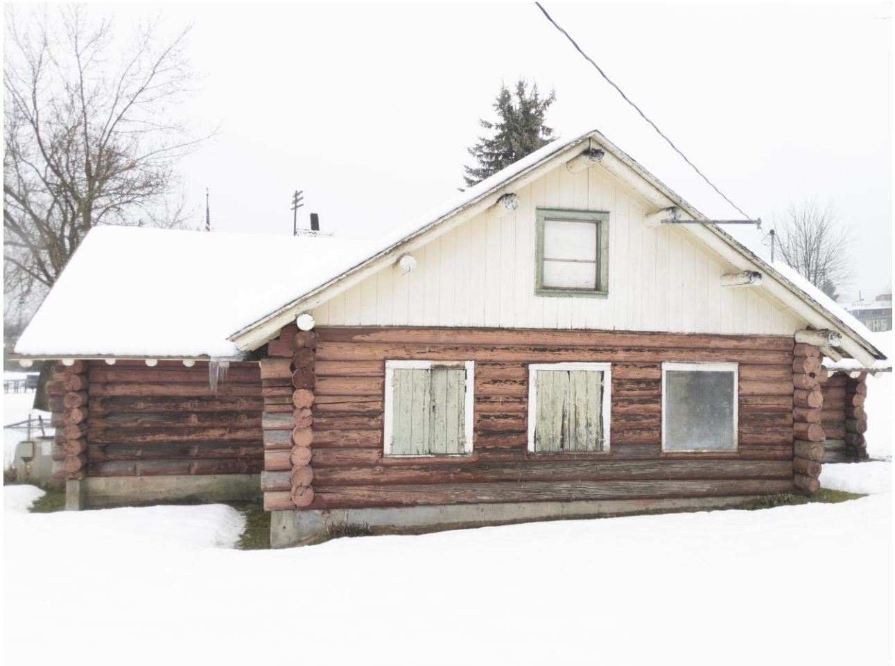
Photo #5: View of west elevation. Camera facing east-northeast.
