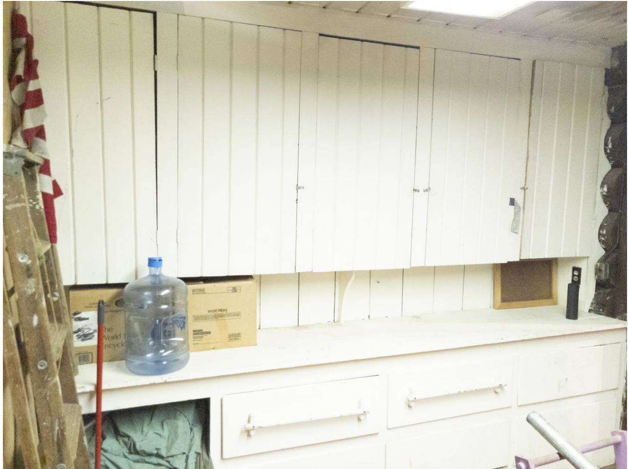
Photo #13: View of cabinetry in storage room. Camera facing northwest.
