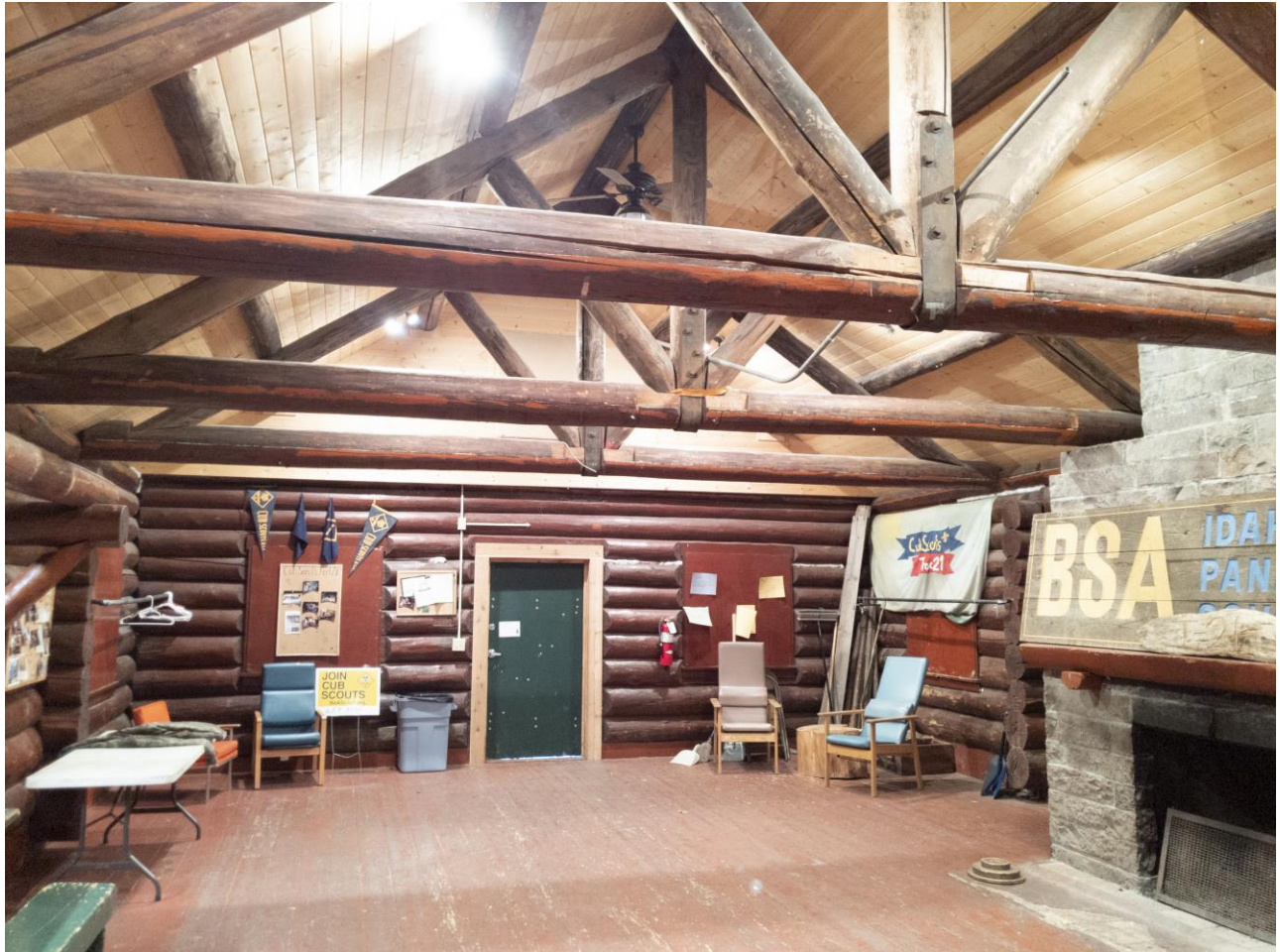
Photo #9: View of main room facing entrance. Camera facing east.
