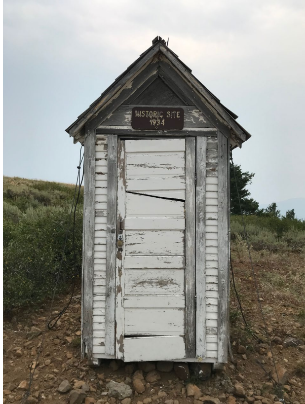
Photo #8. Historic outhouse. Facing west at east elevation.
