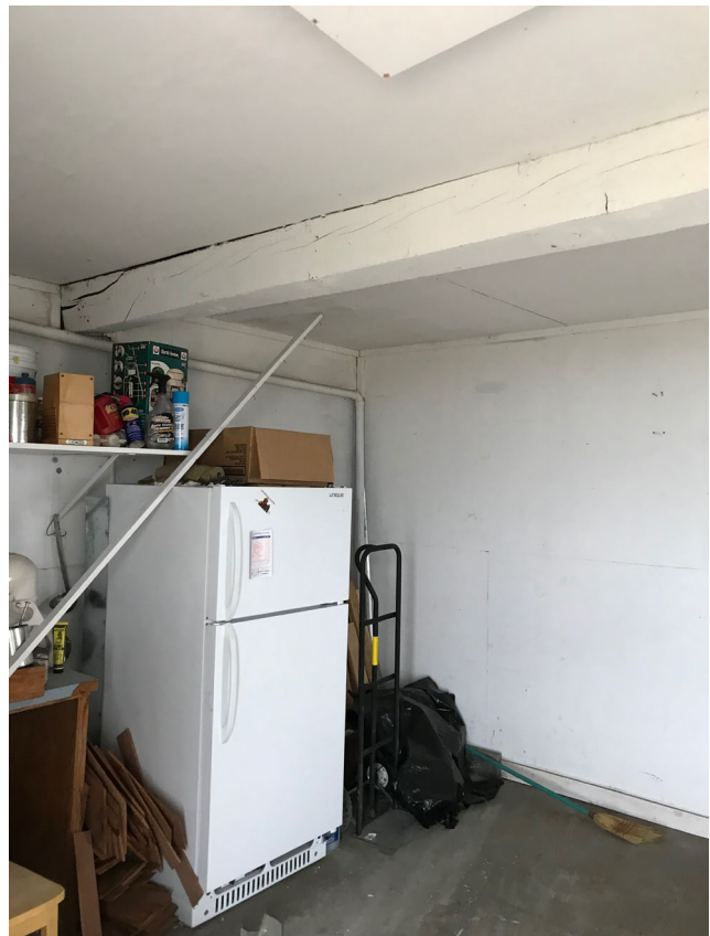
Photo #36. Lookout storage room interior showing original support beam. Facing northeast.
