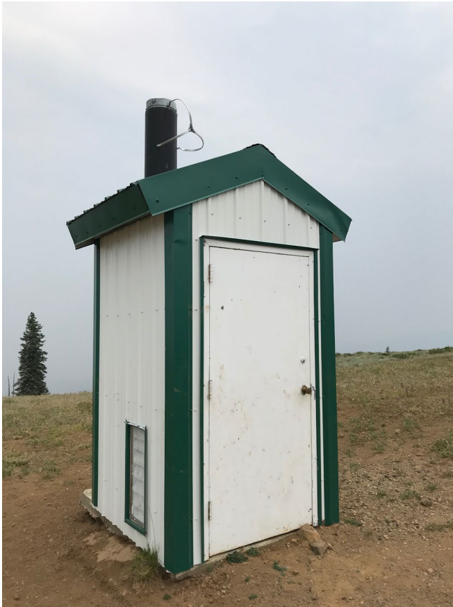
Photo #13. Modern latrine. Facing southwest at north and east elevations.
