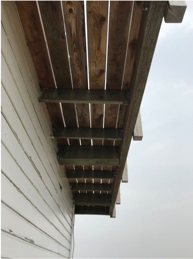
Photo #23. Catwalk underside (planks replaced in 2019) North elevation. Facing west.
