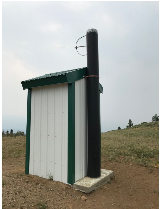
Photo #14. Modern latrine. Facing northeast at west and south elevations.
