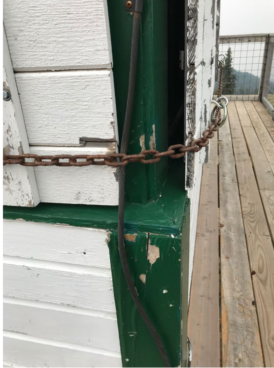
Photo #26. Lightning harness and facade detail. East elevation. Facing north northwest.
