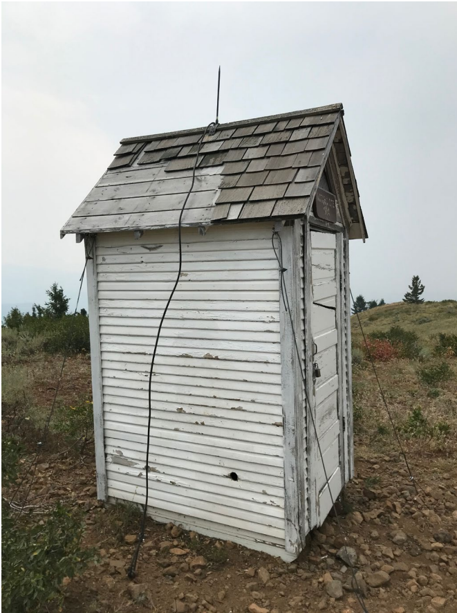
Photo #11. Historic outhouse. Facing south at north elevation.
