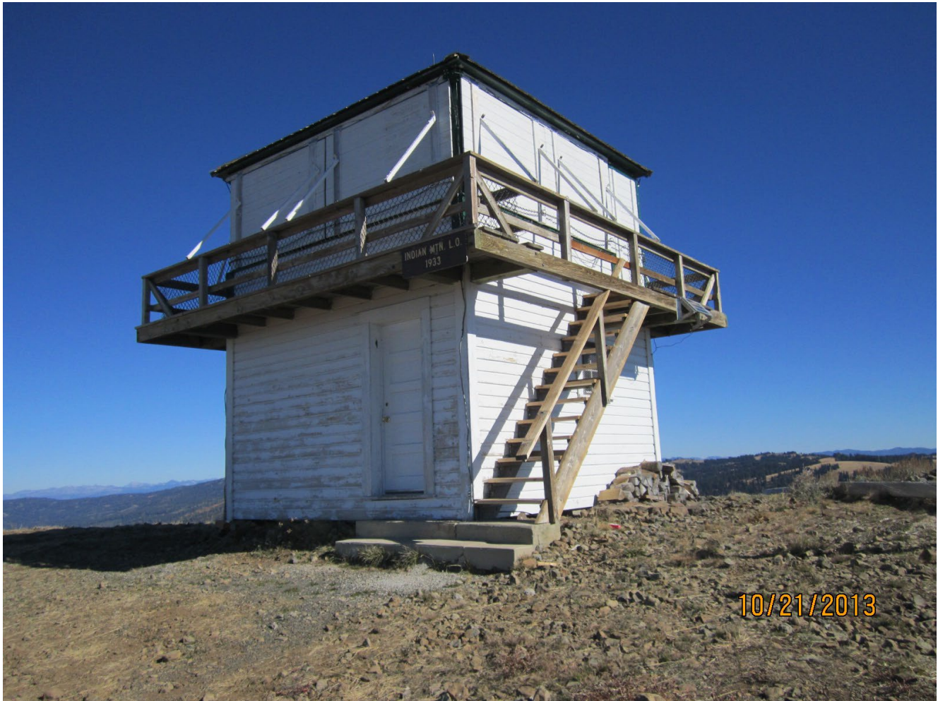
Photo #49. Lookout building. Before railing and stair restoration. Facing northeast.
