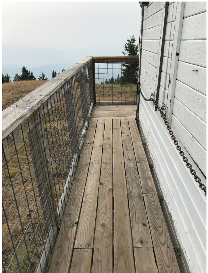
Photo #24. Catwalk, railing (restored in 2019), lightning harness. East elevation. Facing south
