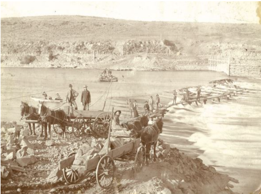
Figure 27. Circa 1911 photograph of workers building the Snake River retaining wall to create the falls. Source: Idaho Falls Magazine, January 26, 2022.
