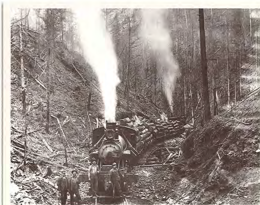
The Milwaukee Lumber Company moves burned timber from the 1910 fire with Heisler Engine pulling train. See "1910 Fire" on page 118.
