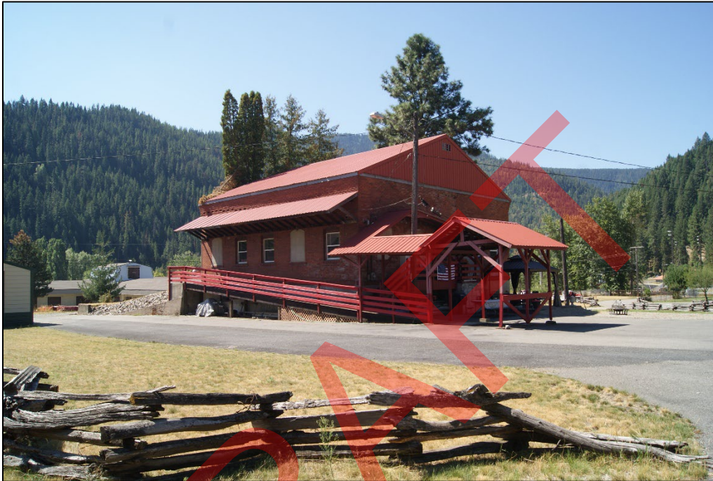
Photo 33. Steam Plant (resource 2), north and east elevations, view southwest. 2025.
