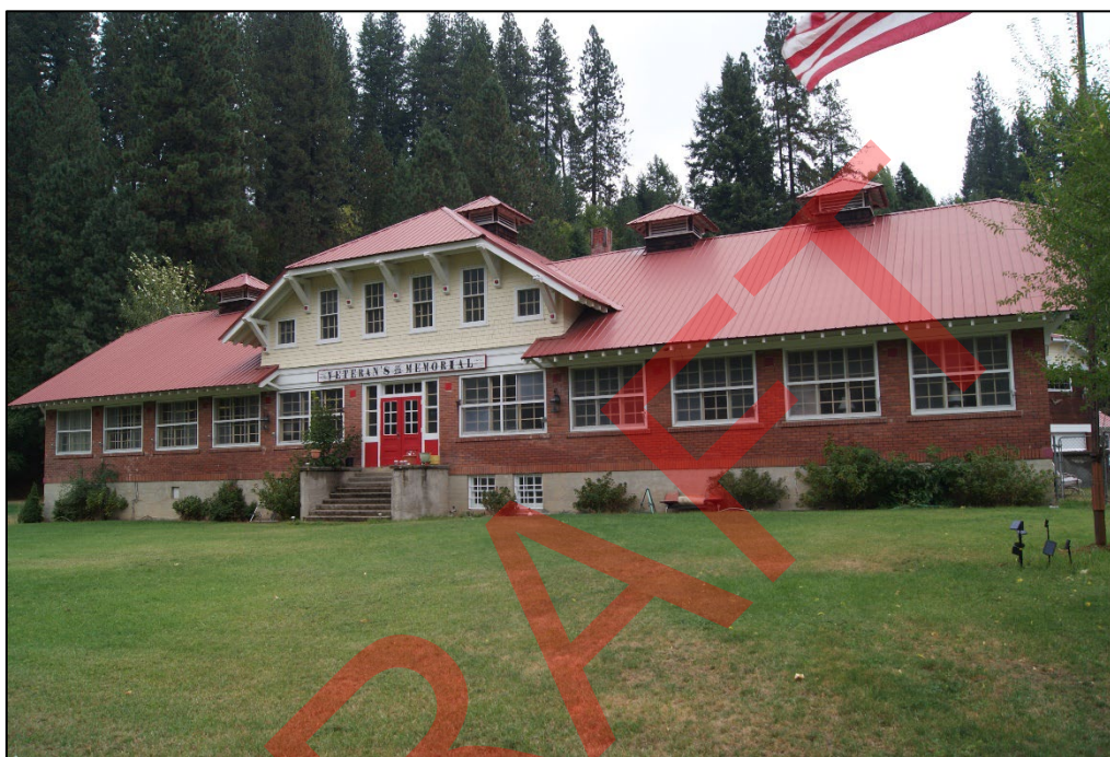
Photo 49. Shoshone County Poor Farm Isolation Hospital (Memorial Hall, resource 3), view northwest. 2024.
