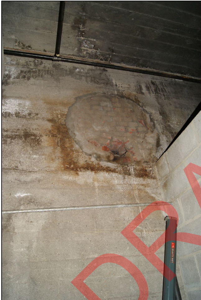
Photo 45. Steam Plant (resource 2) basement, infilled smokestack opening, view northeast. 2025.
