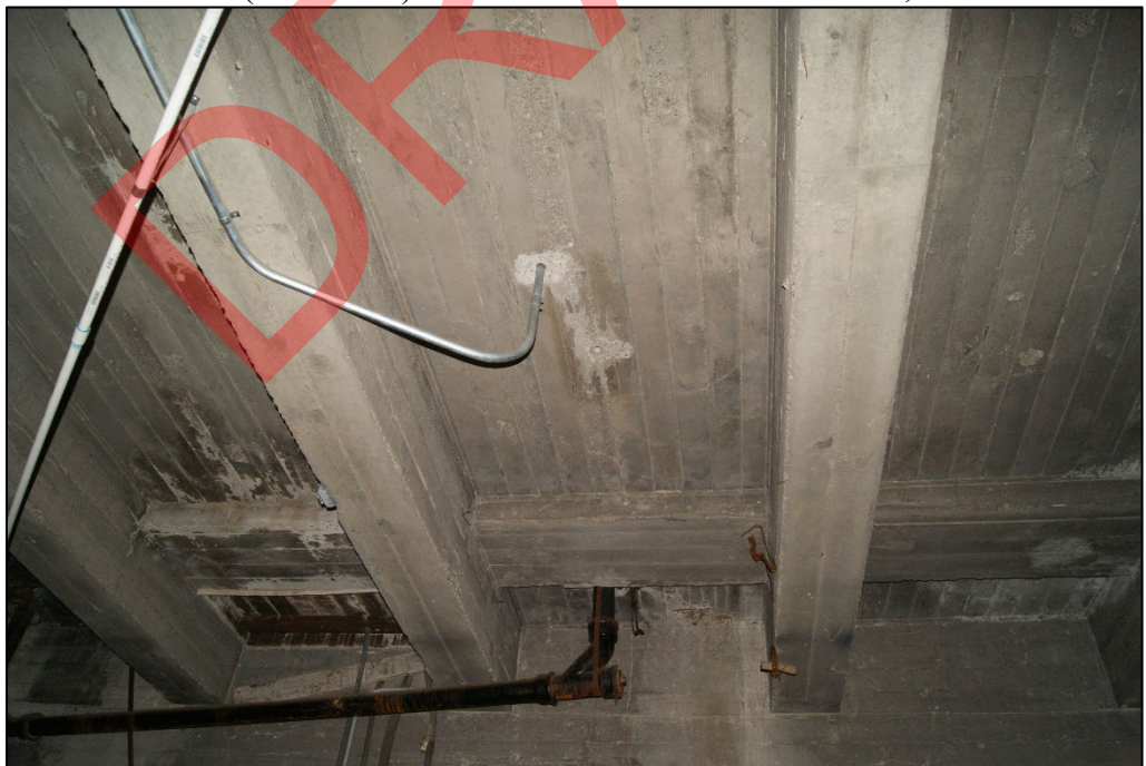
Photo 44. Steam Plant (resource 2) basement, concrete beam detail, view east. 2025.
