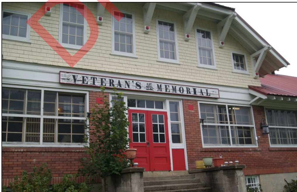
Photo 50. Memorial Hall (resource 3) main entry detail, view northeast. 2024. Continuation Sheet page 94
