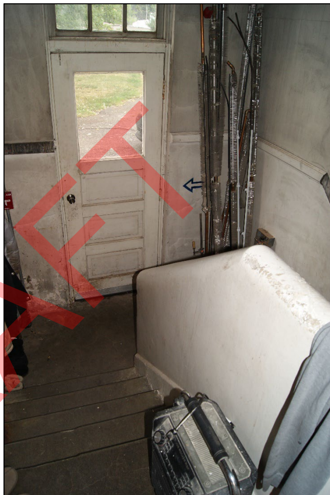
Photo 30. Infirmary (resource 1) stairs from first floor to basement, view west. 2024.
