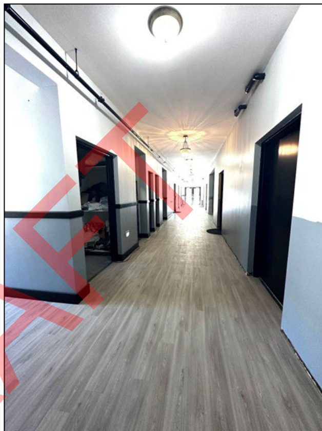
Photo 16. Infirmary (resource 1, now hotel) first-floor hallway, view east. Elizabeth Allison 2023.
