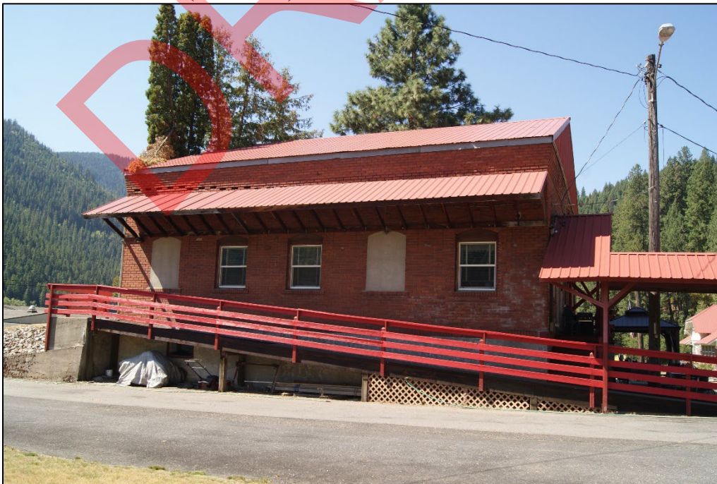
Photo 34. Steam Plant (resource 2), east elevation, view west. 2025.
