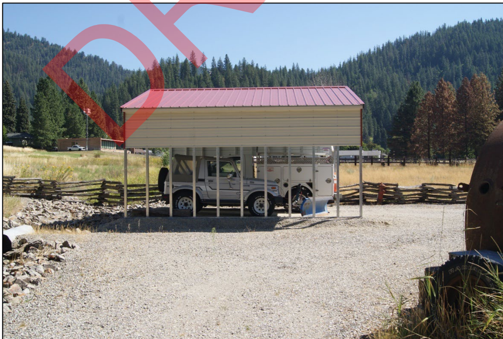
Photo 74. Steel vehicle shelter (resource 7), west elevation, view east. 2025.
