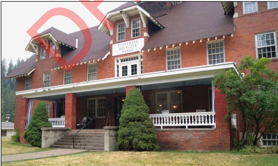
Photo 14. Infirmary (resource 1) main entry porch, south elevation, view northwest. 2024.
