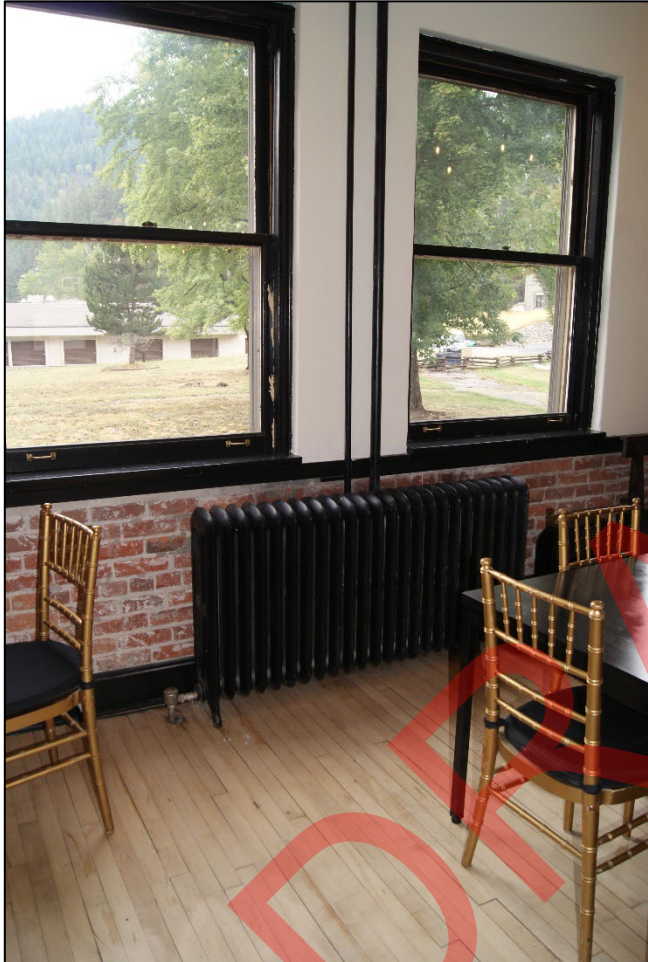
Photo 19. Infirmary (resource 1) dining room, view northwest. Note original (1917) brick masonry walls, radiator, and windows, view northwest. 2024.
