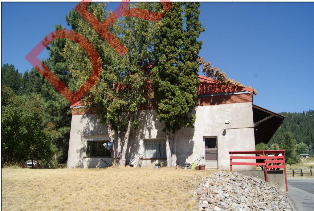
Photo 36. Steam Plant (resource 2), south elevation, view north. 2025.
