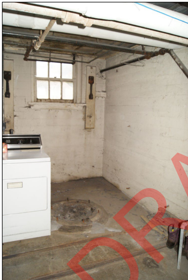
Photo 29. Infirmary (resource 1) laundry room, view west. 2024.
