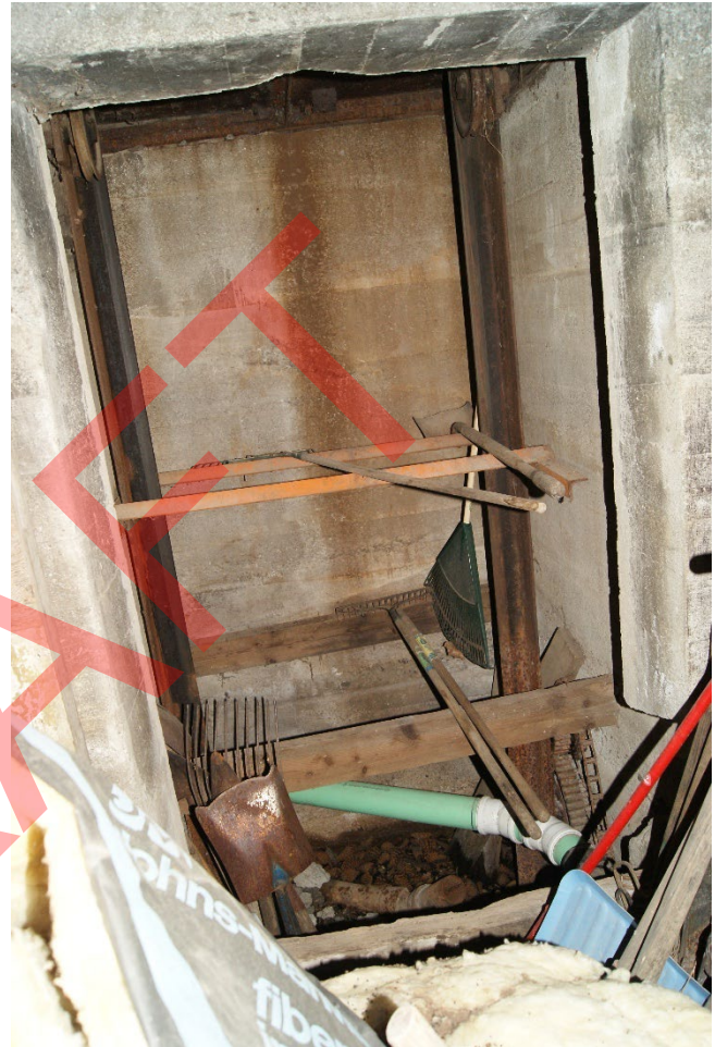
Photo 48. Steam Plant (resource 2) basement, equipment elevator remnants, view west. 2025.
