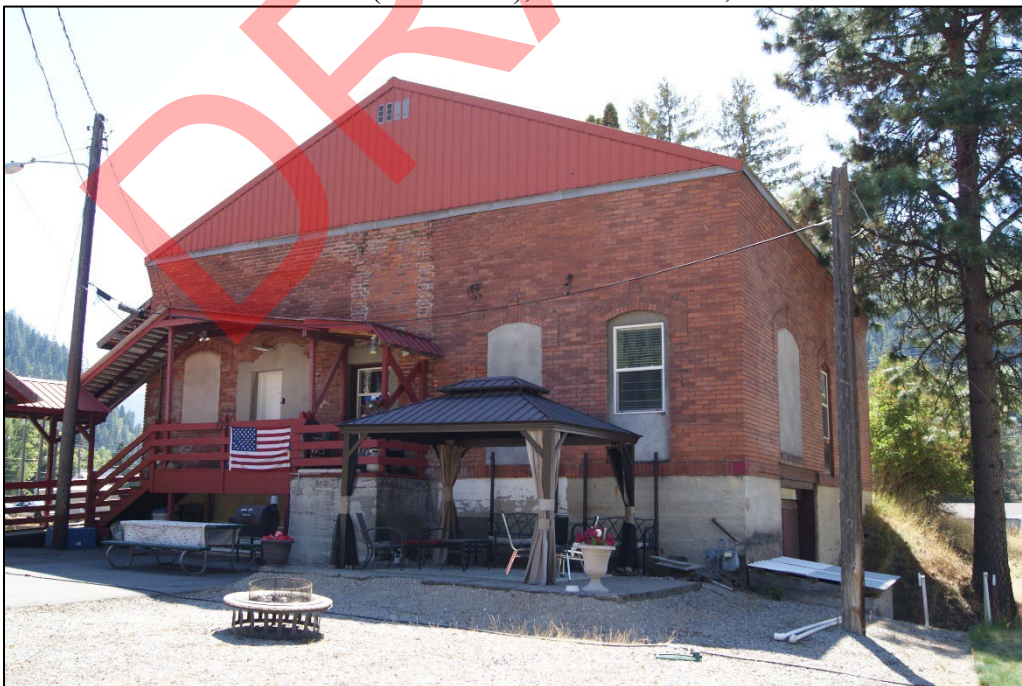
Photo 38. Steam Plant (resource 2), west and north elevations, view southeast. 2025.
