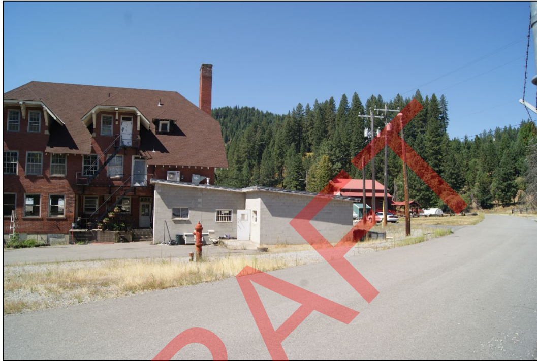
Photo 10. Infirmary (resource 1), east elevation of north wing with CMU addition, view west. 2025.
