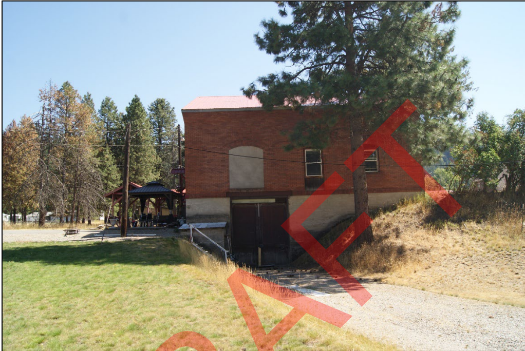
Photo 37. Steam Plant (resource 2), west elevation, view east. 2025.
