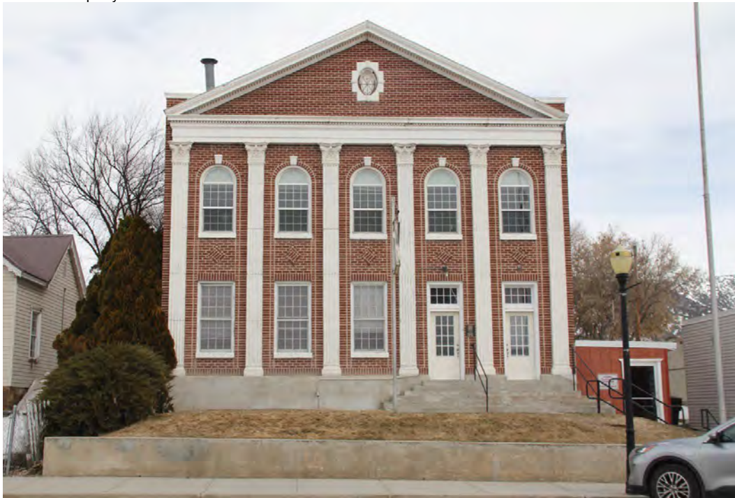
Photograph 1. Exterior, west (main) façade from Main Street. Camera facing east.
