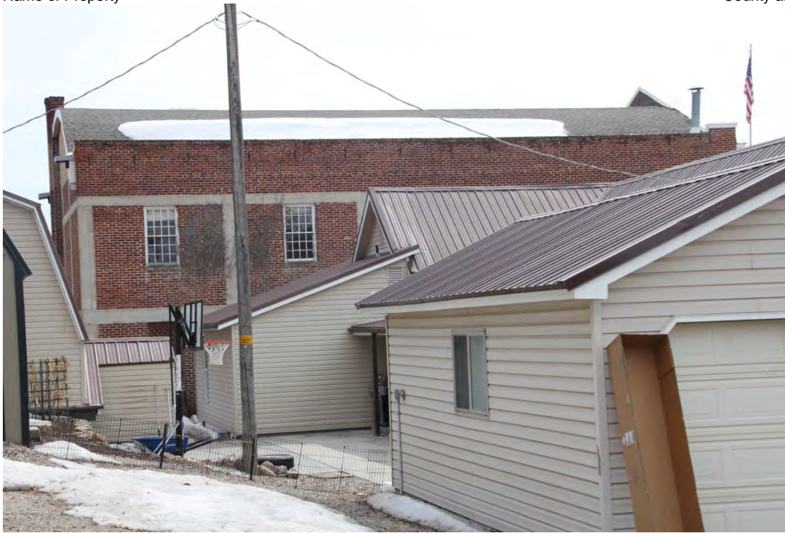
Photograph 5. Exterior, north elevation and barrel roof as seen from 100 North. Camera facing south.
