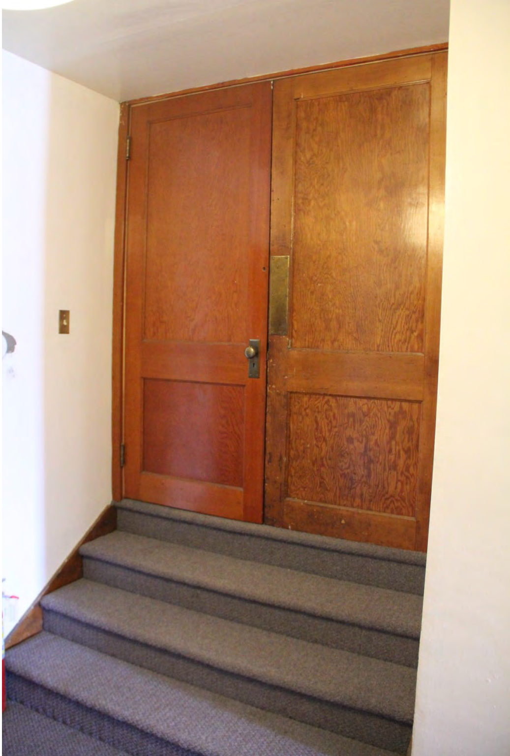
Photograph 28. Interior, First Floor, double doors in Hallway that lead to the second-floor stairway. Camera facing southeast.
