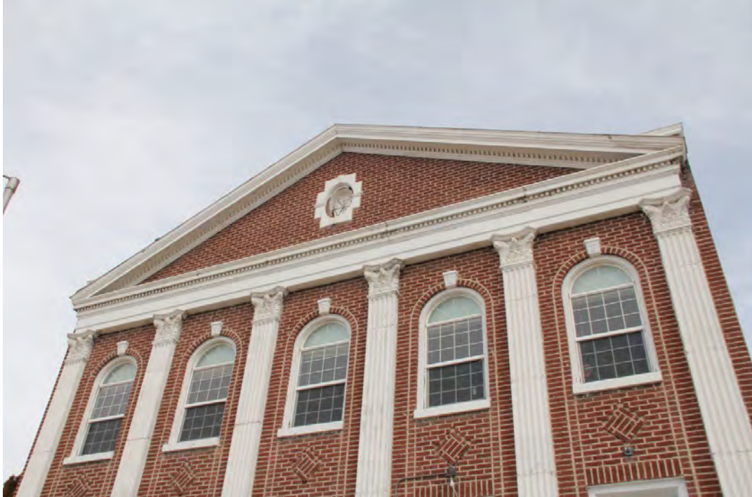
Photograph 3. Exterior, west (main) façade detail of second story and temple-front cornice. Camera facing east.
