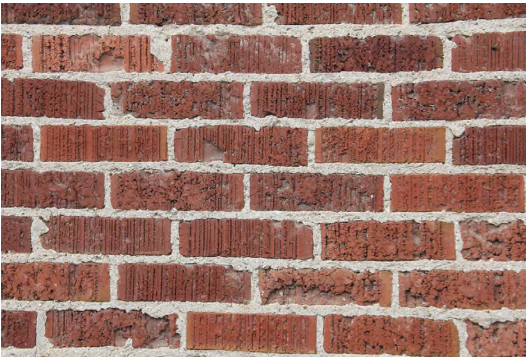
Photograph 11. Exterior, detail of brick on south elevation. Camera facing north.
