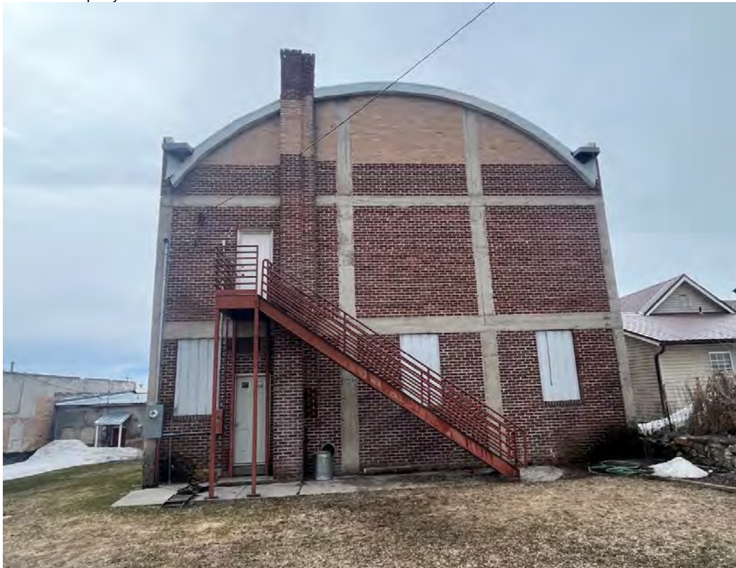
Photograph 7. Exterior, east (rear) elevation. Camera facing west.
