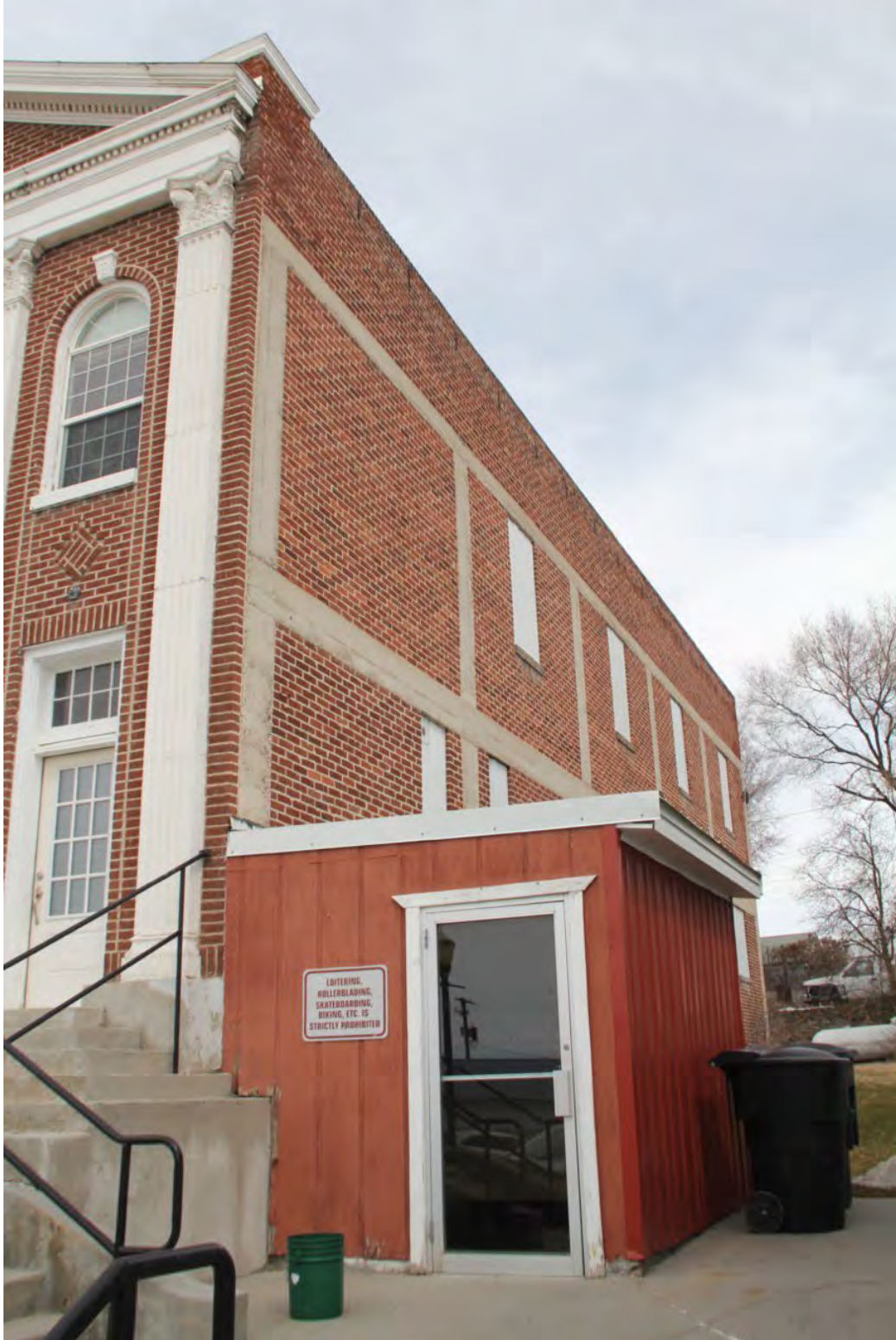
Photograph 9. Exterior, south elevation with 1977 addition enclosing stairs to the basement. Camera facing east.
