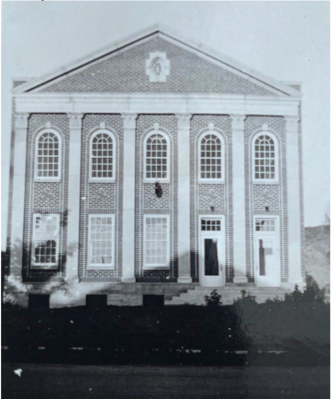
Figure 11. The American Legion Malad Post 65 ca. 1935, soon after construction was completed. Source: American Legion Post 65 archives.
