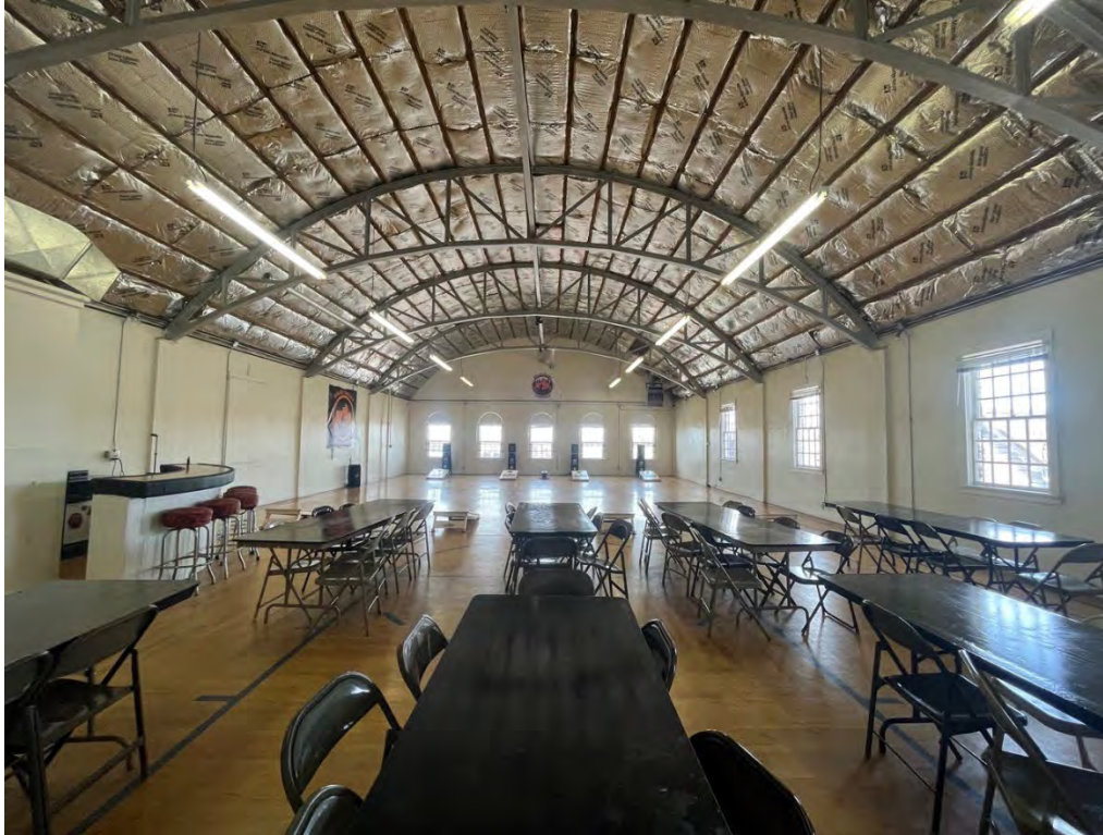
Photograph 30. Interior, Second Floor, wide view of Legion Hall. Camera facing west.
