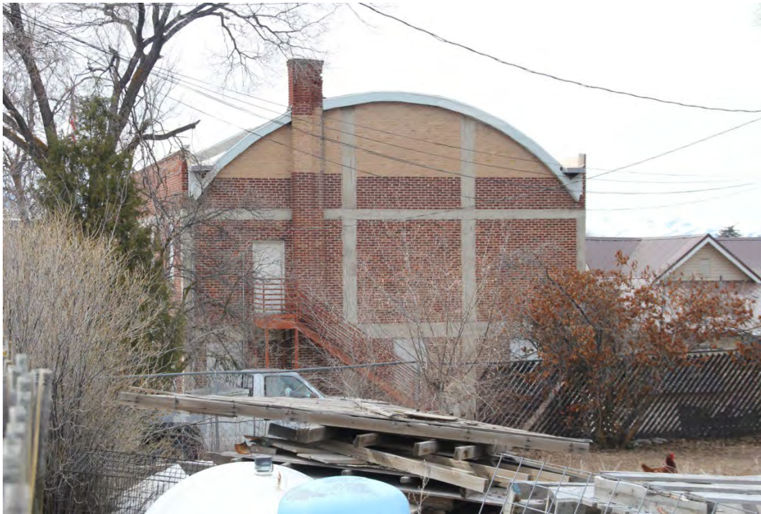
Photograph 6. Exterior, east (rear) elevation showing barrel roof. Camera facing west.
