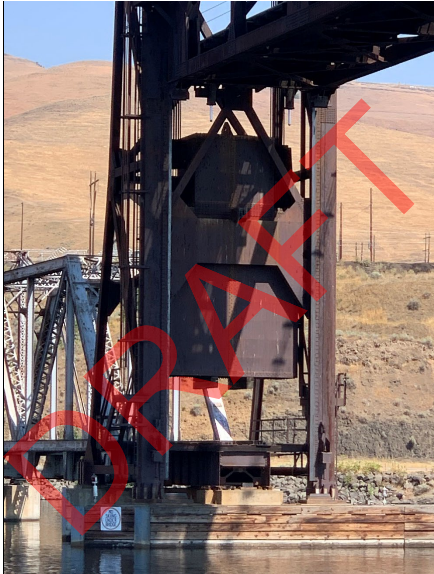
Photo 10. View looking at the northern counterweight of the vertical lift span.
