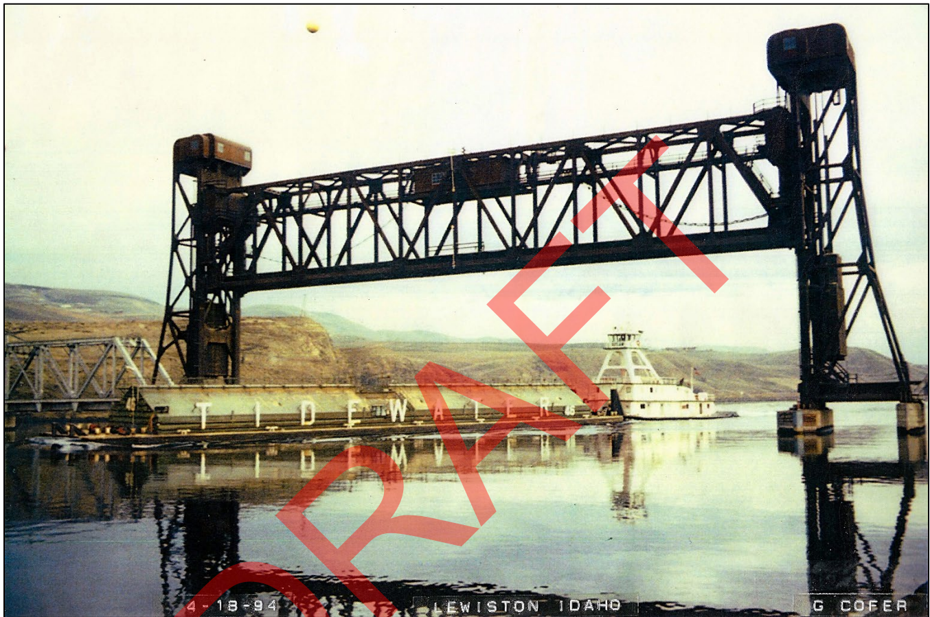
Figure 8. View looking northeast at the Clearwater River Camas Prairie Railroad Bridge's vertical lift span as a barge passes underneath, 1994. Photo courtesy of the Nez Perce County Historical Society and Museum.
