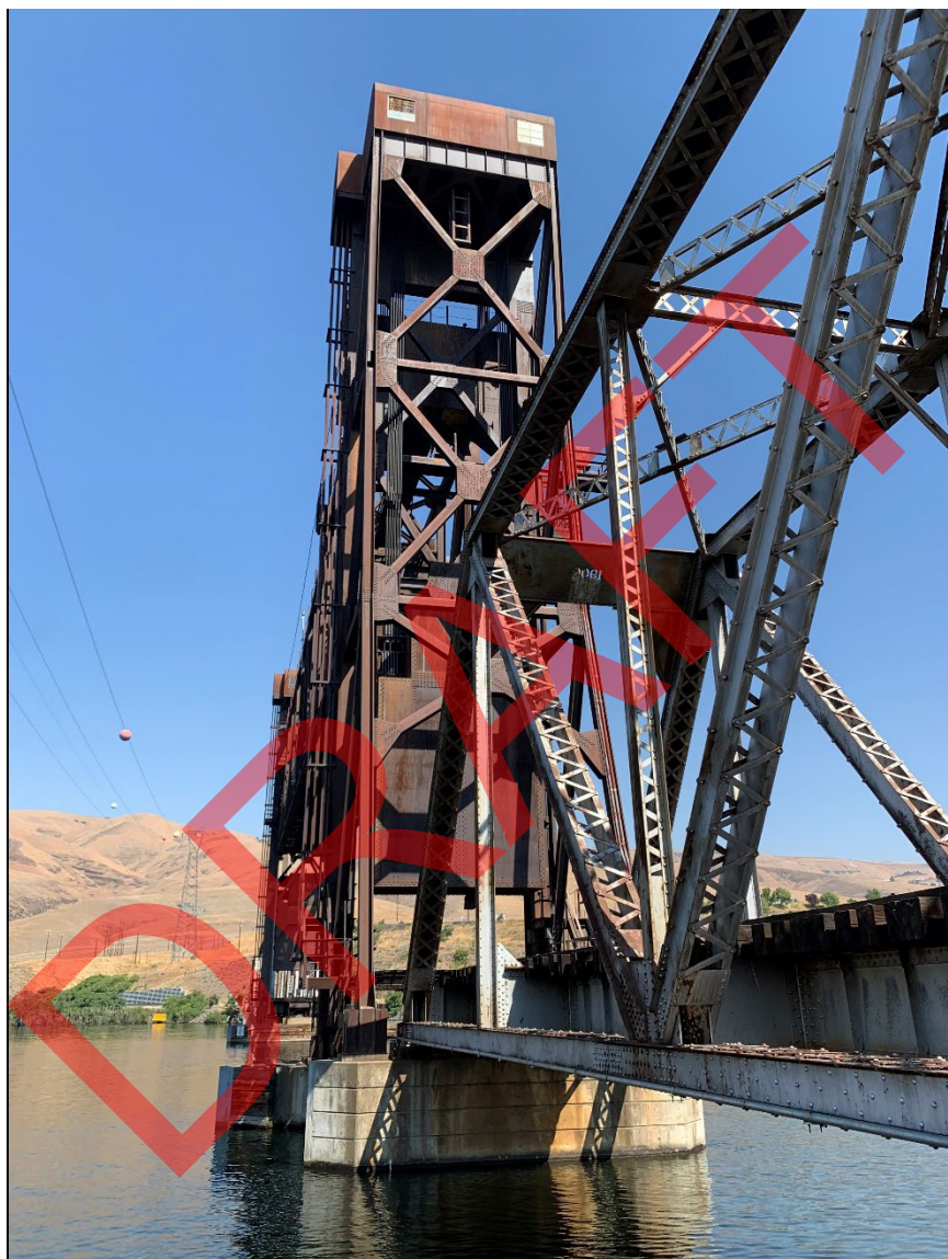
Photo 5. View looking north at the counterweights and towers of the vertical lift span.
