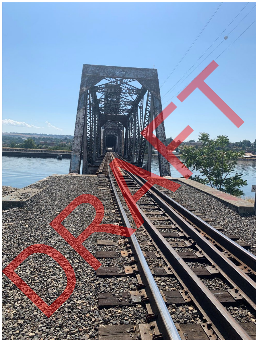
Photo 11. View looking south at the northernmost Warren truss span of the bridge.
