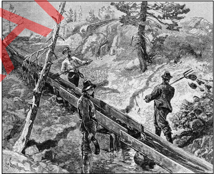
Figure 3. Miners working placers with a sluice. Illustration by Henry Sandham in The Century . Courtesy of the Library of Congress, https://www.loc.gov/pictures/item/90713942/ .
