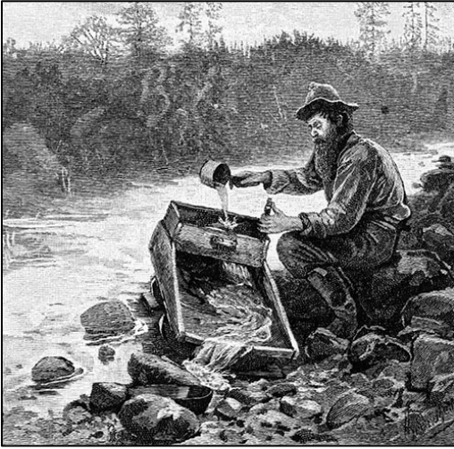
Figure 2. Miner using a rocker. Illustration by Henry Sandham in The Century . Courtesy of the Library of Congress, https://www.loc.gov/pictures/item/90713945/ .
