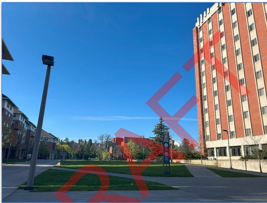
Photo 35: View of LLC Complex (10LT2276 – 2285) and Theophilus Tower (10LT2301) from Paradise Creek St., Image by Nathan J. Moody, May 1, 2025.
