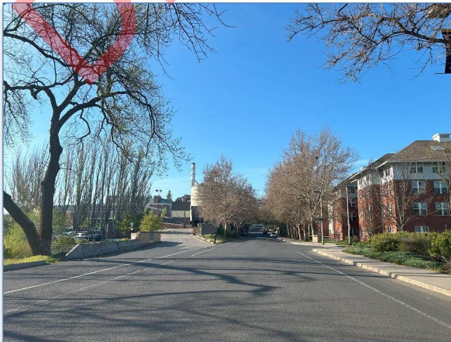
Photo 36: View of Energy Plant (10LT558) and LLC Complex (10LT2276 – 2285) from Line St., Image by Nathan J. Moody, May 1, 2025.
