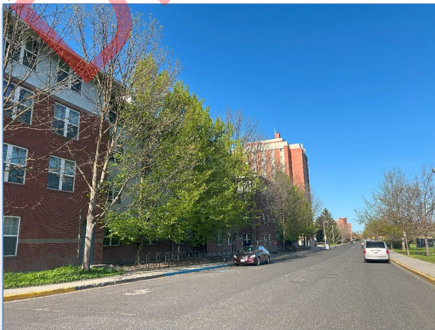
Photo 34: View of LLC Complex (10LT2276 – 2285) and Theophilus Tower (10LT2301) from Paradise Creek St., Image by Nathan J. Moody, May 1, 2025.
