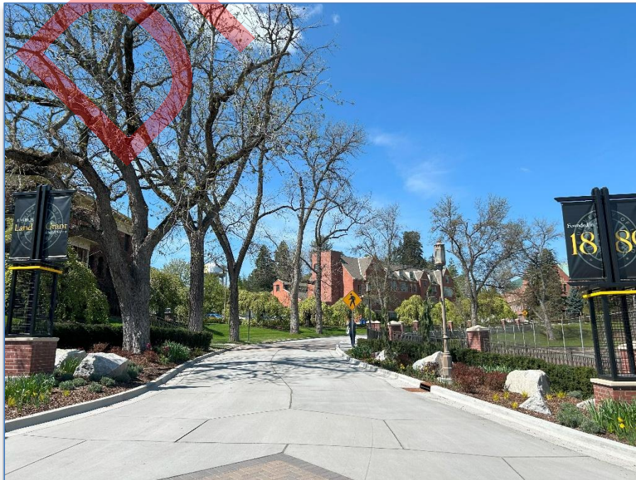
Photo 8: View from Campus Dr. and Blake Ave. Ridenbaugh Hall (10LT47) and Niccolls Home Economics Building (10LT506) in view, Image by Nathan J. Moody, April 30, 2025.
