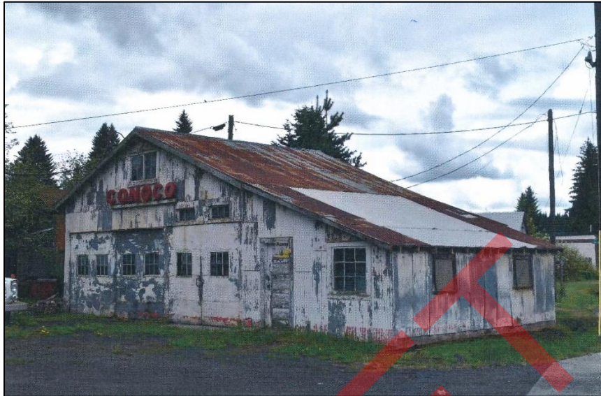
Front (north) and west side facades, looking south
