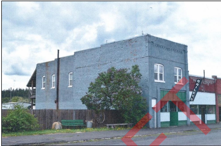
Front (north) façade, looking southwest
