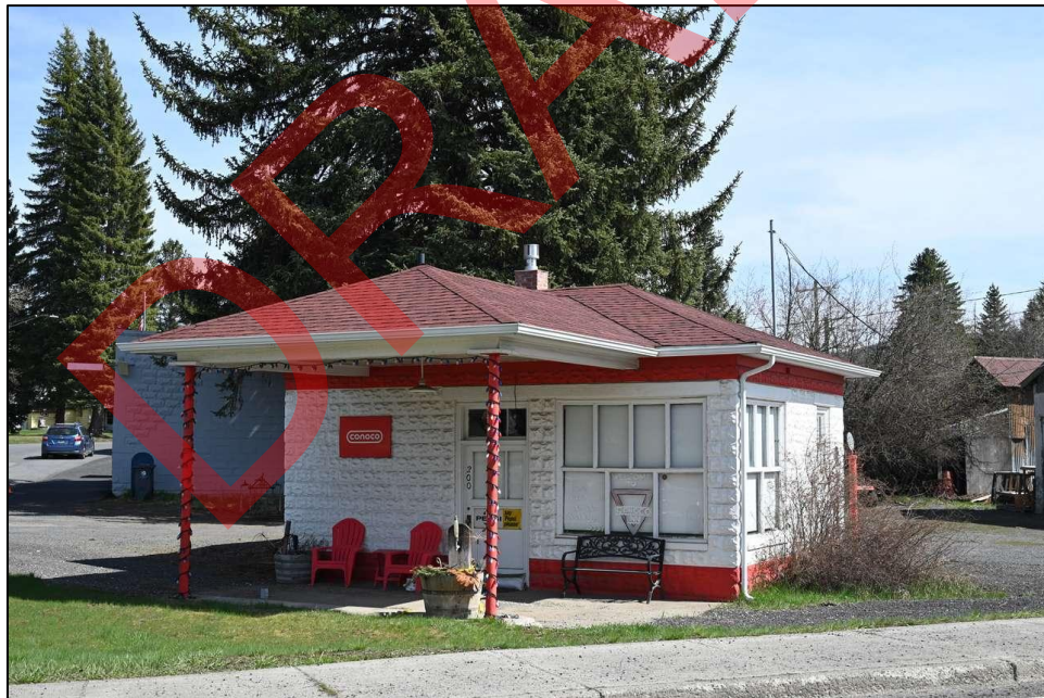
7 of 14. ID_LatahCounty_BovillHistoricCommercialDistrict_0007 Northwest and west facades, looking southeast
