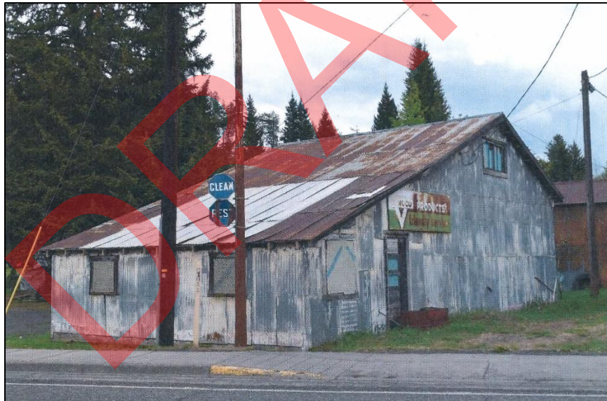
West side and rear (south) facades, looking northeast
