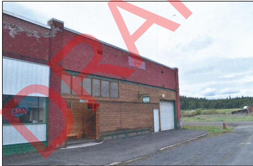
Front (north) façade, looking southwest
