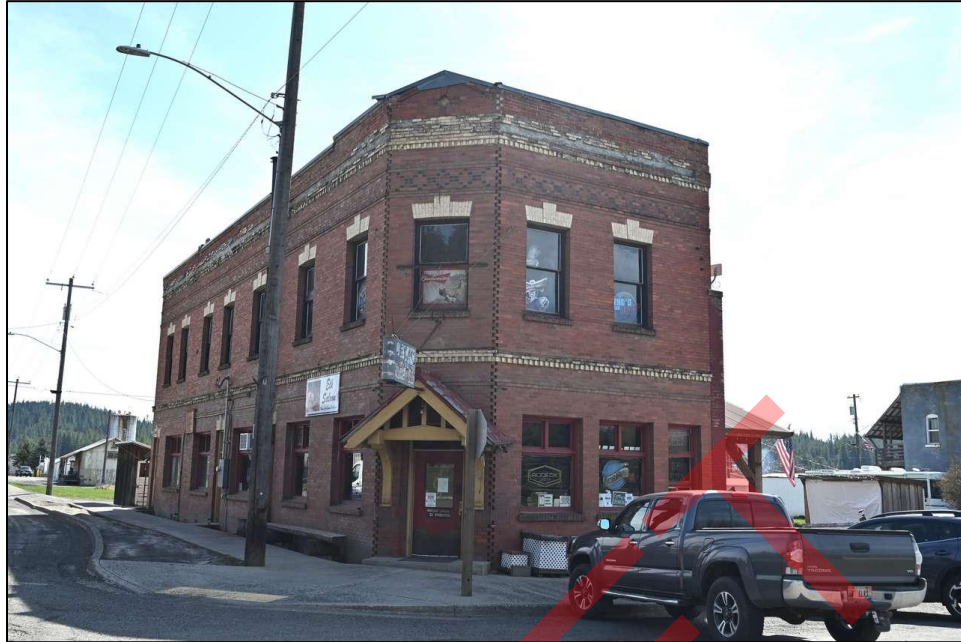
6 of 14. ID_LatahCounty_BovillHistoricCommercialDistrict_0006 East and north facades, looking southwest
