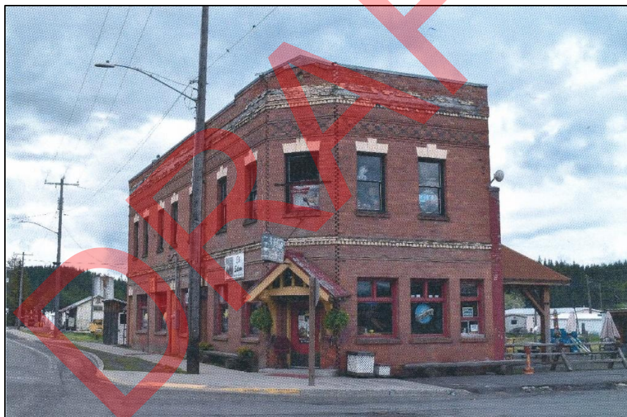
East side and front (north) facades, looking southwest
