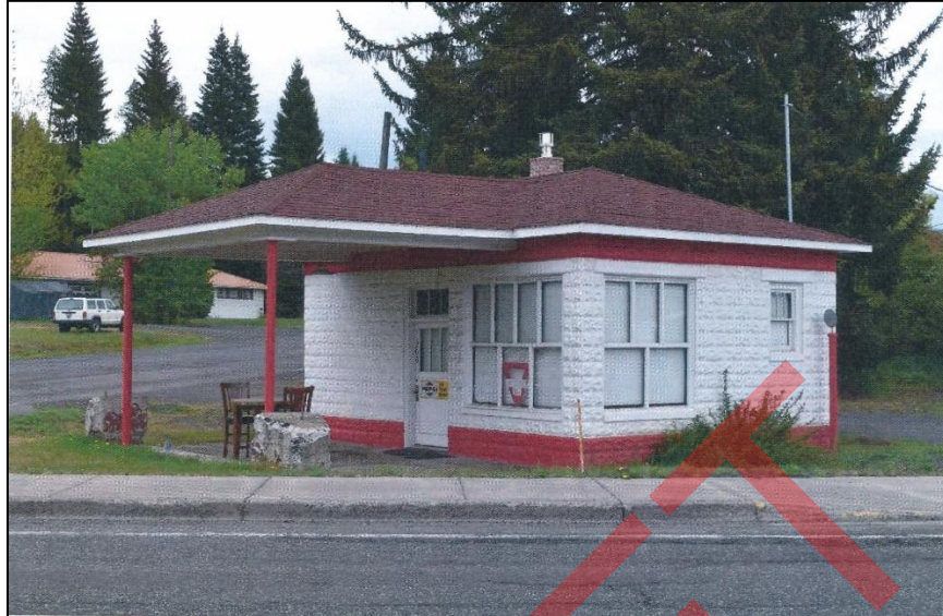
Front (northwest) and side façades, looking east
