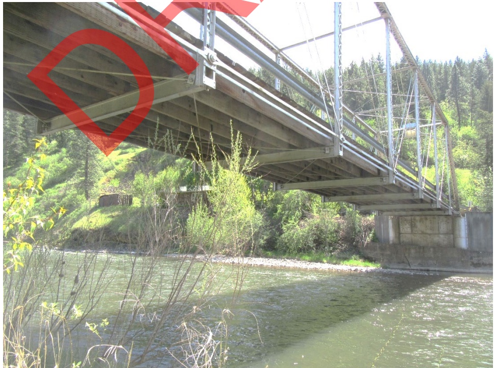
Photo 12. View of the southern abutment looking southeast.
