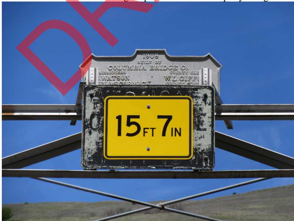
Photo 8. Detail of the Sperry Bridge sign.
