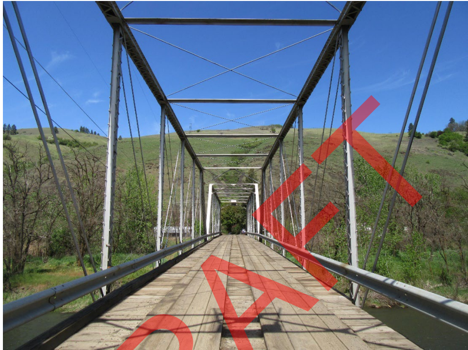
Photo 7. Detail of the bridge superstructure of the Sperry Bridge.
