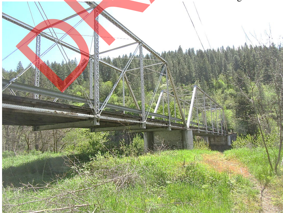
Photo 10. View of the central pier and southern abutment looking southeast.
