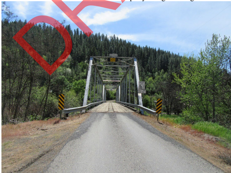
Photo 2. View of the Sperry Bridge north approach looking south.
