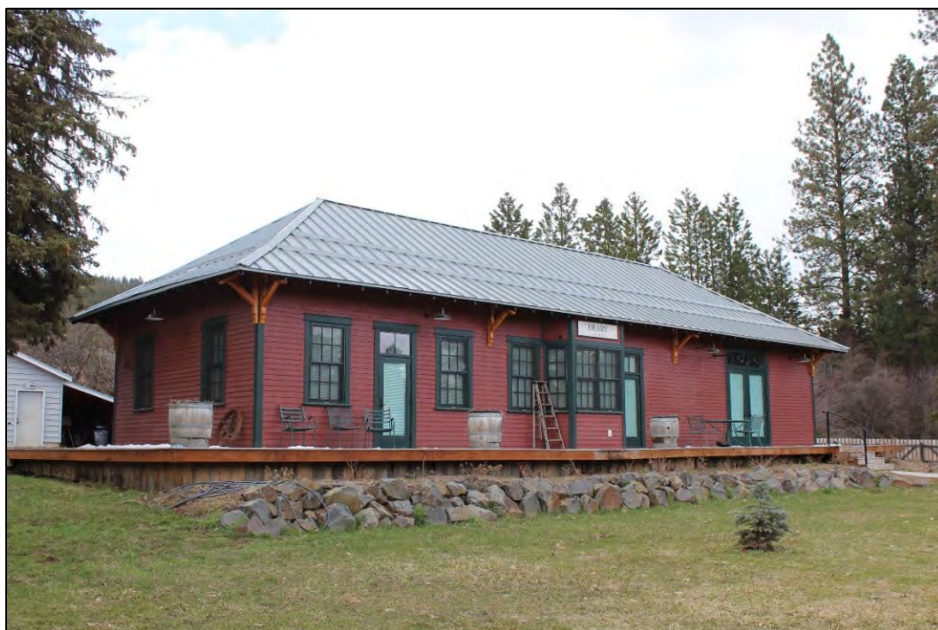
Photo 20 of 20: Refurbished and moved train depot (410 Main Street)
