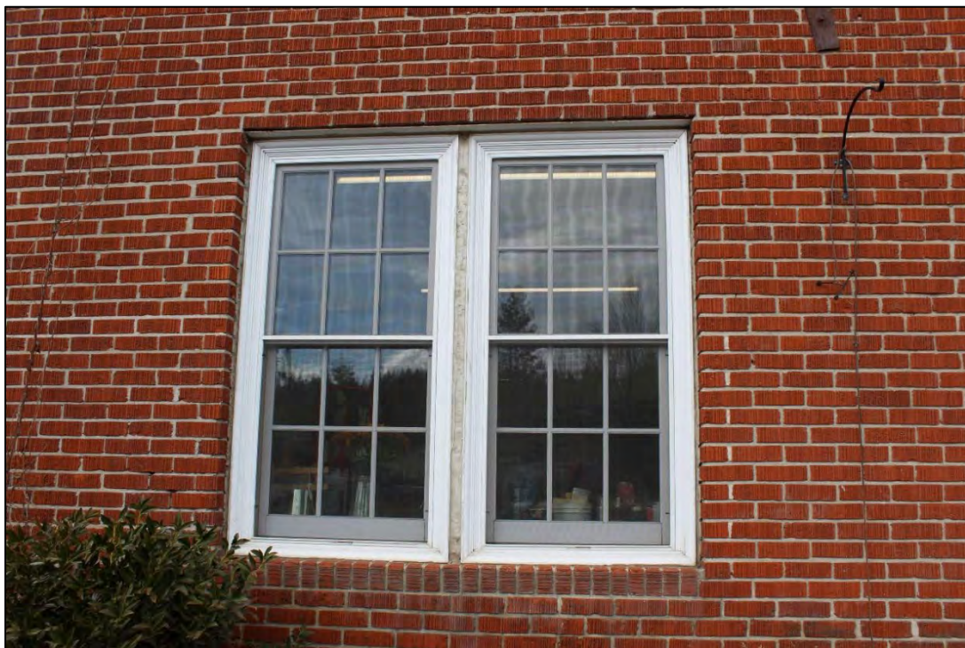
Photo 4 of 20: Windows on south elevation, typical
