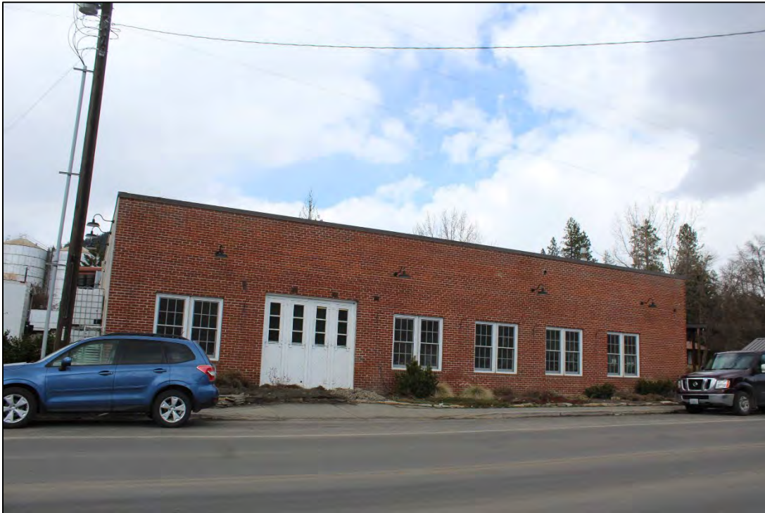
Photo 3 of 20: South elevation, looking north
