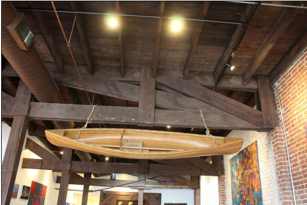
Photo 13 of 20: Truss detail, dining room, looking west
