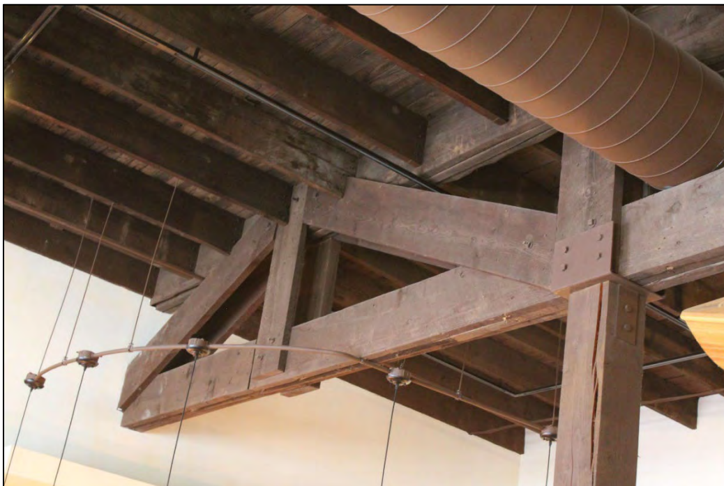
Photo 12 of 20: Truss detail, dining room, looking southwest
