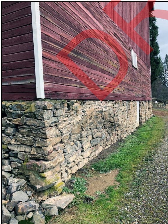
Photo 4. Wood barn, detail view of stone foundation, south end, view to north.
