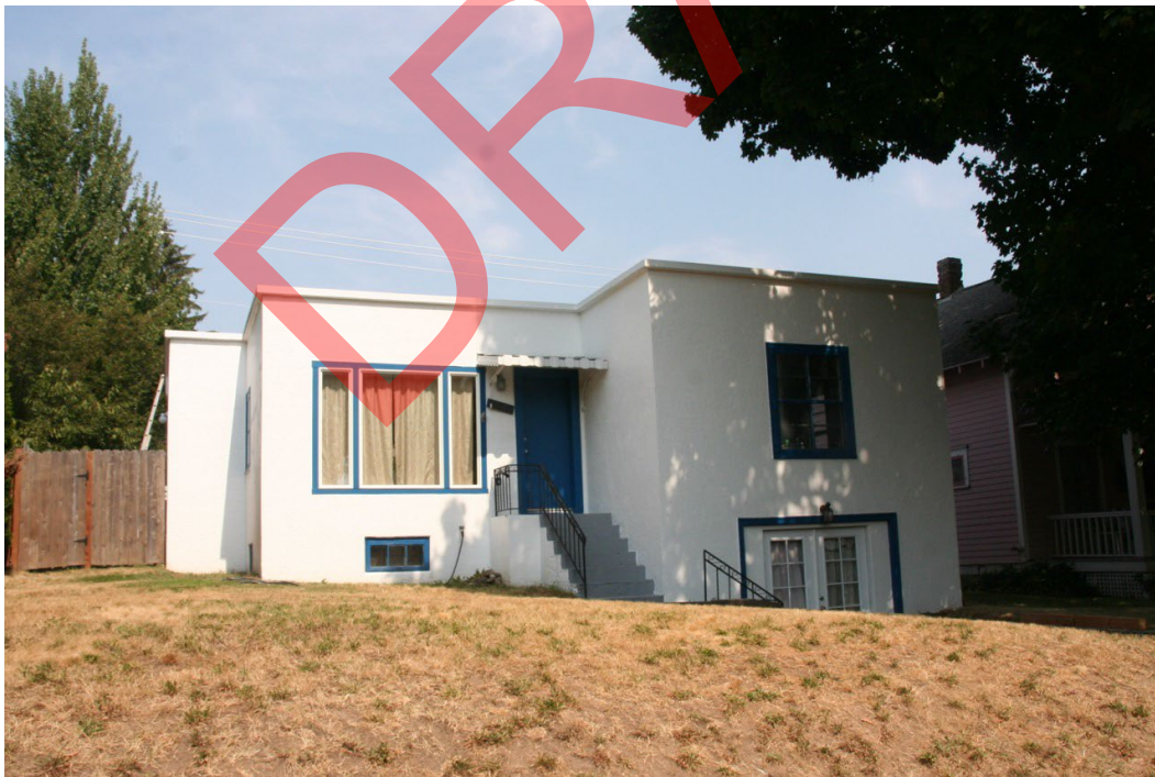
90. Example of the International style at 1011 E. Lakeside Ave. prior to non-contributing alterations. Camera facing north.
