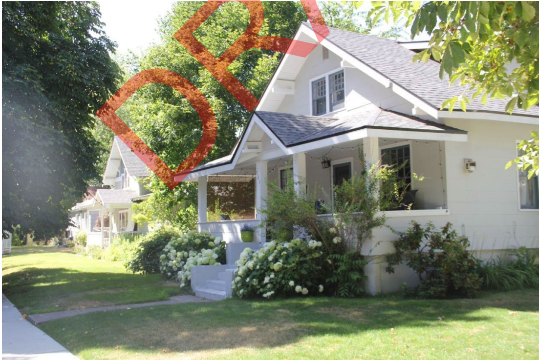
33. North side of Indiana Ave. at 8th St. Camera facing northwest.
