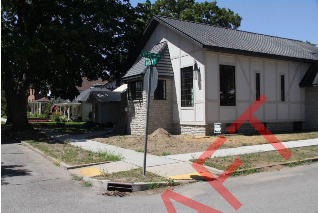
25. Renovated former church at 521 E. Garden Ave. Camera facing northwest.
