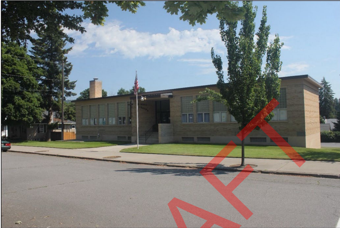
91. Example of the International style at 406 N. 10th St. Camera facing east.
