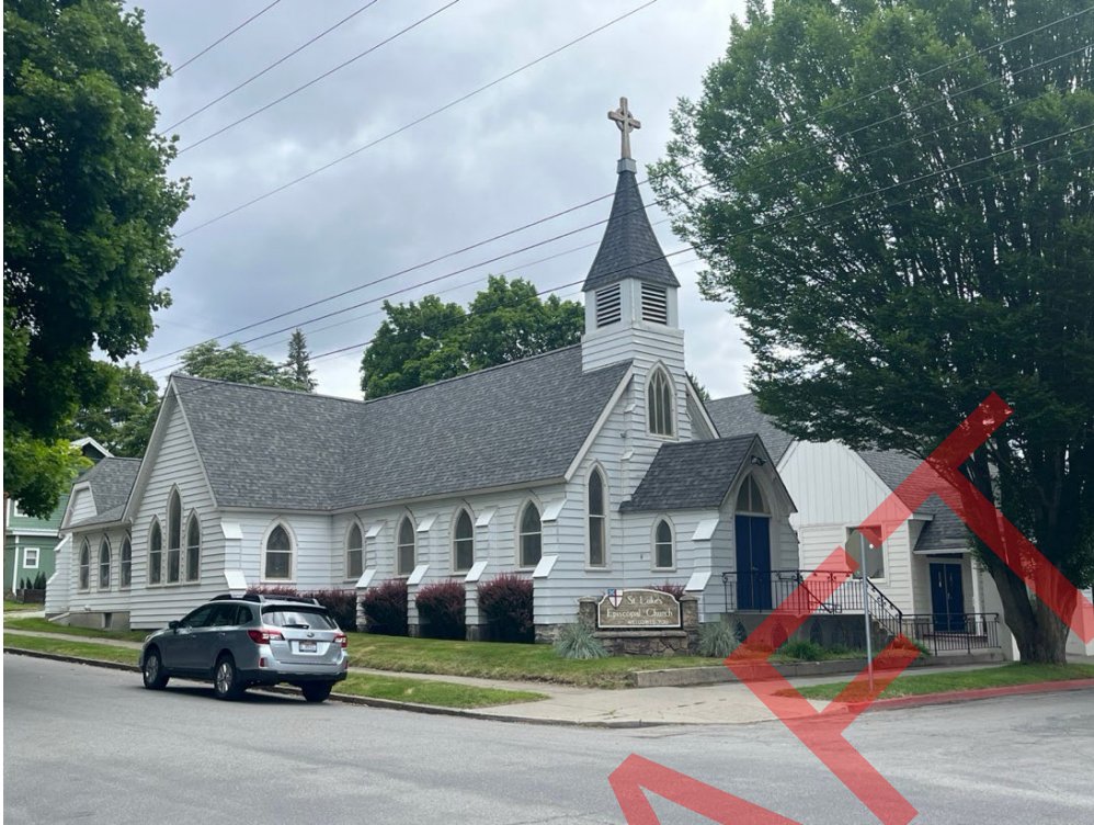
63. Example of the Gothic Revival style at 501 E. Wallace Ave. Camera facing northeast.
