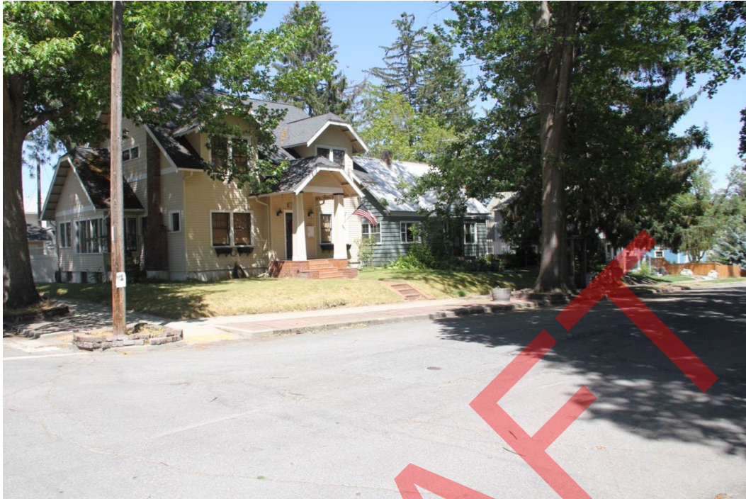
42. North side of Coeur d'Alene Ave. at 10th St. Camera facing northeast.
