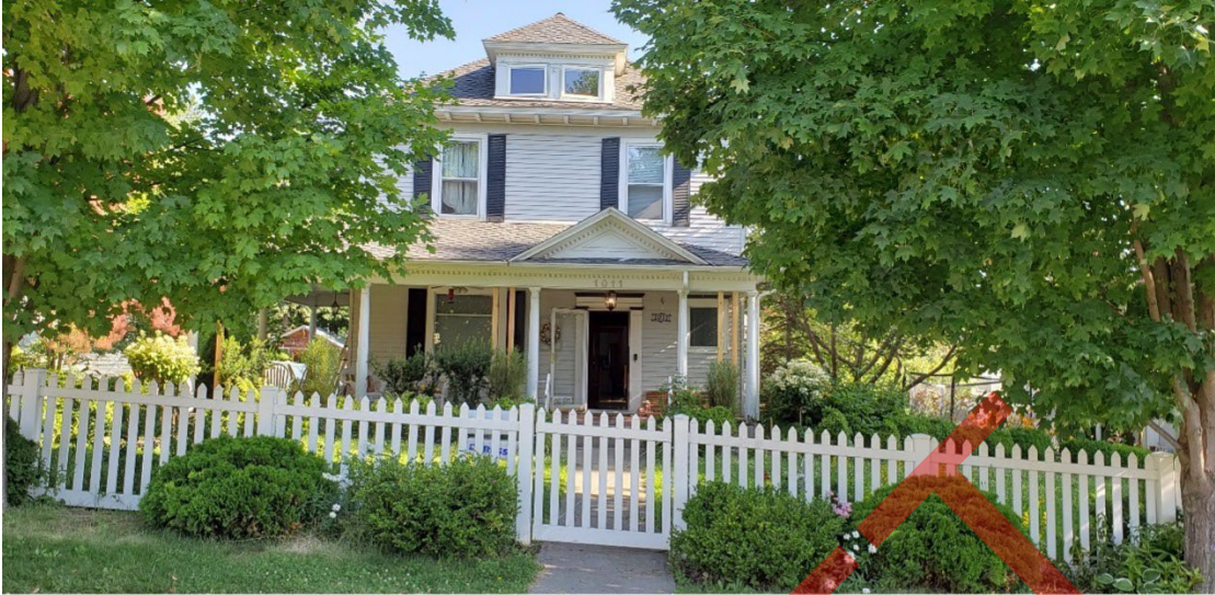
55. Example of the Colonial Revival style at 1011 E. Garden Ave. (to be replaced) Camera facing north.
