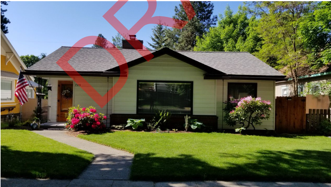
92. Example of Ranch style at 706 E. Garden Ave. Camera facing south.
