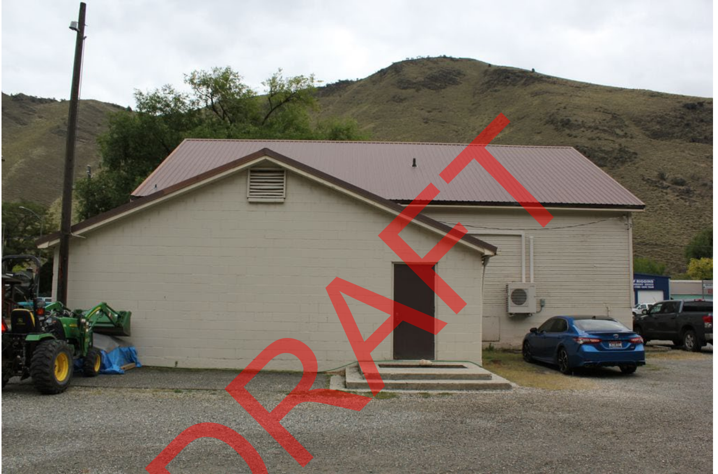
Photo 6 of 21. ID_IdahoCounty_RigginsHighSchool_0006 Rear (northwest) elevation and addition, looking southeast.
