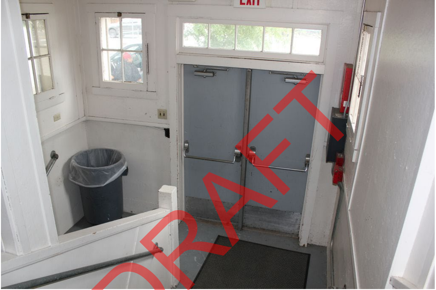
Photo 12 of 21. ID_IdahoCounty_RigginsHighSchool_0012 Interior at the primary entrance.
