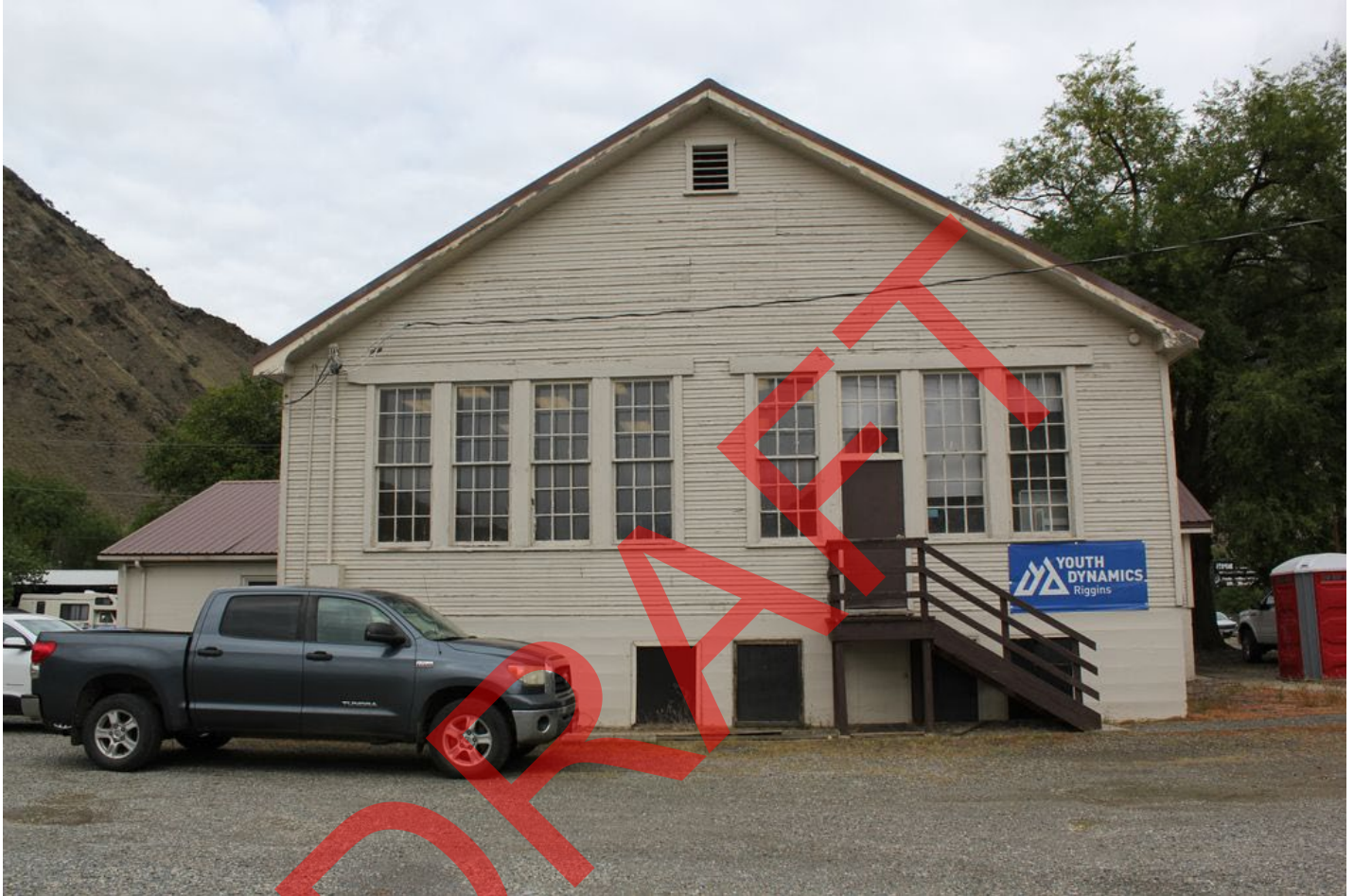
Photo 8 of 21. ID_IdahoCounty_RigginsHighSchool_0008 Side (southwest) elevation, facing northeast.
