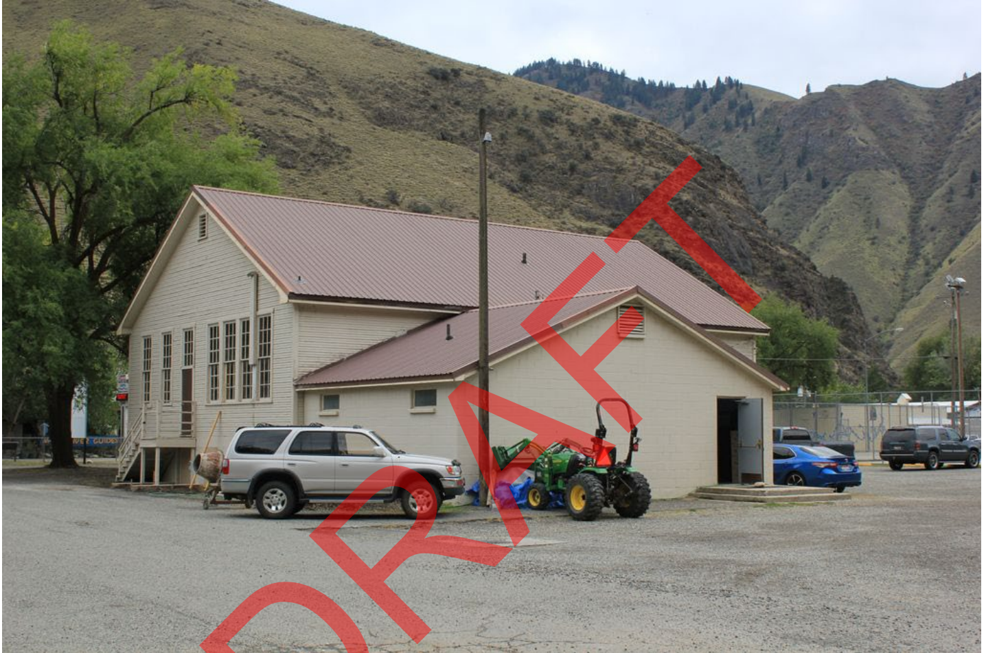
Photo 5 of 21. ID_IdahoCounty_RigginsHighSchool_0005 Overall view of the rear of the school from the north, looking south.
