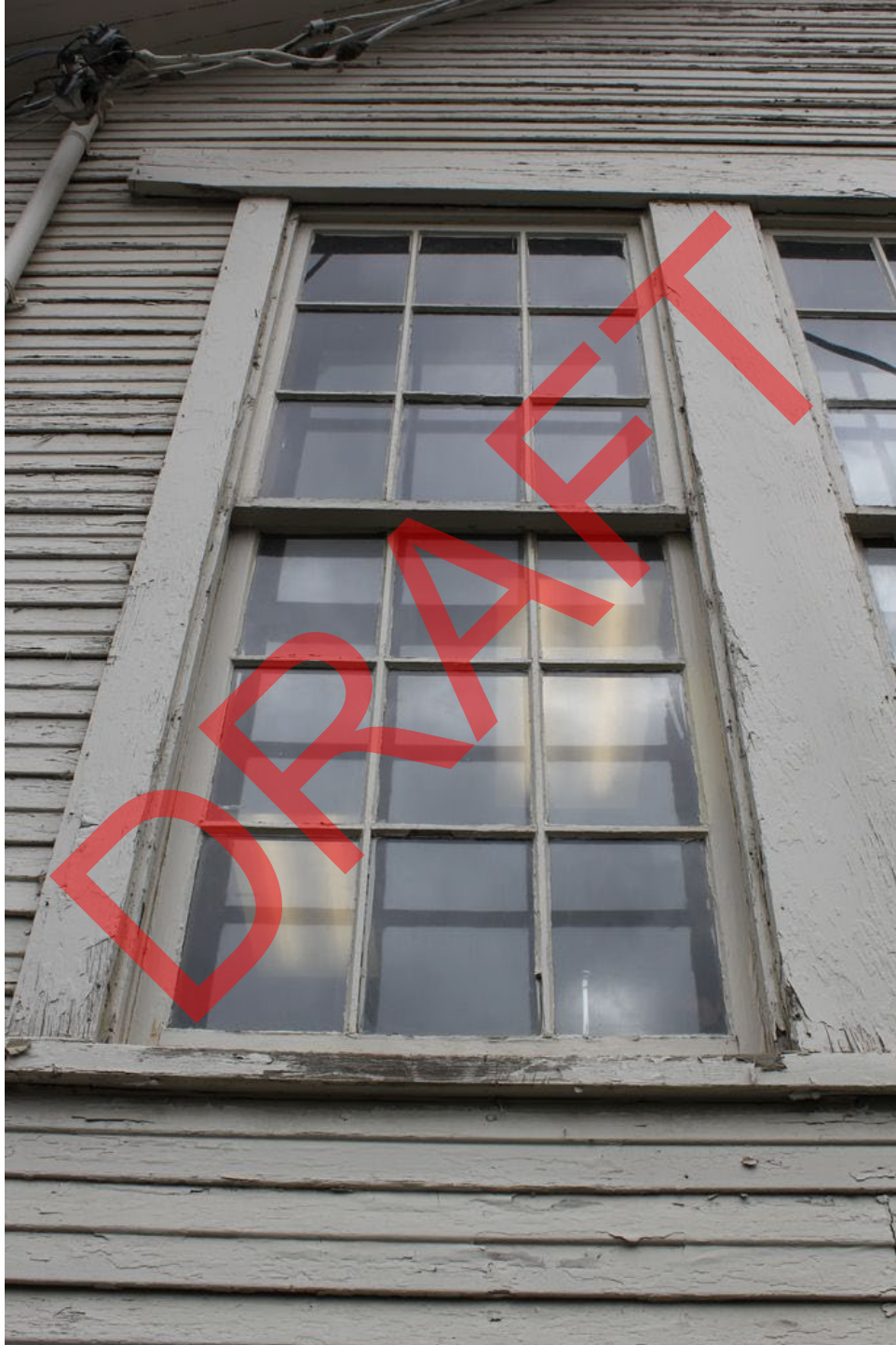
Photo 11 of 21. ID_IdahoCounty_RigginsHighSchool_0011 Close-up of a window on southeast façade.
