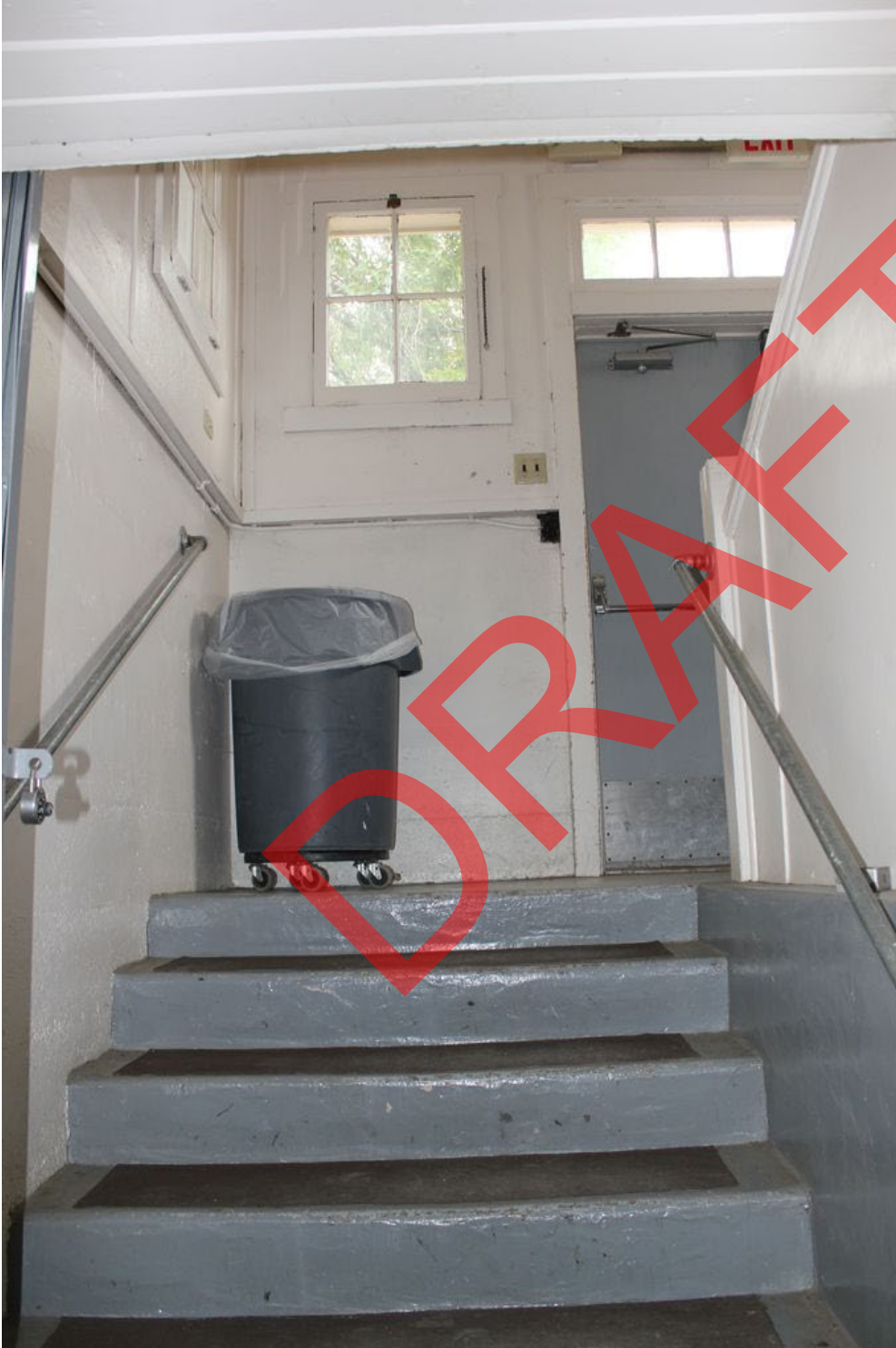
Photo 19 of 21. ID_IdahoCounty_RigginsHighSchool_0019 Stairs leading from primary entry vestibule to basement.
