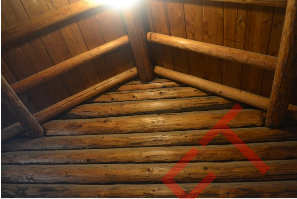
Photo 25: Detail of roof rafter joinery in entrance vestibule, facing north.
