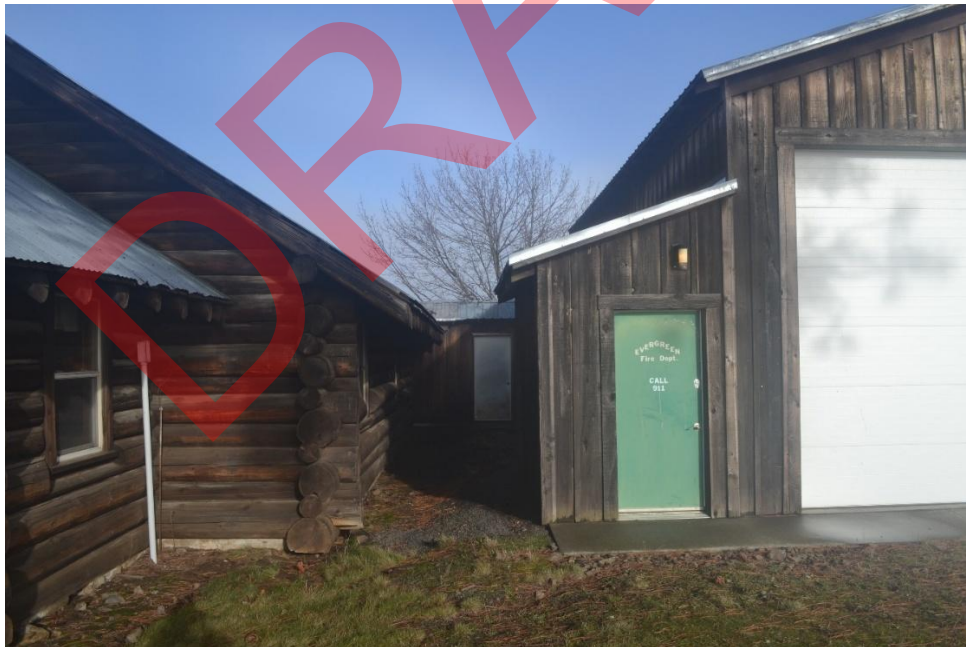
Photo 18: Front elevation showing "hyphen" connection between buildings, facing north.
