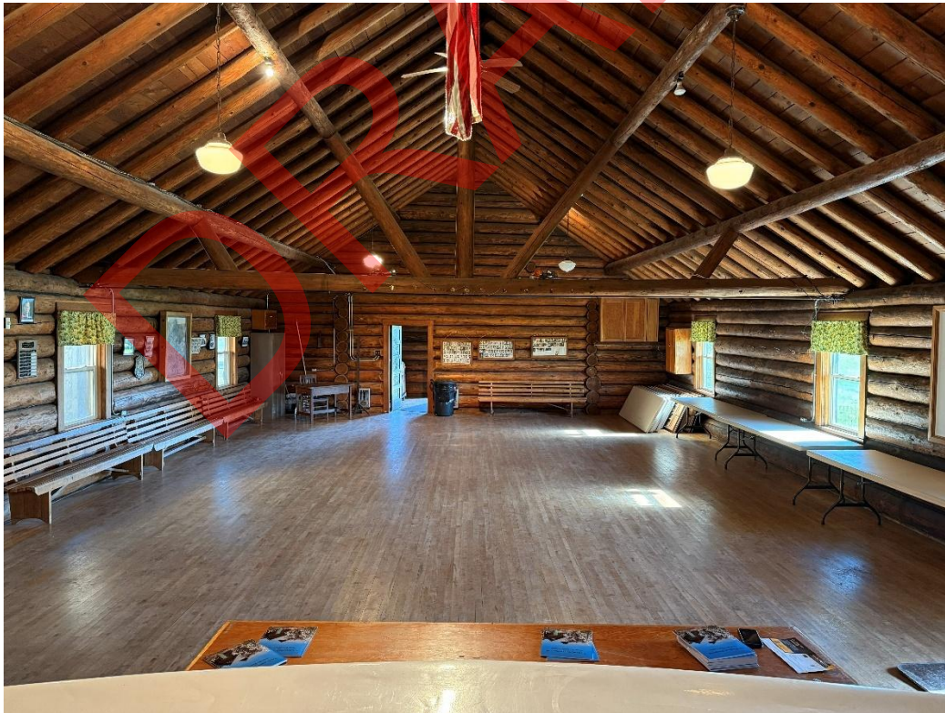
Photo 32: Interior of Evergreen Grange Hall, facing south from the stage. (DE photo)
