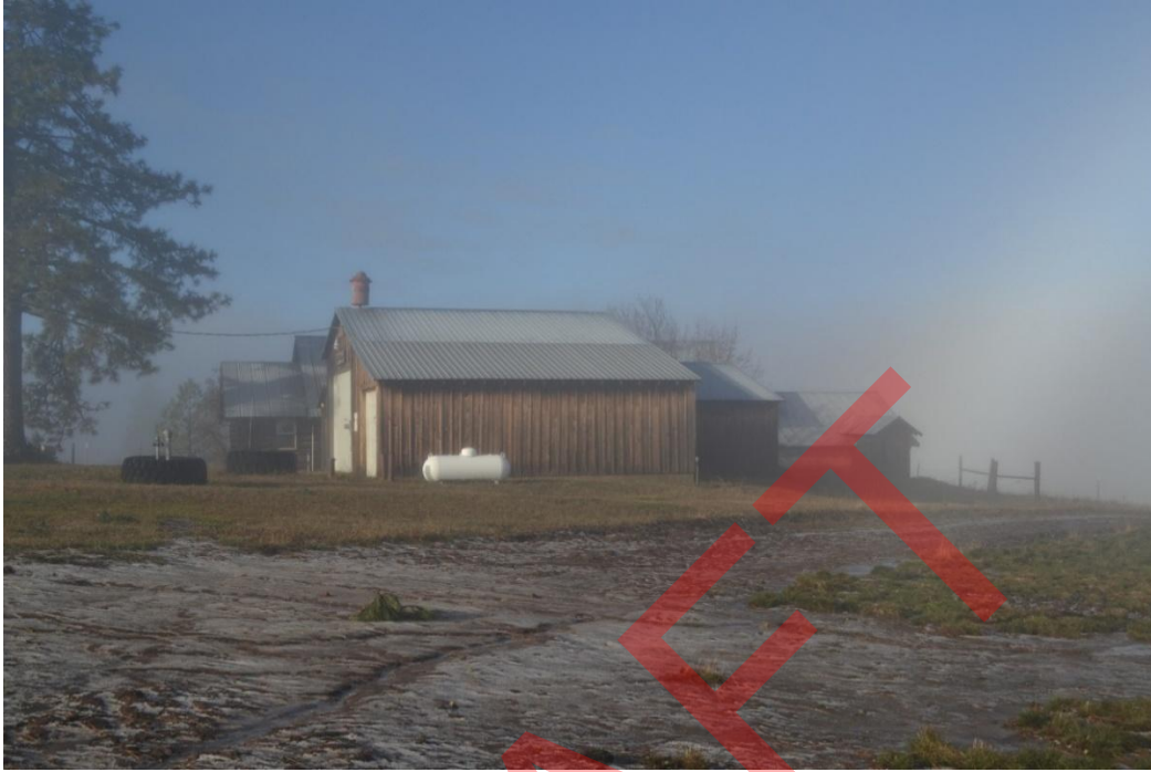
Photo 15: Side elevation, facing west.
