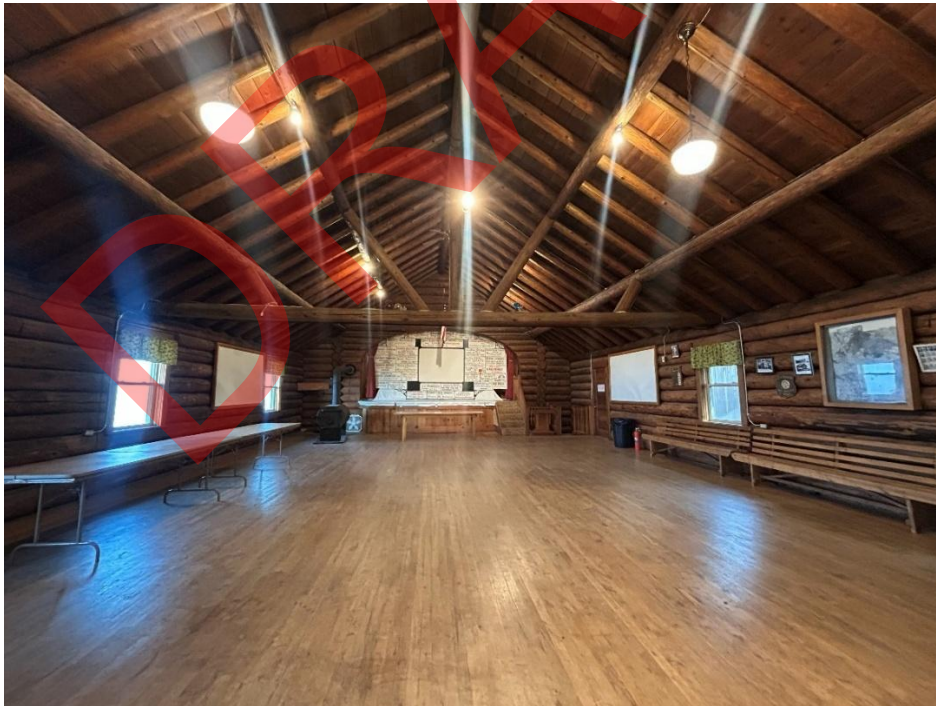
Photo 28: Interior of Evergreen Grange Hall, facing north.
