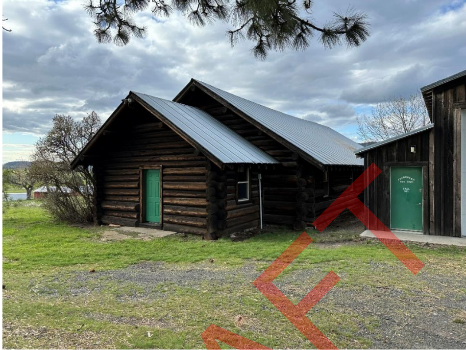
Photo 17: Front elevation, facing north.
