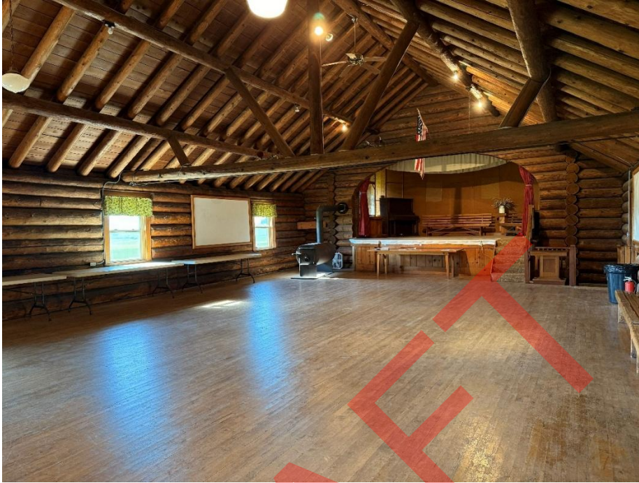
Photo 27: Interior of Evergreen Grange Hall, facing north by northwest. (DE photo)
