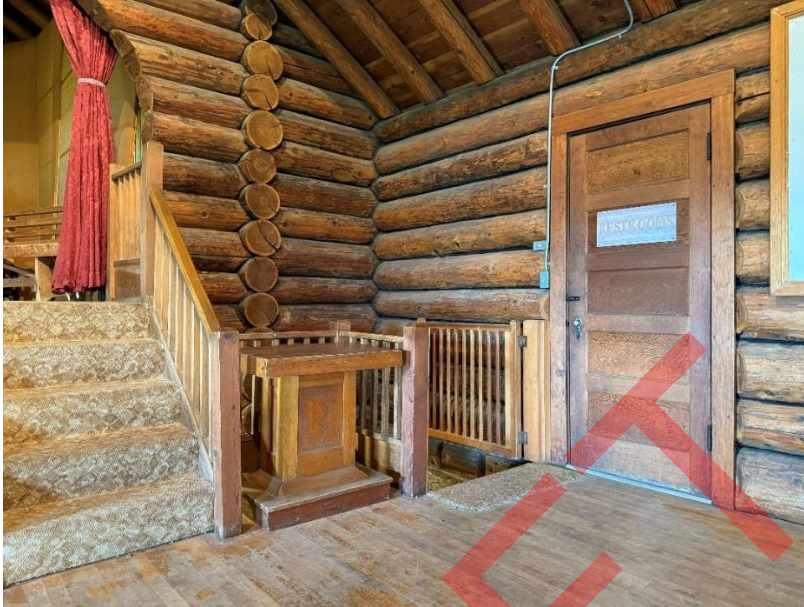
Photo 39: From left to right, stage stairs, stairs to basement, and door to bathrooms, facing northeast. (DE photo)
