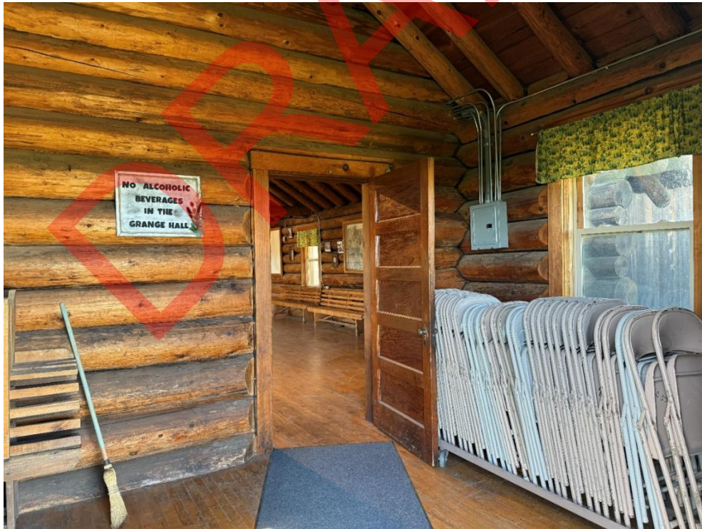
Photo 22: Entrance vestibule, facing north by northwest. (DE photo)
