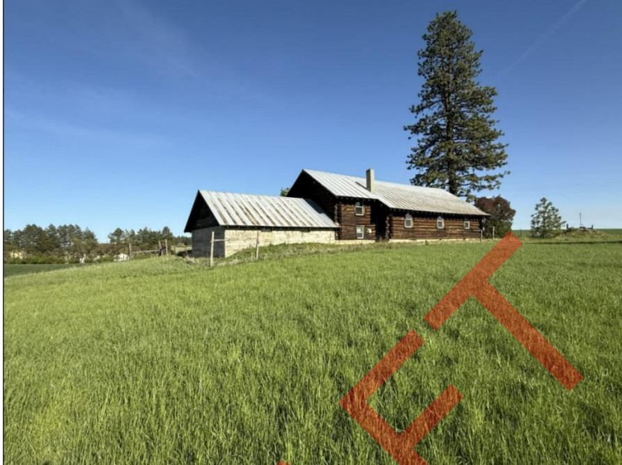
Photo 7: Side elevation, facing east by southeast. (DE photo)
