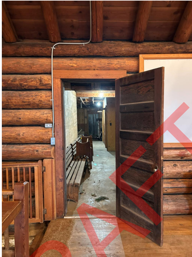
Photo 59: Door from Evergreen Grange Hall to hallway to restrooms, facing east.
