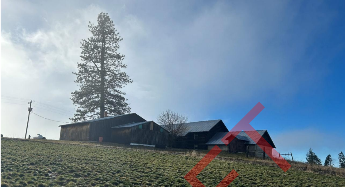
Photo 9: Rear elevation, facing southwest.
