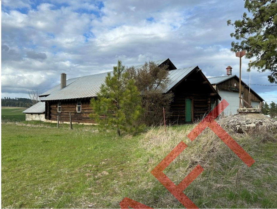
Photo 5: Side elevation, looking northeast (DE photo)
