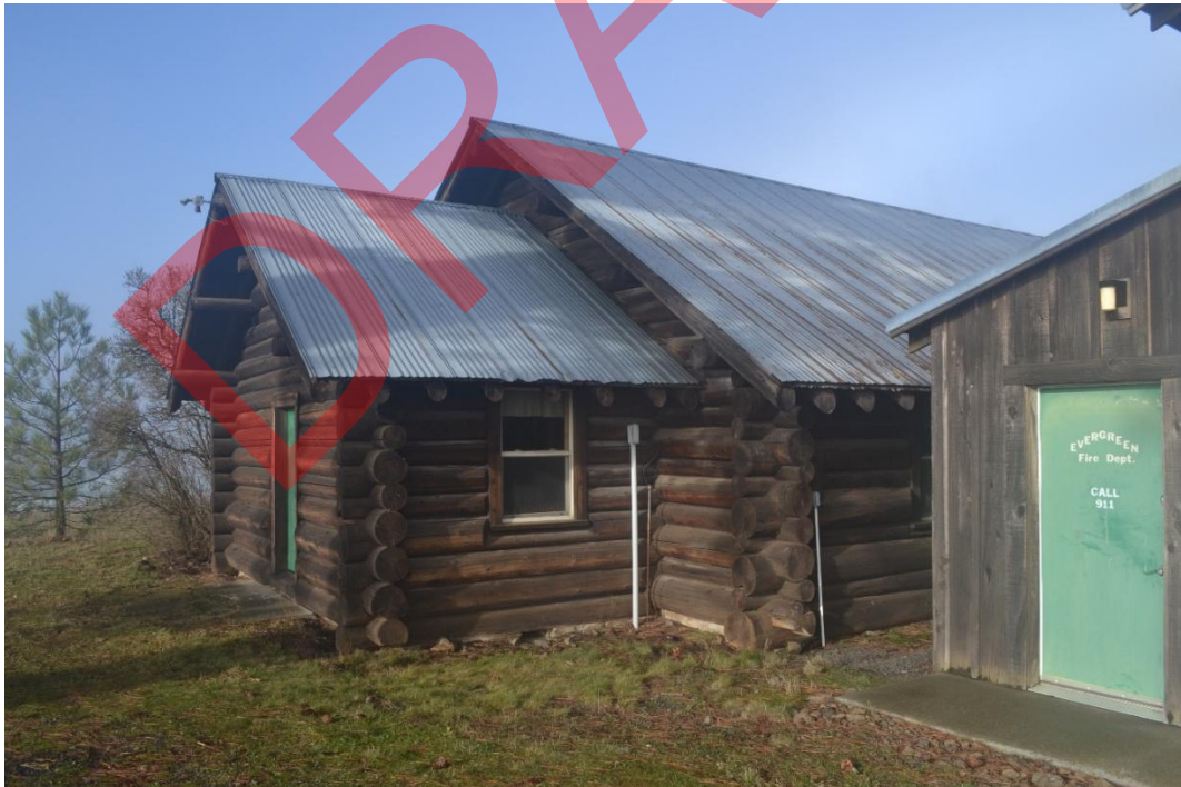
Photo 20: Front façade, facing west by northwest.
