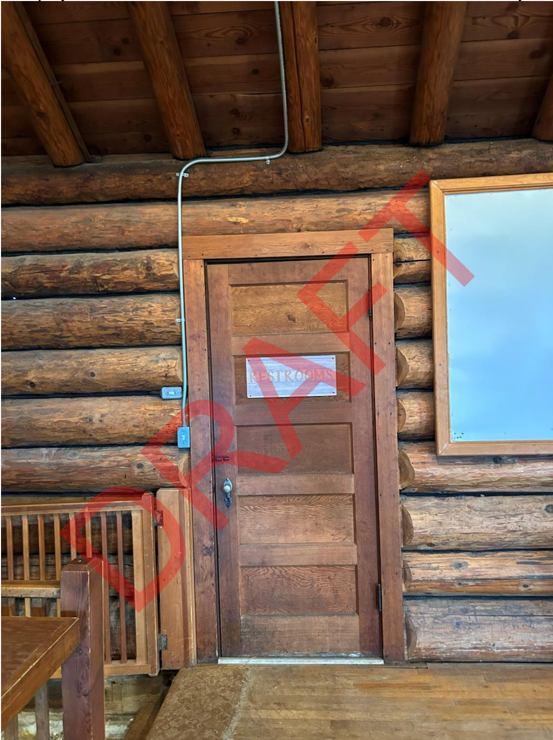
Photo 44: Door on east wall of Evergreen Grange Hall leading to restrooms.
