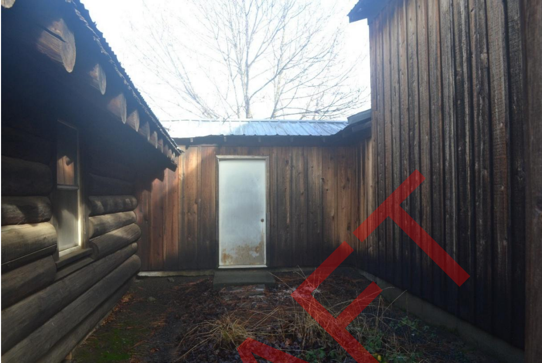
Photo 19: Detail of hyphen connection between buildings, facing north.
