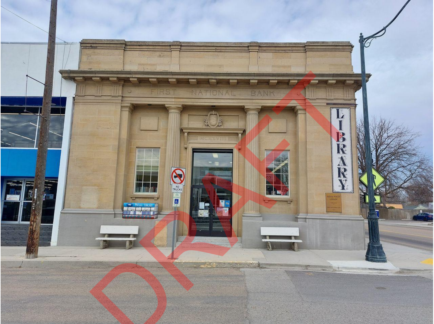
Photo 1 of 24. ID_Canyon_ParmaStateBank_0001 View of primary east elevation, camera facing west
