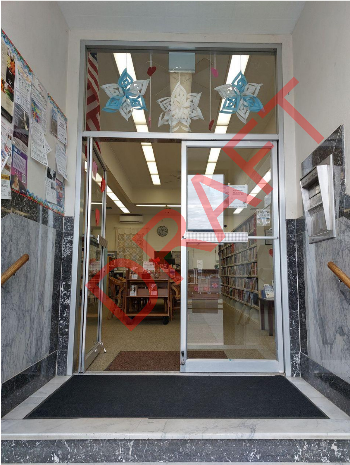
Photo 10 of 24. ID_Canyon_ParmaStateBank_0010 View of vestibule interior, camera facing west
