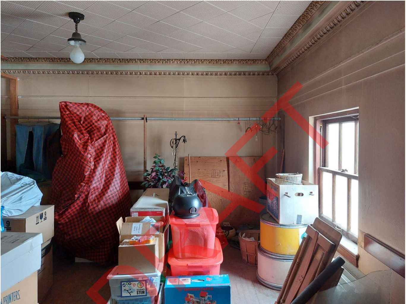
Photo 19 of 24. ID_Canyon_ParmaStateBank_0019 View of mezzanine level at the southwest corner, camera facing south
