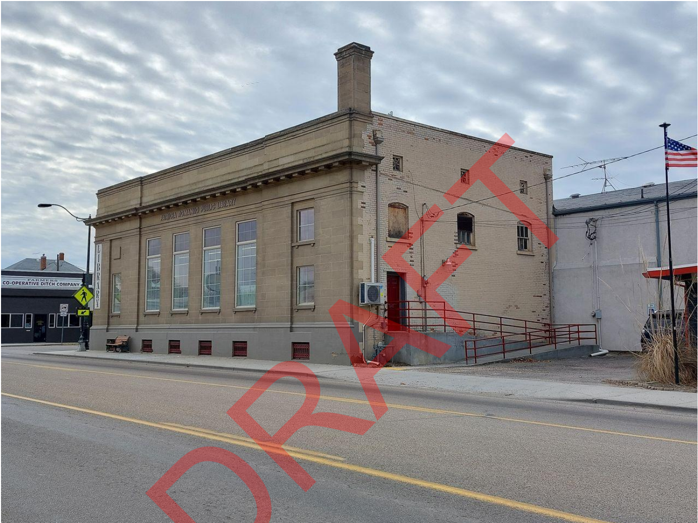
Photo 4 of 24. ID_Canyon_ParmaStateBank_0004 View of north (side) and west (rear) elevations, camera facing southeast
