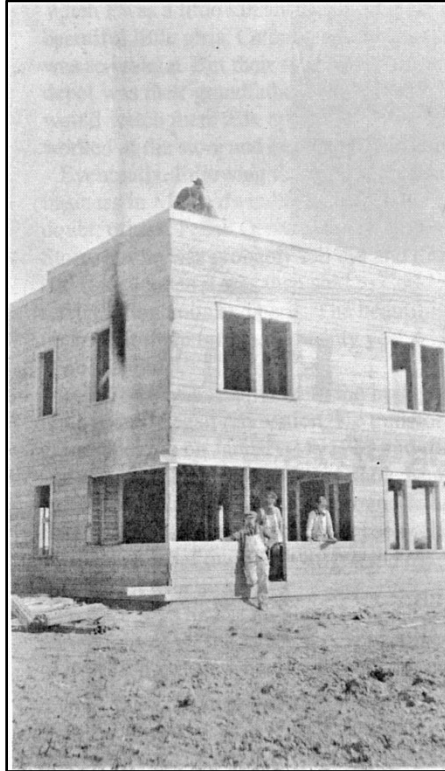
Figure 6. Gardner Hotel under construction, 1919.
