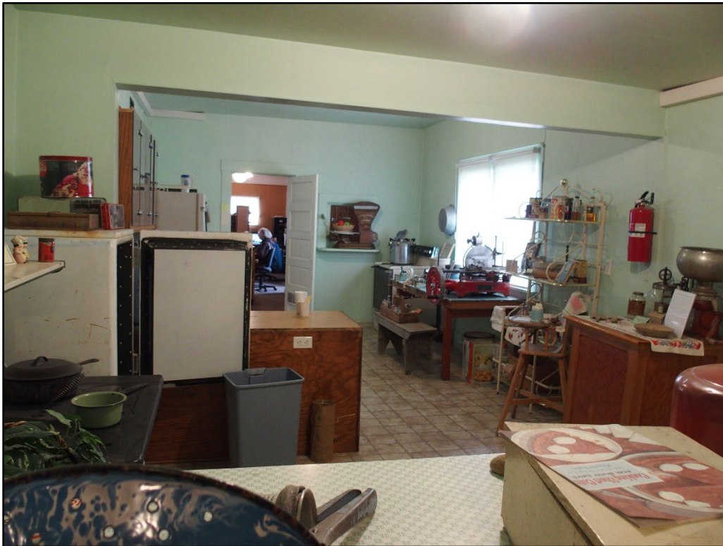
Photograph 14. Interior, first floor, kitchen, camera facing west.
