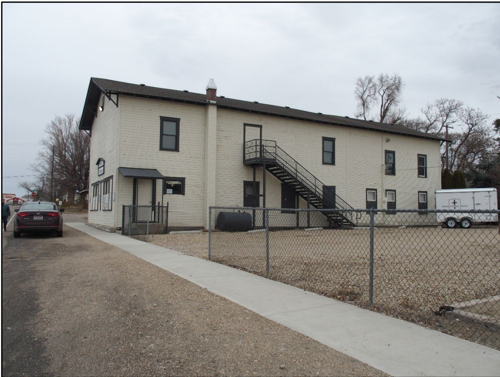
Photograph 8. Façade (left) and south elevations, view looking northeast.
