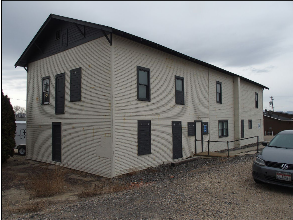
Photograph 5. East (left) and north (right) elevations, camera facing southwest.
