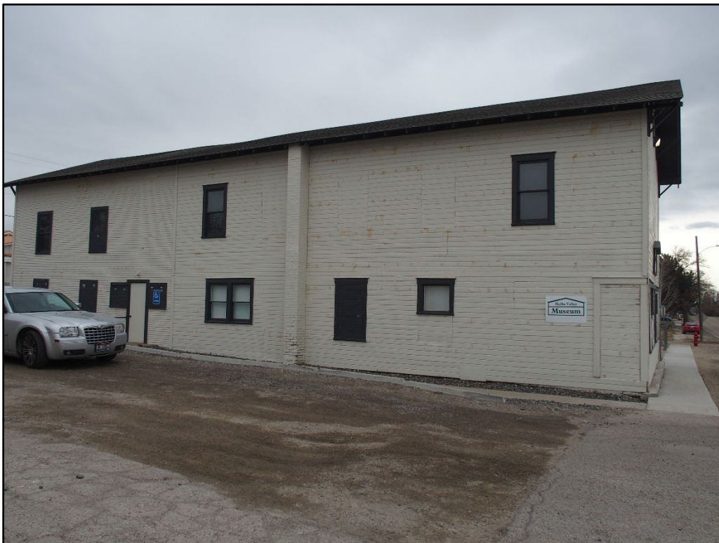
Photograph 4. North elevation, camera facing southeast.
