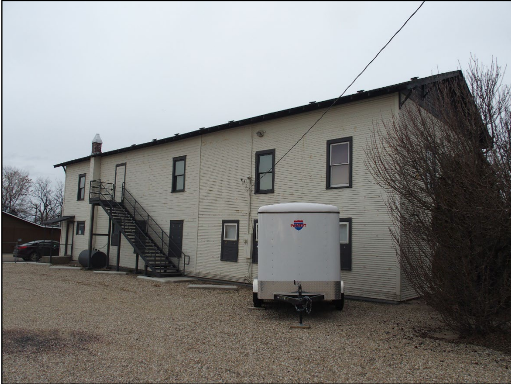
Photograph 7. South elevation, camera facing northwest.
