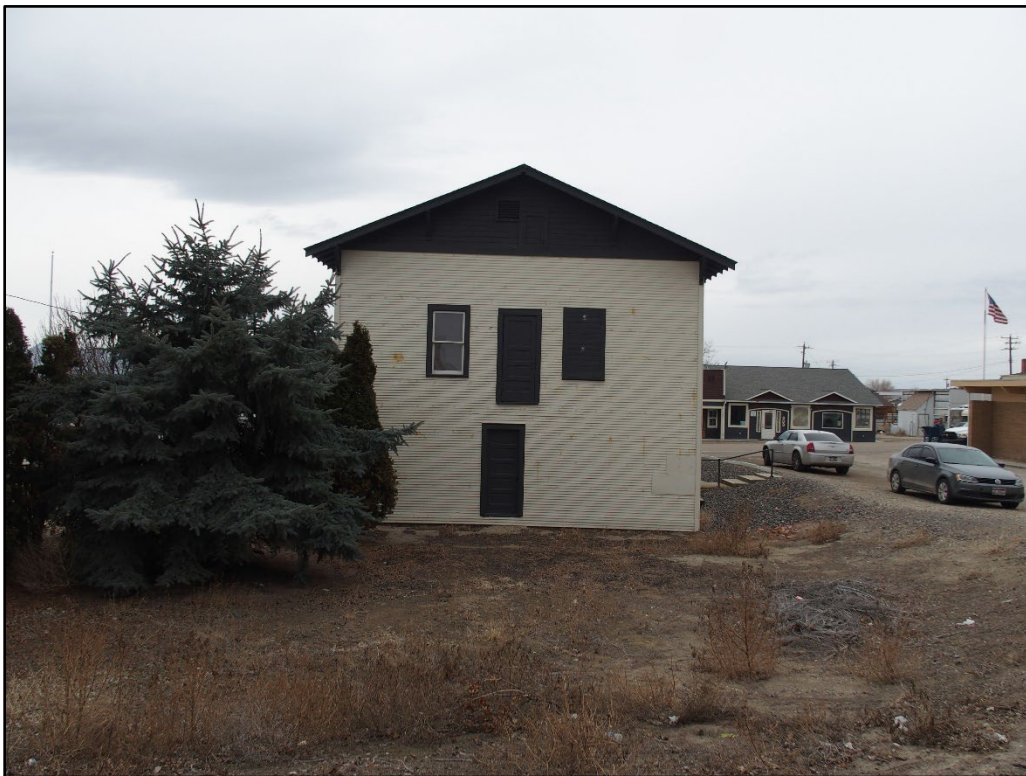
Photograph 6. East elevation, camera facing west.
