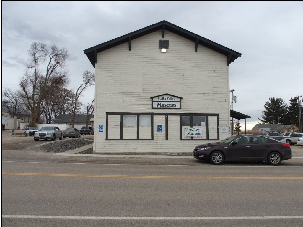
Photograph 1. Façade (west elevation), camera facing east.
