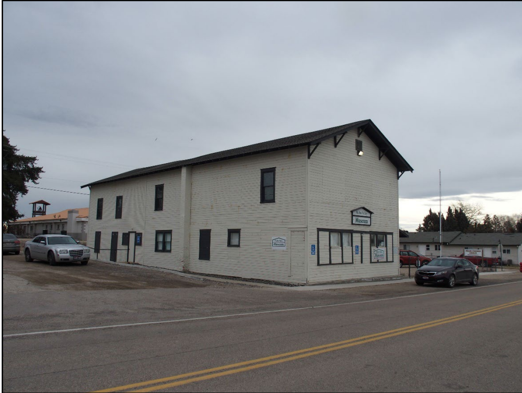
Photograph 3. North elevation (left) and façade (right), camera facing southeast.
