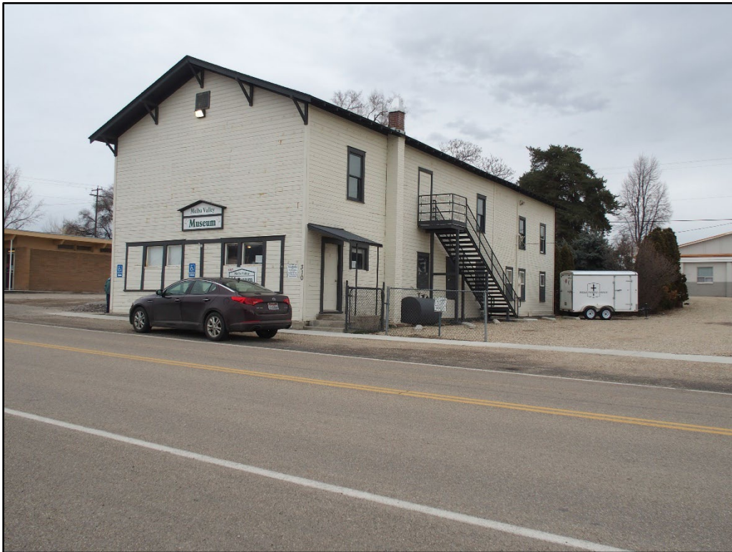
Photograph 2. Façade and south elevation, camera facing northeast.
