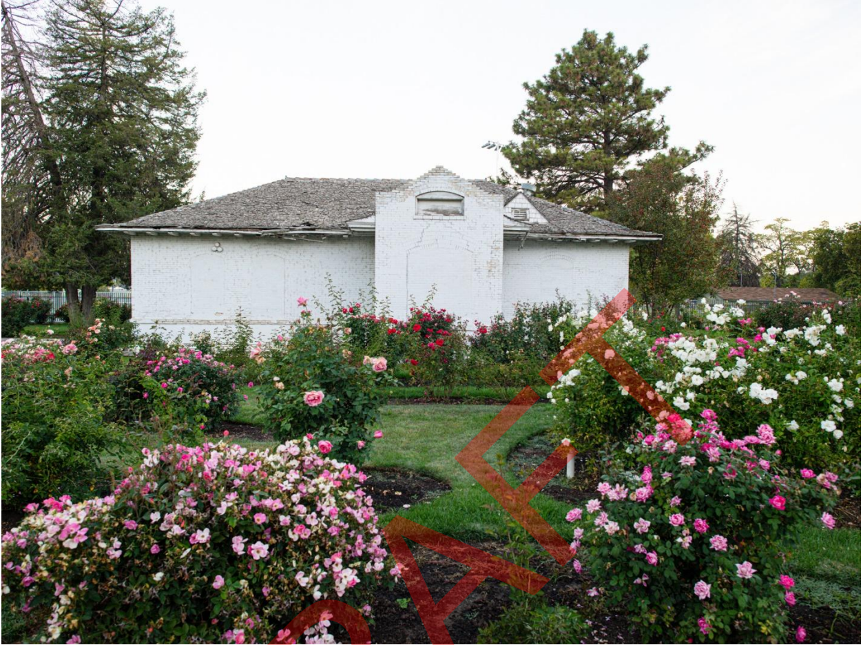
Photo 5 of 15. ID_ CanyonCounty _CaldwellRoseGarden_0005 View of pumphouse, camera facing west. Photo by Guy Hand, October 2024.
