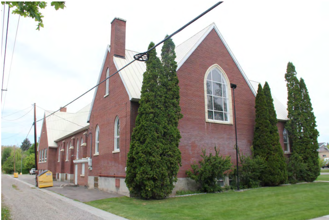
Photograph 4. Exterior, east and rear (south) facades. Camera facing northwest.
