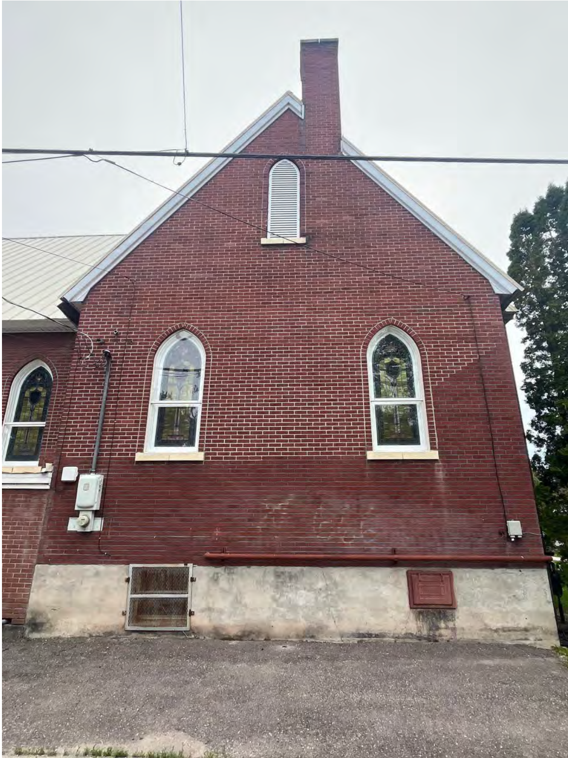
Photograph 7. Exterior south façade, east wing. Camera facing north.
