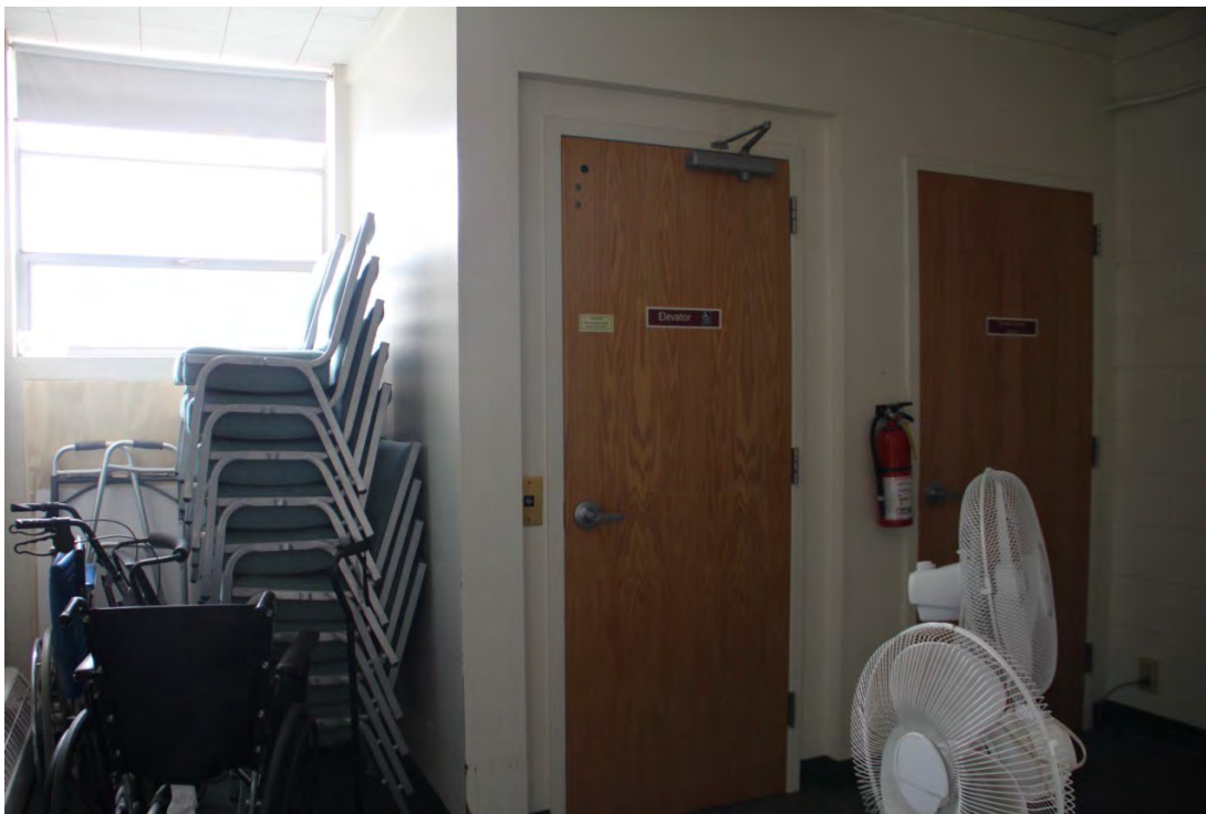
Photograph 26. Interior, basement, former classroom turned storage and elevator core. Camera facing west.
