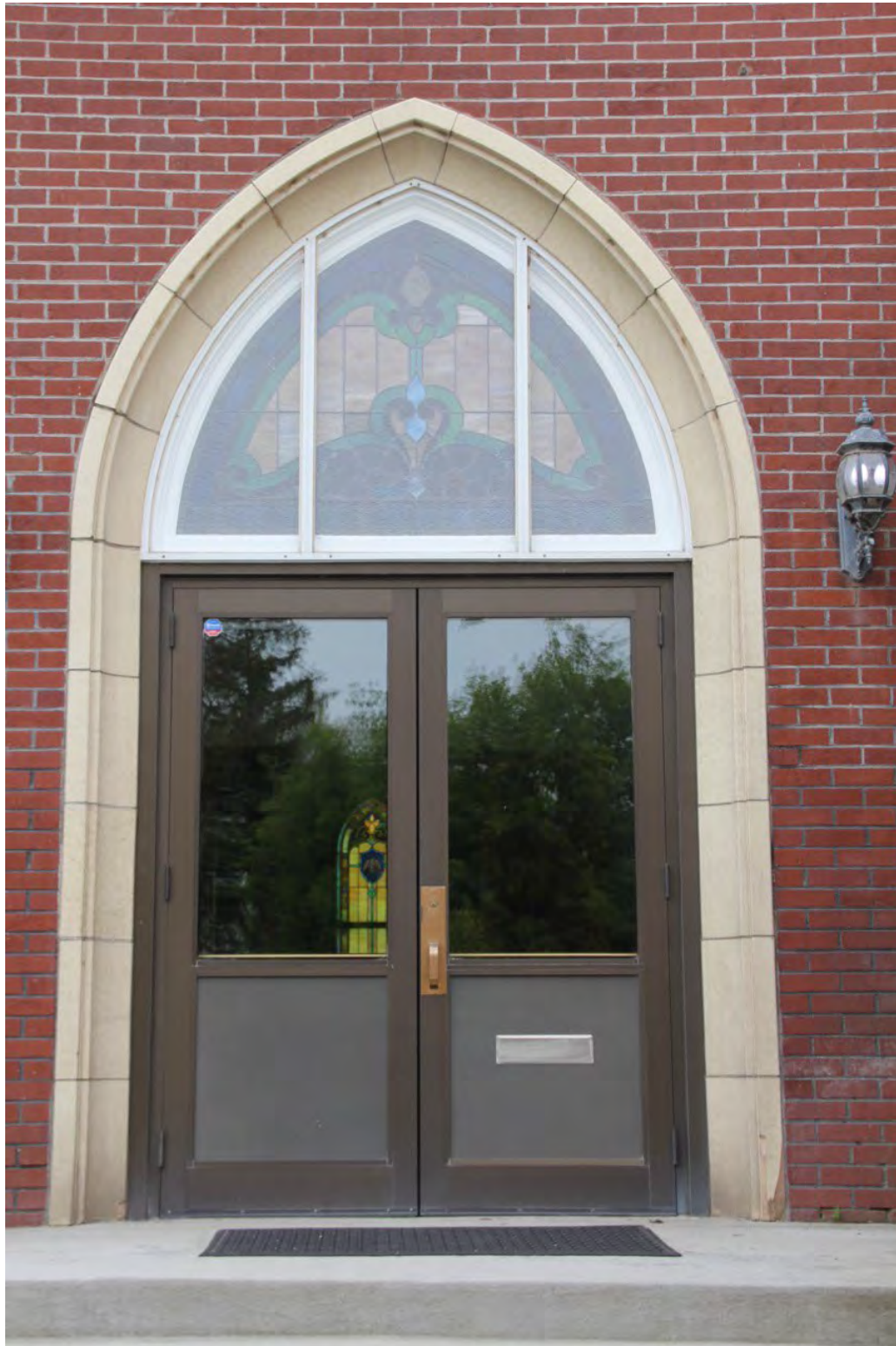
Photograph 14. Exterior, north (main) façade), detail of entryway with terra cotta surround. Camera facing south.
