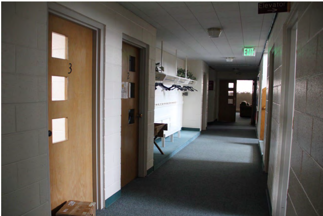
Photograph 24. Interior, basement, hallway in 1959 addition showing typical finishes. Camera facing south.
