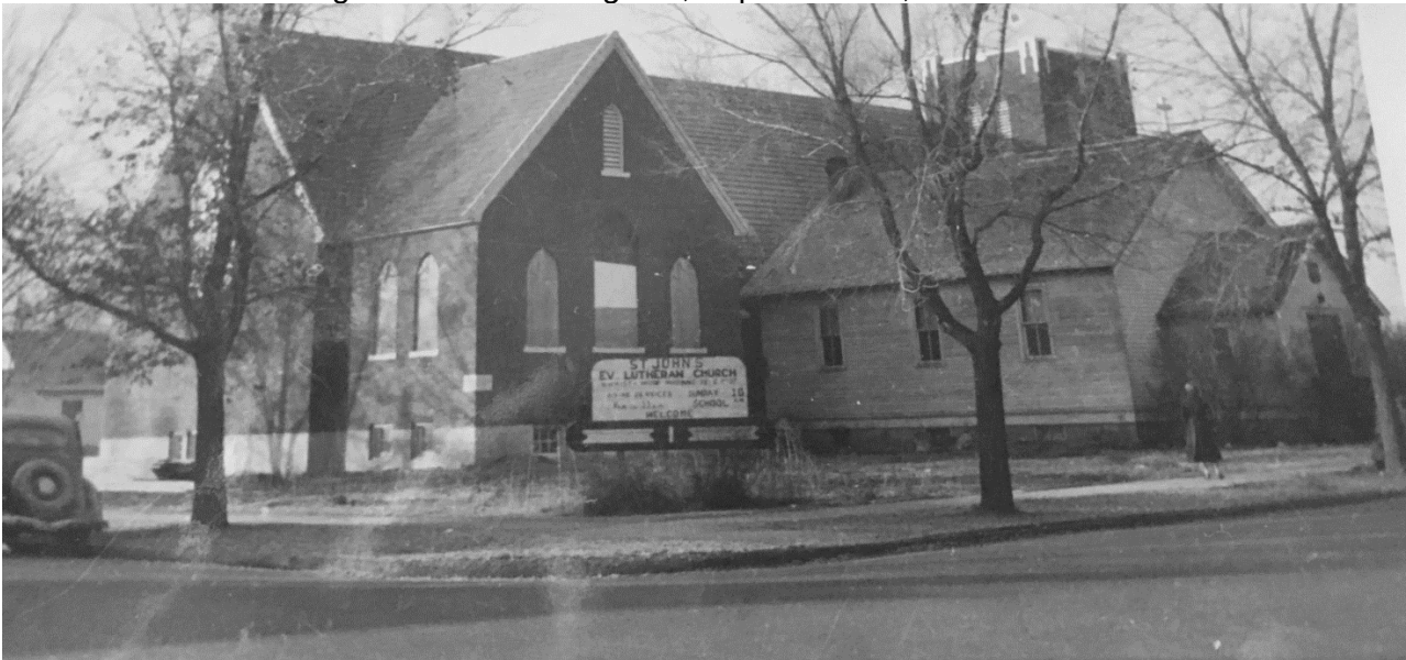
Figure 8. View of St. John during construction in September 1949 with the “old white church” in the elbow of the building. Source: Post Register , September 29, 1949.
