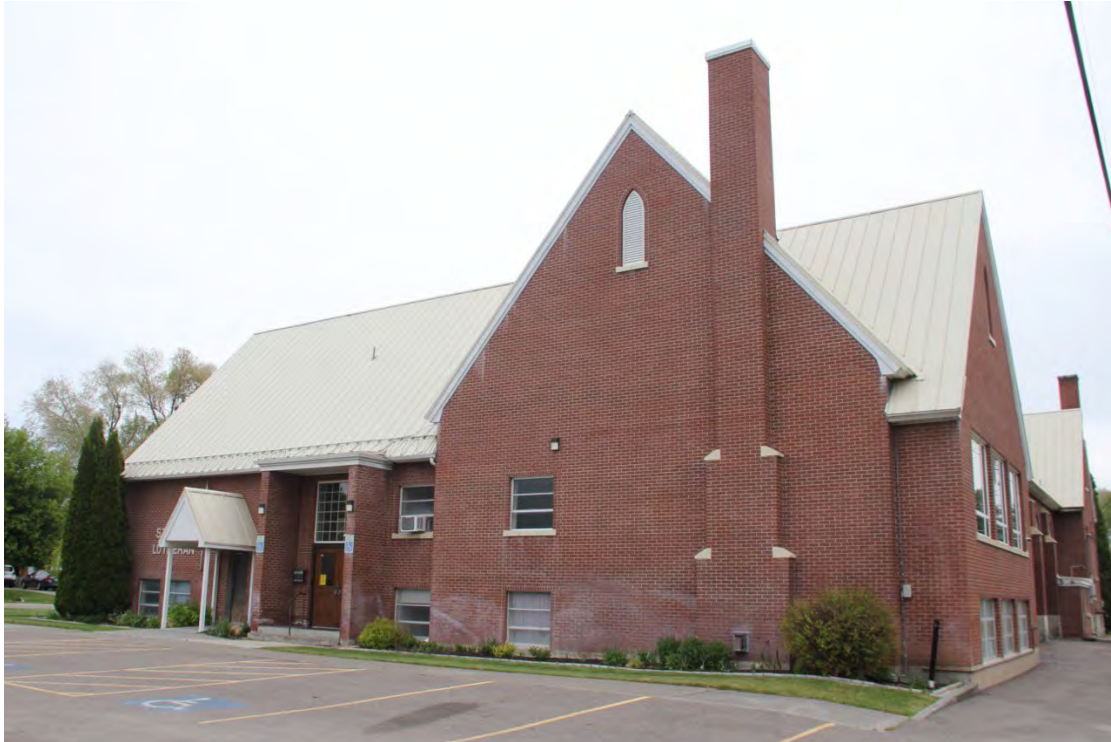
Photograph 9. Exterior, south (rear) and west facades of 1959 addition. Camera facing northeast.
