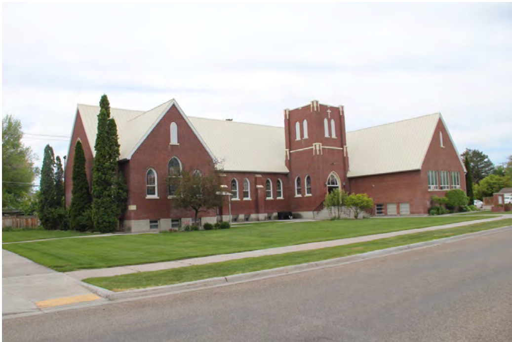
Photograph 2. Exterior, north (main) and east facades. Camera facing southwest.
