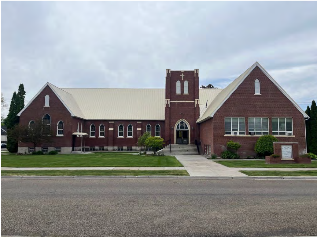
Photograph 1. Exterior, north (main) façade with bell tower entrance and 1959 addition to the right. Camera facing south.
