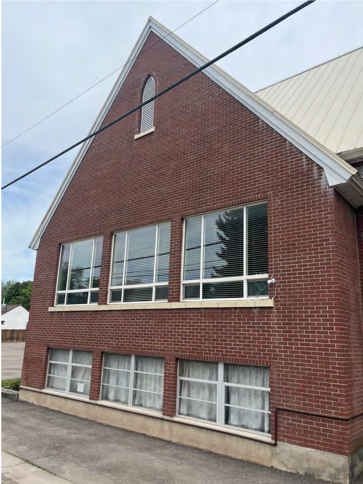
Photograph 8. Exterior, south façade, west wing / 1959 addition. Camera facing northwest.
