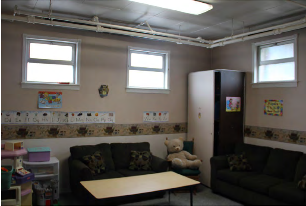
Photograph 21. Interior, basement, nursery showing original aluminum windows. Camera facing northeast.
