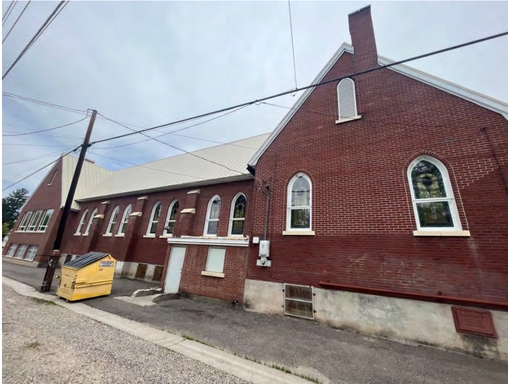
Photograph 5. Exterior, south façade with 1959 addition on left. Camera facing northwest.
