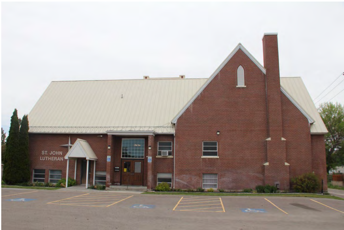
Photograph 10. Exterior, west façade of 1959 addition. Camera facing east.
