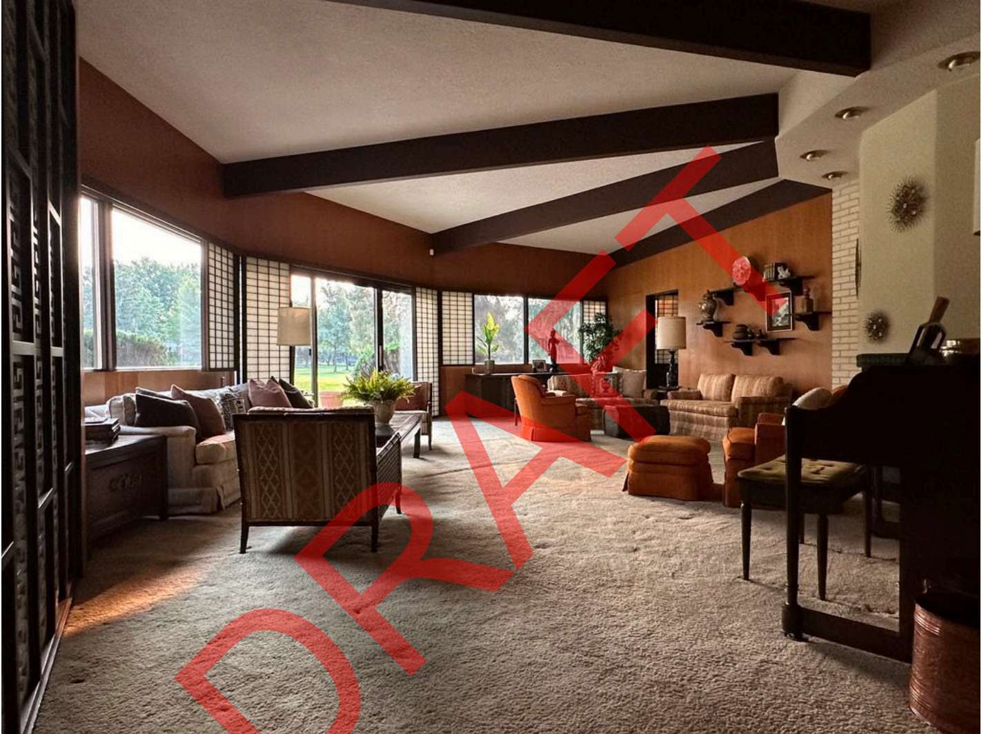
Photo 12 of 26. ID_AdaCounty_BrookoverGordonandBarbaraHouse_0012 View of the living room with the glu-lam ceiling beams radiating from the central fireplace toward the sliding doors to the patio. Note the shoji screens covering the windows.
