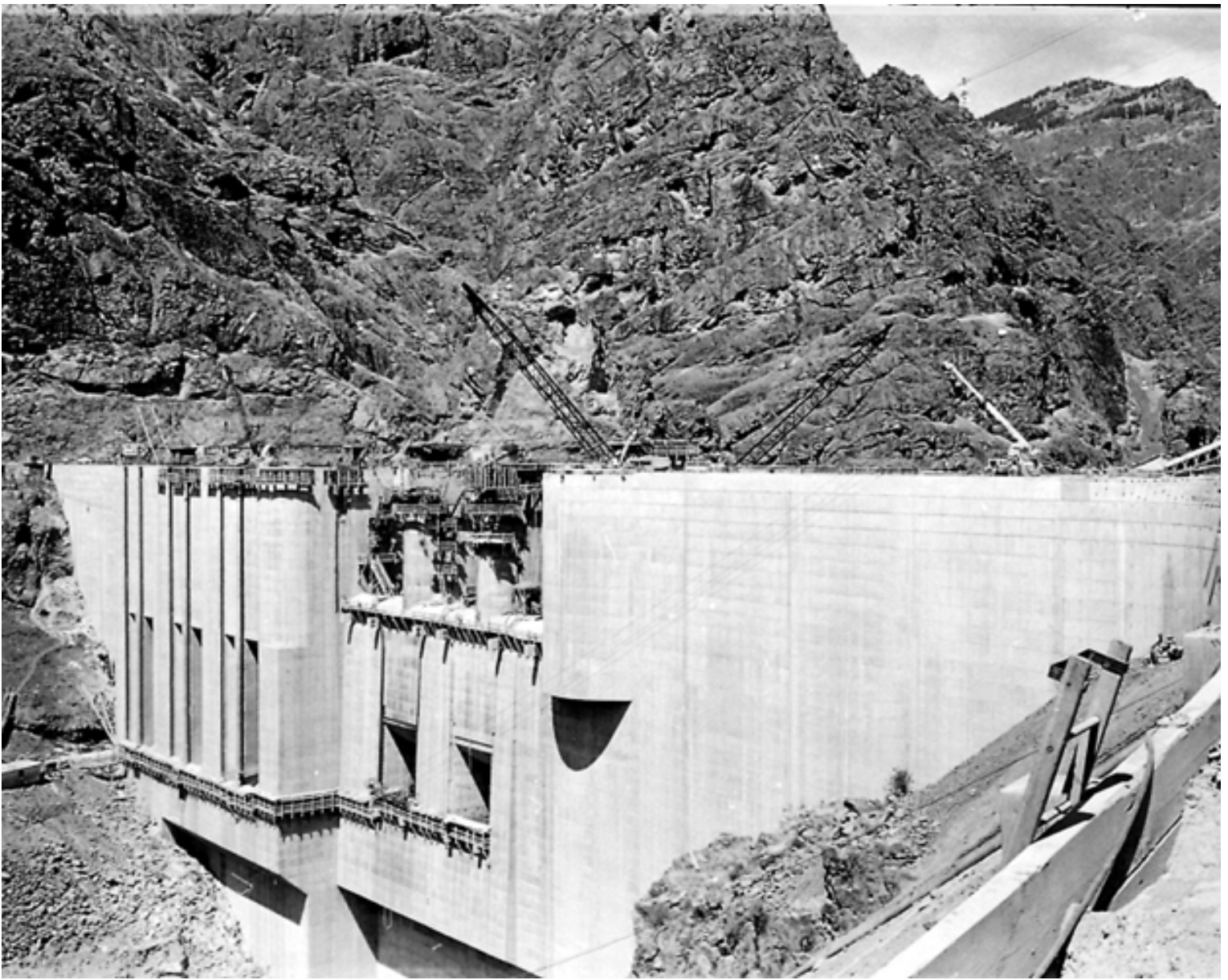
Figure 35 - The Hells Canyon Dam on the Snake River border between Oregon and Idaho was completed in 1967. It is one of Idaho's largest hydroelectric complexes, with an installed generation capacity of 391 MW and a 188,000 acre-ft. reservoir of impounded water behind it. P2006-18-755a. Bob Lorimer, "Hells Canyon Dam, 1967-08-09" Idaho State Archives.
