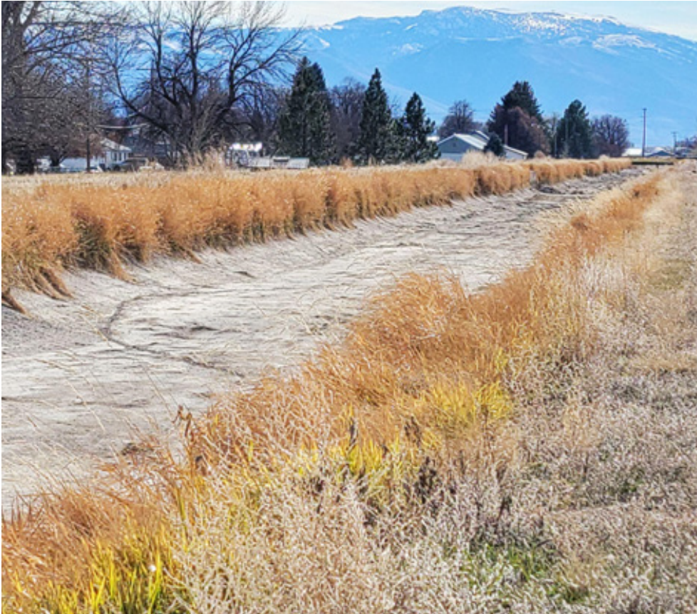
Figure 22 - “B Canal” of the Minidoka Gravity Division, Rupert, Idaho, with Mount Harrison in the background, November 2021. Laura Woodworth-Ney personal collection. This canal, along with all of the main and lateral canals on the Minidoka Project and other active irrigation projects, fill with water in April and drain by the end of the irrigation season.
