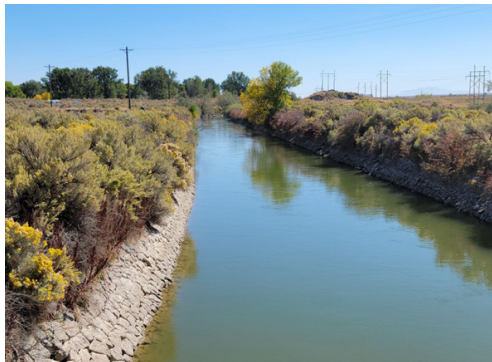
Figure 4 - Main Canal from Lake Walcott, part of the Minidoka Project's conveyance system, September 2021, Laura Woodworth-Ney, Photographer. Portions of the Main Canal are lined with lava rock dating from the Civilian Conservation Corps era of the 1930s.
