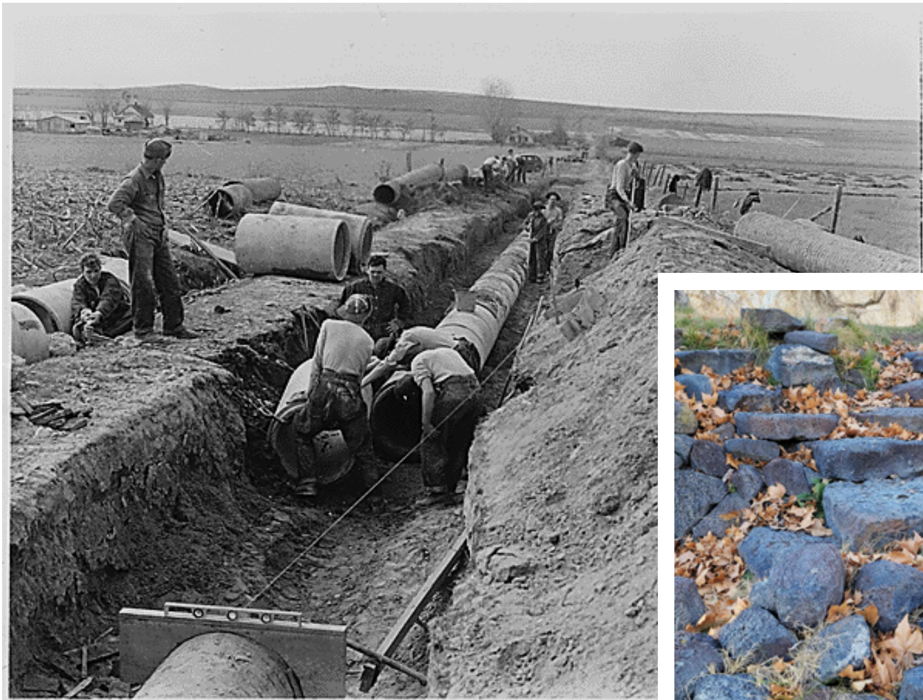
Figure 33 - "CCC Camp BR-24 Boise Project, Marsing, Idaho: Photo of crew placing 24" concrete pipe," 14 March 1941. Department of the Interior, Bureau of Reclamation, Civilian Conservation Corps Division, 1937-1942, Record Group 115, National Archives and Records Administration at Denver. ARC #293519.
