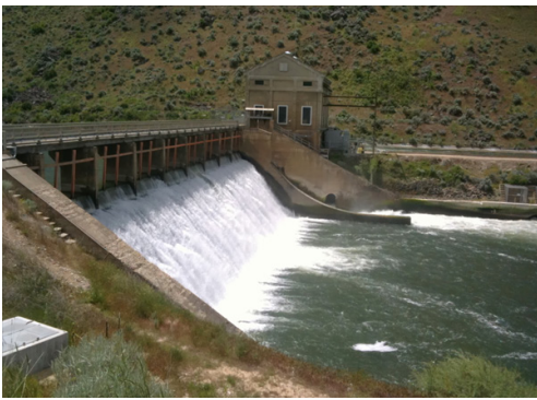
Figure 3 - Boise Diversion Dam, Boise Project, Boise, July 2017, Laura Woodworth-Ney, Photographer. Shows the dam and part of the main intake system diverting water into the New York Canal (in the background), which is part of the system's conveyance system.
