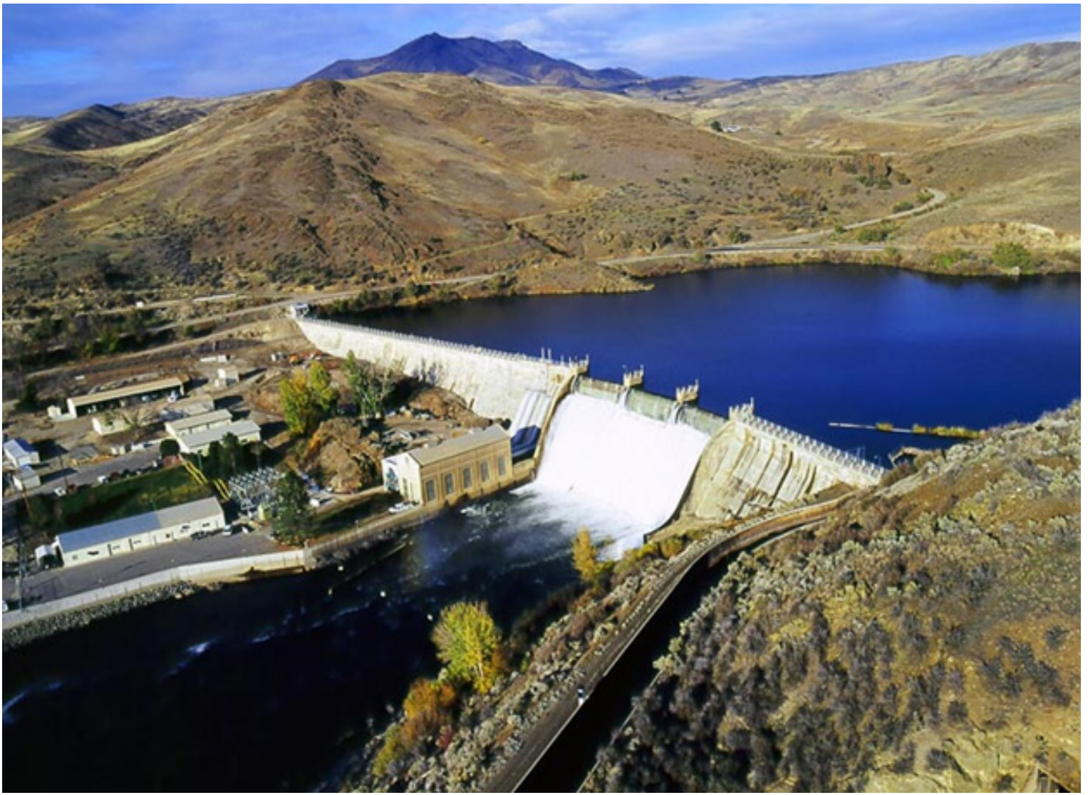
Figure 31 - Black Canyon Diversion Dam, on the Payette River, is a concrete gravity dam that diverts water to the Payette Division, Boise Project, through Black Canyon Canal (shown in the foreground). Bureau of Reclamation, August 3, 2016.
