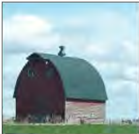
Figure 15. Barn with Gothic arch roof.
