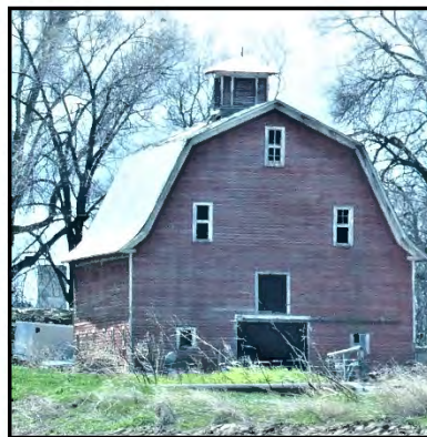
Figure 11 (left). English gambrel roof.
