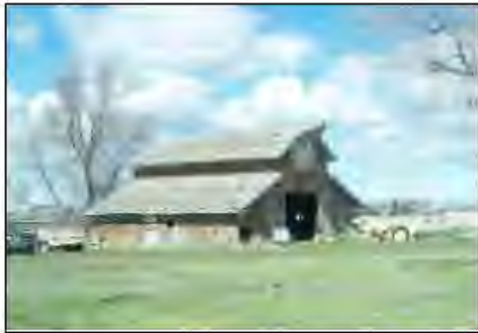
Figure 13. Barn with monitor roof.
