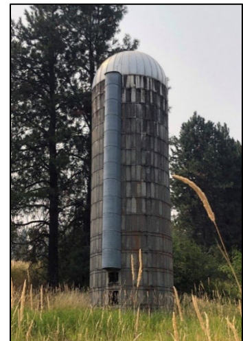
Figure 32. A concrete silo at 5690 East Heine Road.
