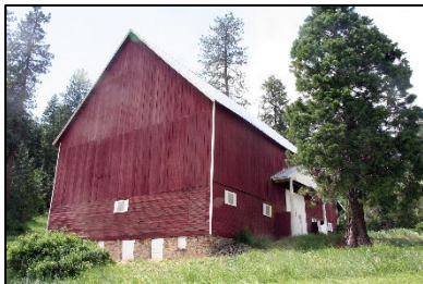
Figure 21. Simple Gable barn at 4174 West Cougar Gulch Road.
