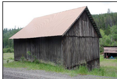
Figure 22. A Gable barn set into the hillside at 12777 West Cougar Gulch Road.
