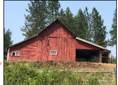
Figure 23. A Broken Gable barn at 4570 South Stach Road.
