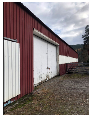
Figure 31. Example of a steel arena at 4175 West Cougar Gulch Road.
