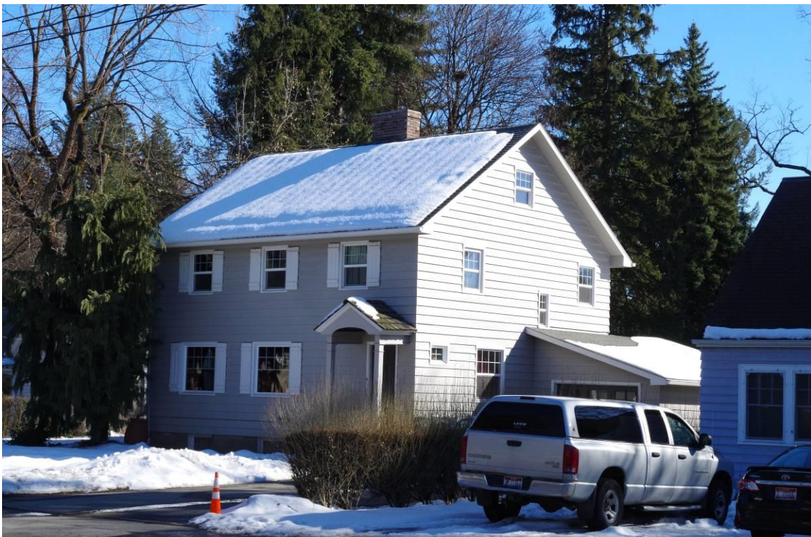
FIGURE 21: Hansen House, 815 East 6 th St., Moscow, Idaho Built by Harry Campbell in 1936
