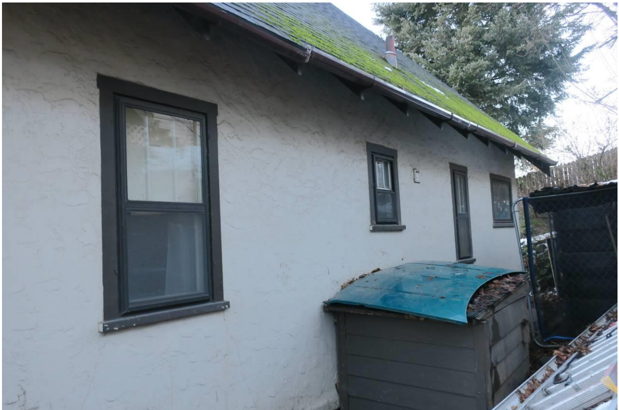
Photo 4: View West of northeast elevation
