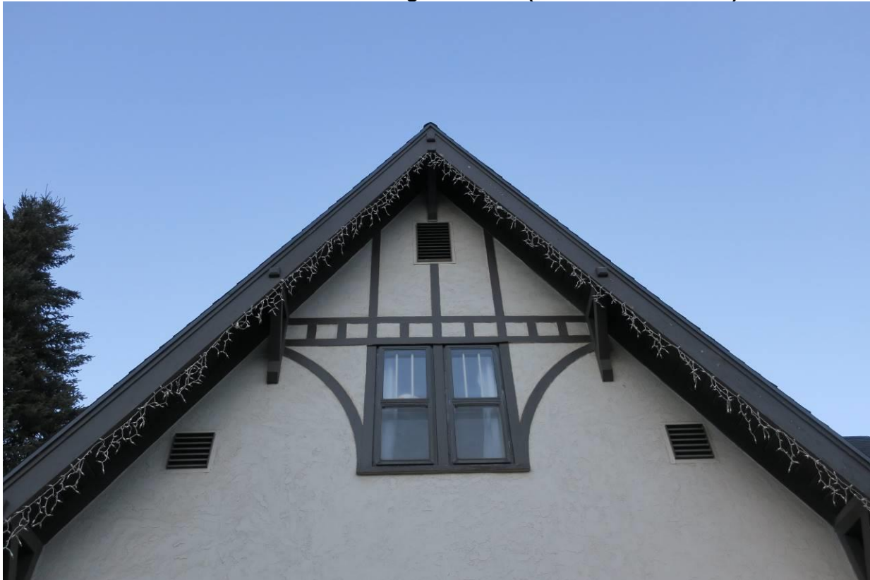
Photo 7: View Northeast of gable detail (southwest elevation)
