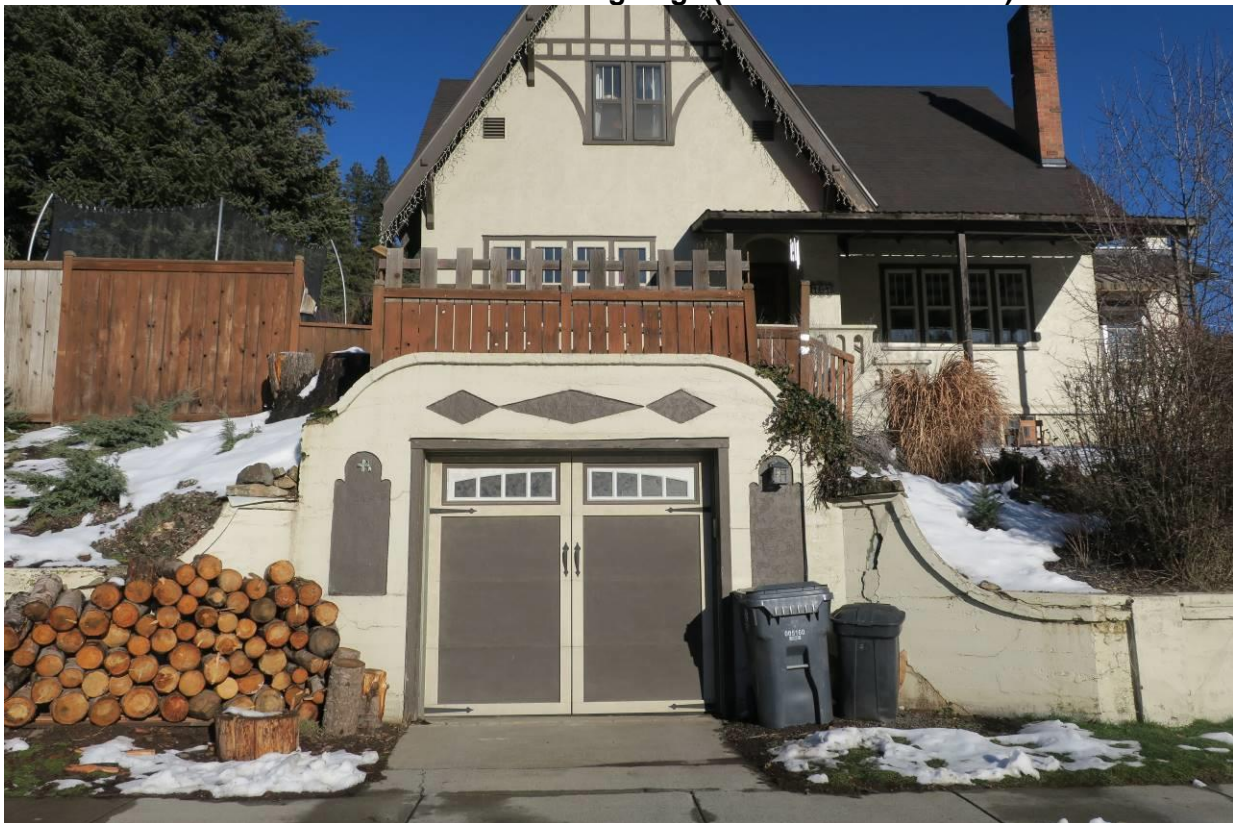
Photo 6: View Northeast of garage (southwest elevation)
