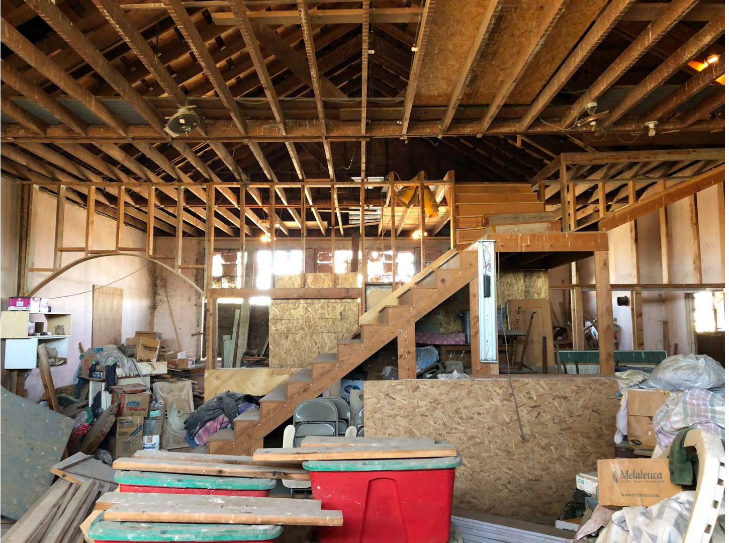
Photo 11. ID_JeromeCounty_GreenwoodSchool_0011 Interior, classroom space, looking east
