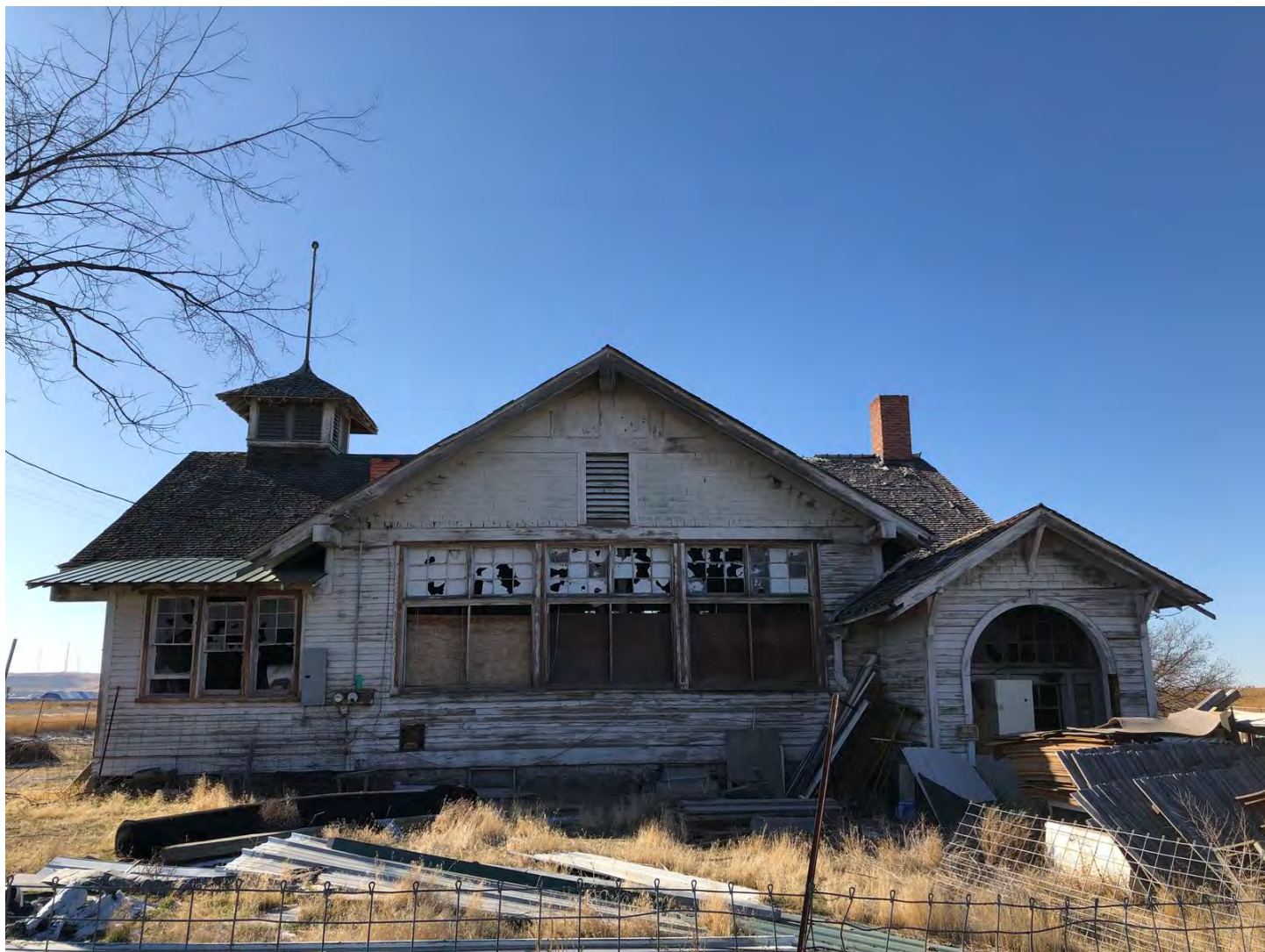
Photo 6. ID_JeromeCounty_GreenwoodSchool_0006 East elevation, looking west
