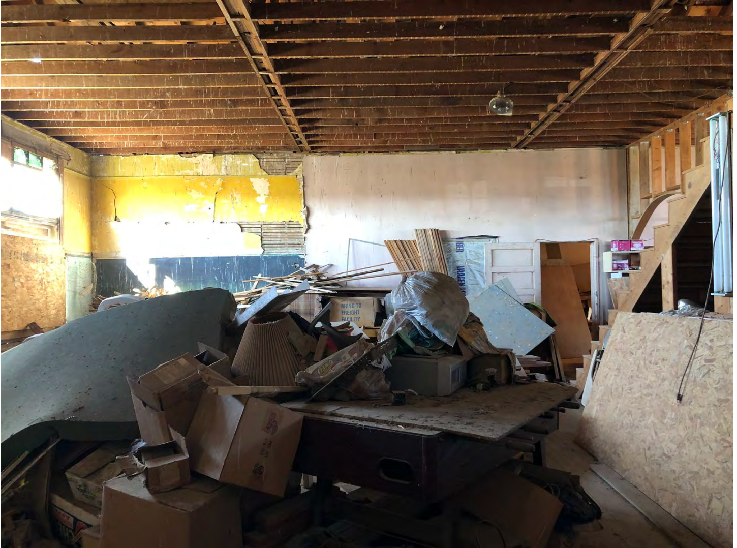
Photo 10. ID_JeromeCounty_GreenwoodSchool_0010 Interior, classroom space, looking north
