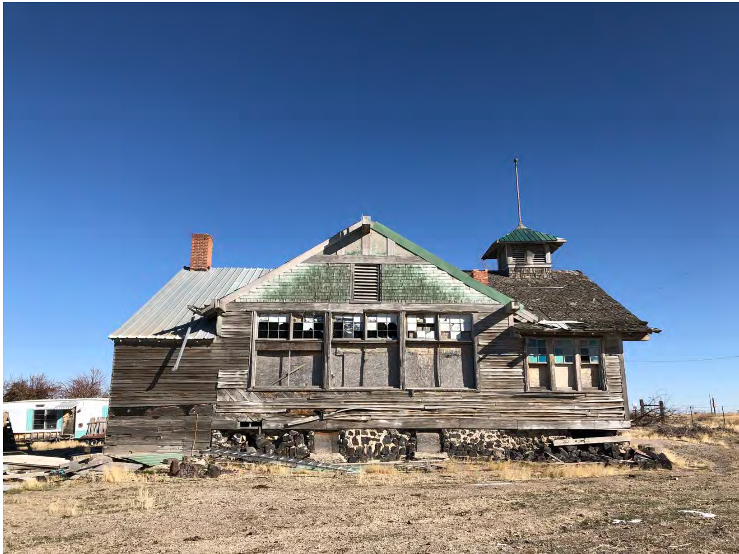
Photo 4. ID_JeromeCounty_GreenwoodSchool_0004 West elevation, looking east
