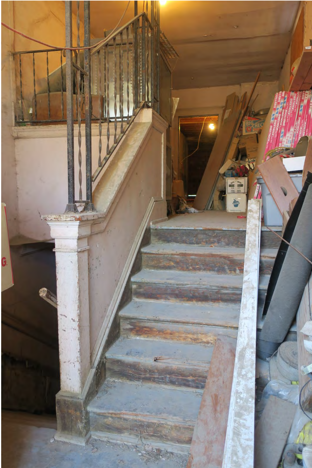
Photo 14. ID_JeromeCounty_GreenwoodSchool_0014 Interior, staircase at northeast entry, looking west
