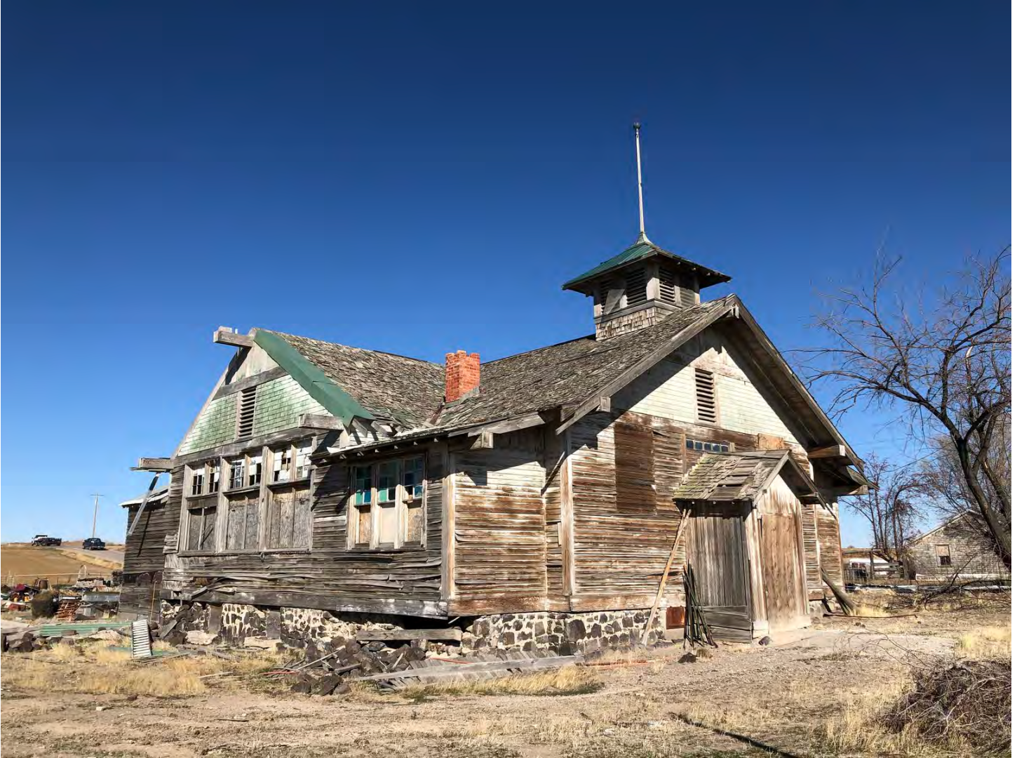
Photo 3. ID_JeromeCounty_GreenwoodSchool_0003 Primary (south) and west elevations, looking northeast
