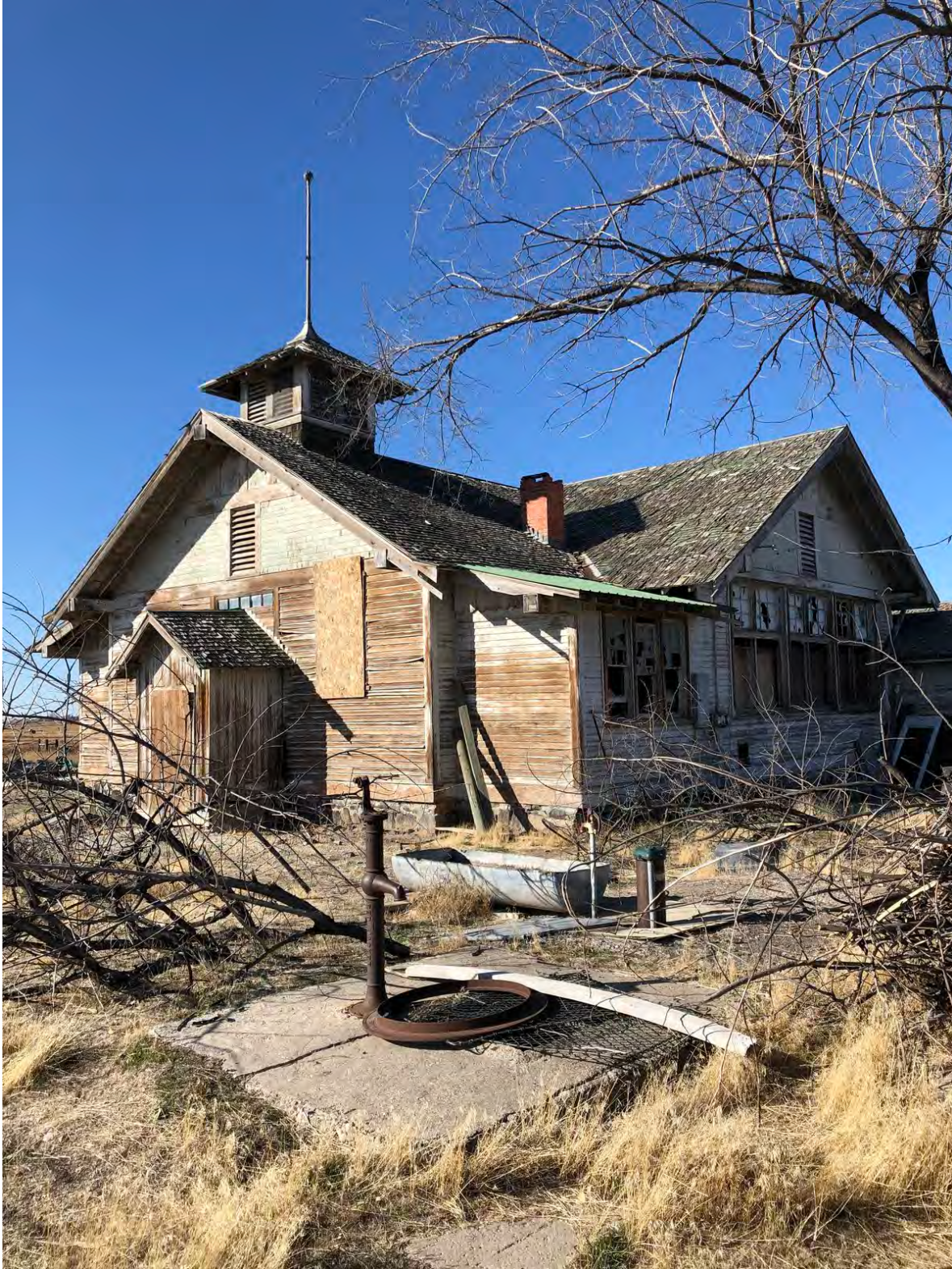
Photo 7. ID_JeromeCounty_GreenwoodSchool_0007 Primary (south) and east elevations, looking northwest
