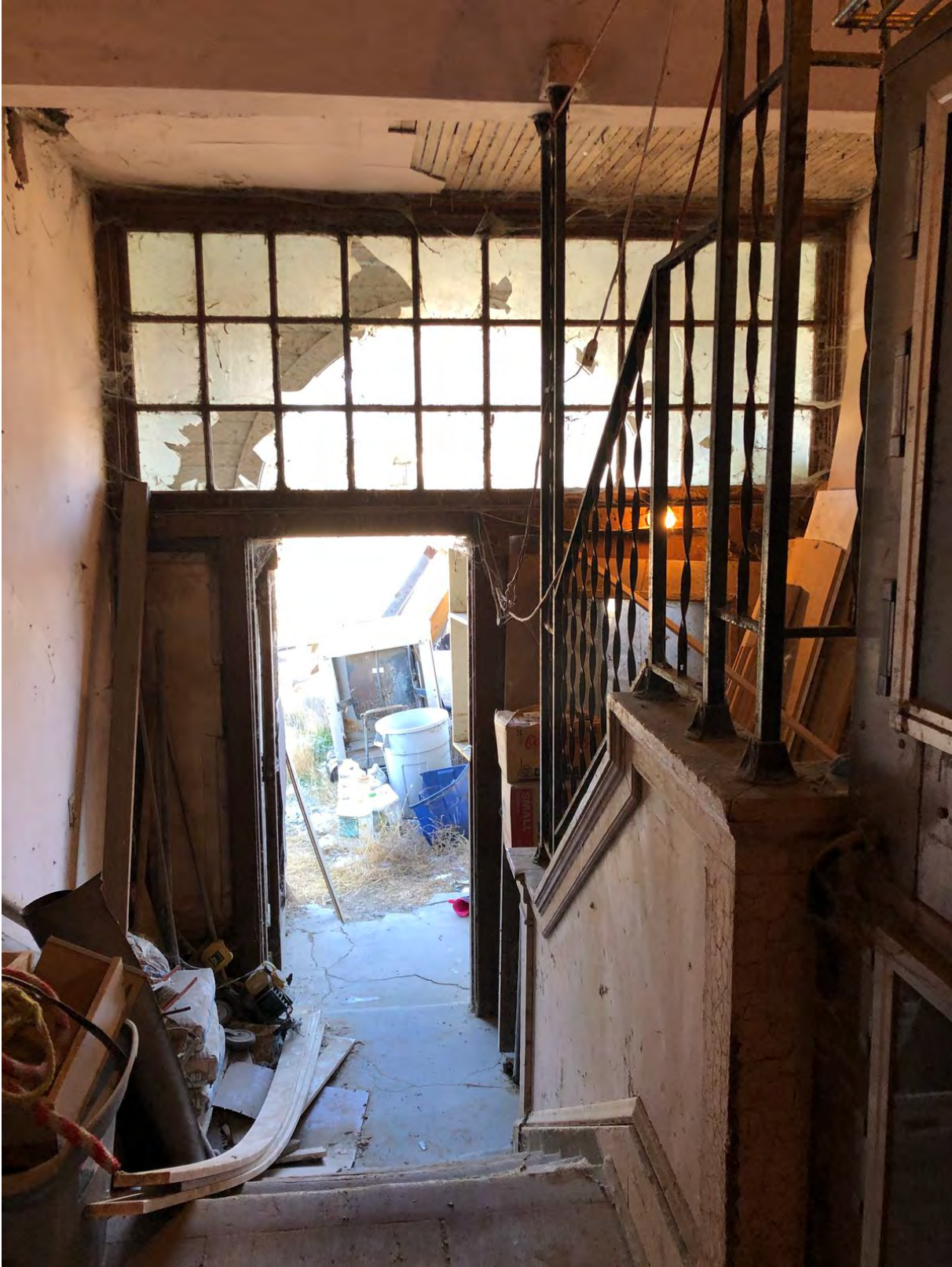
Photo 13. ID_JeromeCounty_GreenwoodSchool_0013 Interior, east entry and staircase, looking east
