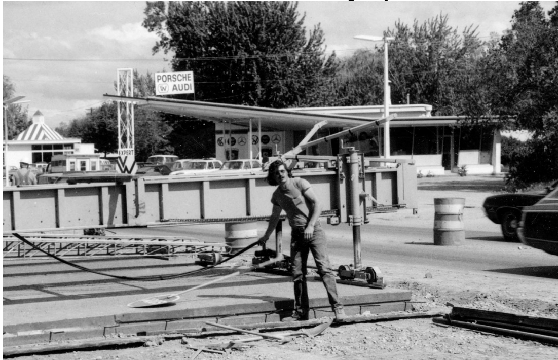
c.1978 State Street Widening Project
