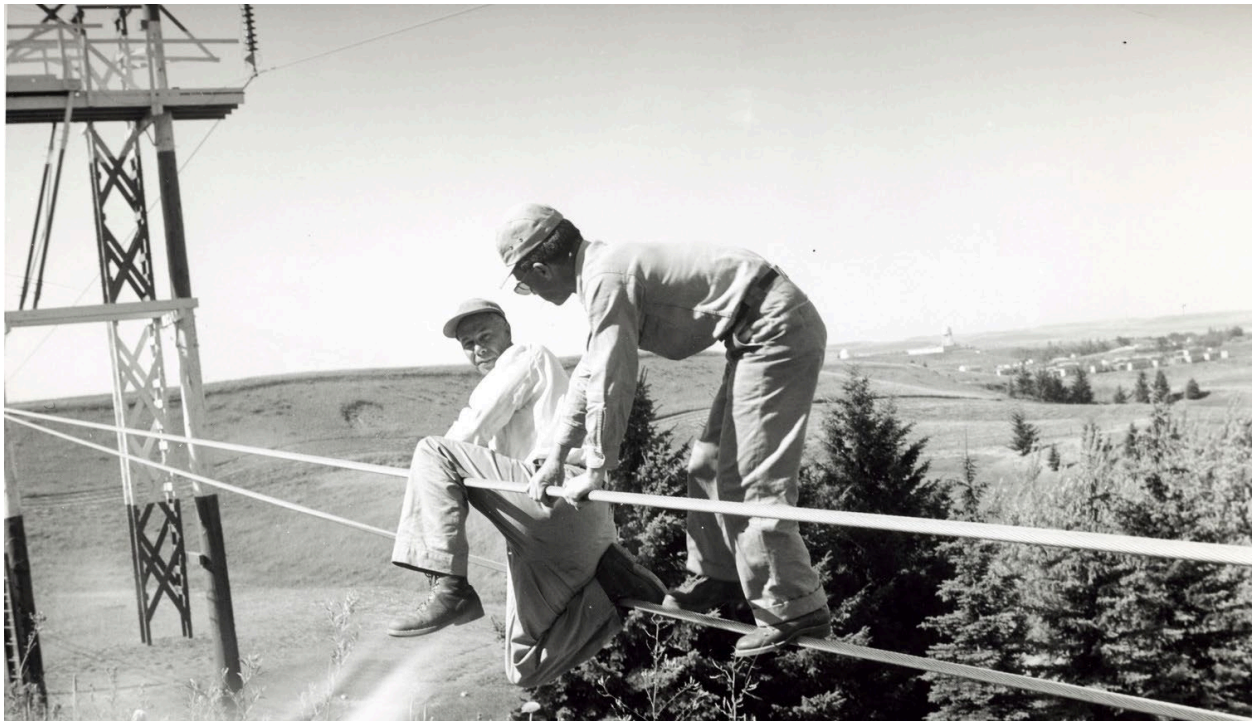
Figure 59. Matt Marjerrison (right) and Merle Poland perform ice unloading tests, July, 1956. 331
