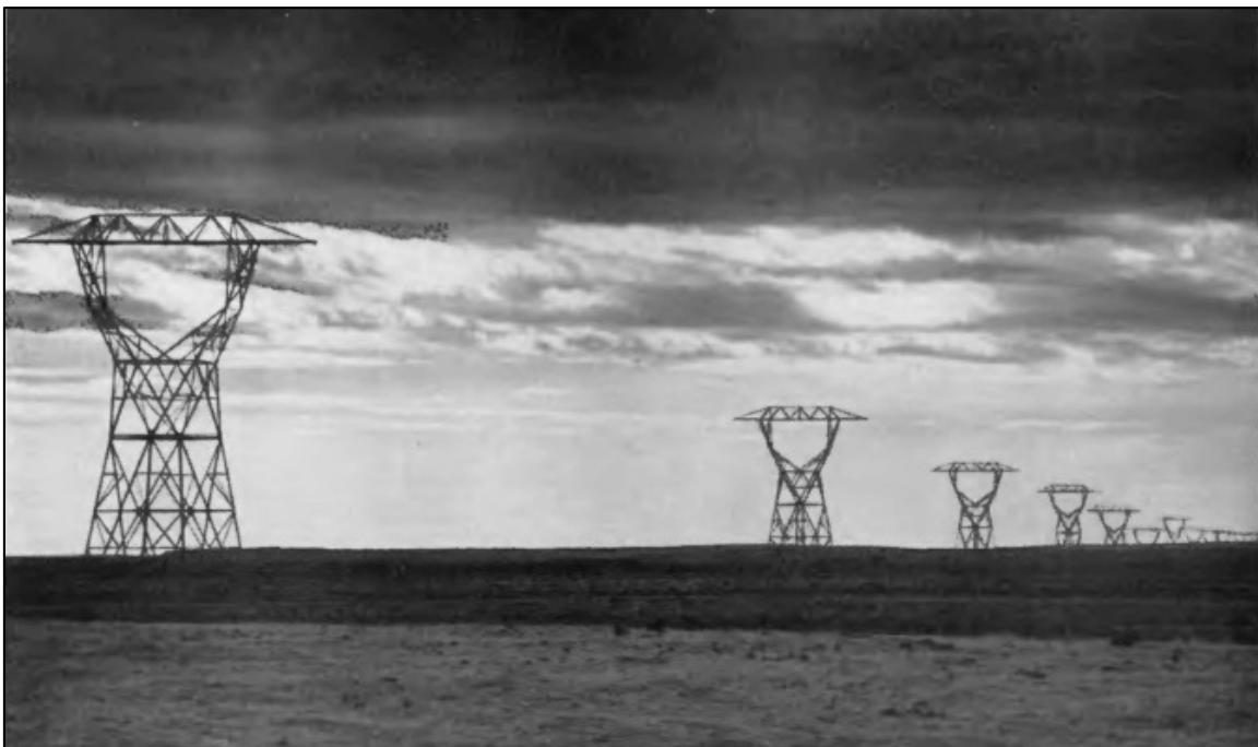
Figure 14. Completed lattice steel towers on the Bonneville-Grand Coulee line near Coulee City, Washington ca. 1939. 116
