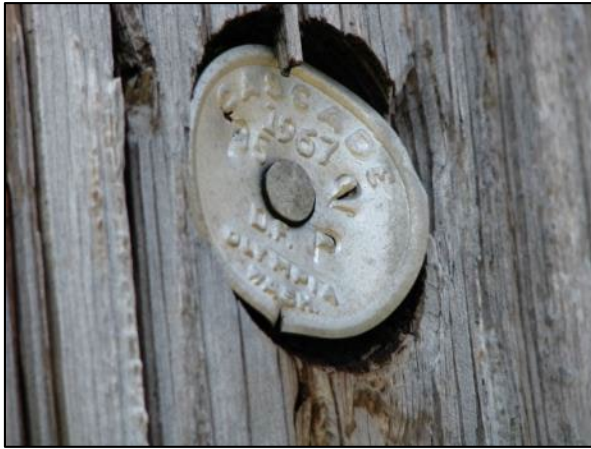
Figure 73. Aluminum Wood Pole Tags indicate supplier information, dates, wood species, preservatives, and other information.
