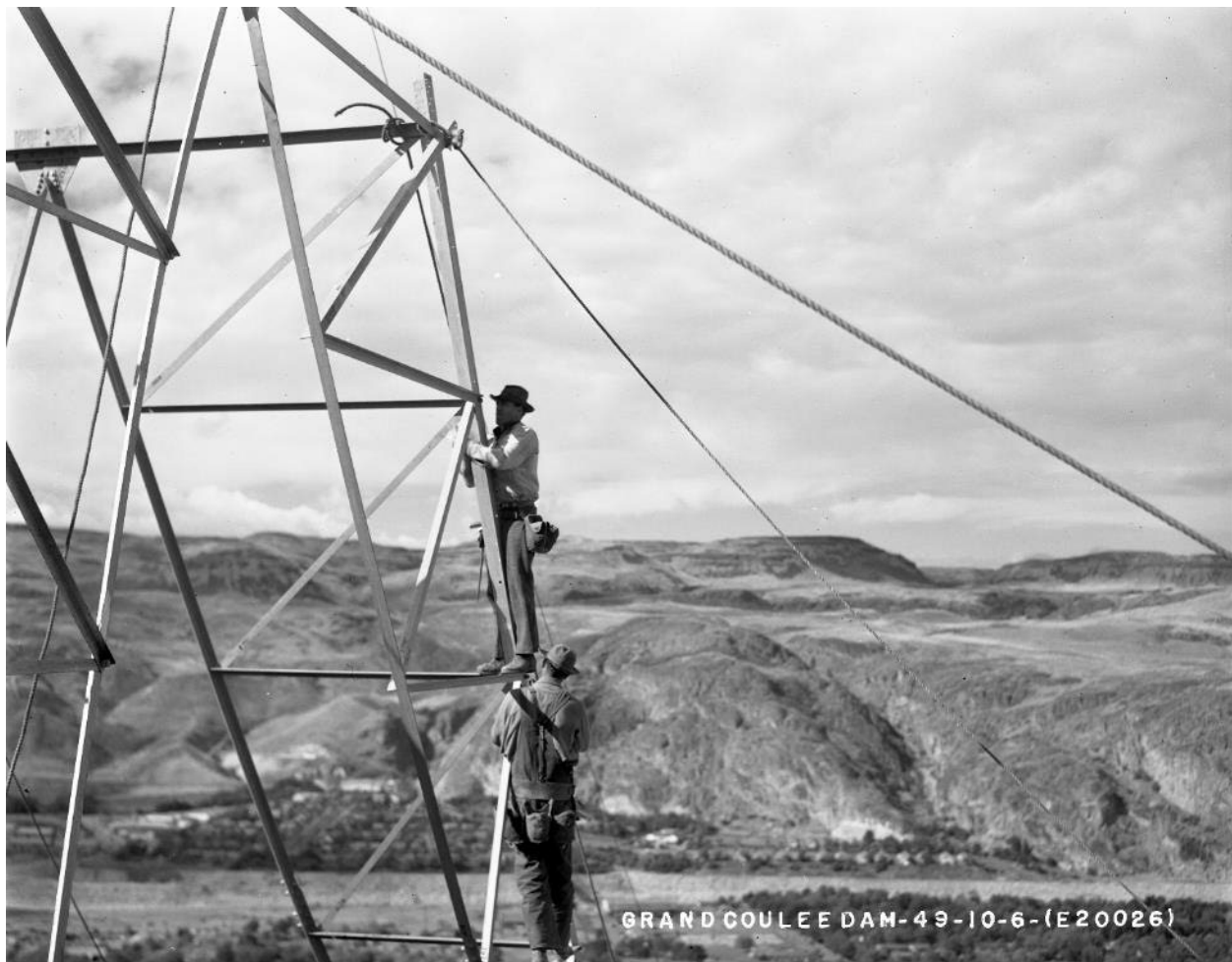
Figure 7. Workers Installing Transmission Structure at Grand Coulee Dam, 1949. 47
