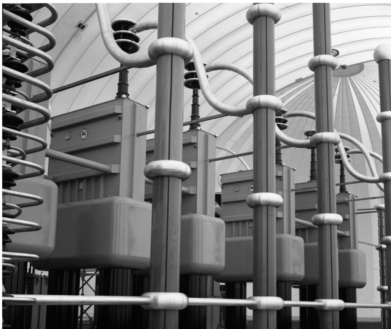
Figure 47. Ultra-high voltage testing equipment at Big Eddy HVDC Test Site, 1963. 295
