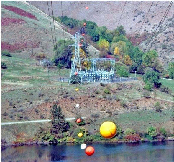
Figure 65. Marker balls near Oxbow Dam, Idaho (left); BPA installs an “Aviation Orange” colored Marker Ball (right), BPA.
