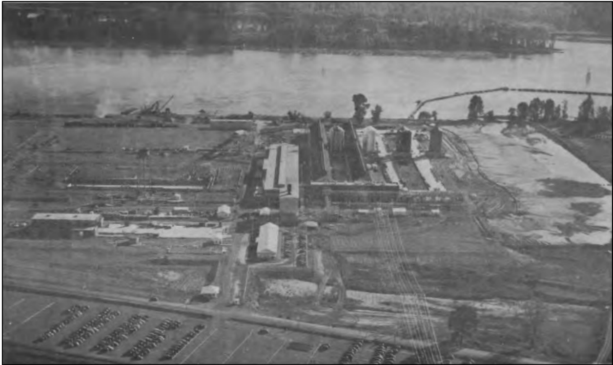
Figure 20. Transmission lines connecting with the Aluminum Company of America (ALCOA) in Vancouver, Washington, ca. 1940. 142
