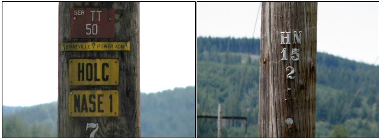
Figure 71. Transmission Structure Signage on Holcomb-Naselle Transmission Line.
