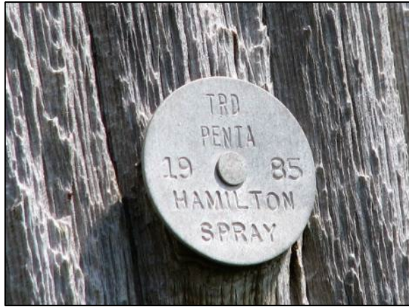
Figure 73. Aluminum Wood Pole Tags indicate supplier information, dates, wood species, preservatives, and other information.
