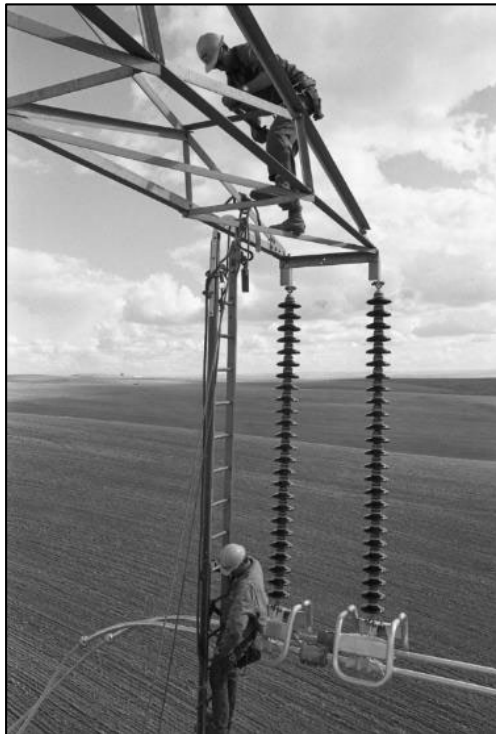
Figure 63. Linemen working on insulators, 1968. 346
