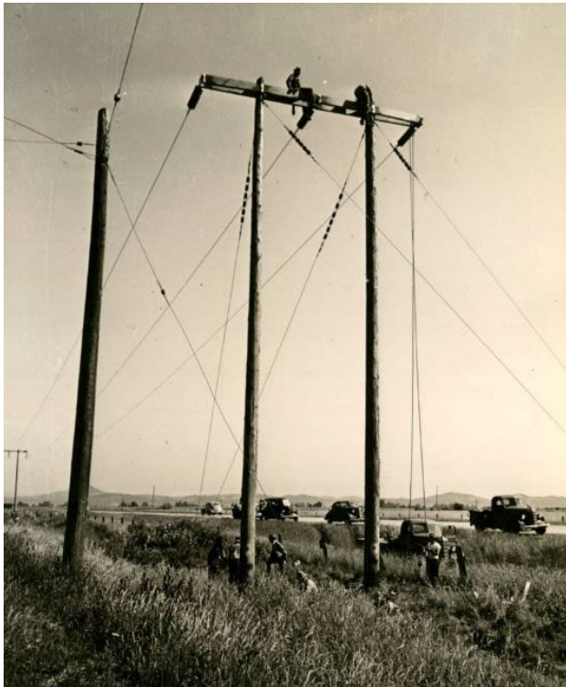
Figure 79. Two-pole H frame structure (left) and 1939 BPA drawing (right). 378
