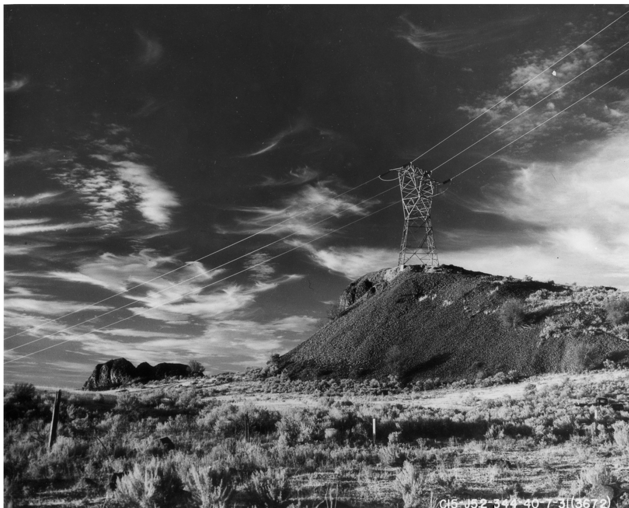
Figure 21. Construction of the 230-kV Grand Coulee-Spokane Line, July 31, 1940. 153
