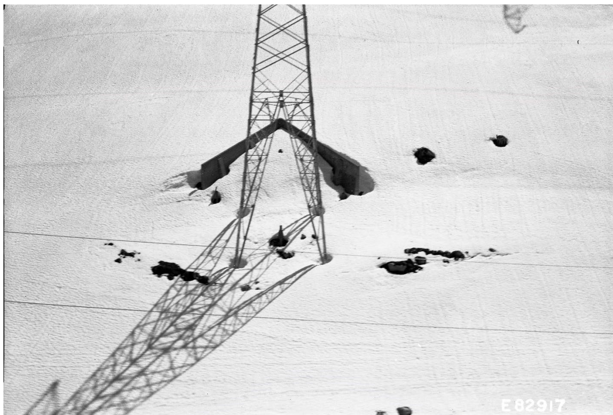
Figure 29. Chief Joseph-Monroe #1 Line, showing Tower 77-1 and its snow deflector, 1971. 205
