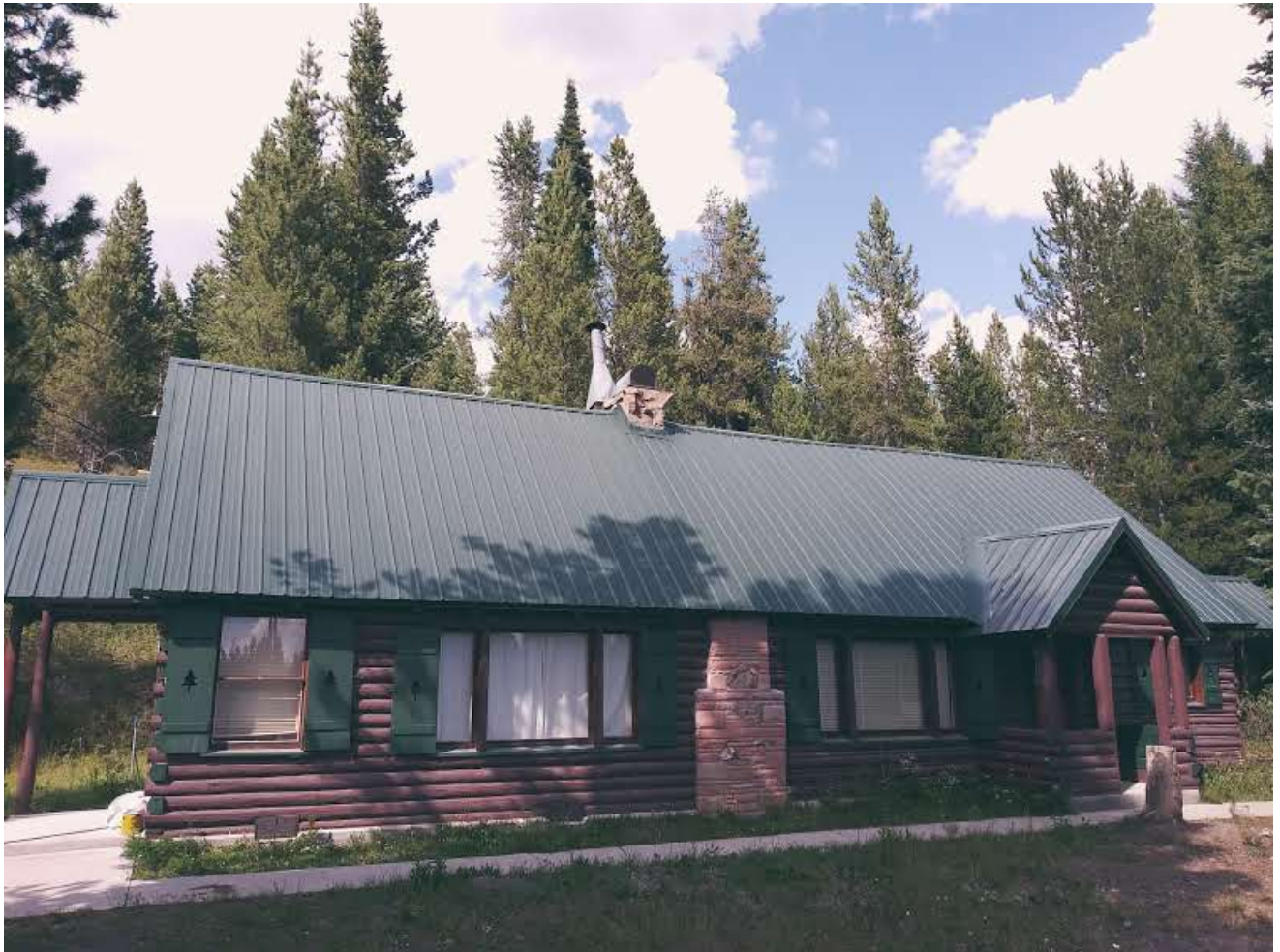
Photo 2: Cabin's south / front elevation looking north.
