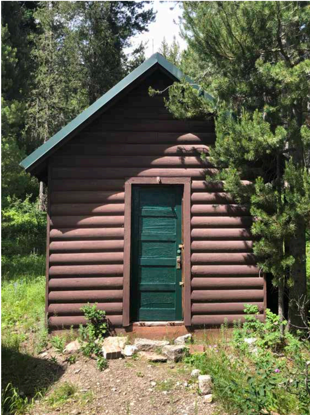
Photo 8: Cabin's storage shed looking north.
