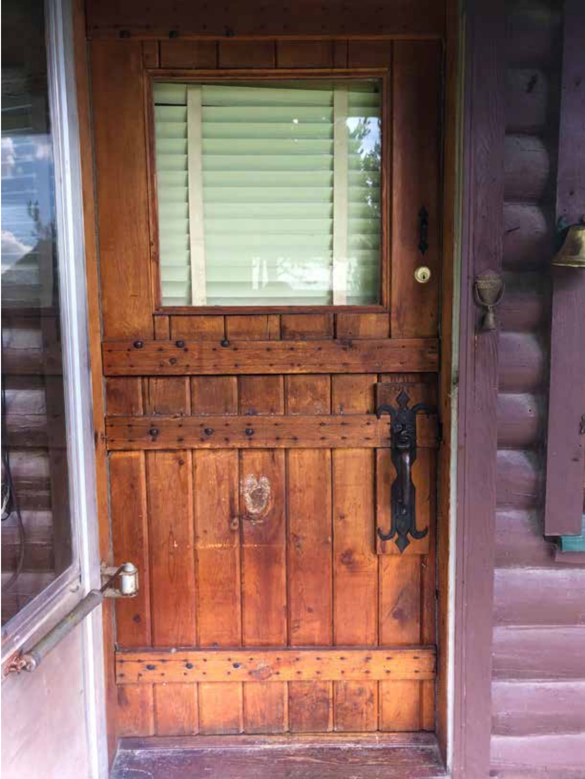
Photo 7: Detail of (kitchen) door on cabin's west / side elevation.
