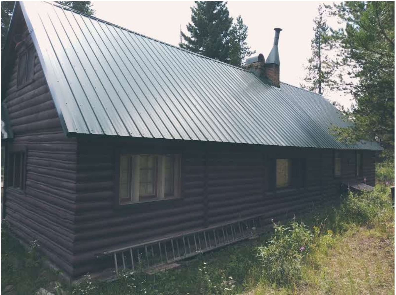
Photo 6: Cabin's east / side and north / back elevations looking southwest.
