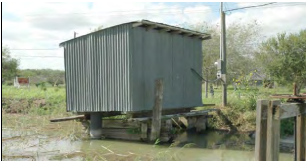
Figure 4.20 Pumping shed, Cameron County Irrigation District, #6, Lower Rio Grande Project (Texas). 219
