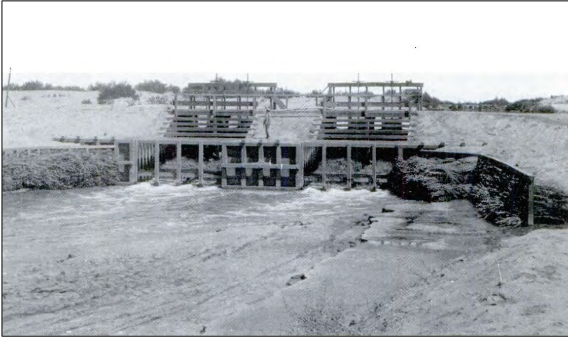
Figure 4.58 Wooden headgate and intake at Sharp's Heading, Imperial Irrigation District, Boulder Canyon Project. 252
