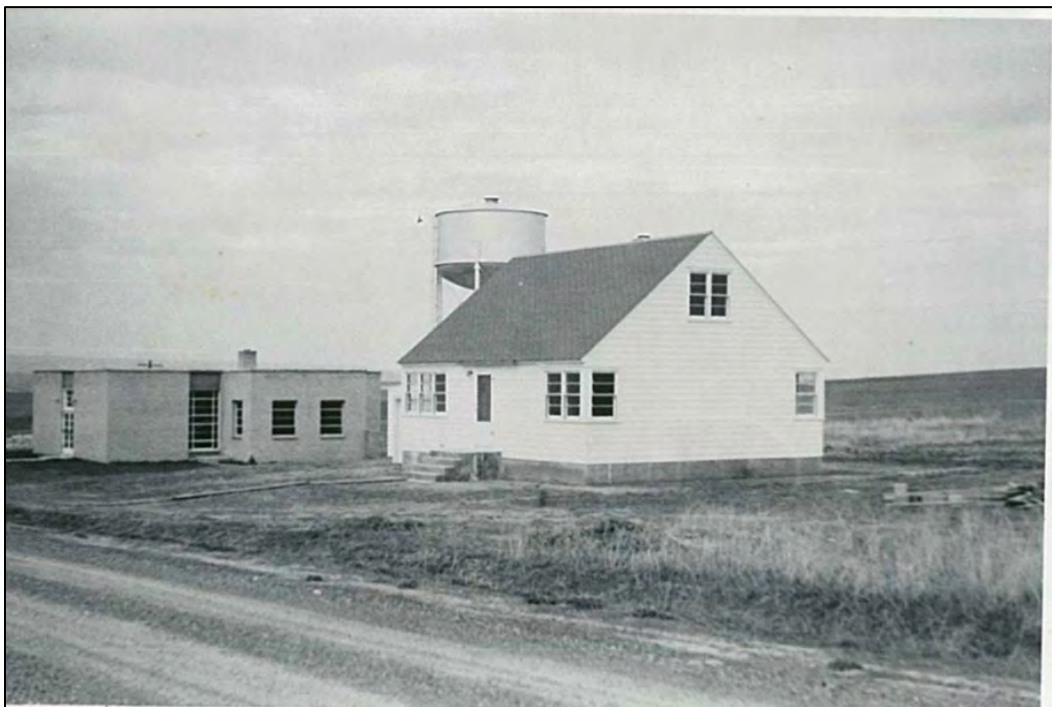
Figure 4.121 Water plant operator's residence at the Lewiston Orchards Project (Idaho). 321
