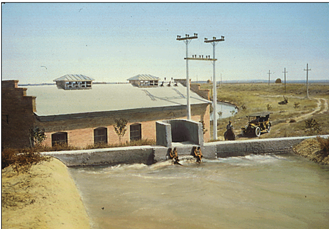
Figure 5.3 Minidoka Pump Plant (Idaho), c1904 (NARA Photograph #294675).
