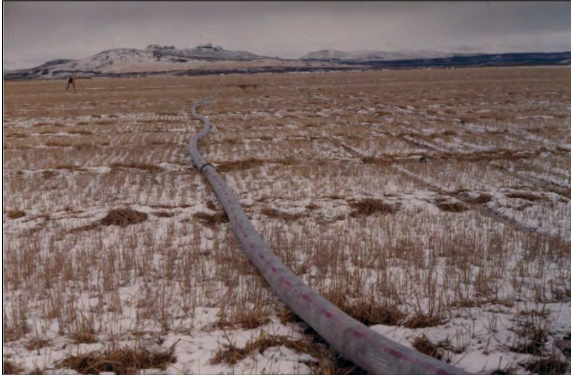
Figure 4.30 Closed drain construction at the Klamath Project, 1973. 227
