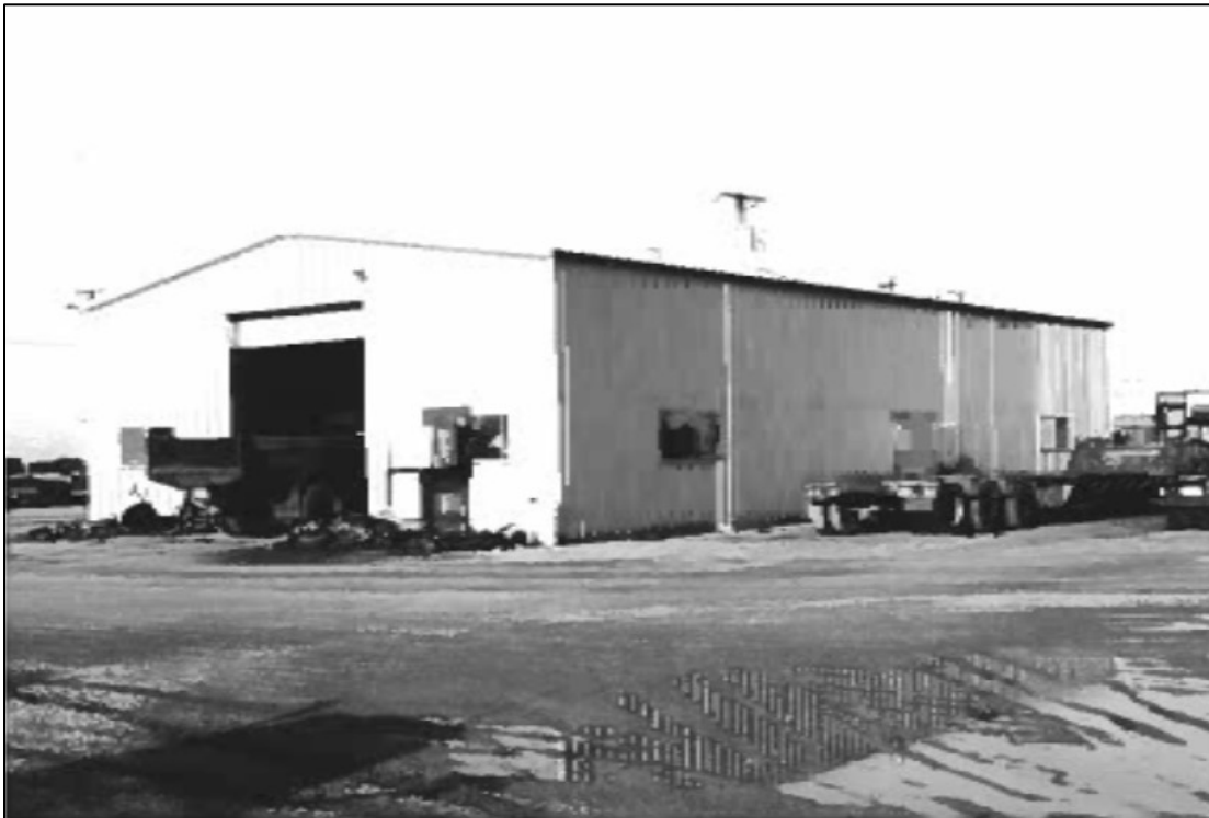
Figure 4.117 Corrugated metal garage WC-48 on the W.C. Altus Irrigation Project (Oklahoma) in 1991. 317
