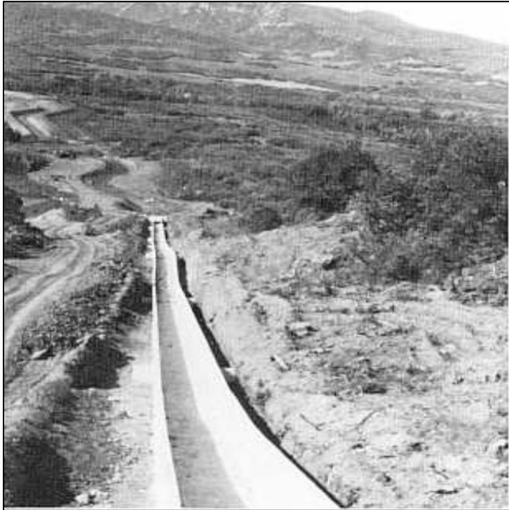
Figure 4.89 An open concrete chute on a steep slope. 284
