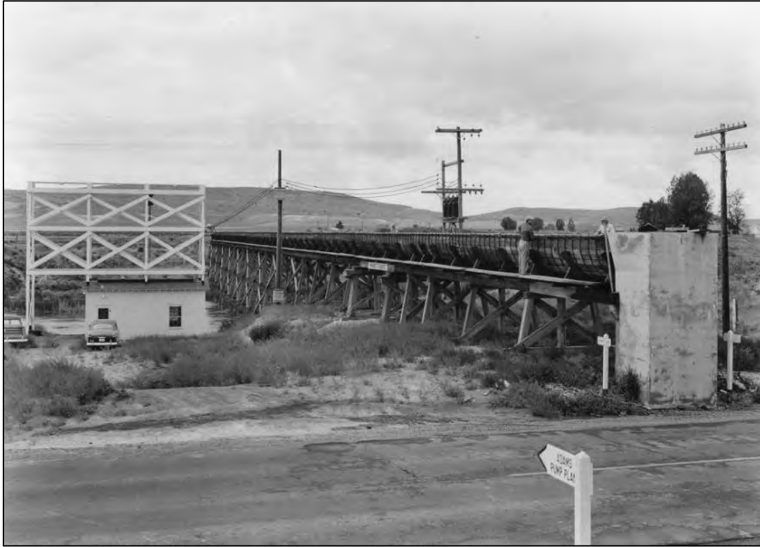
Figure 4.18 Adams pumping Plant (wood structure) on the Klamath Project, also showing flume and concrete siphon, 1950. 217
