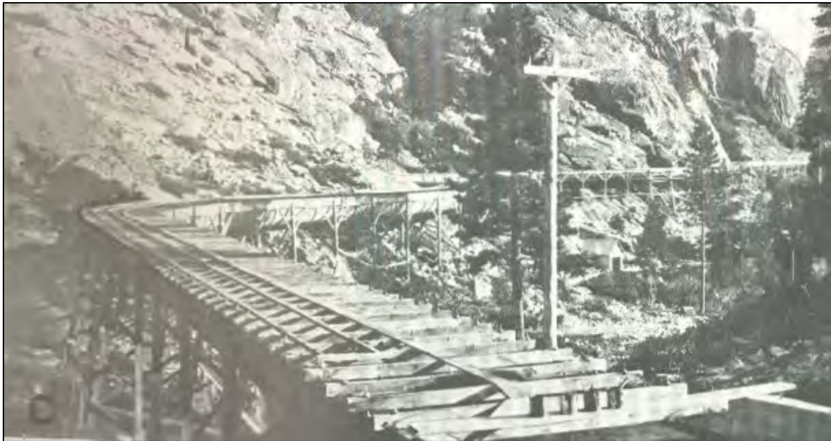
Figure 4.41 Wooden Tieton Bench Flume in the Yakima Project (Washington State). 235
