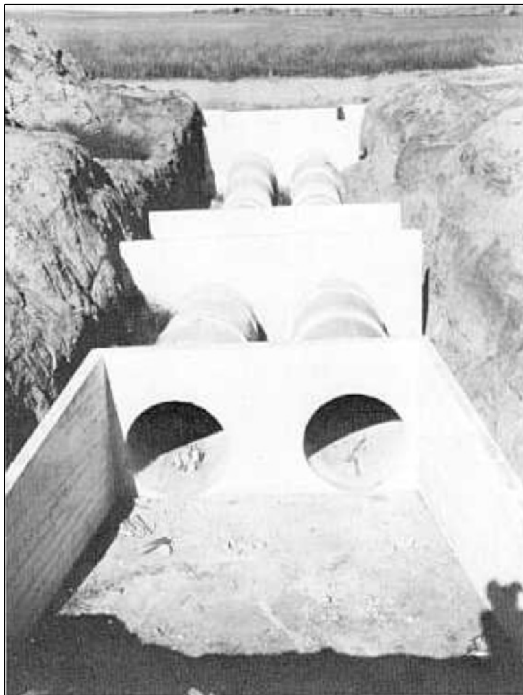
Figure 4.54 A precast concrete pipe culvert being installed on a Reclamation project. 247
