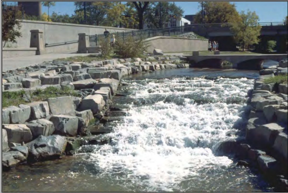
Figure 4.84 A reinforced concrete drop using rocks as the baffle on an unknown Reclamation project (California). 278
