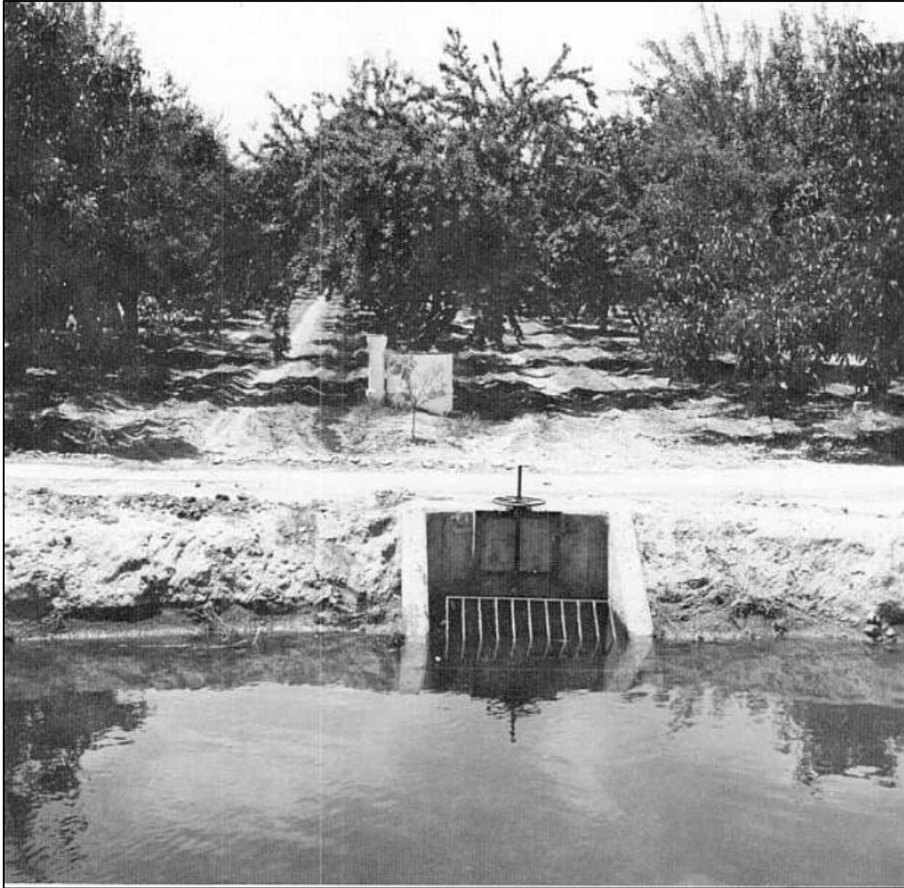
Figure 4.75 Concrete turnout with trash rack that permits water into the field from the lateral canal in an unknown Reclamation project. 267
