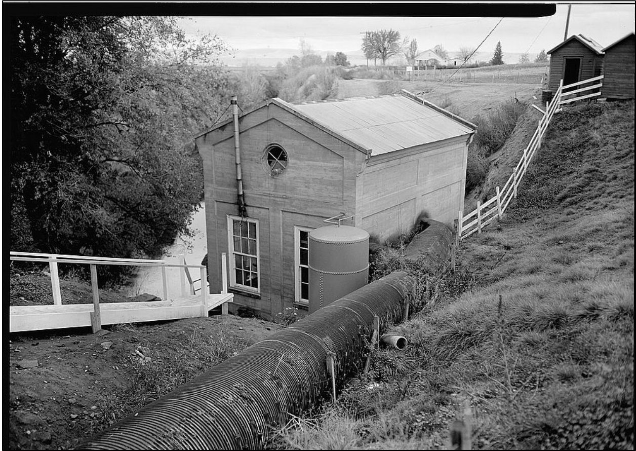
Figure 4.17 Concrete pumphouse on the Yakima Project. 215
