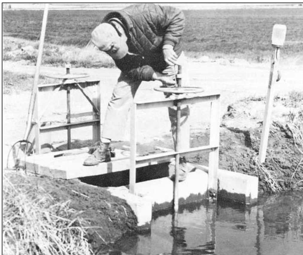
Figure 4.77 Constant Head Orifice Structure with the operator adjusting the headgate. 269
