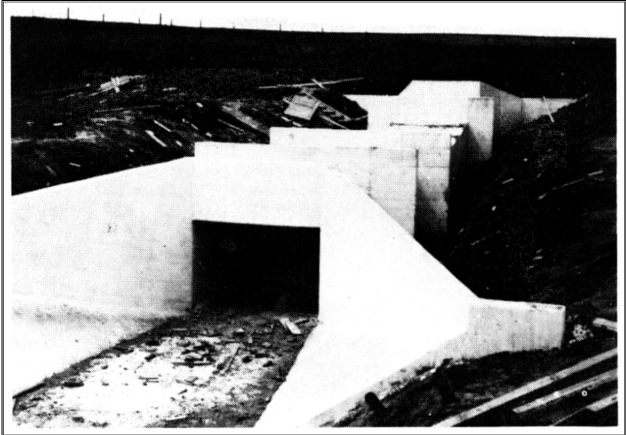
Figure 4.55 A precast concrete box culvert with a percolation collar during installation. 248
