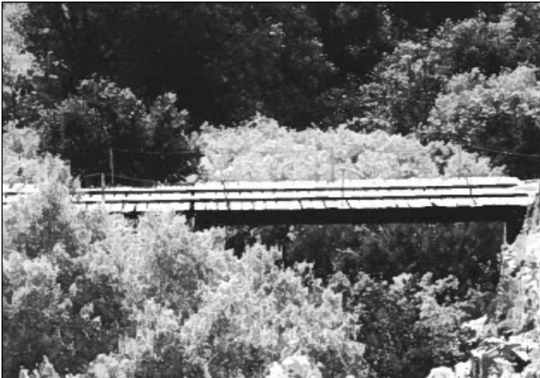
Figure 4.128 Steel constructed bridge over the Altus Dam Diversion Channel (Oklahoma). 328
