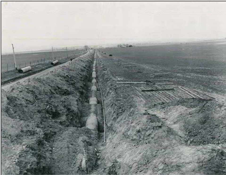
Figure 4.51 Steel pipeline being installed on the Lewiston Orchards Project (Idaho). 244
