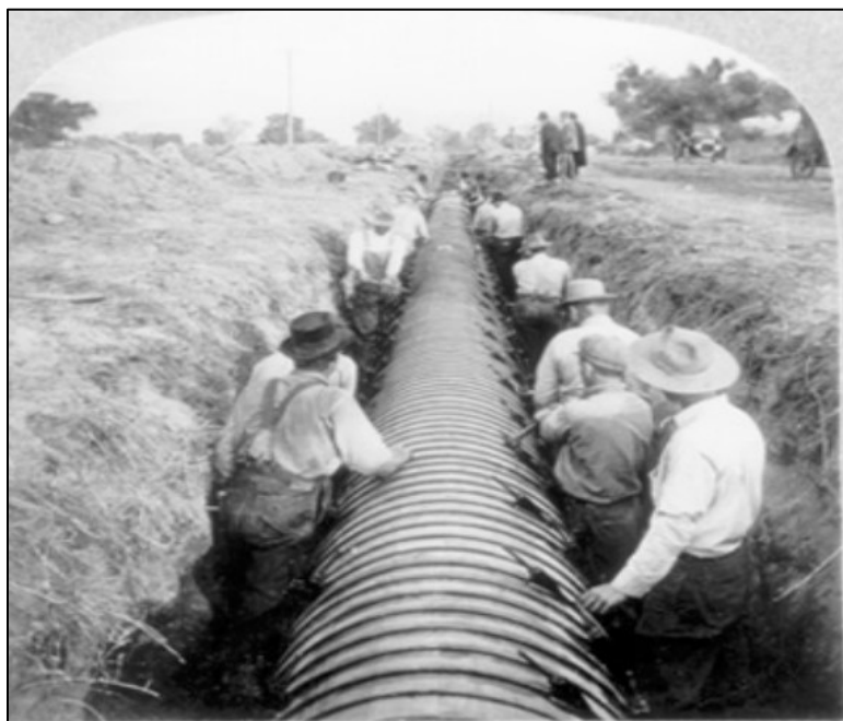
Figure 4.48 Wood stave construction on an early irrigation project (California). 241
