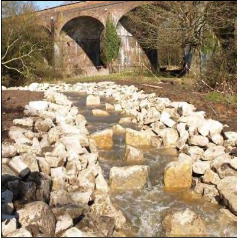
Figure 4.134 Fish bypass channel. 334
