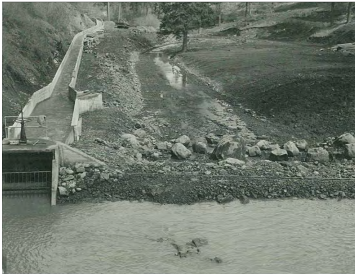
Figure 4.114 This image shows a number of features, including an iron headgate, a trash rack, a sand trap, and a flume as part of the main canal. The sand trap is the wide area behind the headgate where sand and debris can settle before the water enters the flume. The concrete feature on the right is the flushing gate where debris is flushed back into Sweetwater Creek (Idaho). 314
