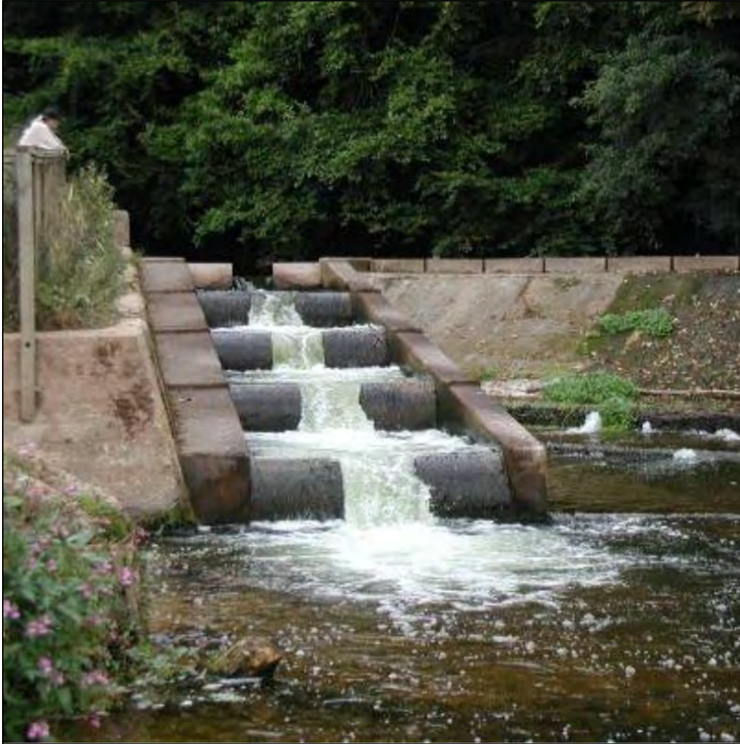
Figure 4.133 Pool and traverse style fish pass. 333
