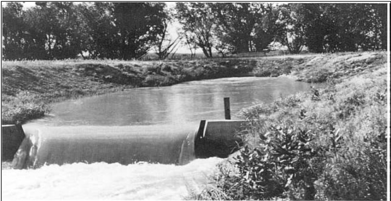
Figure 4.105 A Cipoletti weir with a measuring rod (at right) on an unknown Reclamation project. 304
