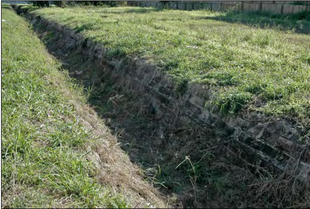
Figure 4.27 Brick-lined lateral canal in the Cameron County Irrigation District in the Lower Rio Grande Project (Texas). 224
