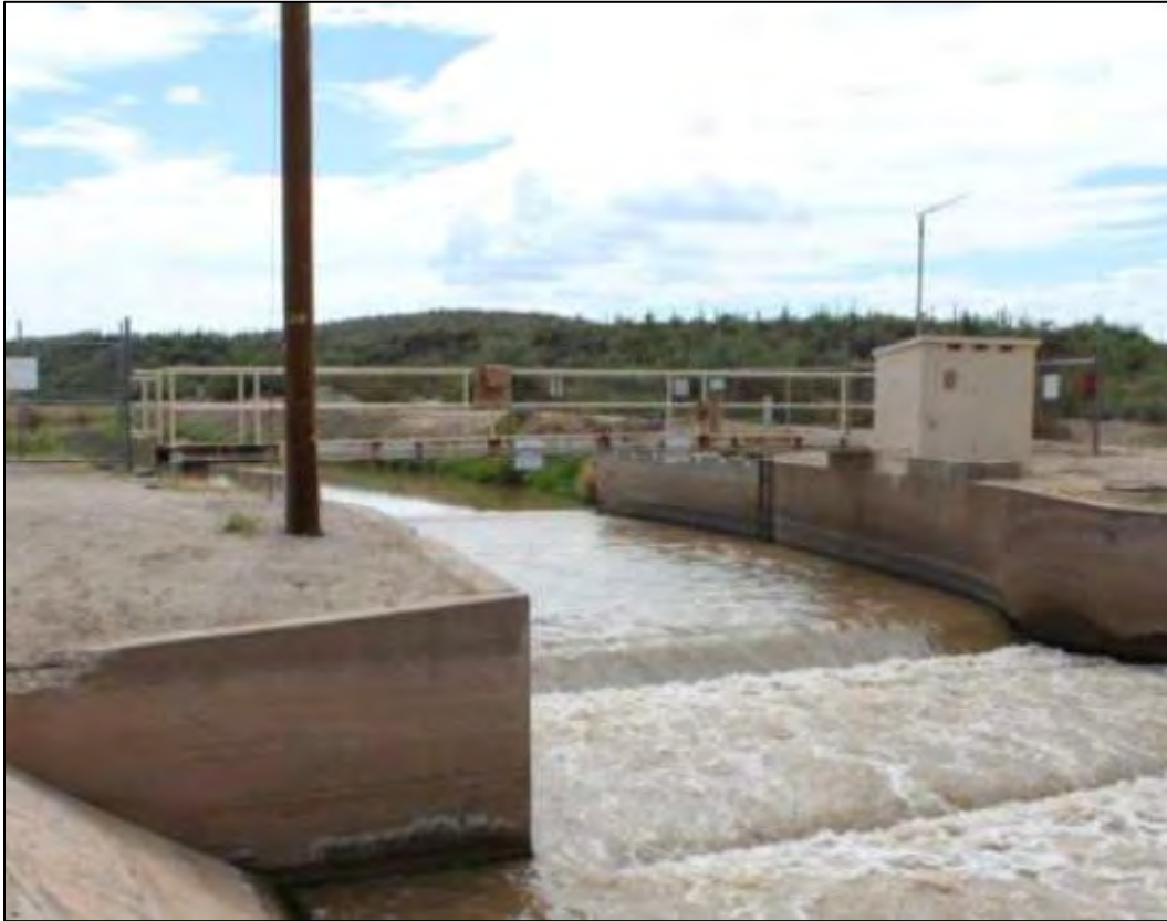
Figure 4.102 This photograph shows the Parshall flume, stilling well, and the gauging well on the right at the Florence Casa Grande Canal in the San Carlos Irrigation Project (Arizona). 301
