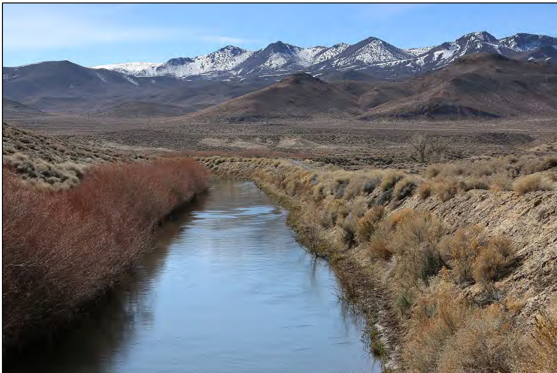
Figure 4.21 The unlined Truckee Main Canal (Nevada) in the Newlands Project was an early Reclamation project. Parts of the canal are still unlined. 221
