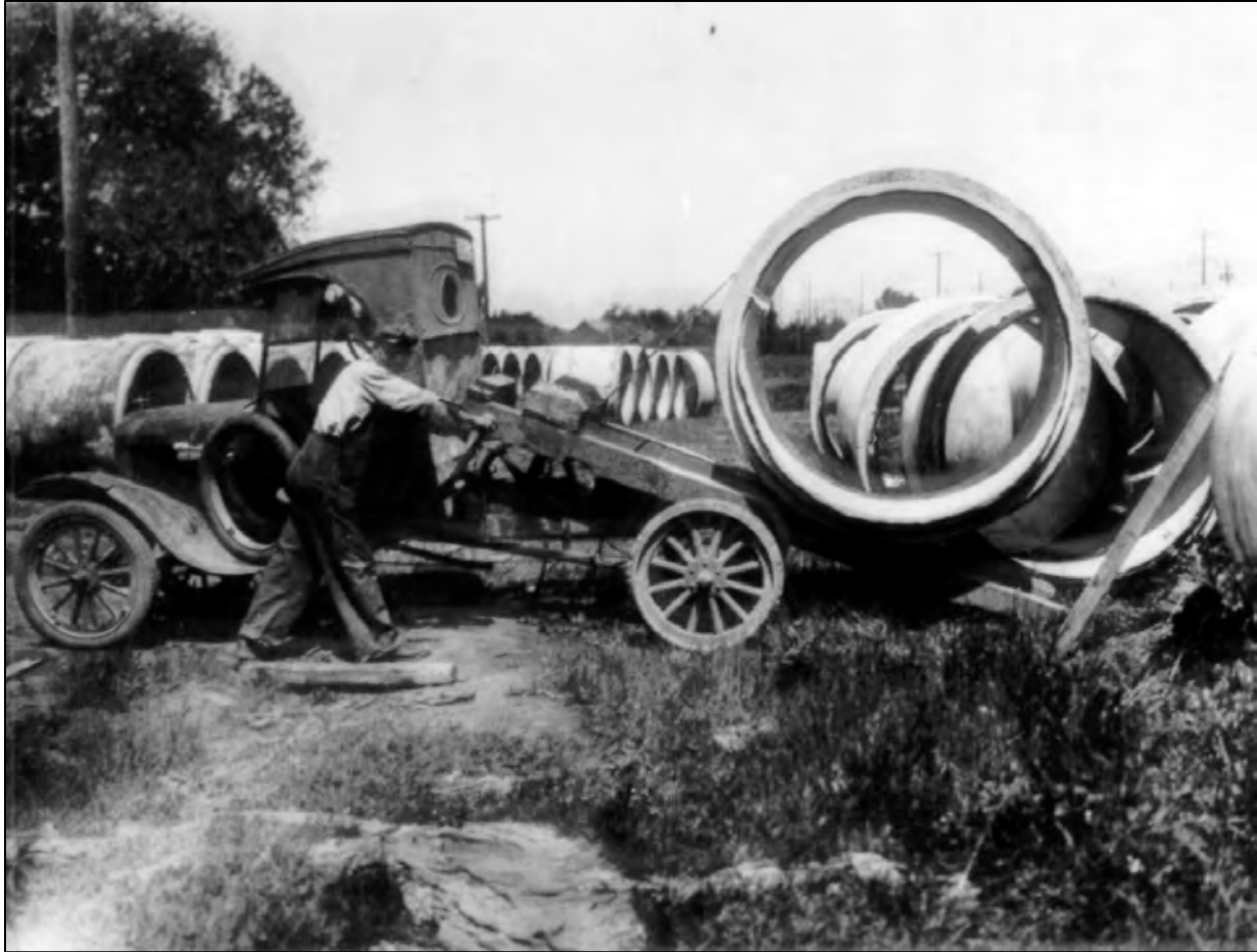
Figure 4.26 Yakima Project. Loading a 60-foot pipe weighing approximately 2.5 tons, 1929 (courtesy of Bureau of Reclamation).
