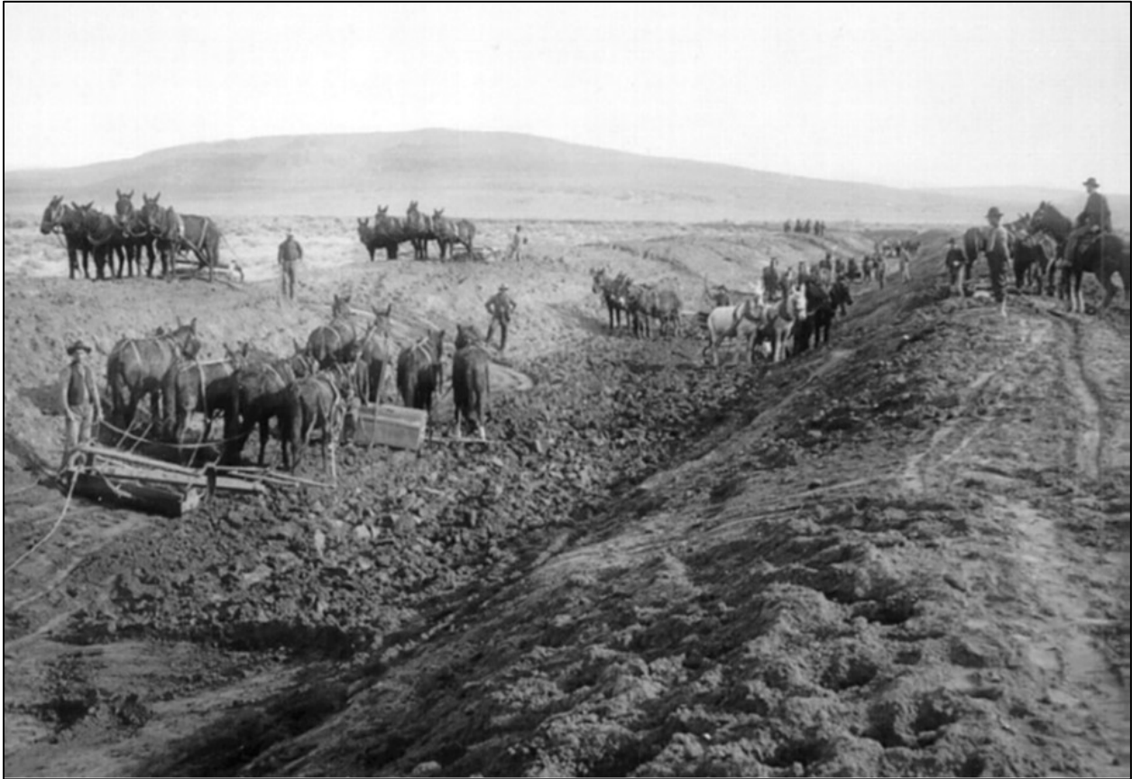
Figure 3.10 A c1912 photograph of the L-line lateral (Newlands Project, Nevada), a part of the water distribution system, under construction. 151
