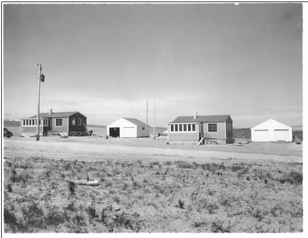
Figure 4.120 Housing projects for ditch riders within the Columbia River Basin Project (Washington). 320
