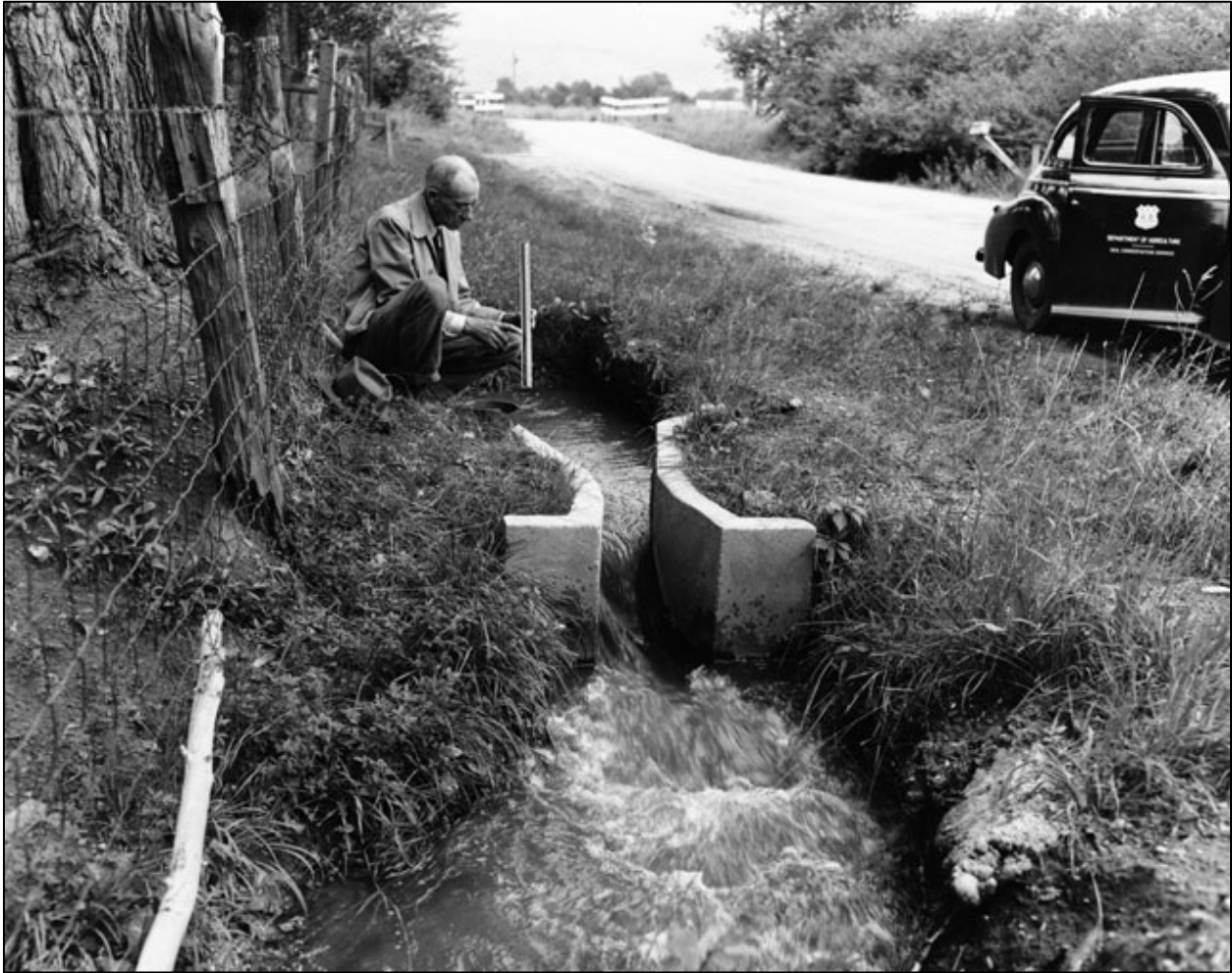
Figure 4.93 Measuring water flow at a concrete Parshall flume (Colorado). 290
