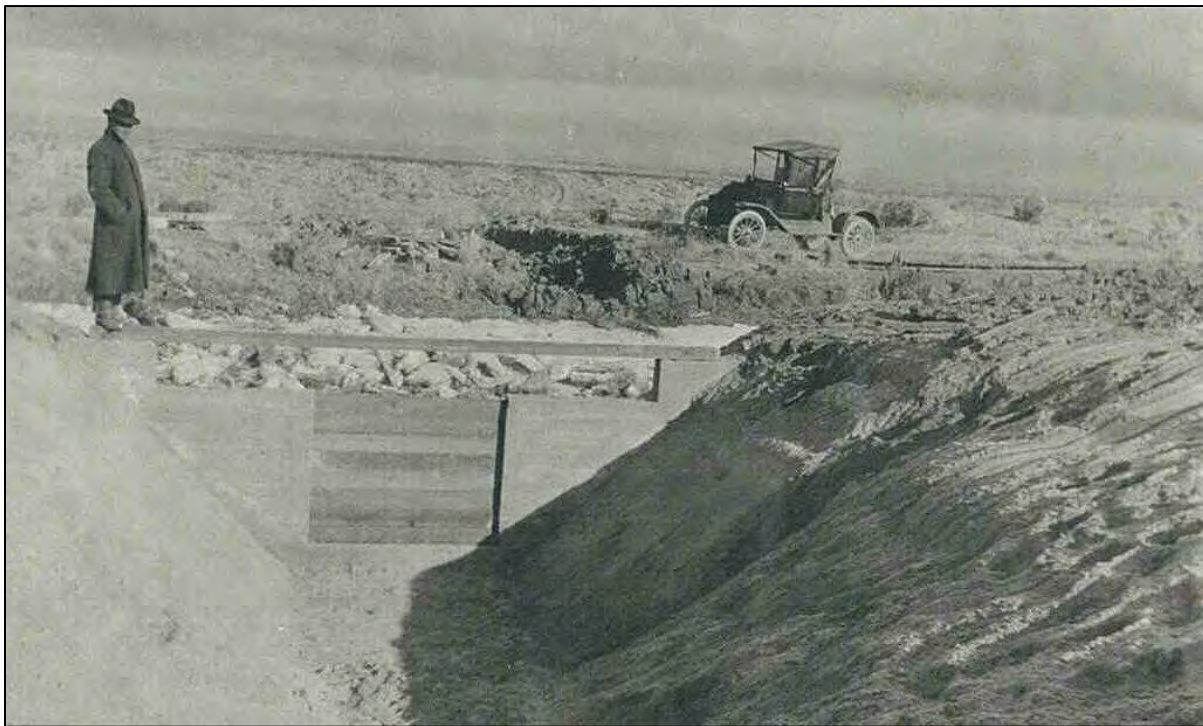
Figure 4.63 A good example of a wooden wasteway gate on the Minidoka Project (Idaho) c1916 (courtesy of Bureau of Reclamation).
