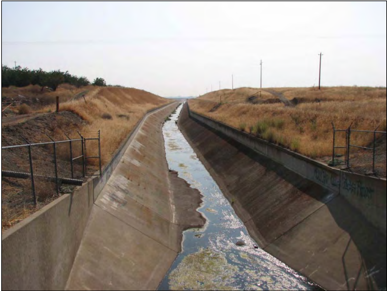
Figure 4.29 Concrete-lined section of the Newman Wasteway, Delta Mendota Canal, CVP (California). 226
