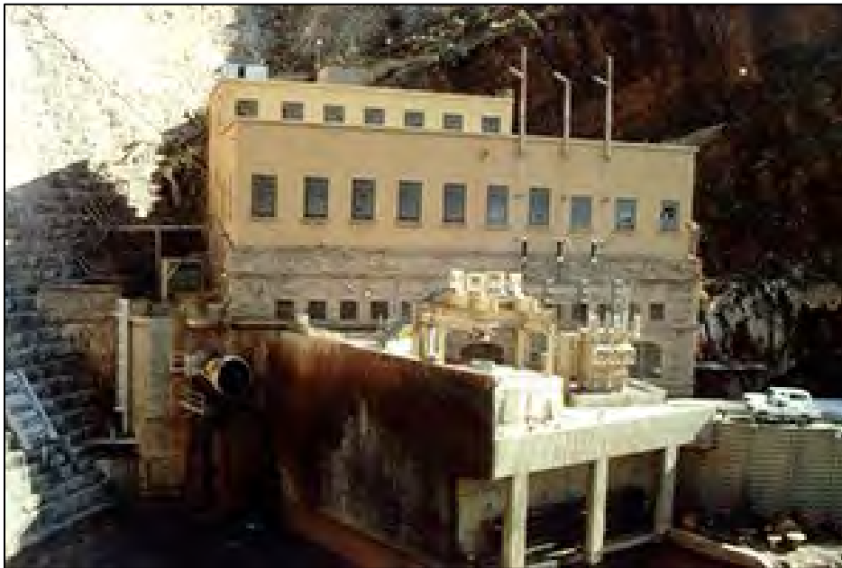
Figure 3.9 Theodore Roosevelt Powerplant (courtesy of Bureau of Reclamation).
