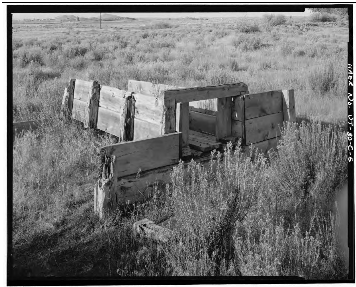
Figure 4.88 Example of a wood chute constructed early 1900 as part of irrigation canals in the Uinta Basin, Utah. 283
