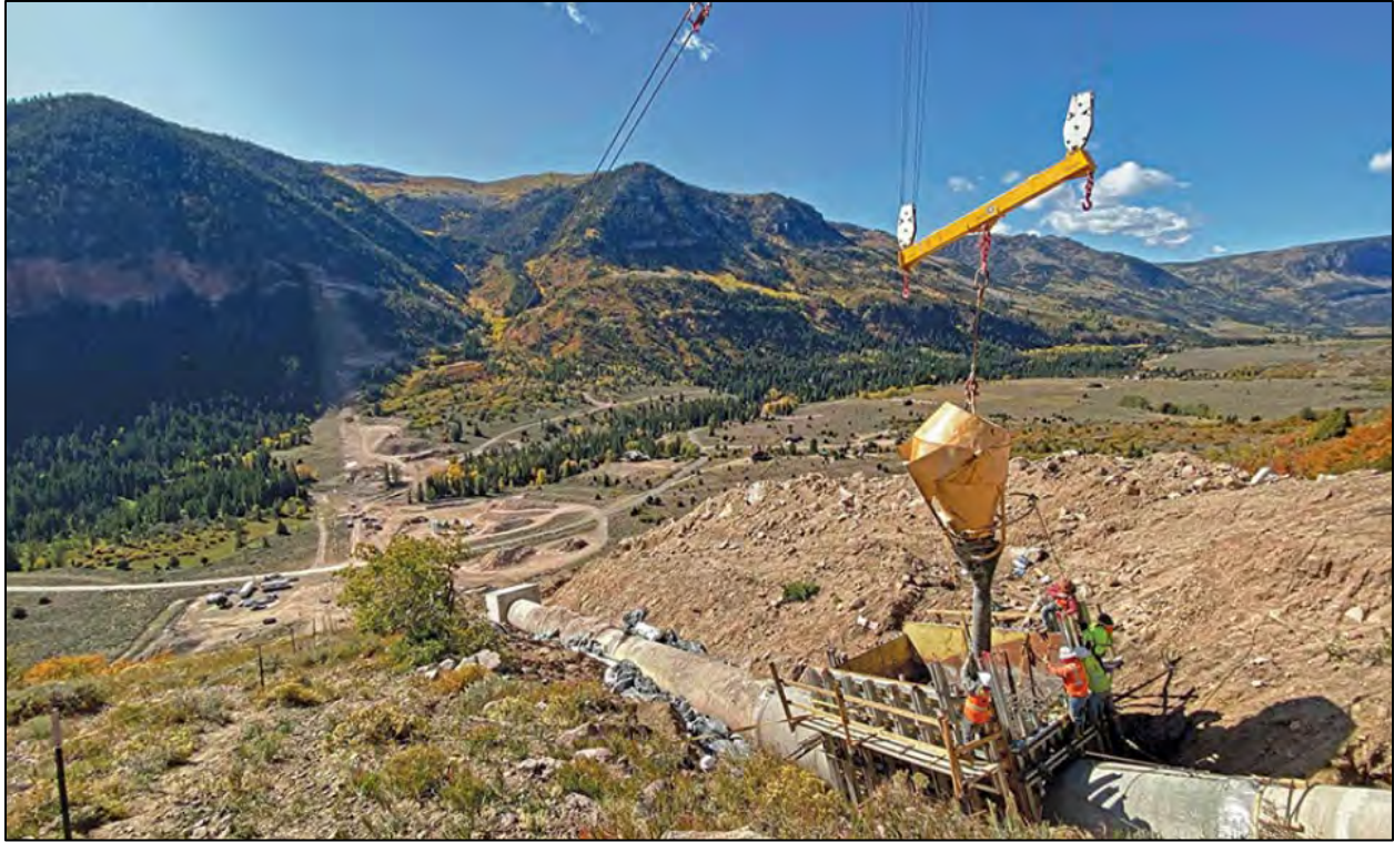
Figure 4.46 North Fork prestressed concrete siphon on the Strawberry Valley Project (Utah). 239
