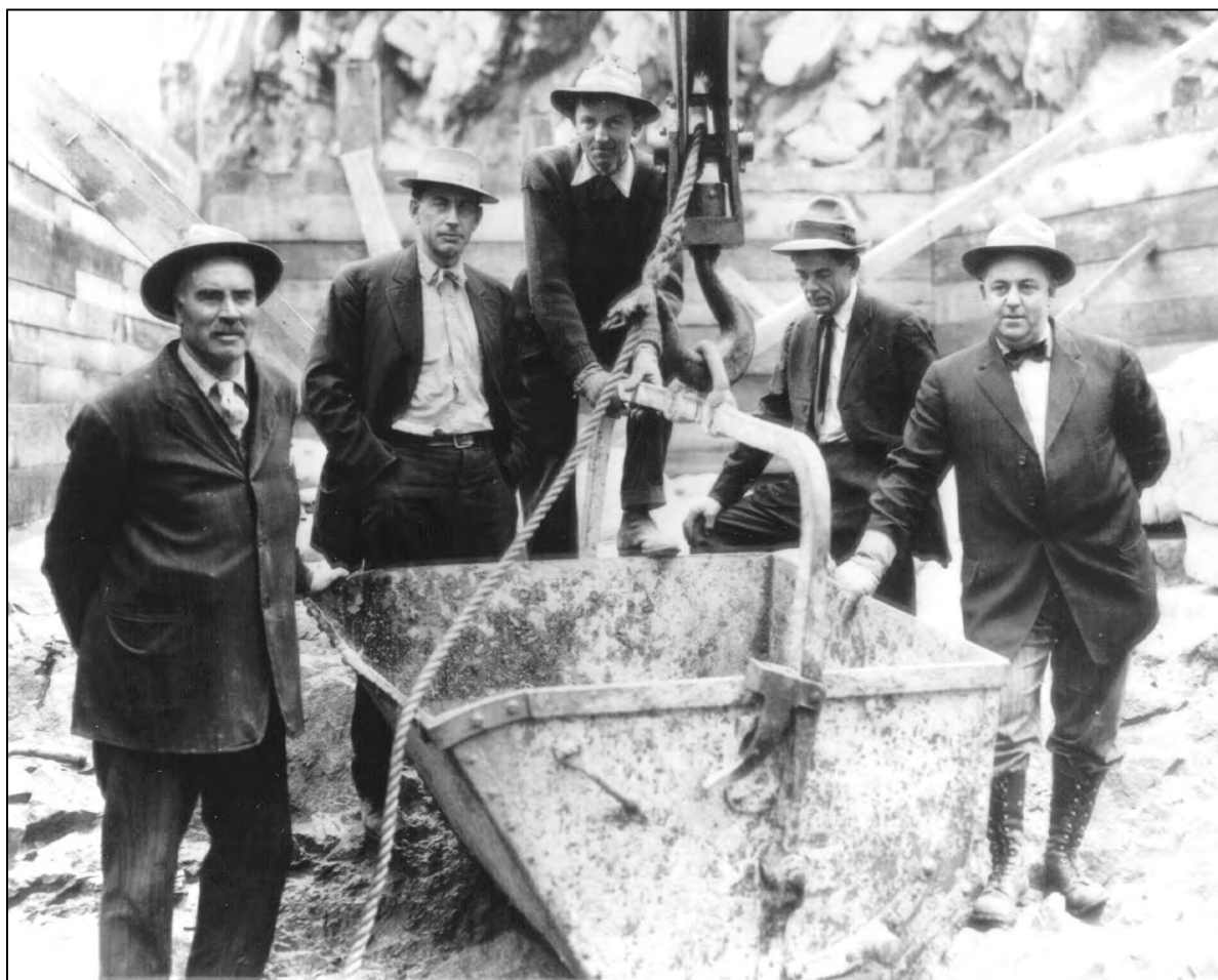
Figure 3.13 The first bucket of concrete ready to be poured on the Arrowrock Dam site on the Boise River. James Munn, spt of const.; A.B. Mayhew, assist. resident engineer; Frank Crowe, shift boss who later worked at Hoover Dam, Shasta Dam, and Deadwood Dam; John Beemer, inspector; and C.H. Paul, resident engineer, 1912. 162
