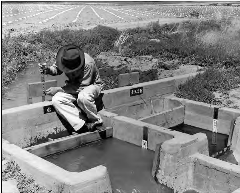
Figure 4.106 Ditch rider delivering water through a weir to a farm ditch. The scale in the photograph indicates 0.51 second feet of water going through the weir to a farm on the Yakima Project (Washington State) (courtesy of Bureau of Reclamation).
