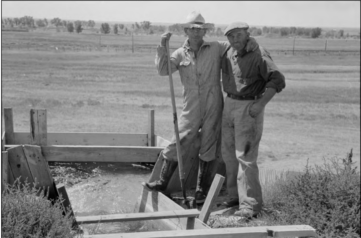
Figure 4.13 This photo shows an early wooden box weir method of measuring water by adjusting the water flow through the gate. These are rarely found on Reclamation projects and are long outdated. 210
