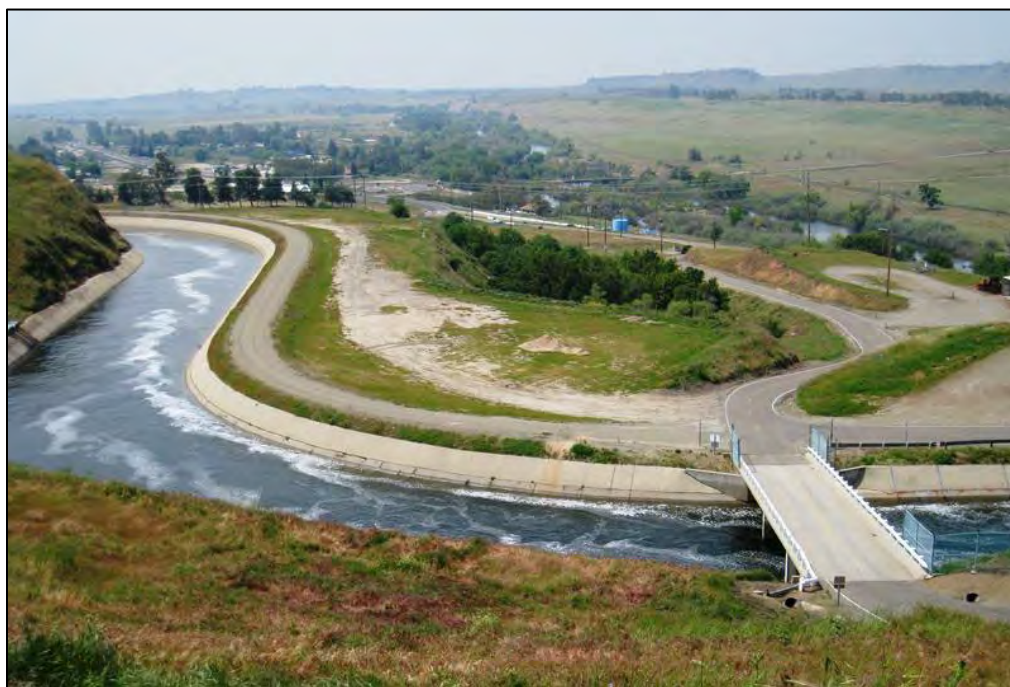
Figure 4.24 An unlined section of the All-American Canal (Arizona), partly lined and partly unlined in the Boulder Canyon Project, was completed in 1942 (courtesy of Bureau of Reclamation).
