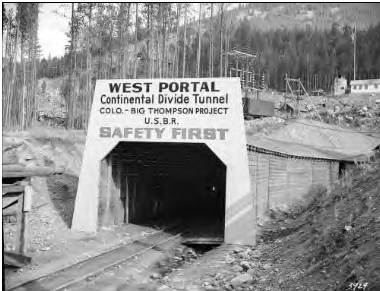
Figure 4.33 The entrance to the Alva B. Adams Tunnel on the west side of the Continental Divide in the Colorado Big-Thompson Project (Colorado) (courtesy of Denver Public Library online).
