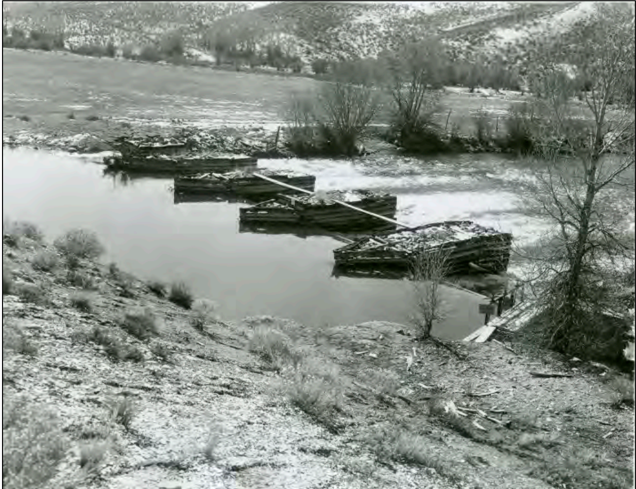
Figure 4.5 A wooden pile and bulkhead on the Blue River in the Colorado—Big Thompson Project, Colorado (courtesy of Bureau of Reclamation).
