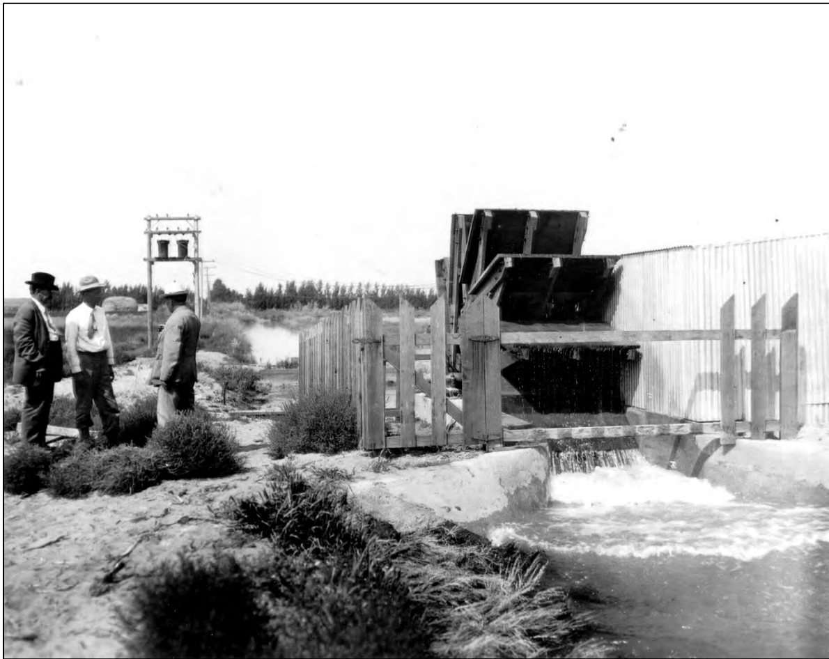
Figure 3.11 Scoop wheel electrically operated. 60% efficient. Lifting water 3 1/2 feet, to irrigate 800 acres, 1914 (courtesy of Bureau of Reclamation).
