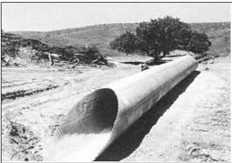
Figure 4.56 Corrugated steel pipe used at a road crossing on an unknown Reclamation project. 249
