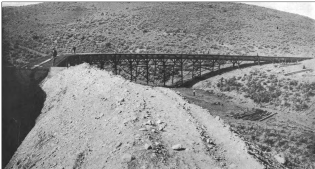
Figure 4.38 A steel flume on steel trusses in the Tieton Distribution System on the Yakima Project (Washington State). 232
