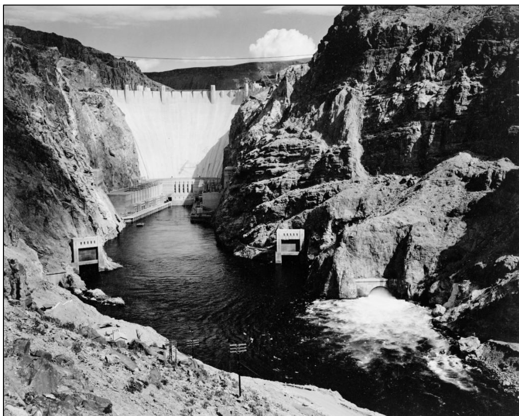
Figure 2.7 The completed Boulder (Hoover) Dam, initiated in 1929 and completed in 1935, the largest dam in the world at that time. 44
