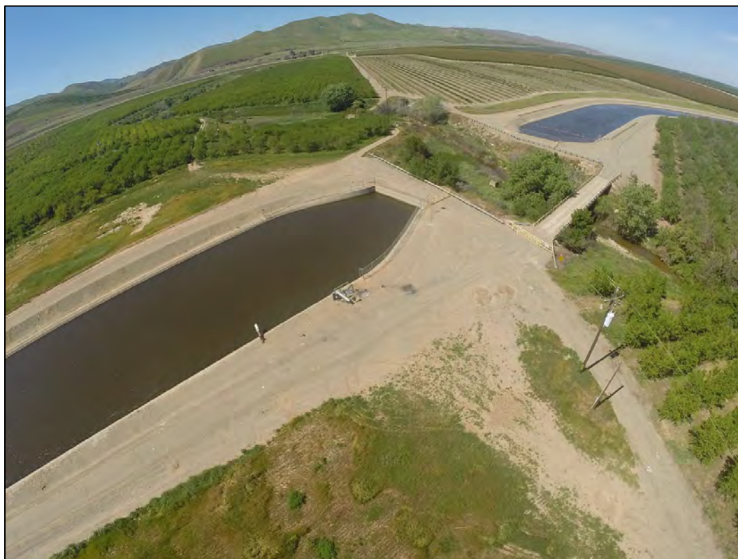
Figure 4.45 Siphon under Patterson Creek on the Delta Mendota Canal, CVP (California) (courtesy of Bureau of Reclamation).
