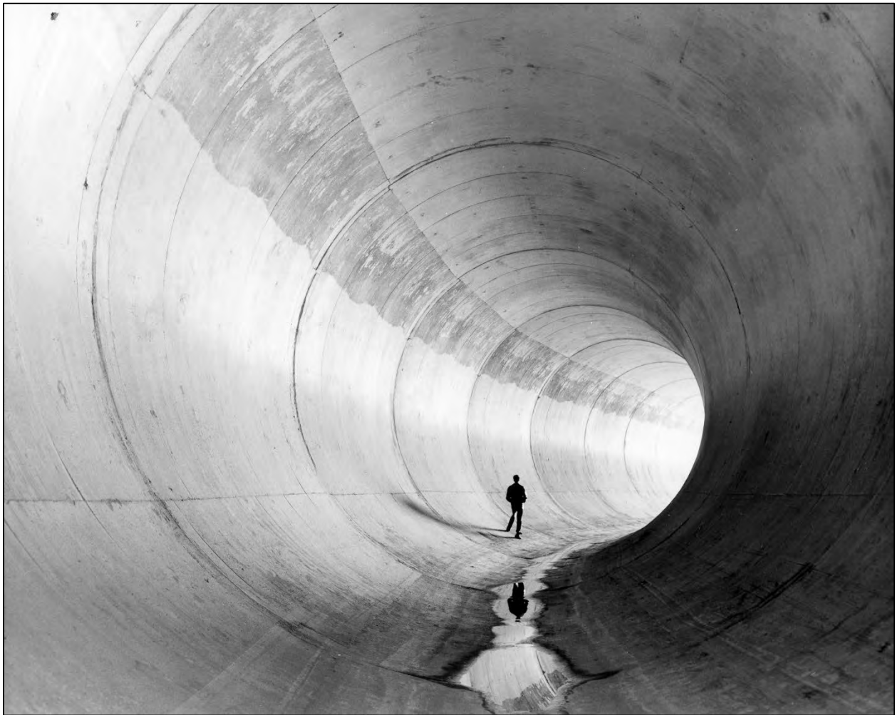
Figure 5.4 Soap Lake Siphon on the Columbia Basin Project (Washington), 1952. 365
