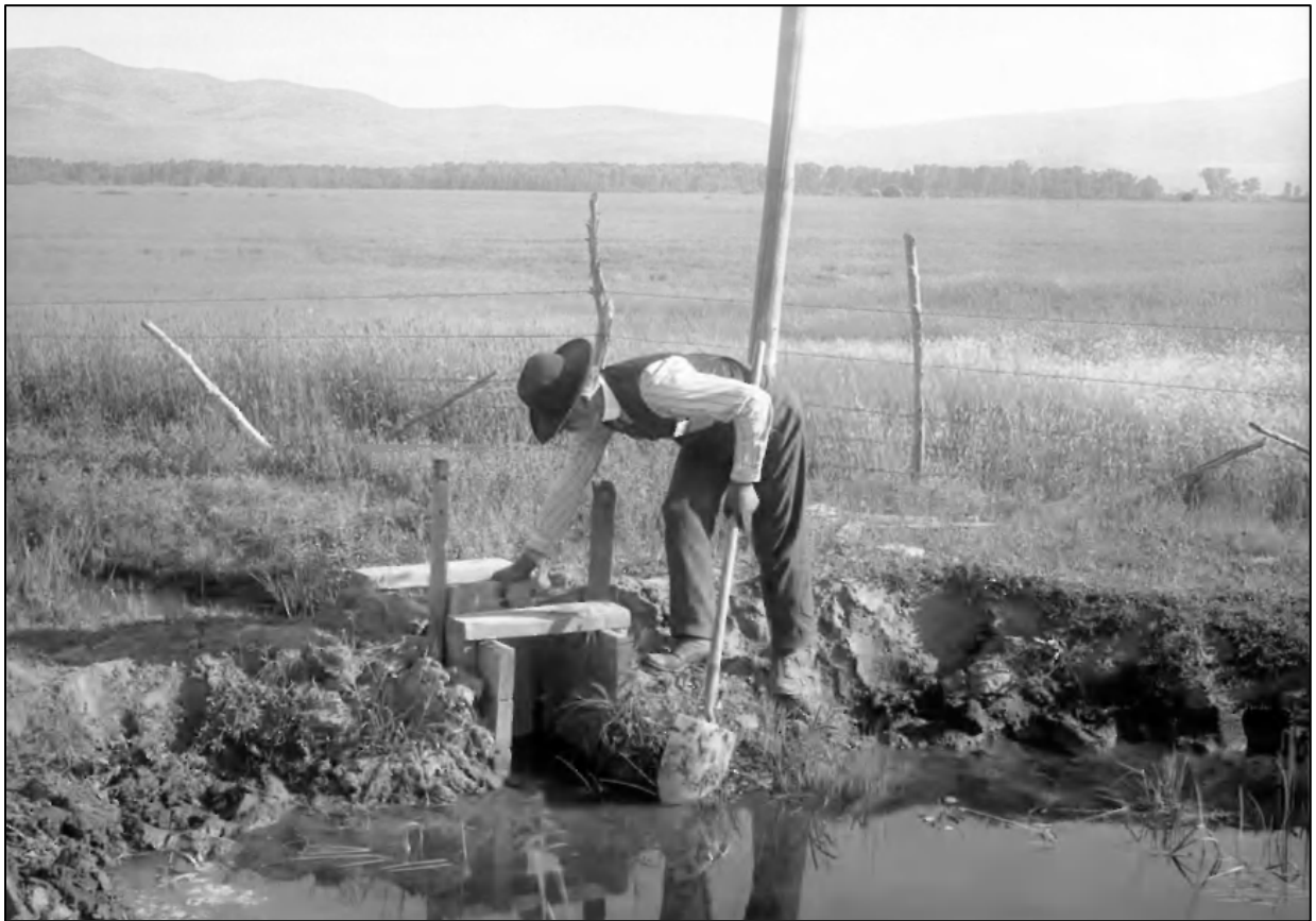
Figure 4.74 Simple hand-operated wooden turnout gate on an unknown Reclamation project (Colorado). 266
