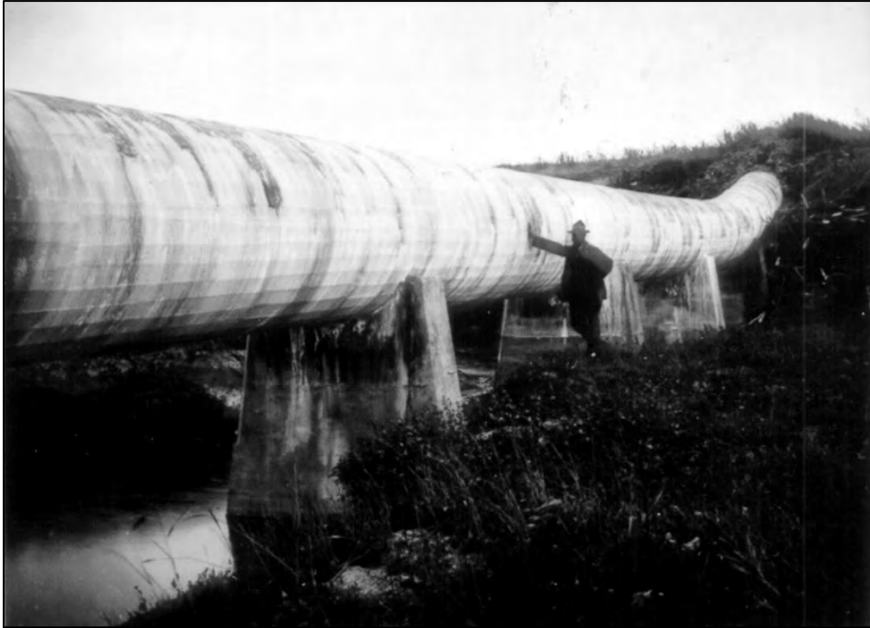
Figure 4.50 Cement pressure pipe on the Sun River Project, Montana, 1908. 243
