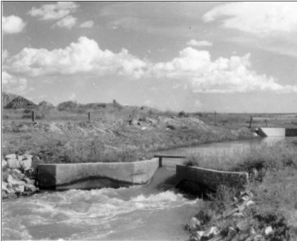
Figure 4.96 A Parshall flume modified to the canal size, emptying water into a stilling basin on an unknown Reclamation project. 295
