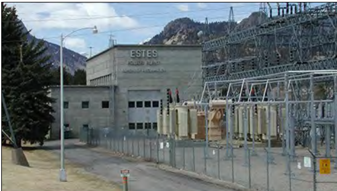
Figure 4.124 An example of a larger powerplant is the Estes Powerplant on the Colorado-Big Thompson Project (Colorado). 324
