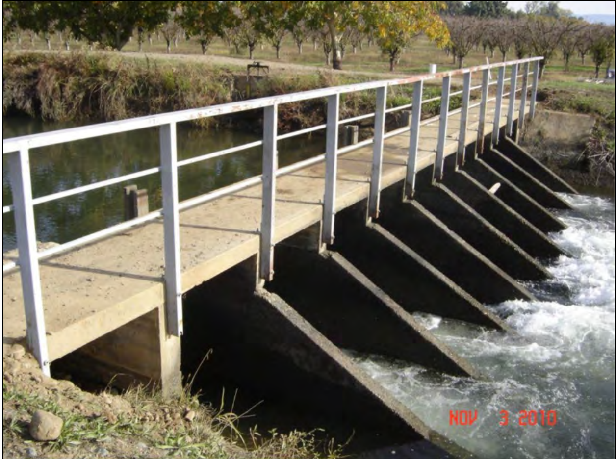
Figure 4.12 Concrete weir with foot bridge on Sutter Butte Main Canal (State of California irrigation project). Note the turnout and orchard in the background. 209
