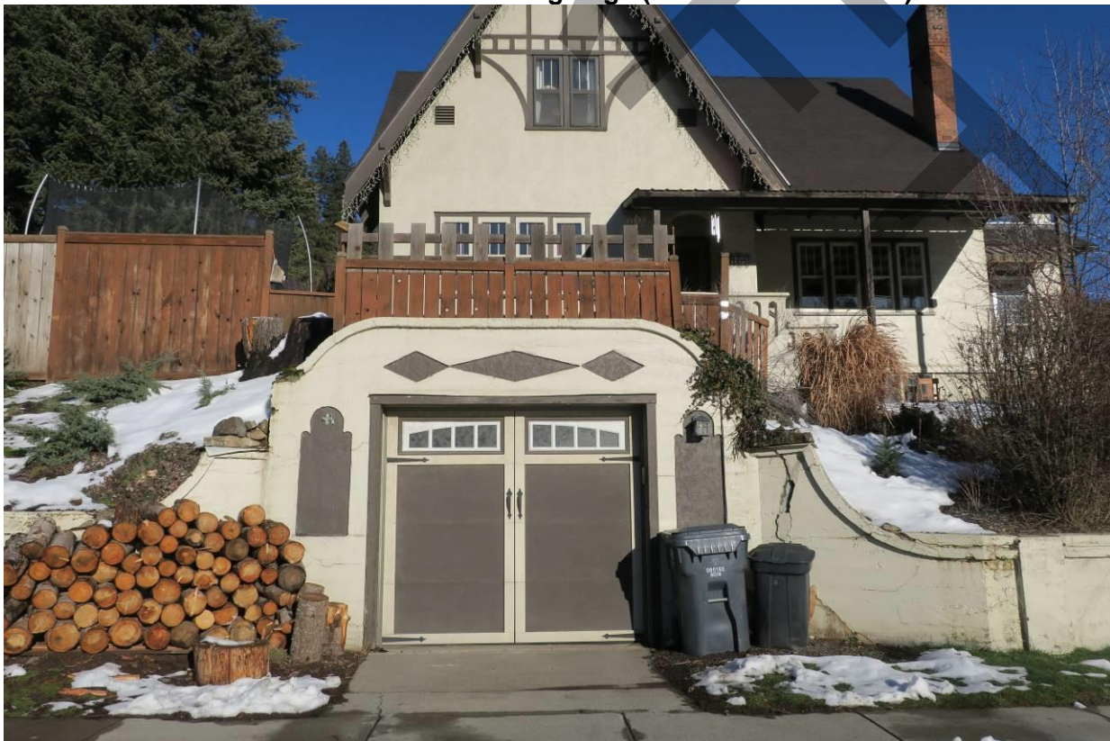
Photo 6: View Northeast of garage (southwest elevation)
