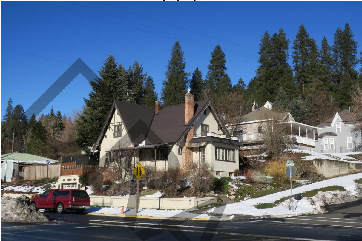
Photo 1: View North of property from South Main Street
