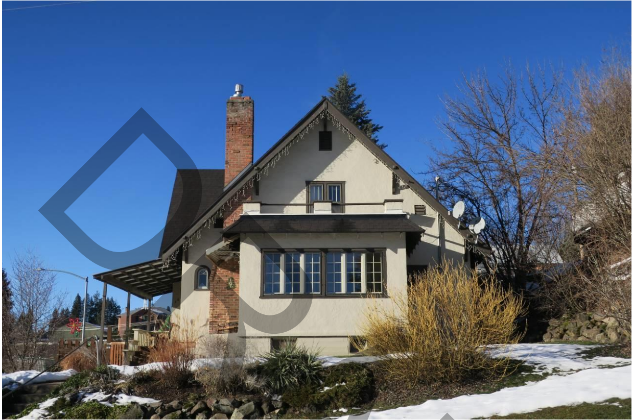
Photo 3: View Northwest of Southeast elevation
