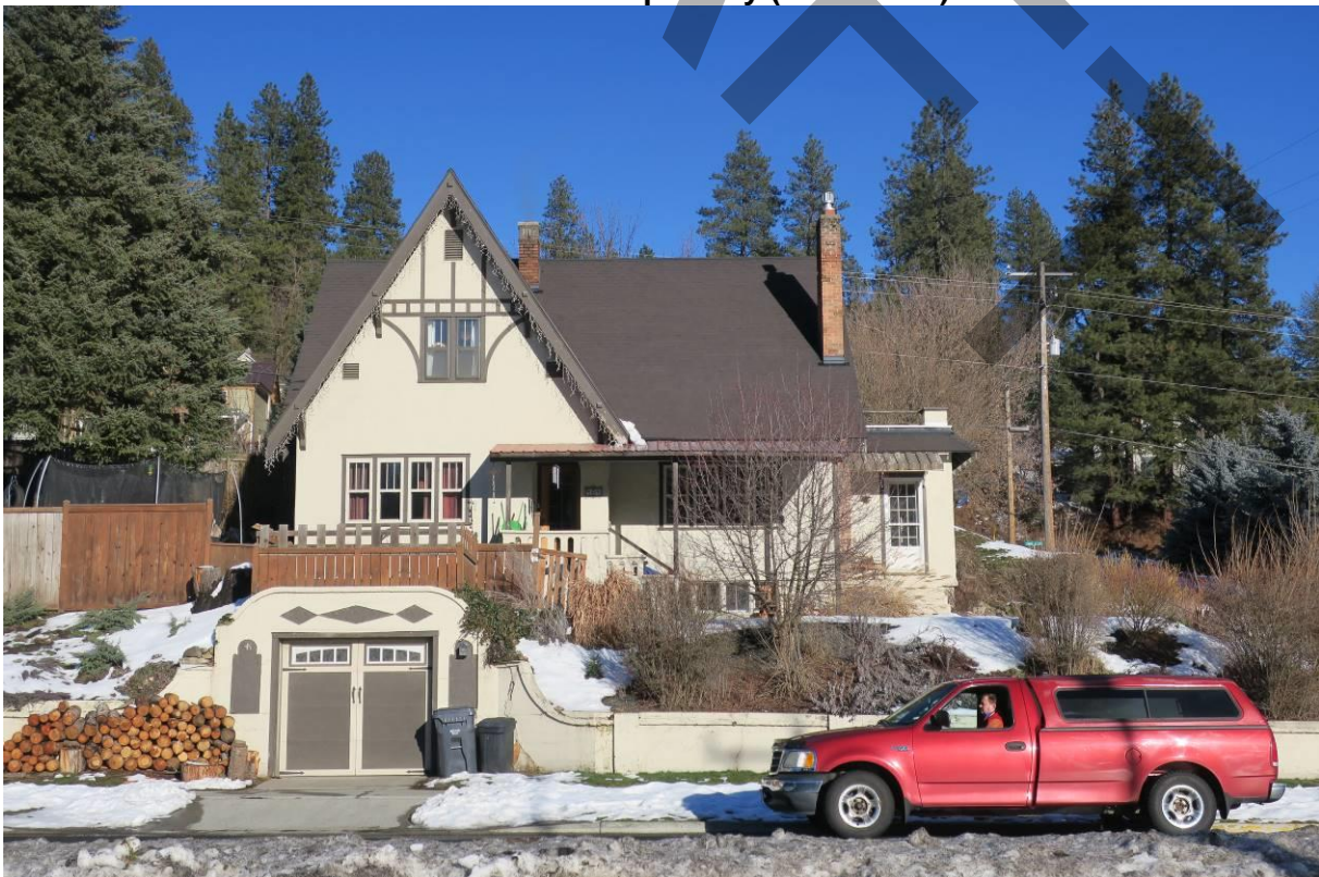
Photo 2: View Northeast of primary (southwest) elevation
