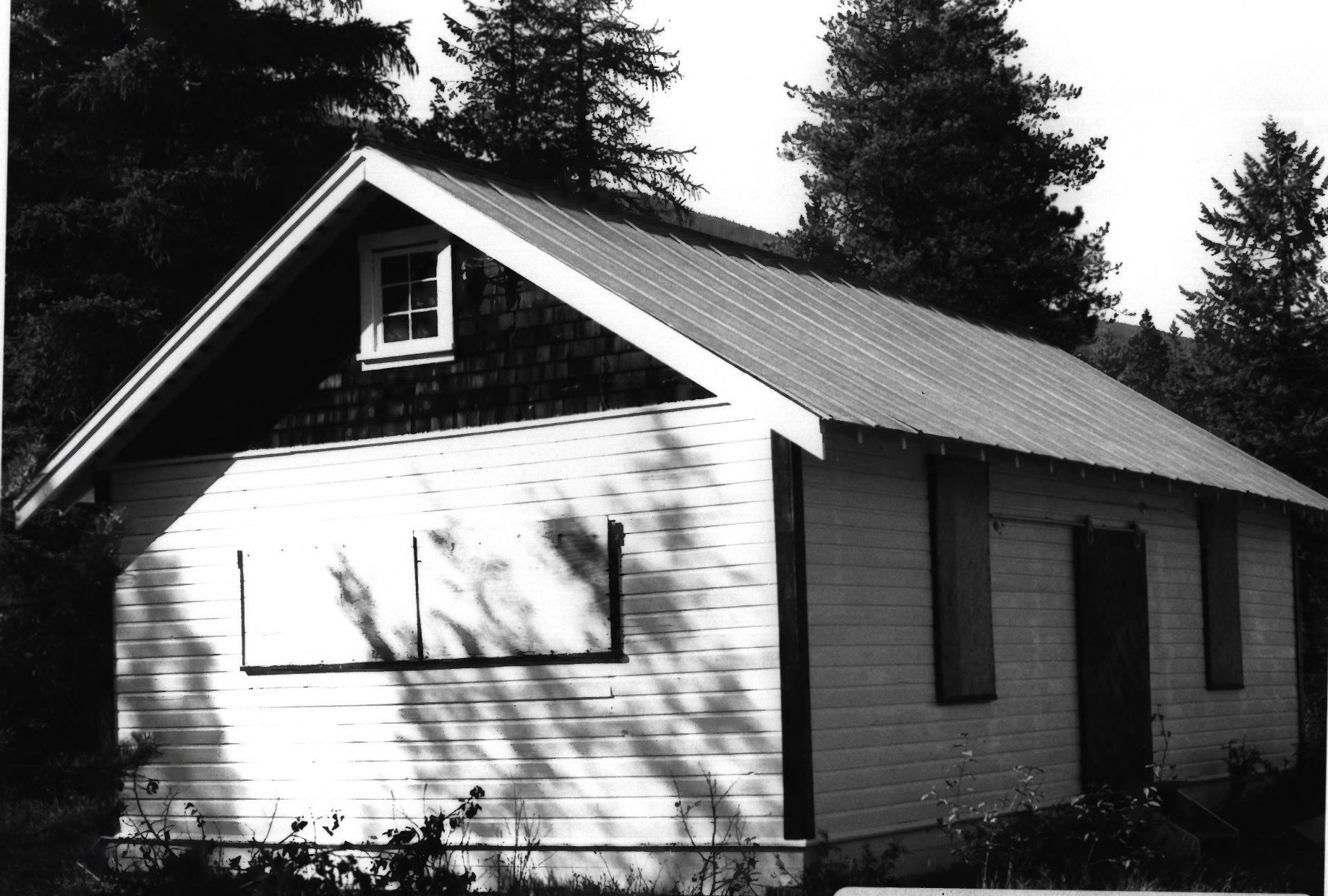
Snyder Historical District Warehouse/Office Facing Northwest
