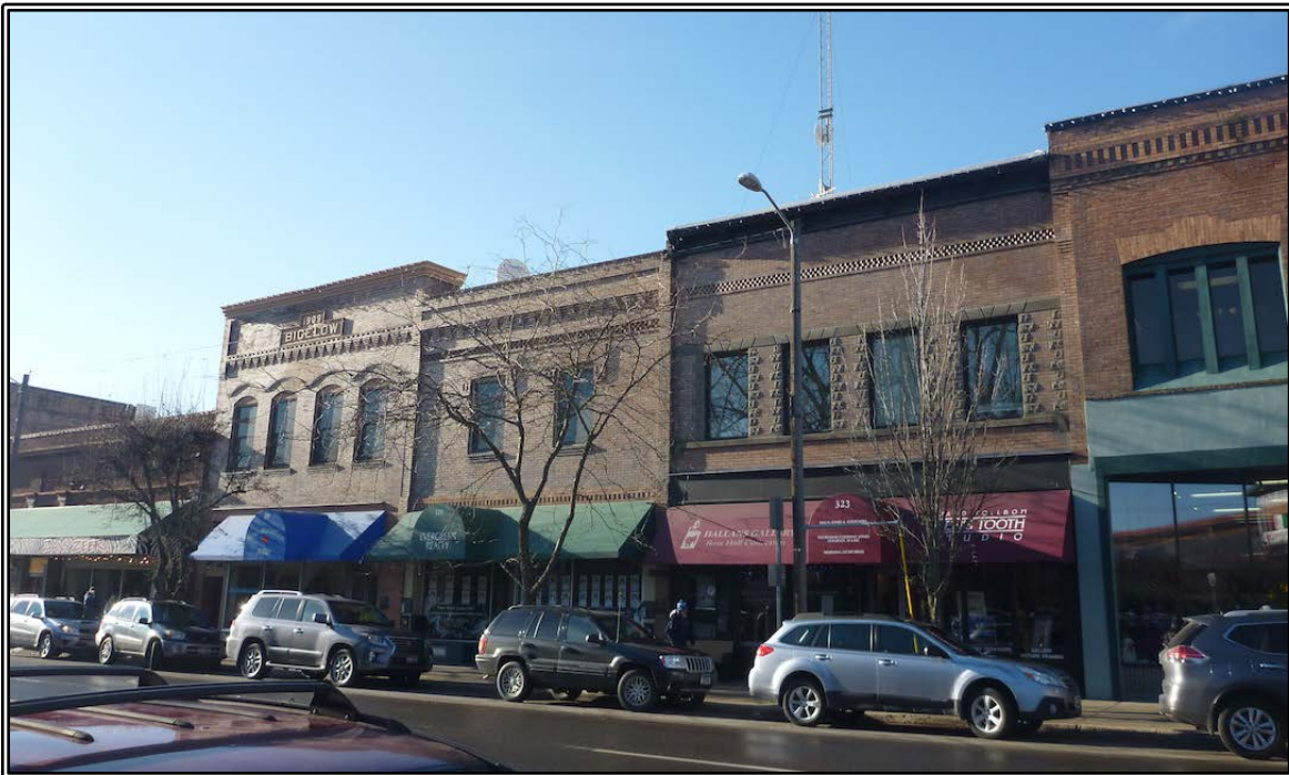
Figure 10: Contemporary south-southwest overview along First Avenue from Cedar Street
