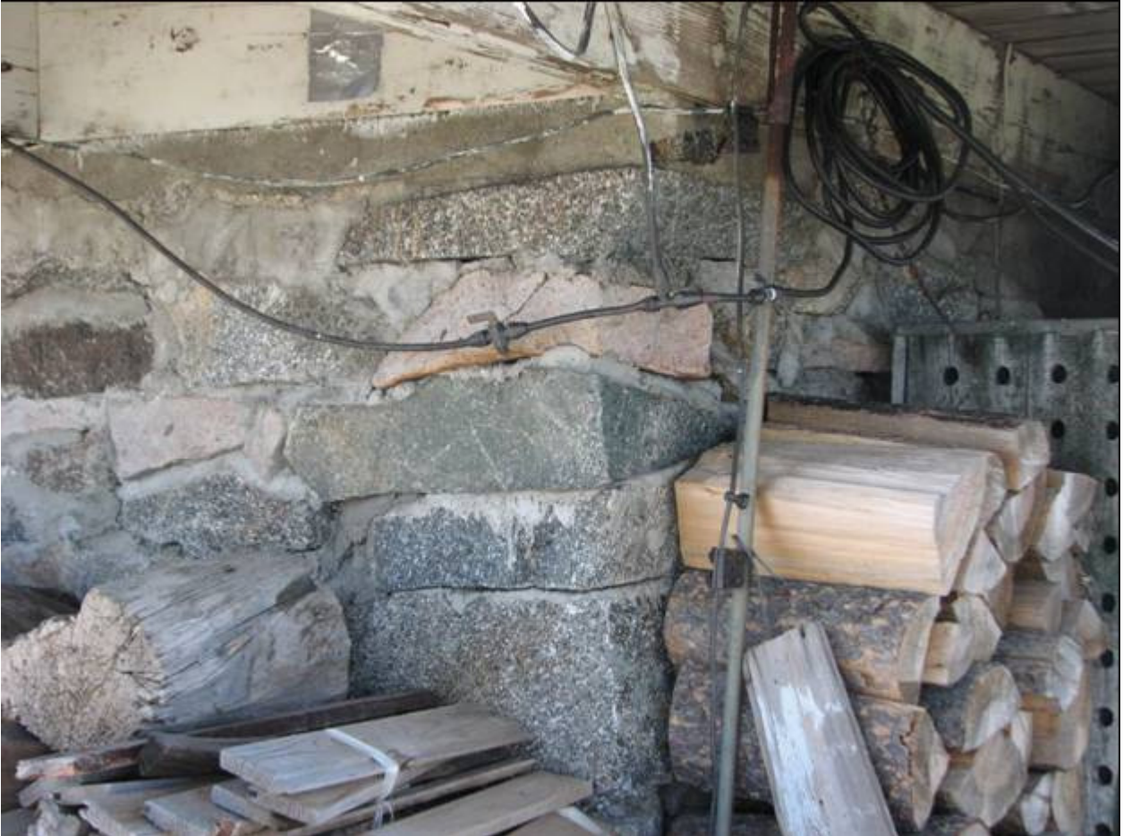
ID_IdahoCounty_Salmon Mountain Lookout_0004. Detail of the mortared stone foundation of lookout.
