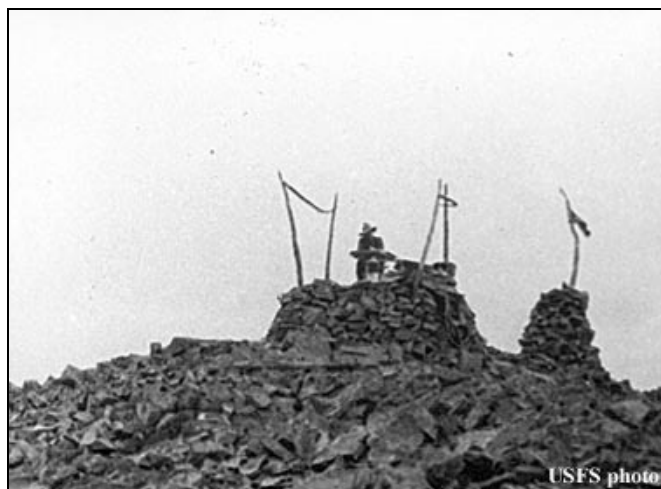
Figure 1. 1922 photo of the Salmon Mountain lookout improvements.
