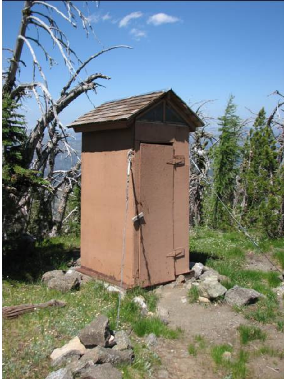
ID_IdahoCounty_Salmon Mountain Lookout_0008. Looking northwest to the south and east (front) walls of the outhouse.
